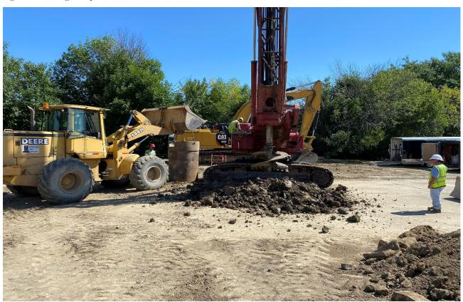
Figure 2 – Lowering 55FT I-beam Pier into Drilled Hole
