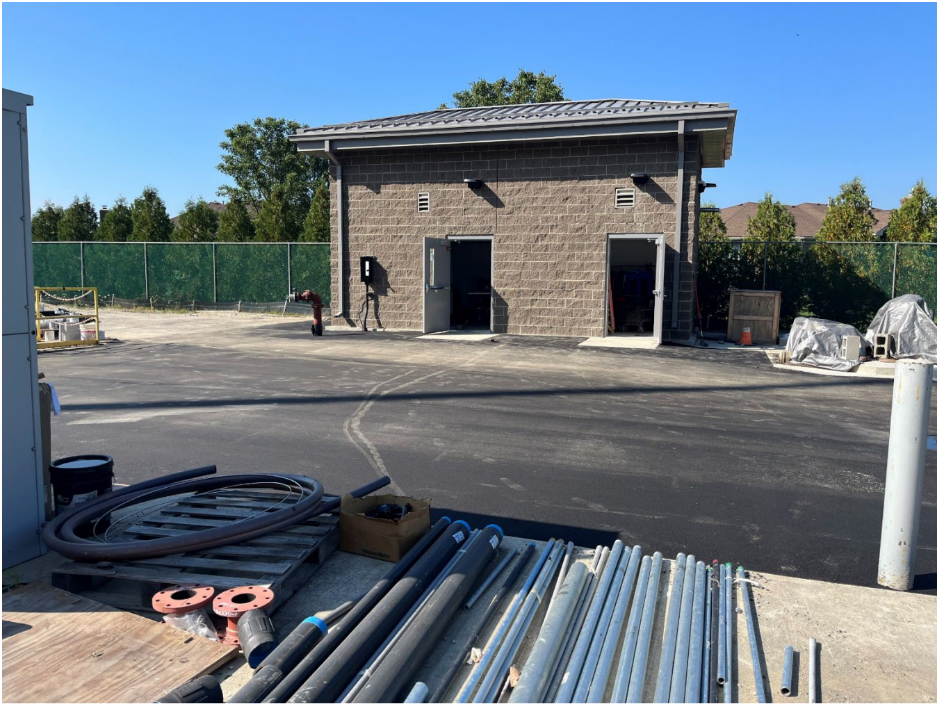
Figure 15 – NGI Chemical Injection Building
