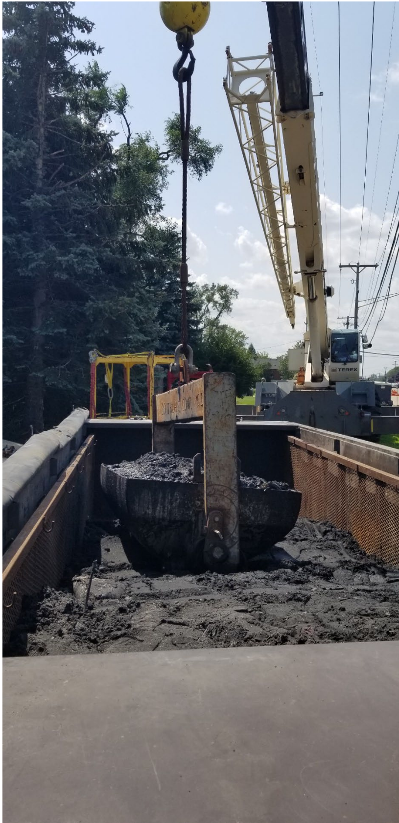
Figure 6 – Debris Removal at MH-05
