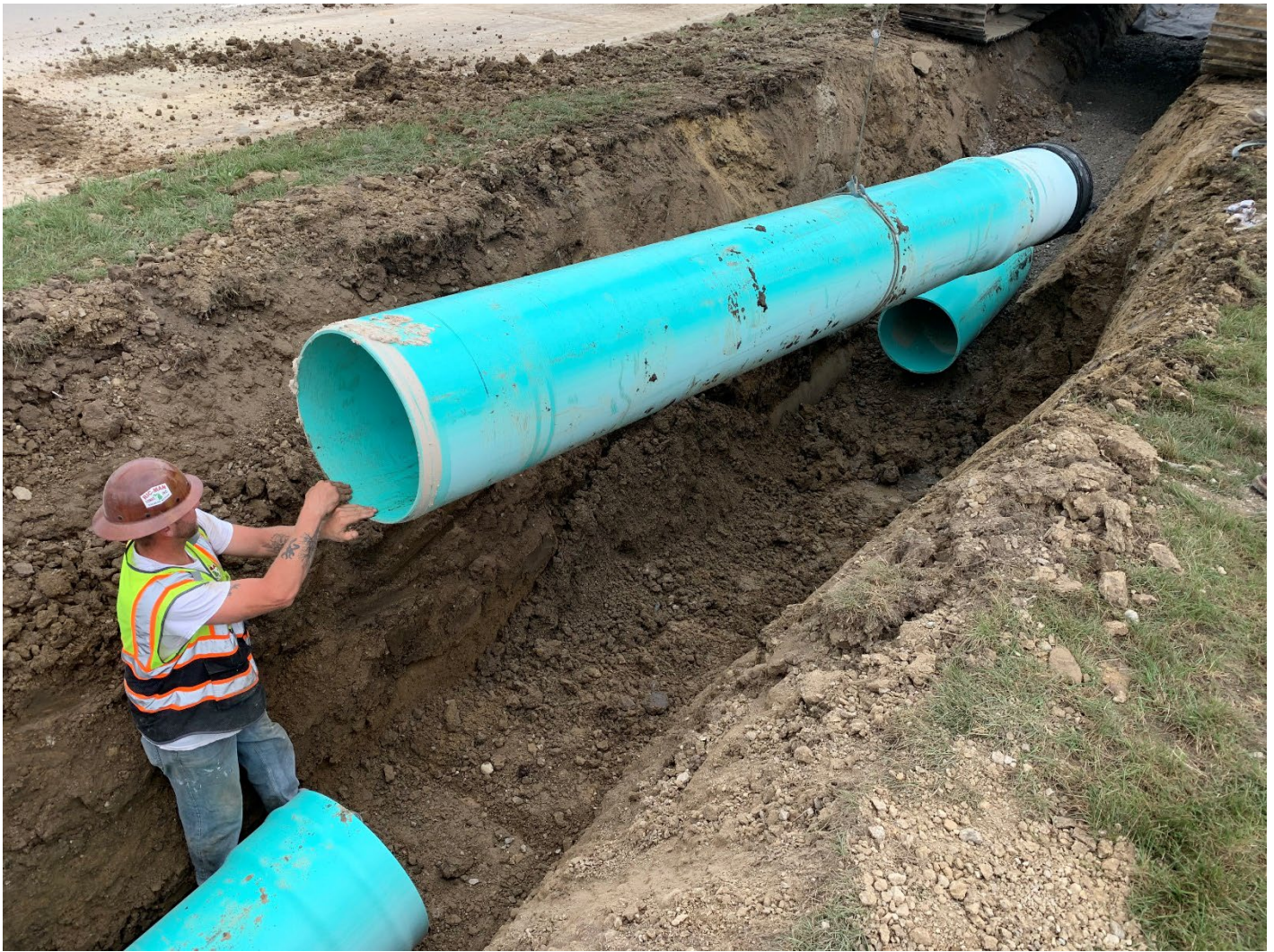
Figure 7 – FAD Installation Along 15 Mile
