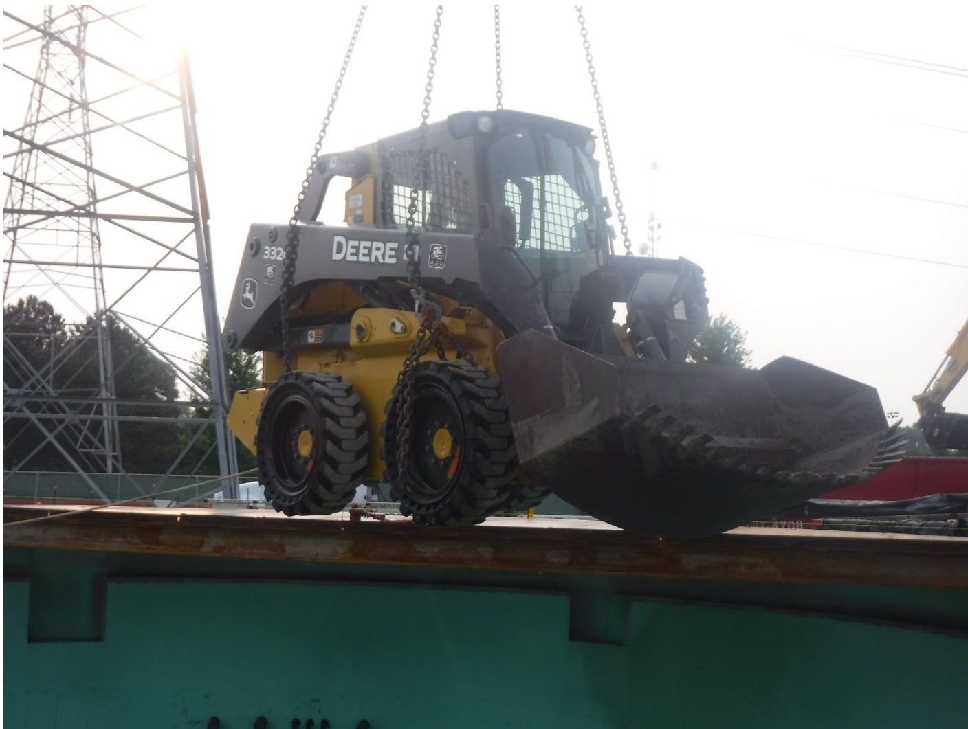
Figure 2 – Lowering Skid-steer into CS-12 for Cleaning Operations
