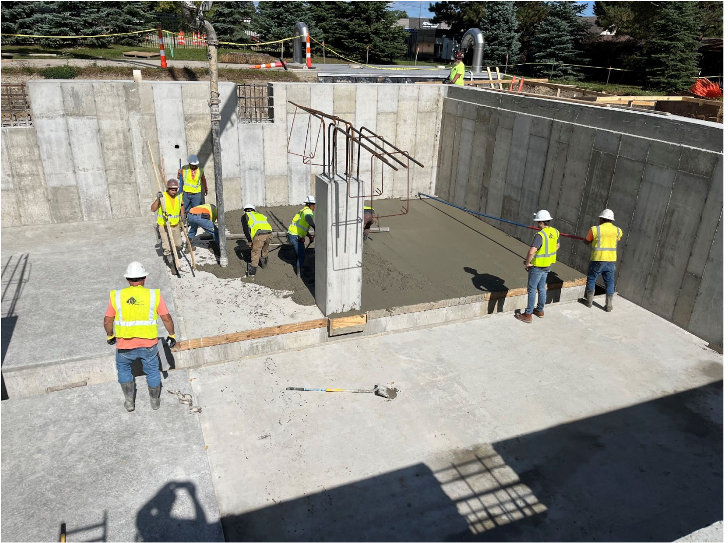
Figure 12 – Fraser Biofilter Concrete Placement
