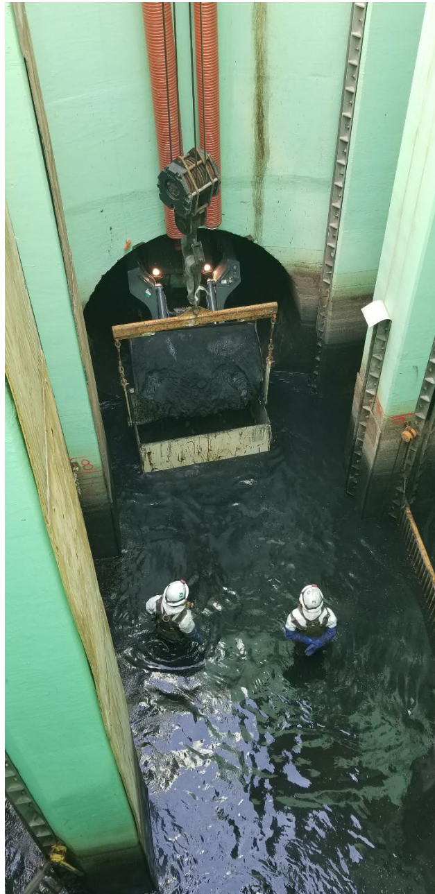
Figure 3 – Skid-Steer Returning to CS-12 during Debris Removal Operation
