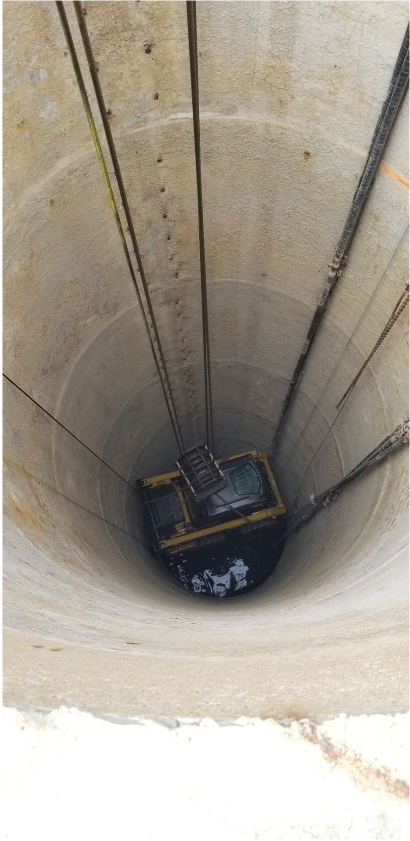
Figure 5 – Lowering in Skid-steer at MH-05
