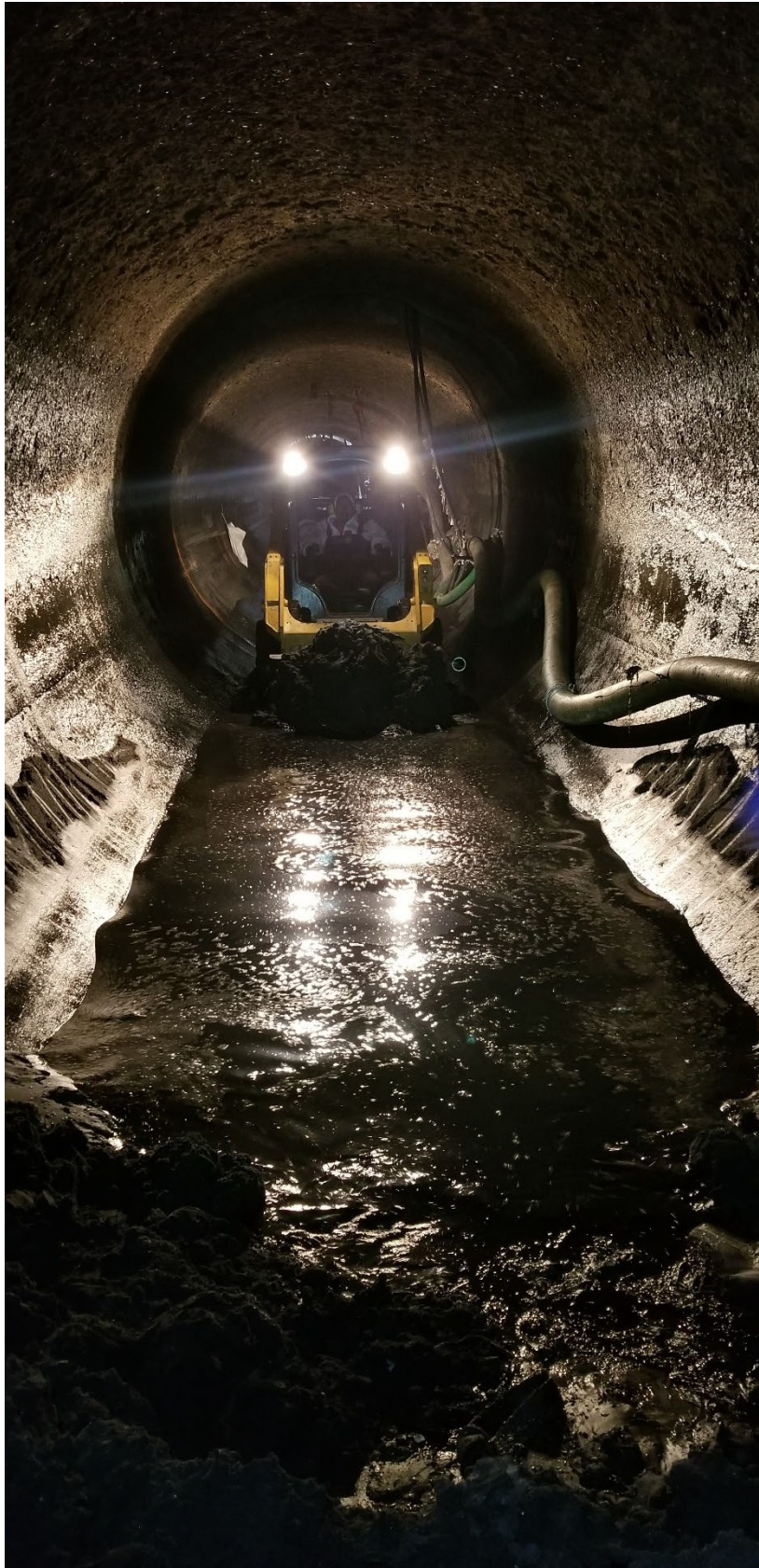
Figure 4 – Debris Removal at MH-05
