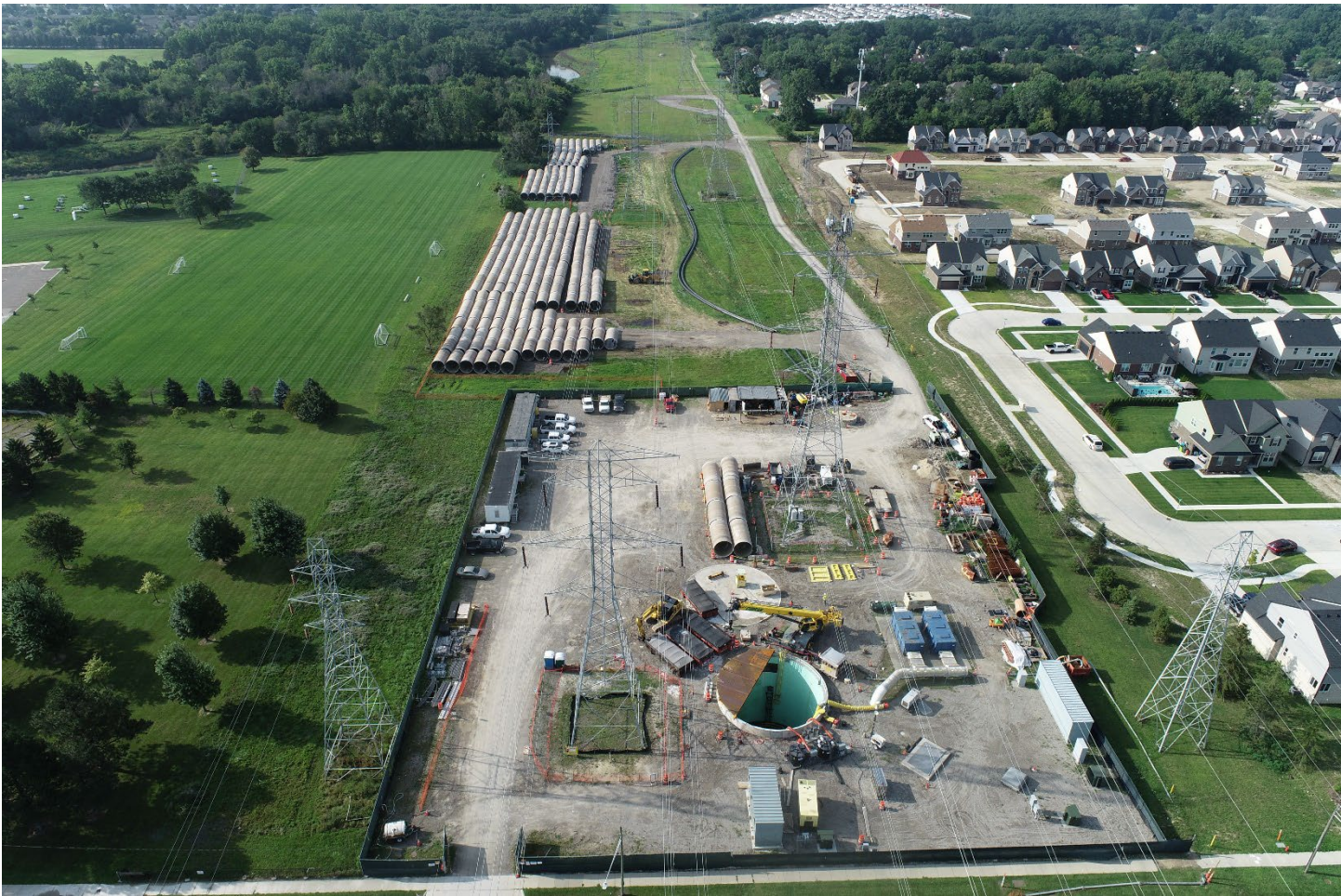
Figure 1 – CS-12 Pump Station, Construction Yard & HOBAS Storage
