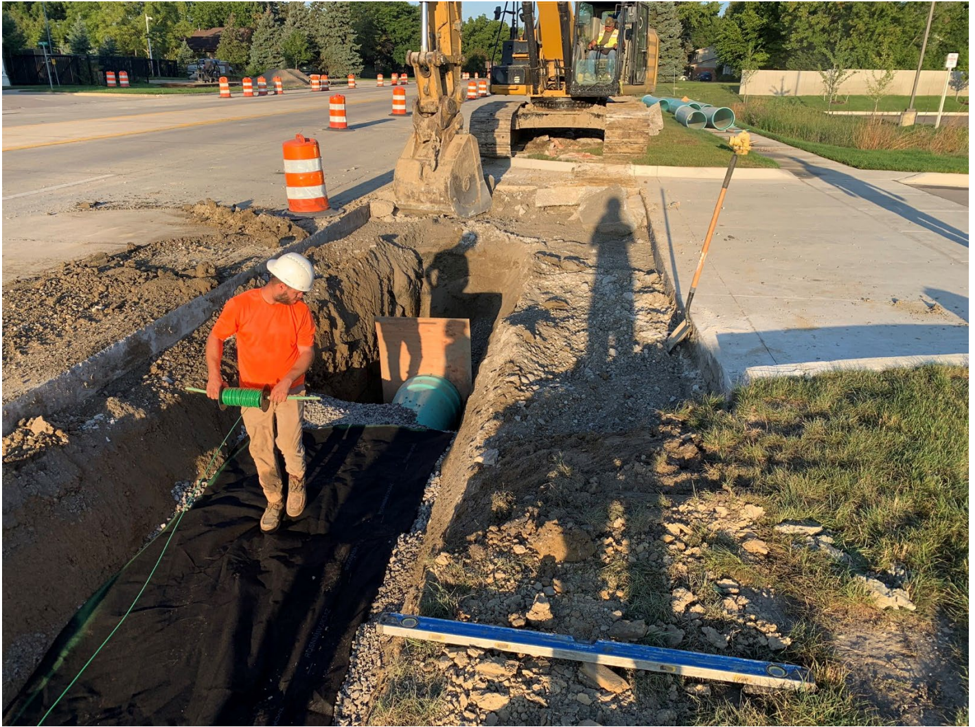
Figure 8 –FAD Installation along 15 Mile
