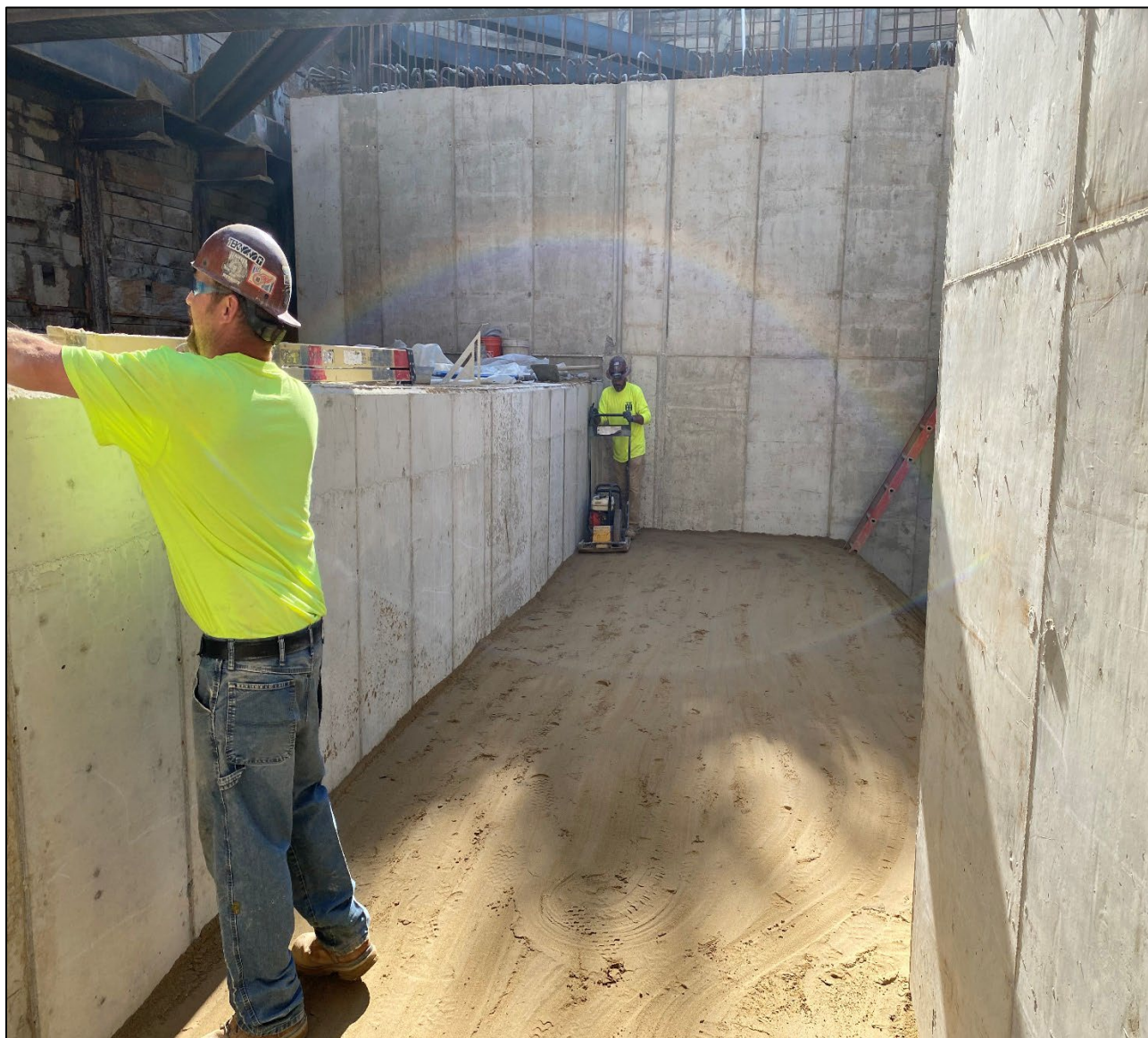
Figure 2 – Compacting Sand Backfill @ Beaconsfield Shaft
