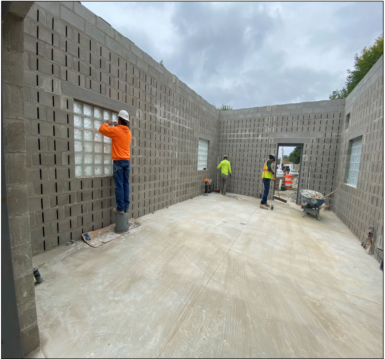
Figure 8 – Interior @ Beaconsfield Control Bldg.
