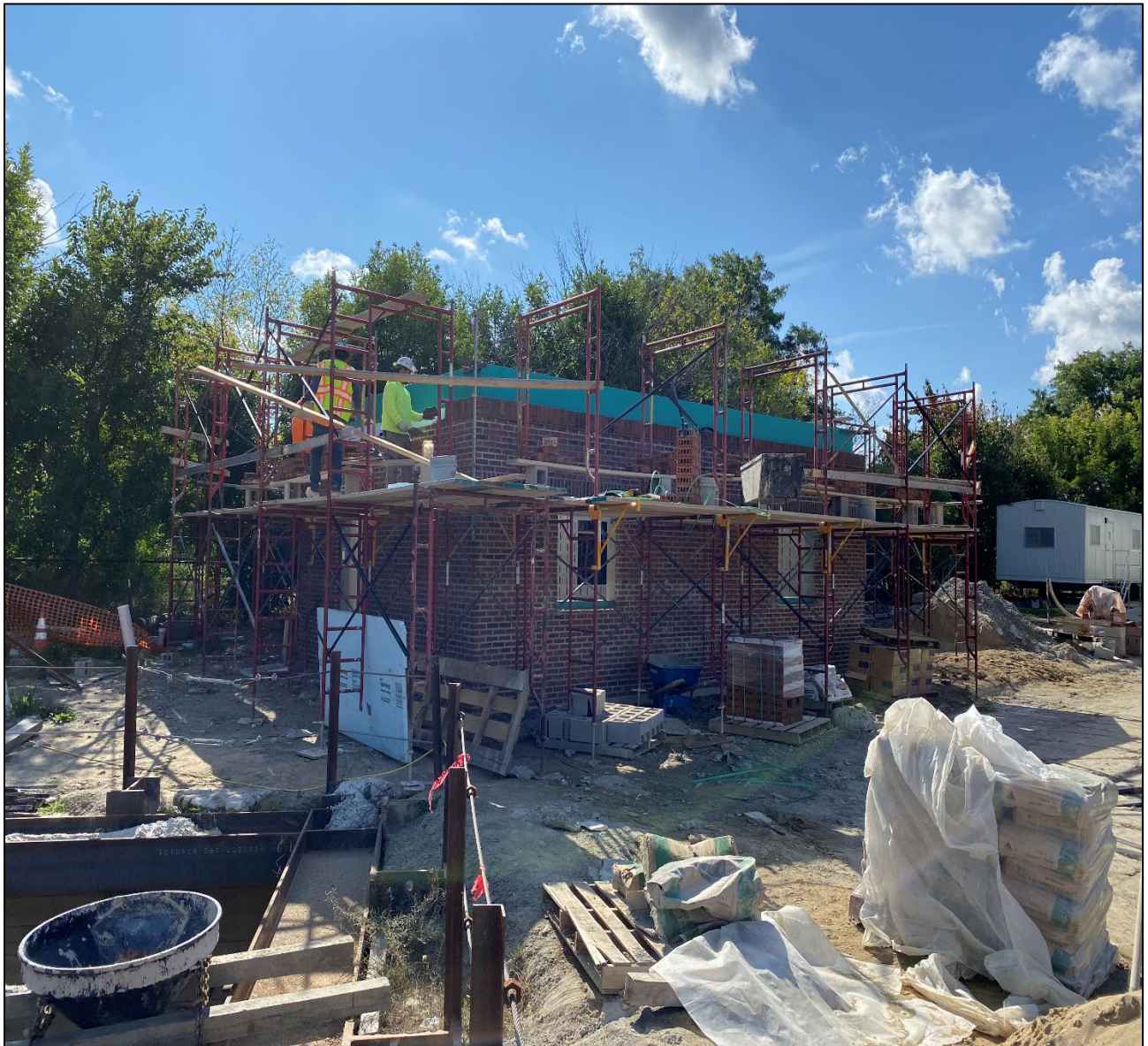
Figure 7 – Installing Brick Vernier @ Beaconsfield Control Bldg.
