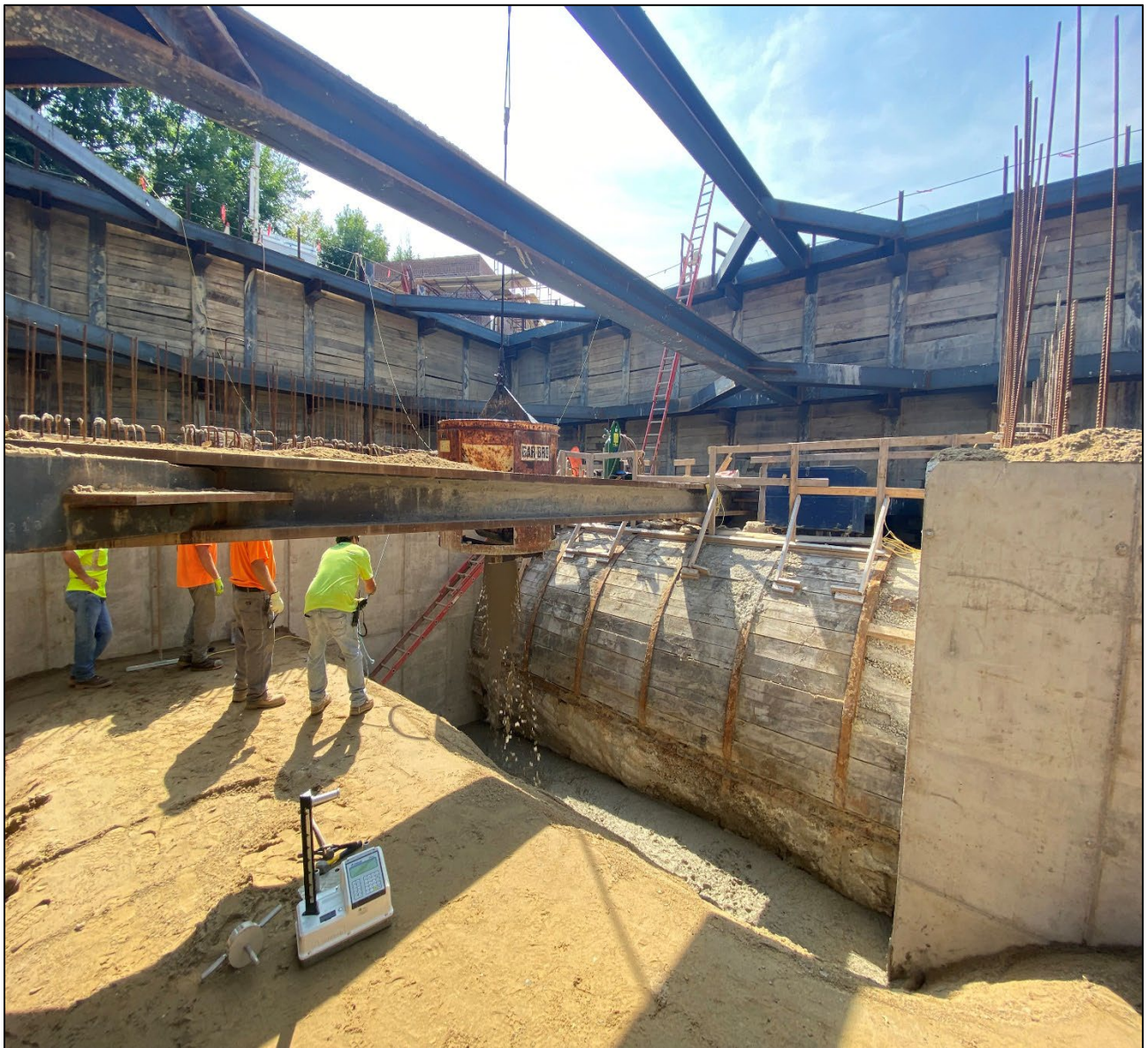
Figure 5 – Concrete Backfill @ North Side of Beaconsfield Tunnel
