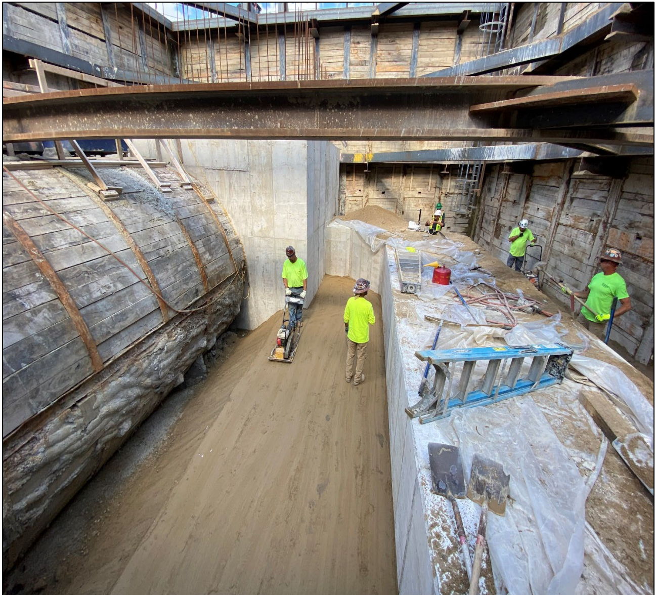
Figure 4 – Backfilling & Compaction @ Beaconsfield Shaft
