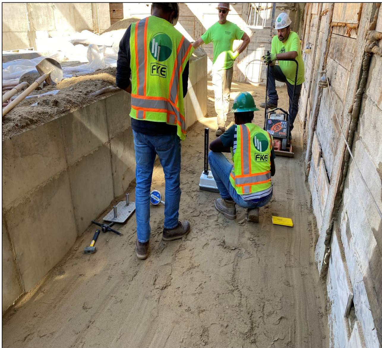
Figure 3 – Density Testing Sand Backfill @ Beaconsfield Shaft
