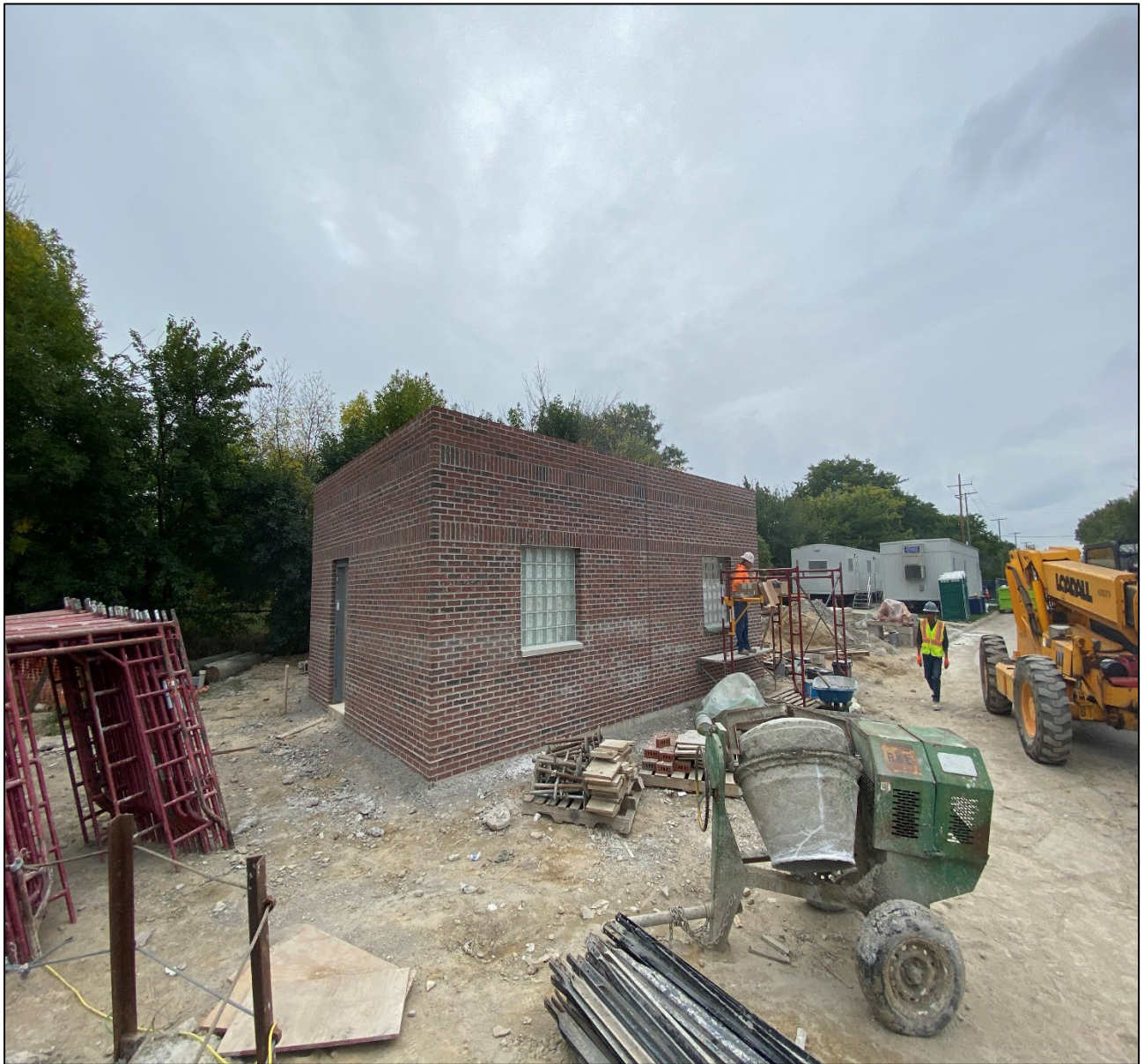
Figure 9 – Installing Glass Block Windows @ Beaconsfield Control Bldg.
