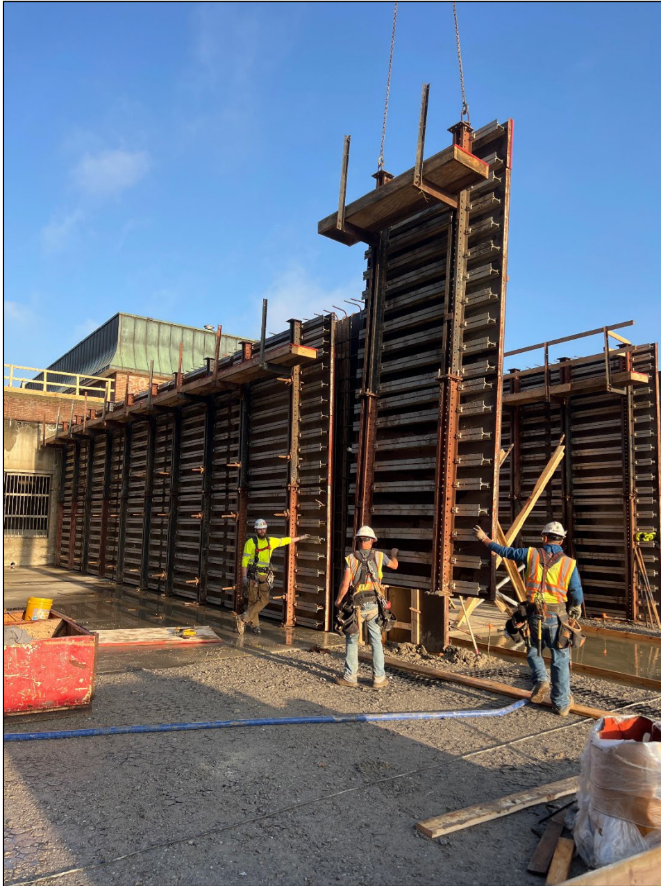
Figure 13 – Forms and re-steel for divider walls (on new base slab)
