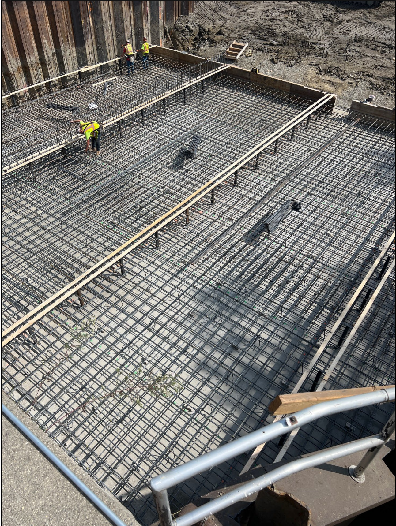
Figure 11 – Rebar within the base slab on the West end.
