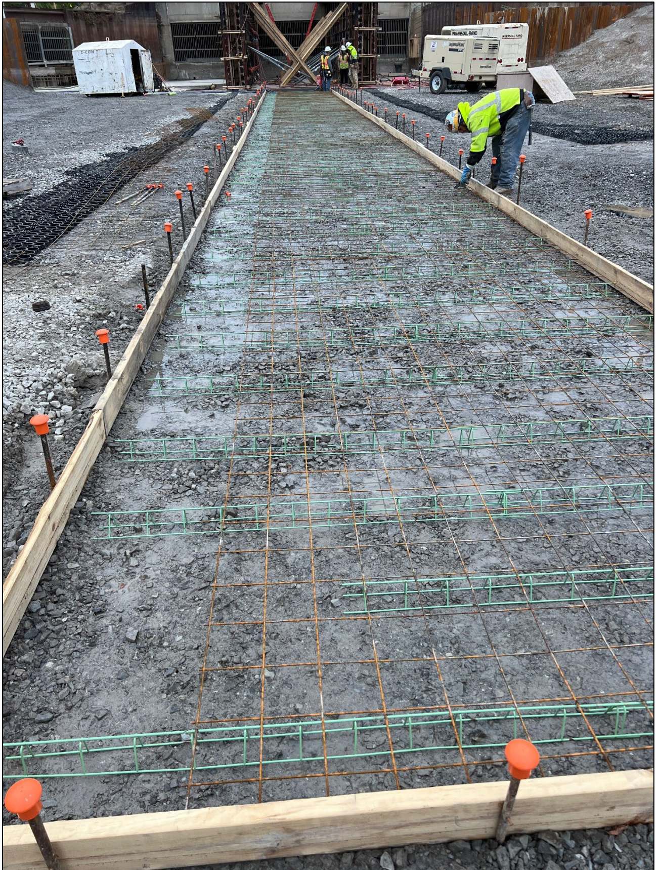
Figure 12 – Access Road Pour adjacent to new stone & geogrid reinforcement
