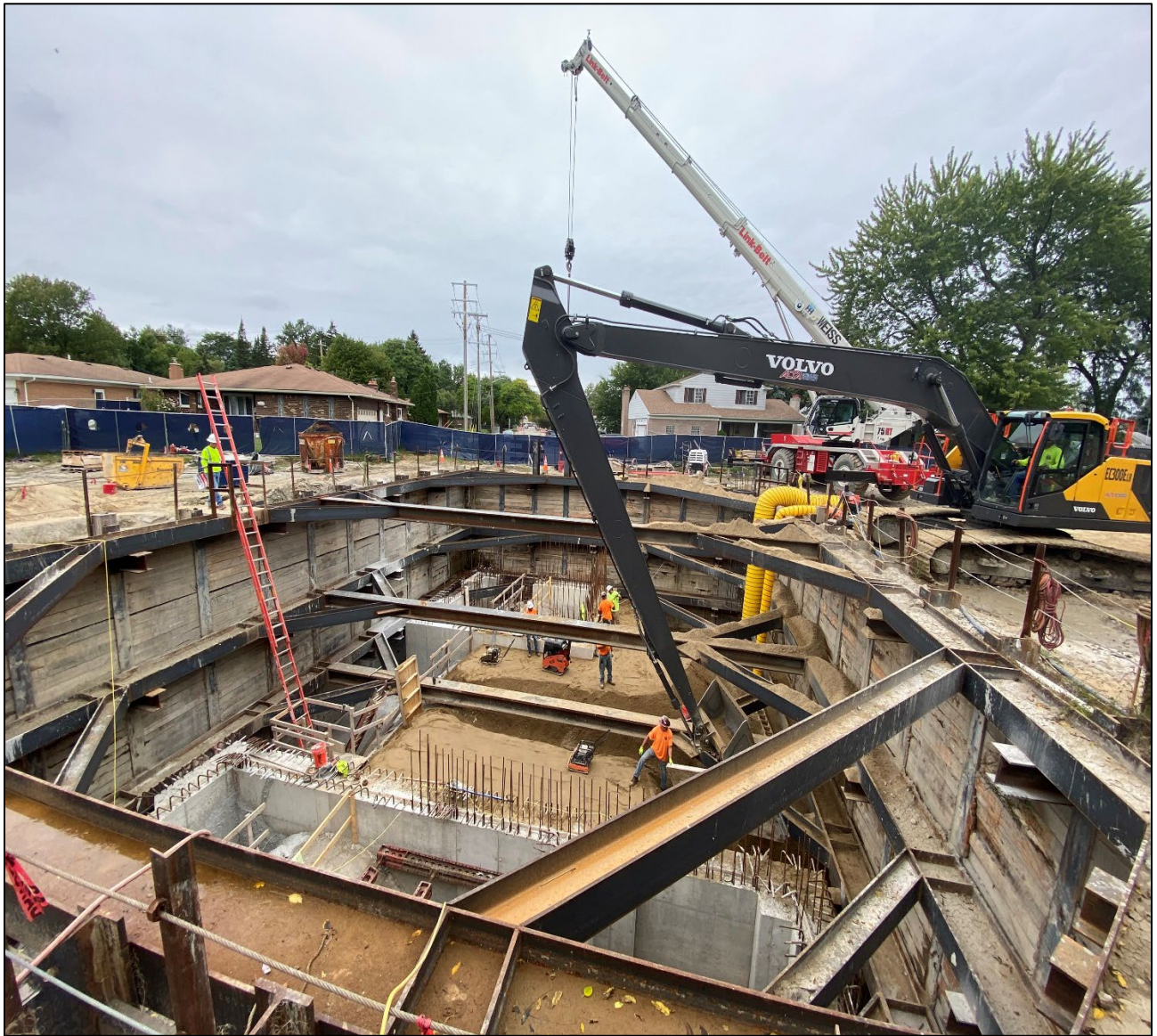
Figure 6 – Placing Sand Backfill @ Beaconsfield Shaft
