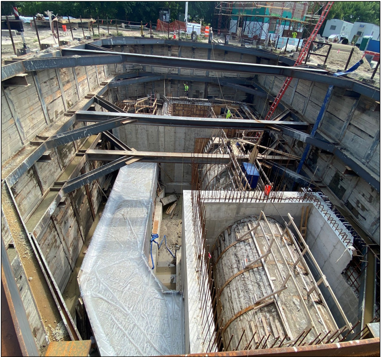
Figure 1 – Placed Concrete Bypass @ Beaconsfield Shaft
