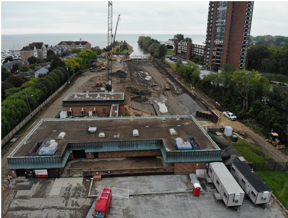
Figure 16 – Drone Aerial at 100 FT Facing East (9/29/23)
