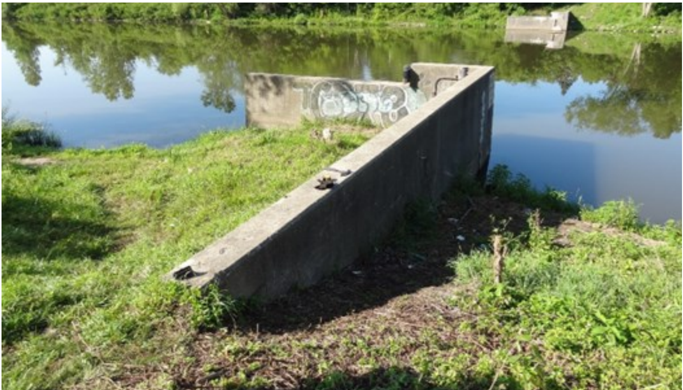
4. Elevation of the east abutment (looking west)
