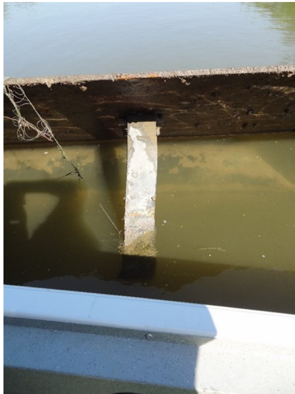
20. Eleventh restraining strap cut (looking down)
