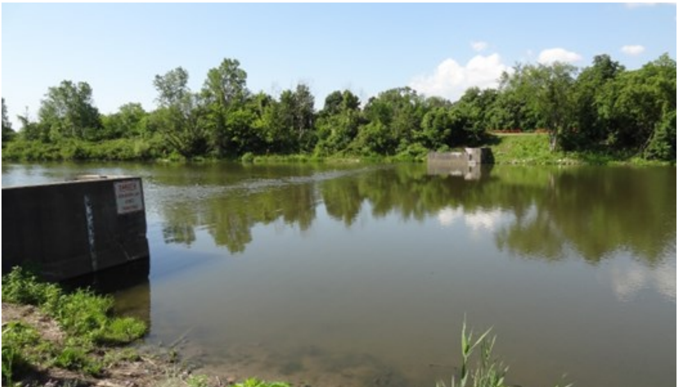
24. Elevation of weir in fully deflated condition (looking south).
