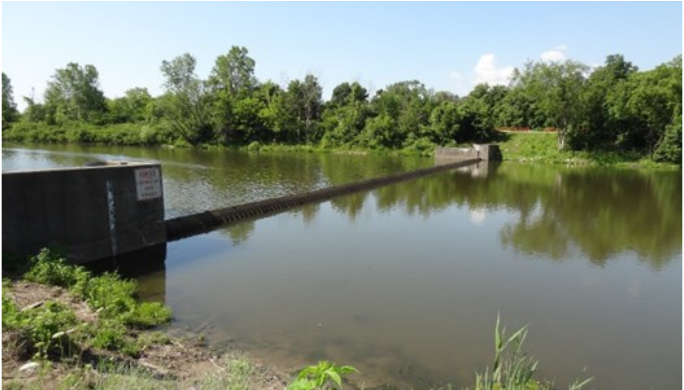
21. Elevation of weir in 100% inflated condition (looking south)
