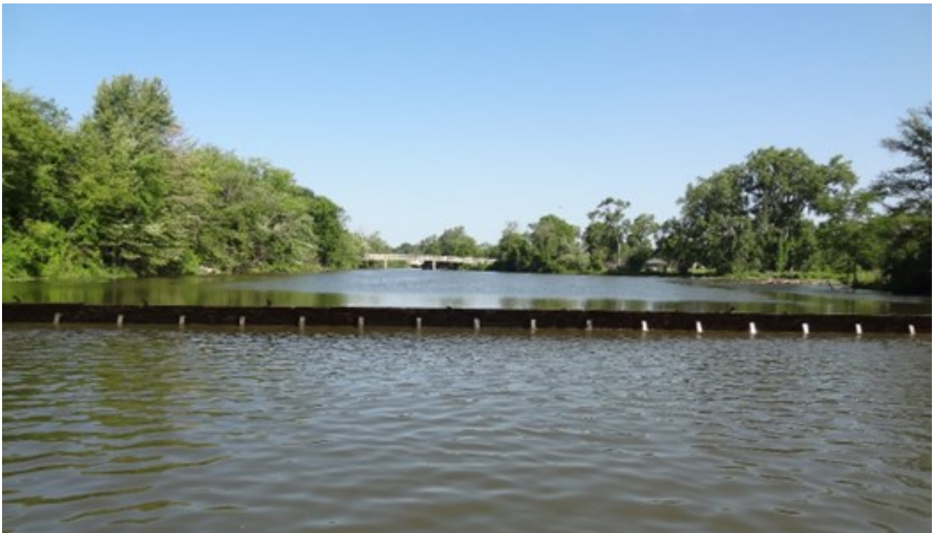
16. Elevation of the back side of the fully inflated weir plates (looking north)
