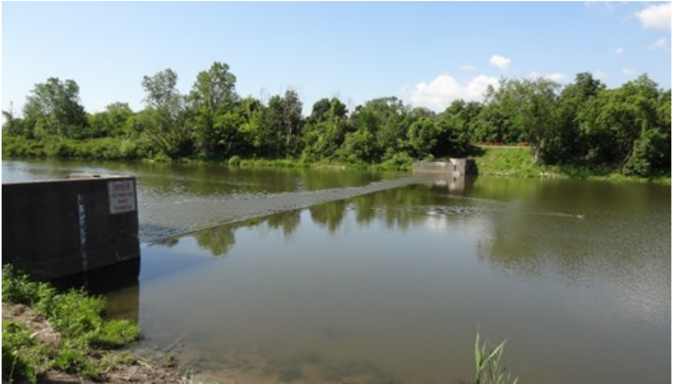
23. Elevation of weir in 25% inflated condition (looking south)
