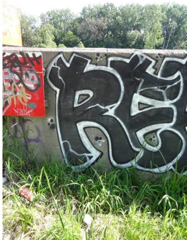
13. Vertical shrinkage crack observed on the interior face of west abutment wing wall (looking east)
