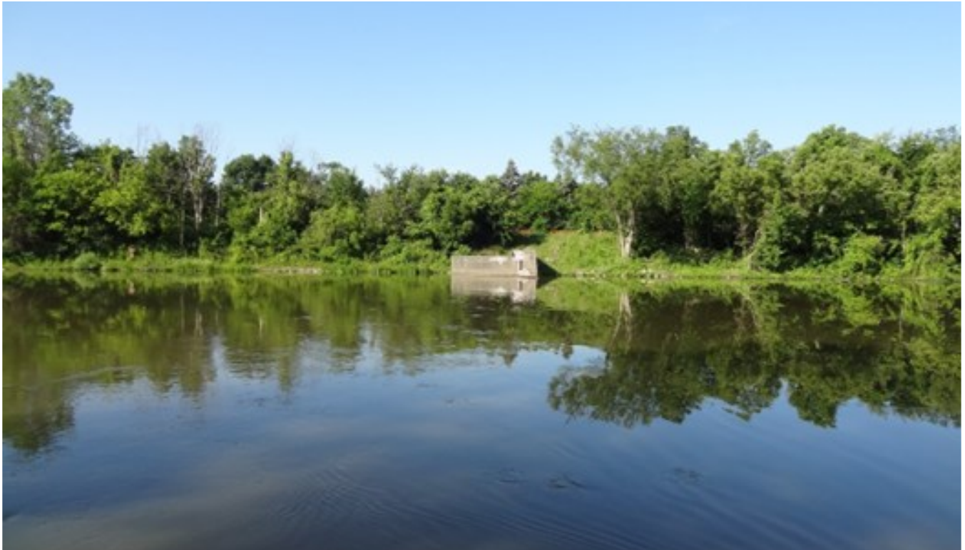
9. Elevation of the wing wall of the west abutment (looking east)
