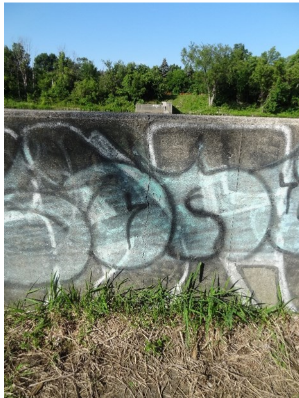
6. Vertical shrinkage crack observed on interior east abutment wing wall (looking west)
