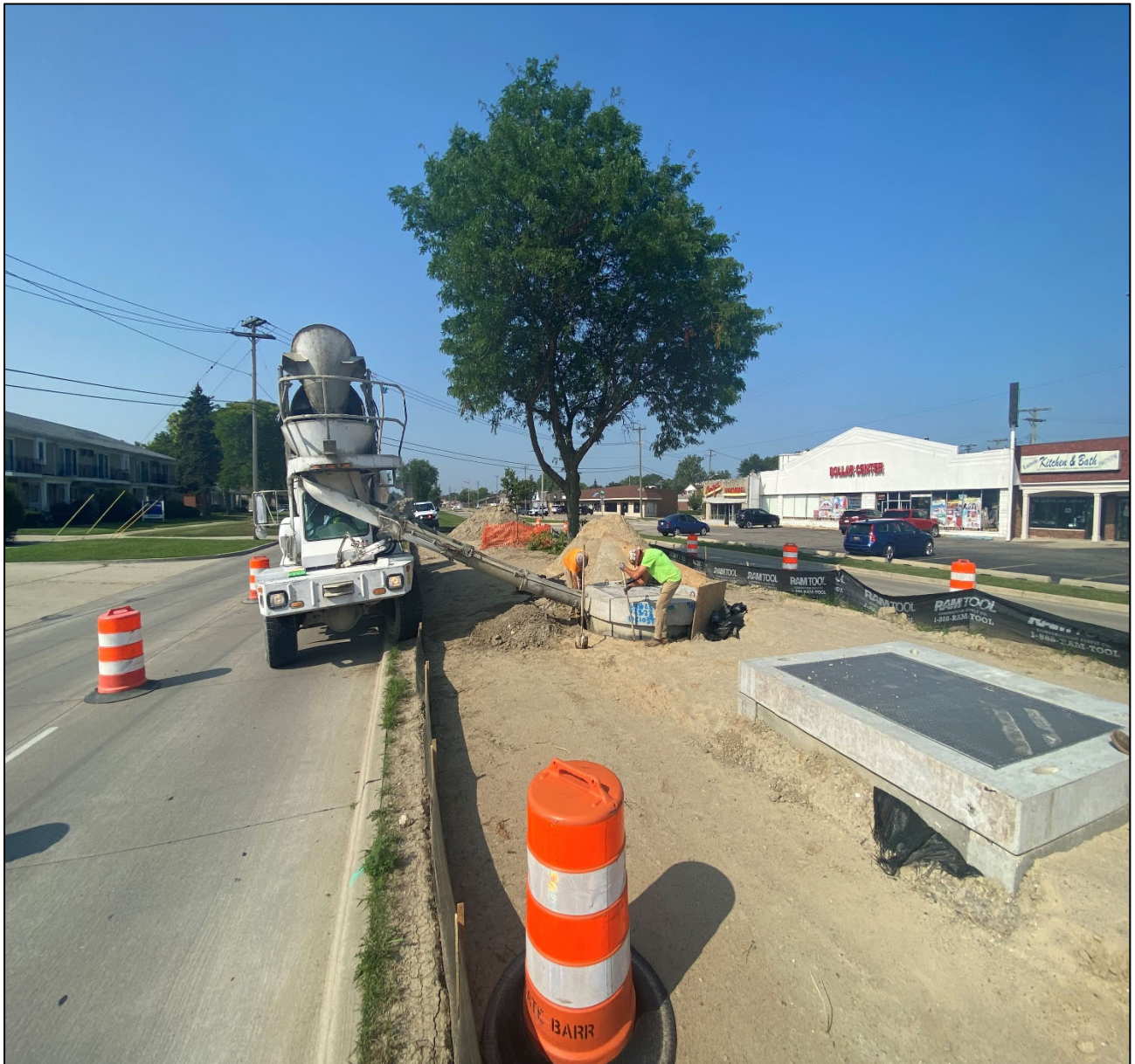
Figure 1 – Placing Concrete Fill for Access Riser @ Kelly Rd.
