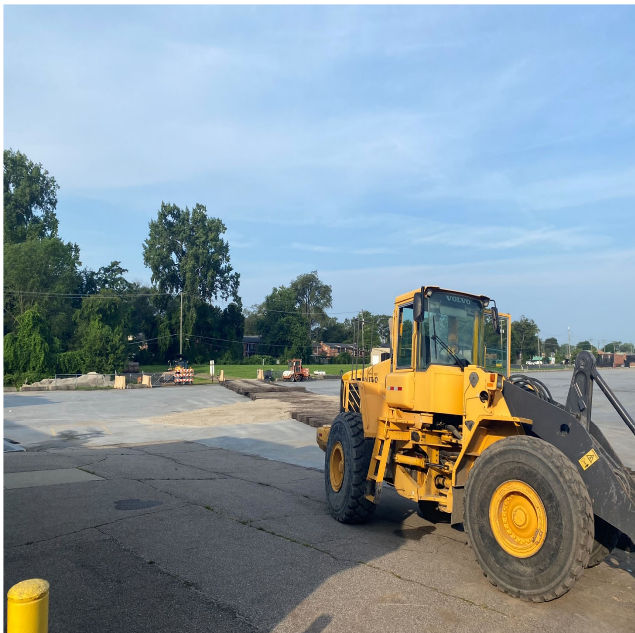
Figure 12 – Crane Mats Being Installed Across the RTB
