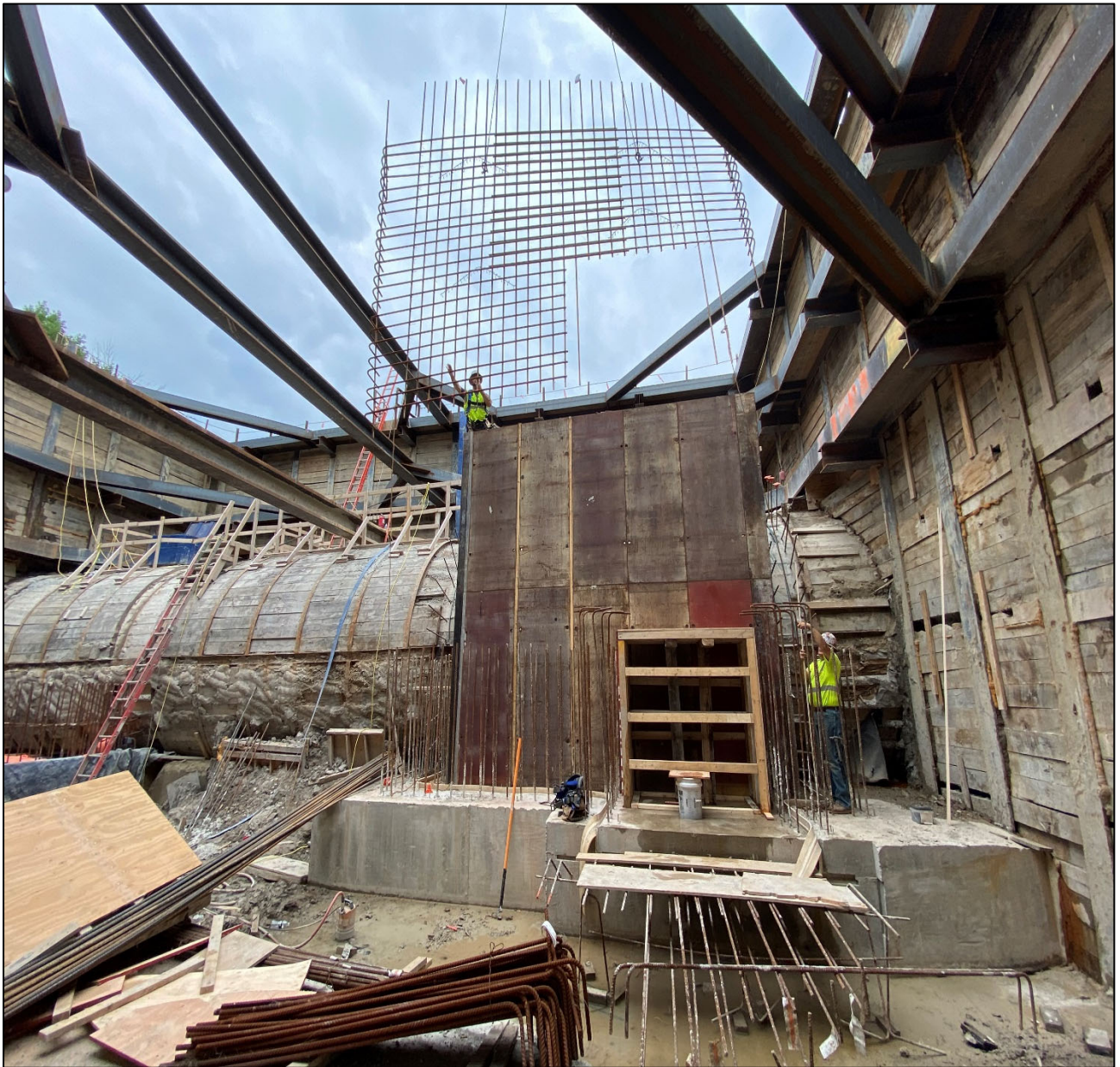
Figure 4 – Installing Reinforcing Steel @ West Wall of Beaconsfield Shaft
