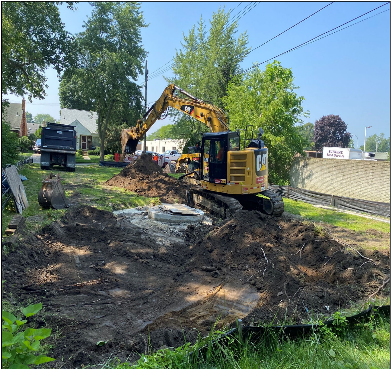
Figure 3 – Excavating for New Access Drive @ Gaukler St.
