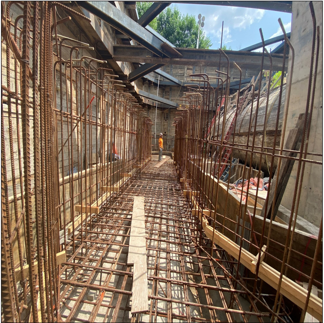
Figure 8 – Installed Reinforcing Steel for Bypass Adjacent to Tunnel @ Beaconsfield Shaft
