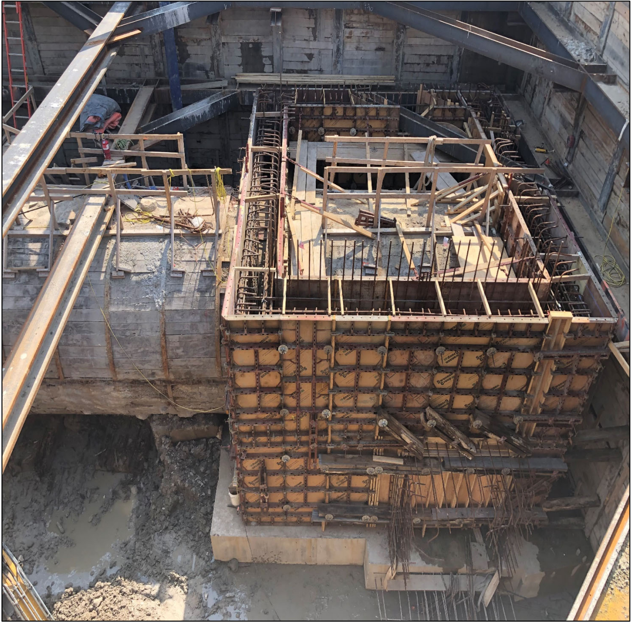
Figure 6 – Installed Concrete Wall Forms @ West Wall of Beaconsfield Shaft
