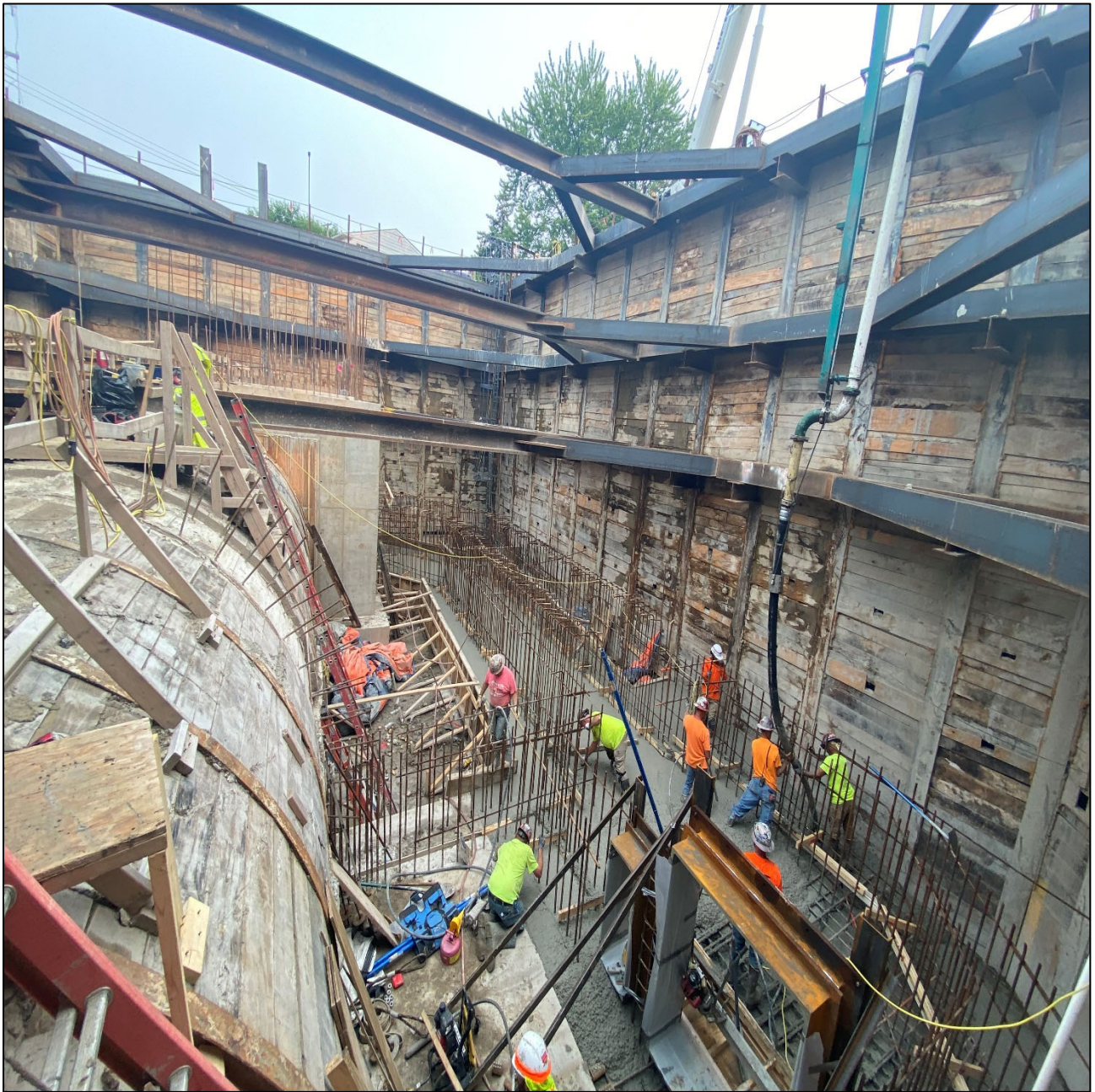
Figure 9 – Placing Concrete Bypass Base Slab via Pump @ Beaconsfield Shaft
