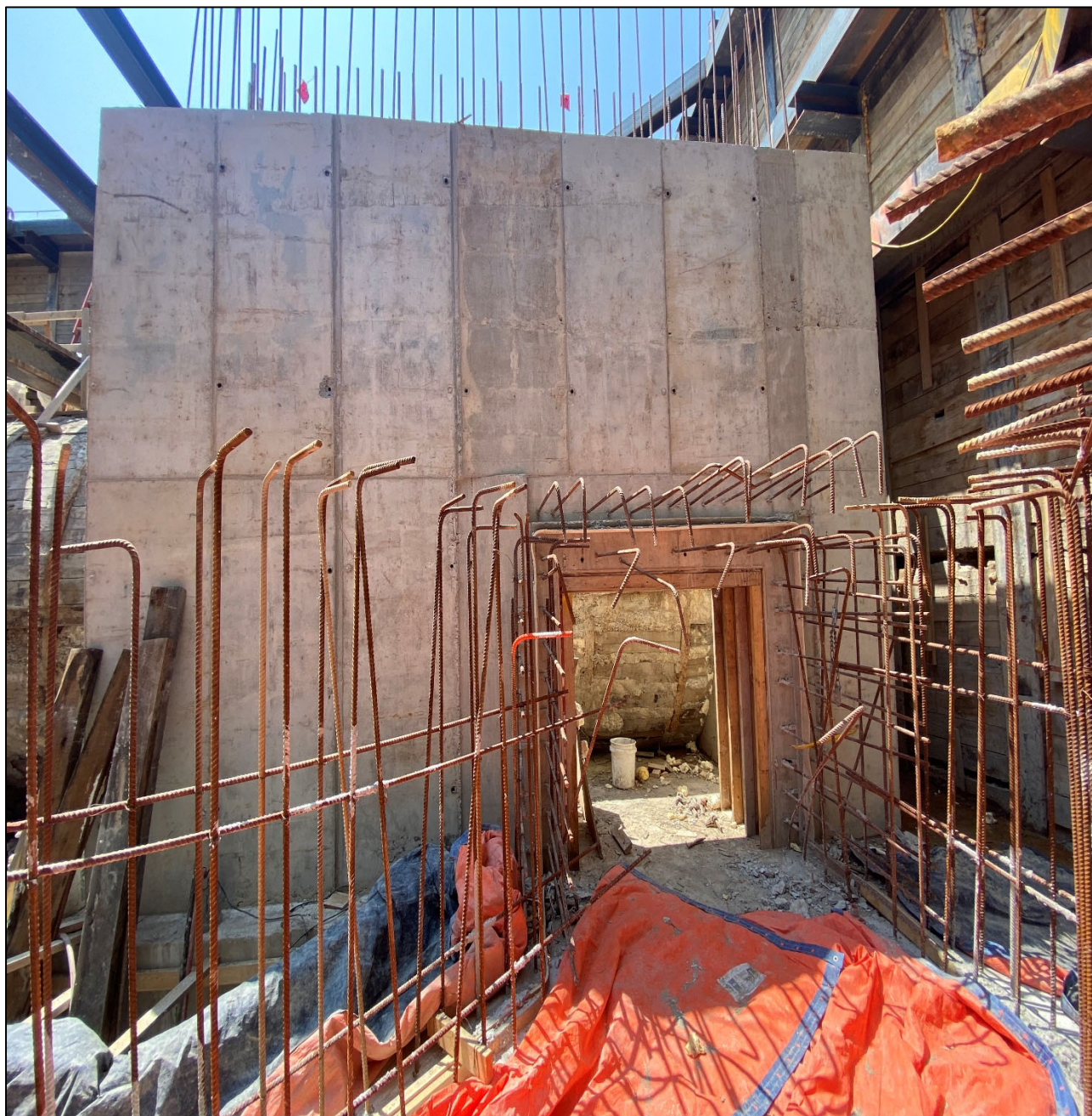
Figure 7 – New Concrete Walls @ West Side of Beaconsfield Shaft
