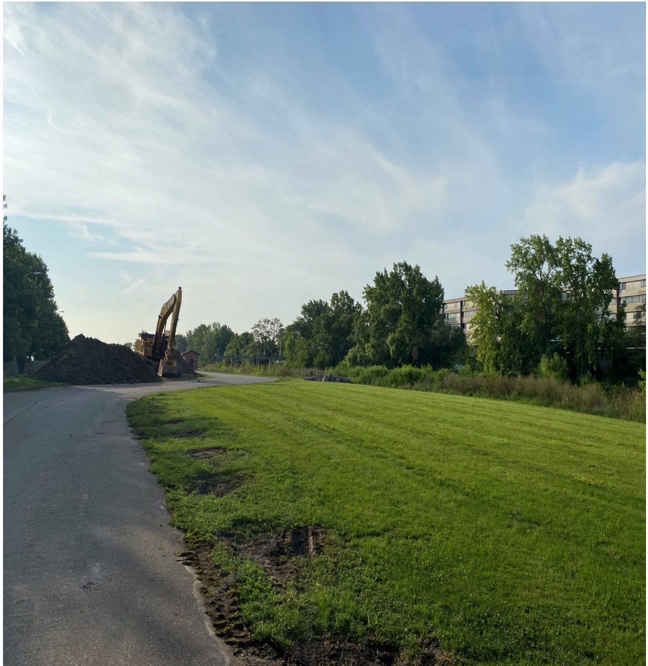
Figure 14 – Interior Fencing Removed
