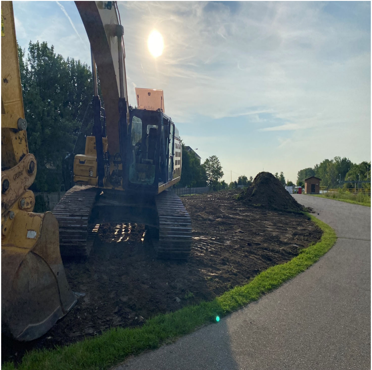
Figure 13 – Excavation work starting at the North Berm.
