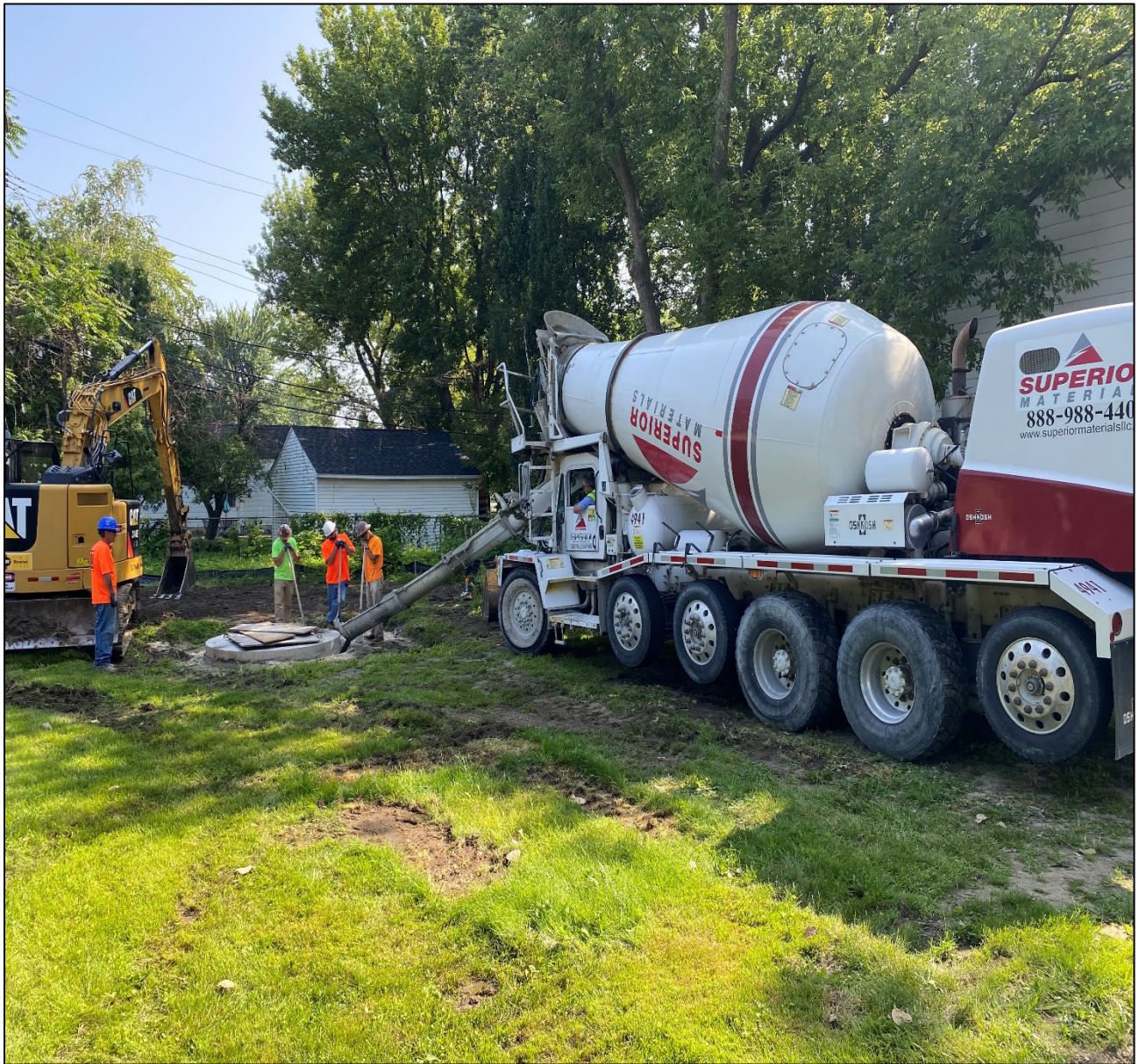
Figure 2 – Placing Concrete Fill for Access Riser @ Gaukler St.
