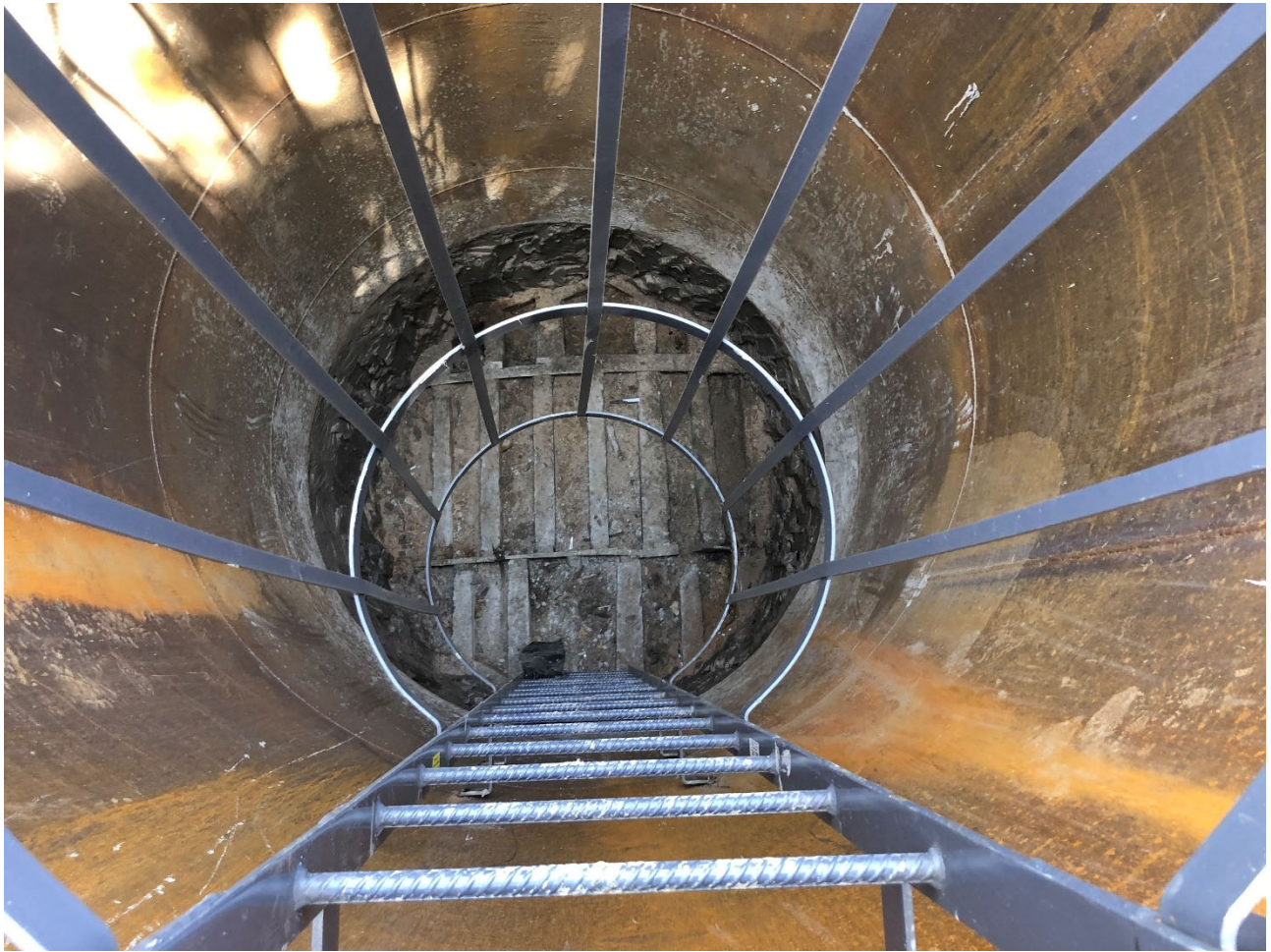
Figure 4 - Kelly Vent Shaft Showing Tunnel Rib and Lagging
