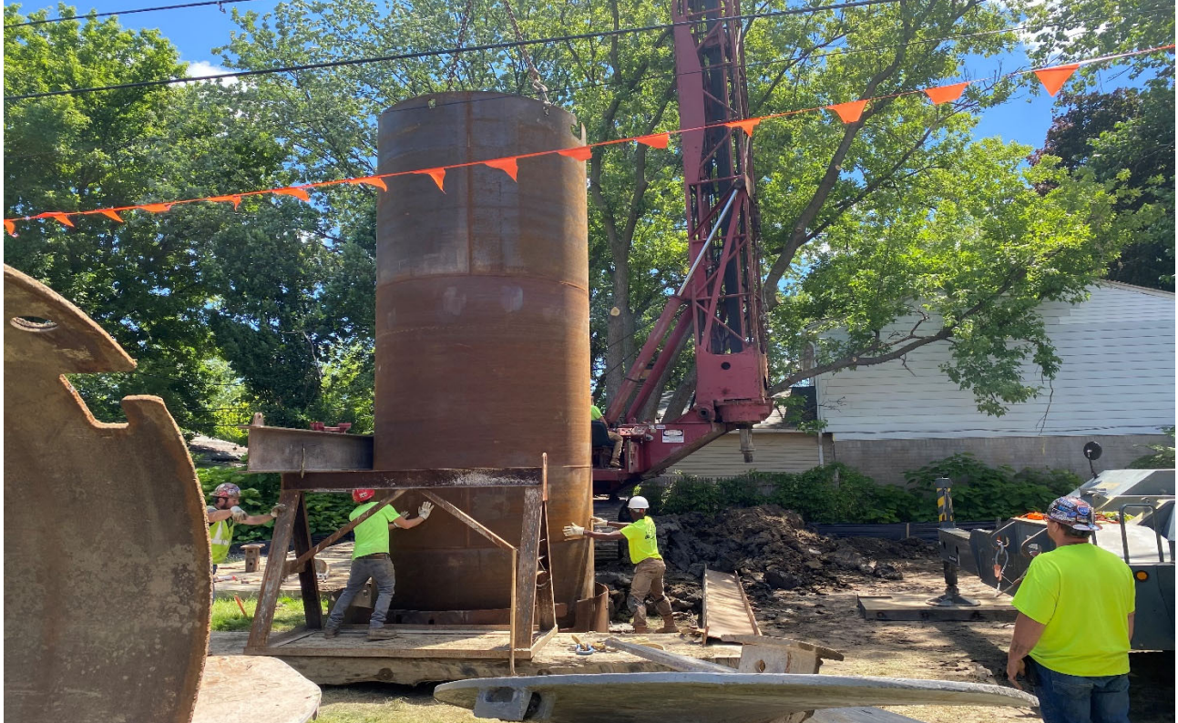
Figure 1 - Shaft to Top of 8-1/2 Relief Pipe at Gaukler Site
