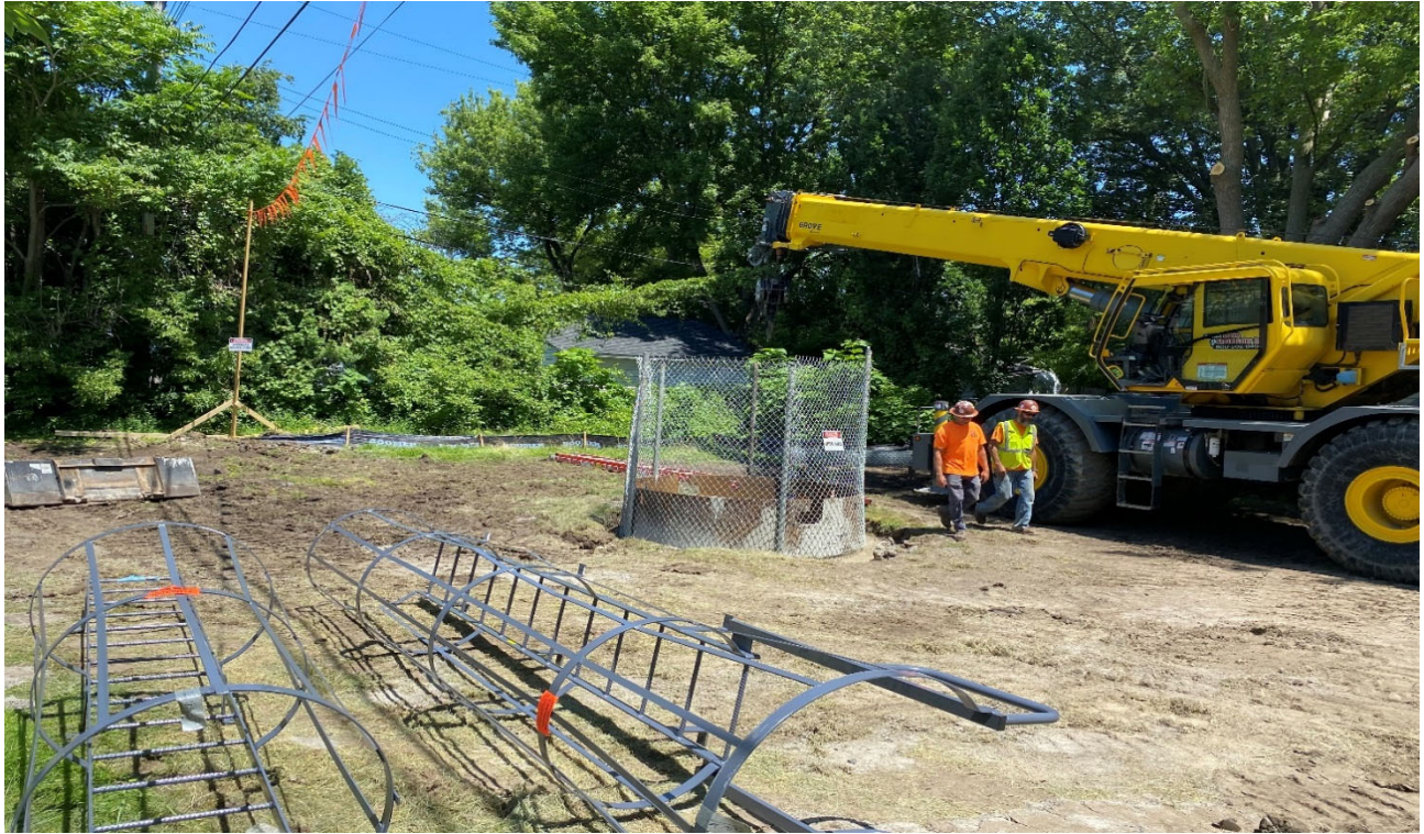
Figure 2 - Installed Shaft at Gaukler Site for New Pressure Relief Vent
