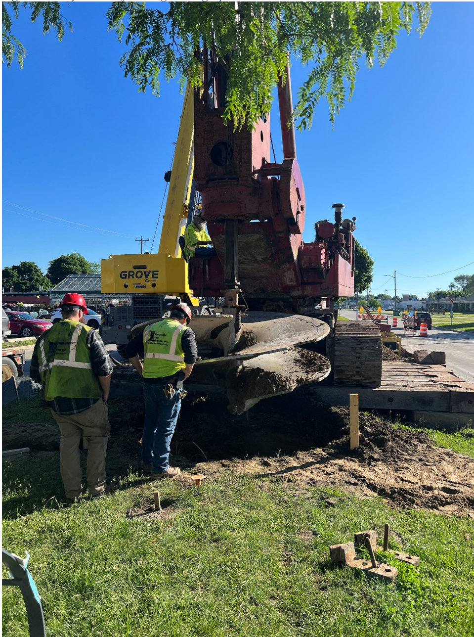
Figure 3 - Kelly Vent Shaft During Drilling Operation
