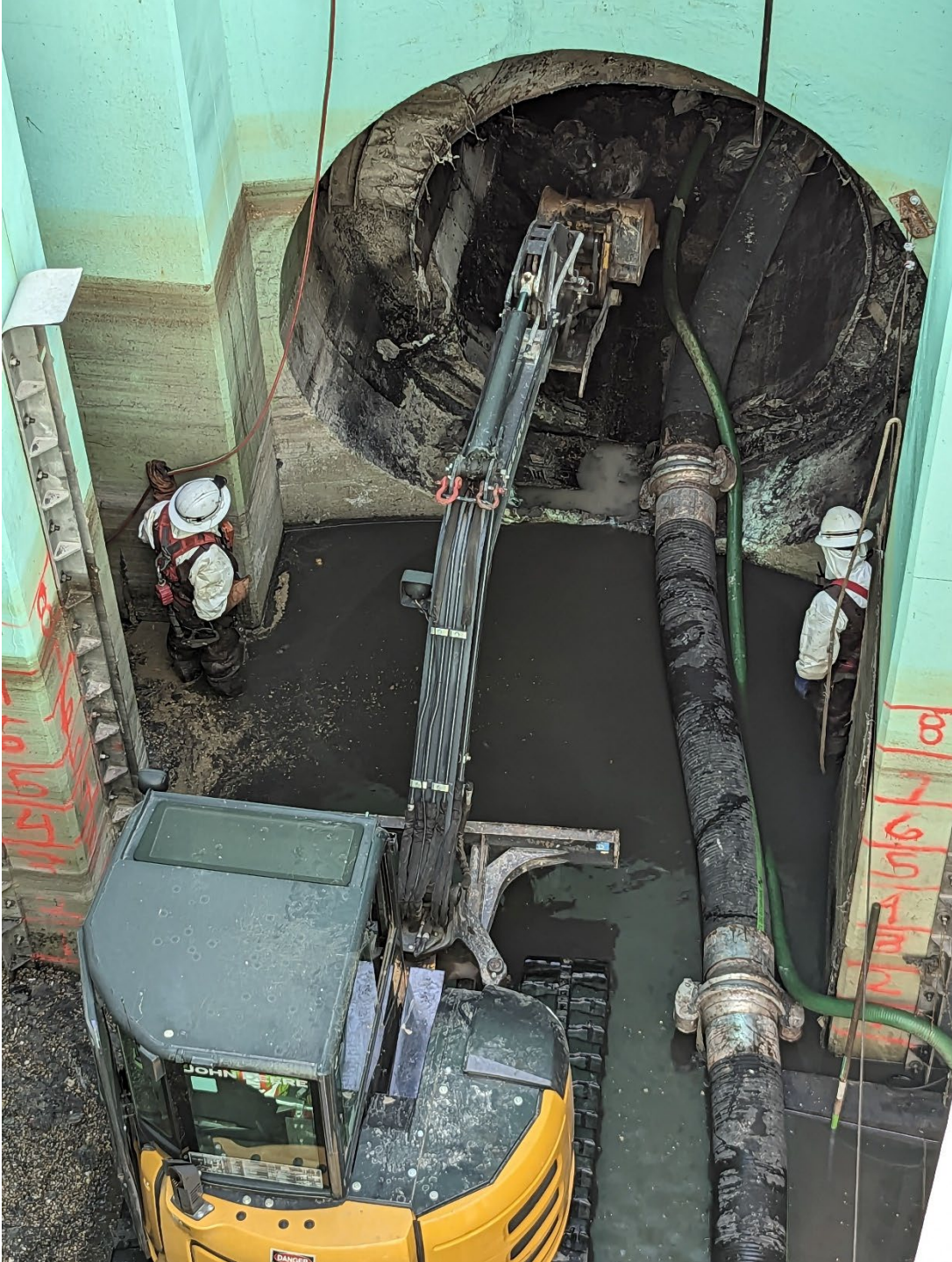
Figure 2 – Demolition of the Temporary Flume Bulkhead
