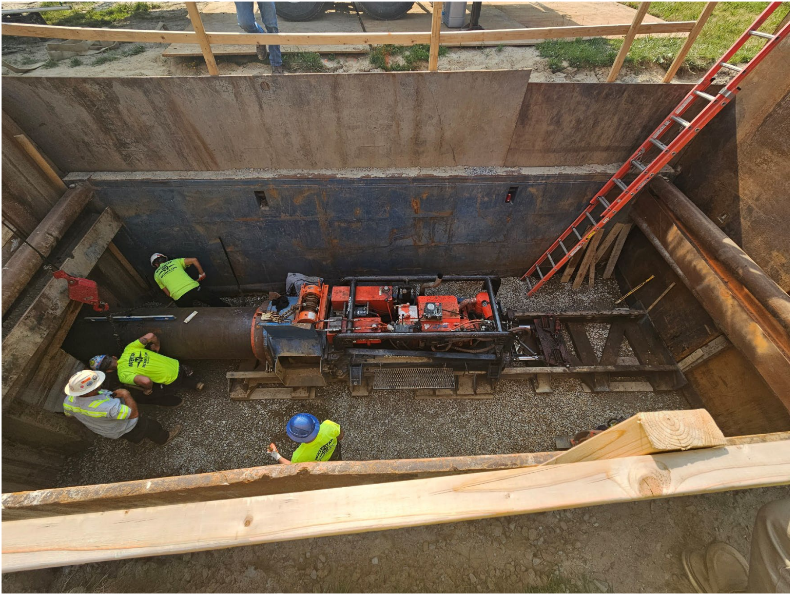
Figure 8 – Jack & Bore of Steel Casing Beneath 15 Mile Road for FAD Line
