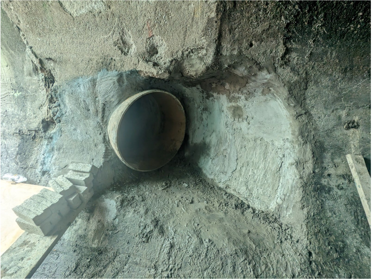
Figure 4 – Drop-Pipe Installation at Southeast Discharge
