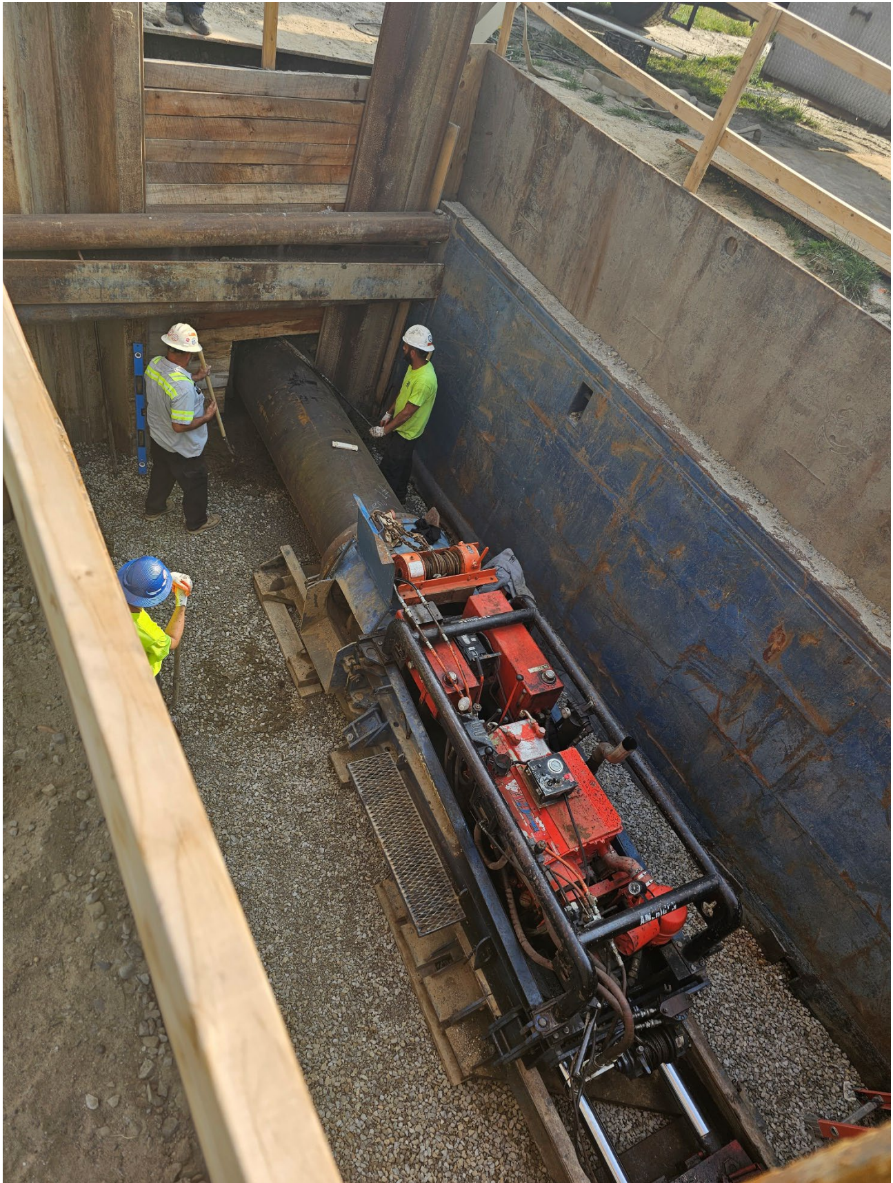
Figure 9 – Jack & Bore of Steel Casing Beneath 15 Mile Road for FAD Line
