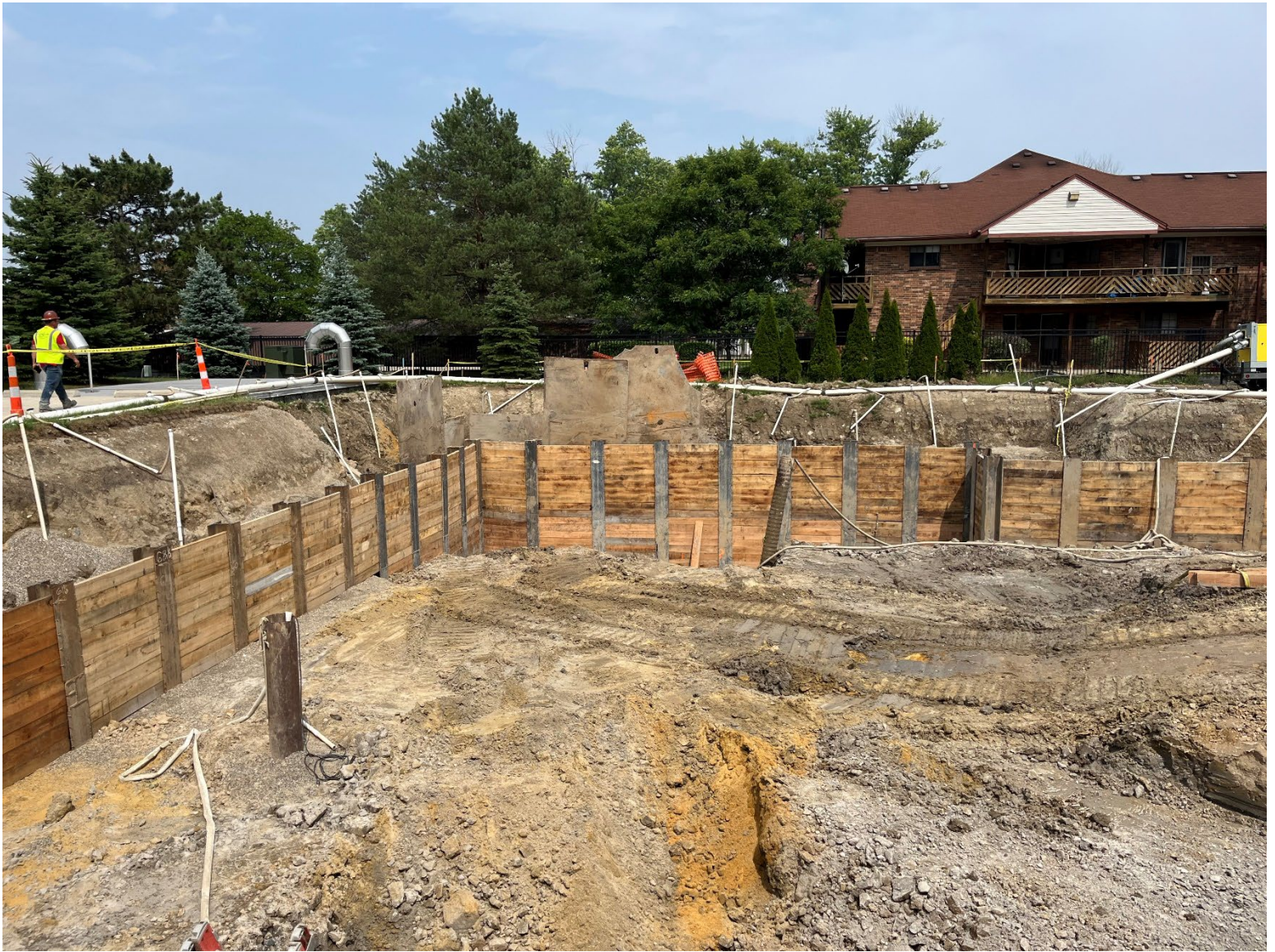
Figure 18 – Construction of the Upper TERS at Fraser Site
