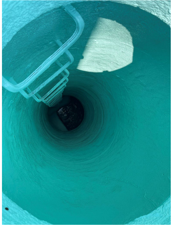
Figure 12 – MA-S-2 (East Side) MH Epoxy Lining
