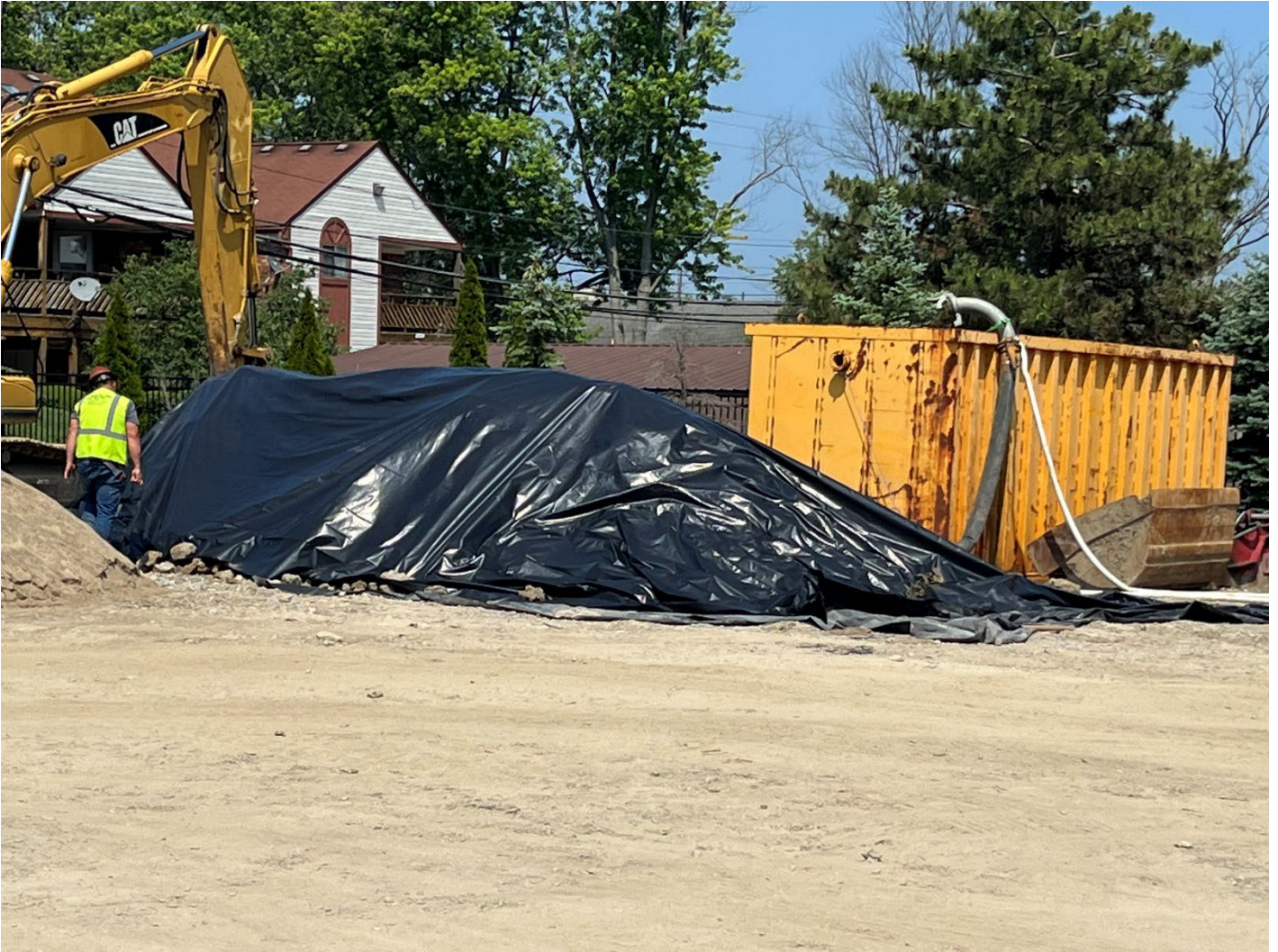
Figure 16 – Staging of Slightly Contaminated Soils at Fraser Site
