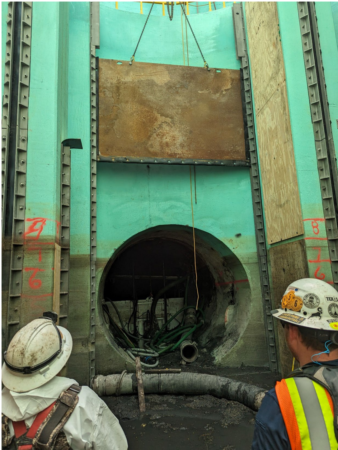
Figure 5 – Dry-Fitting the Temporary Downstream Gate
