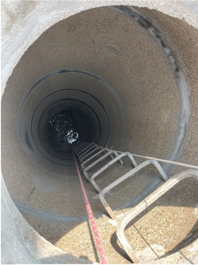
Figure 11 – MA-S-2 (East Side) MH Prep
