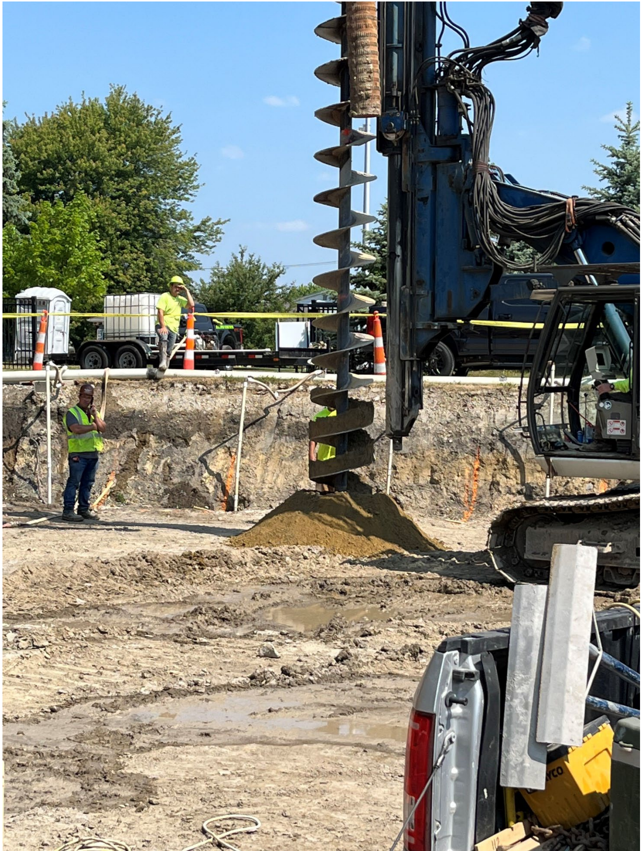
Figure 17 – Drilling Foundation Piles for Lower TERS at Fraser Site
