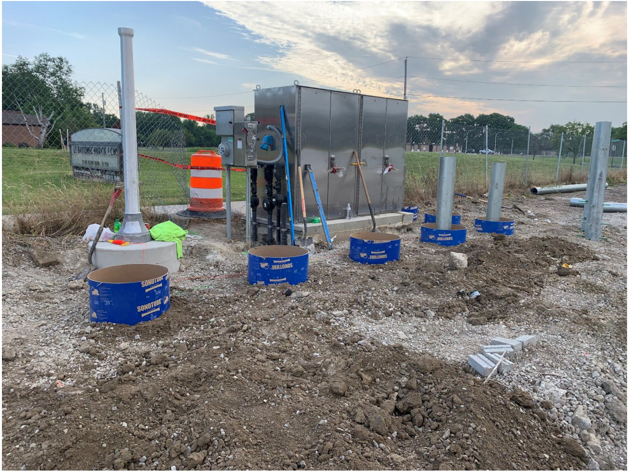
Figure 10 – Installation of Bollards at CS-13 Control Cabinet
