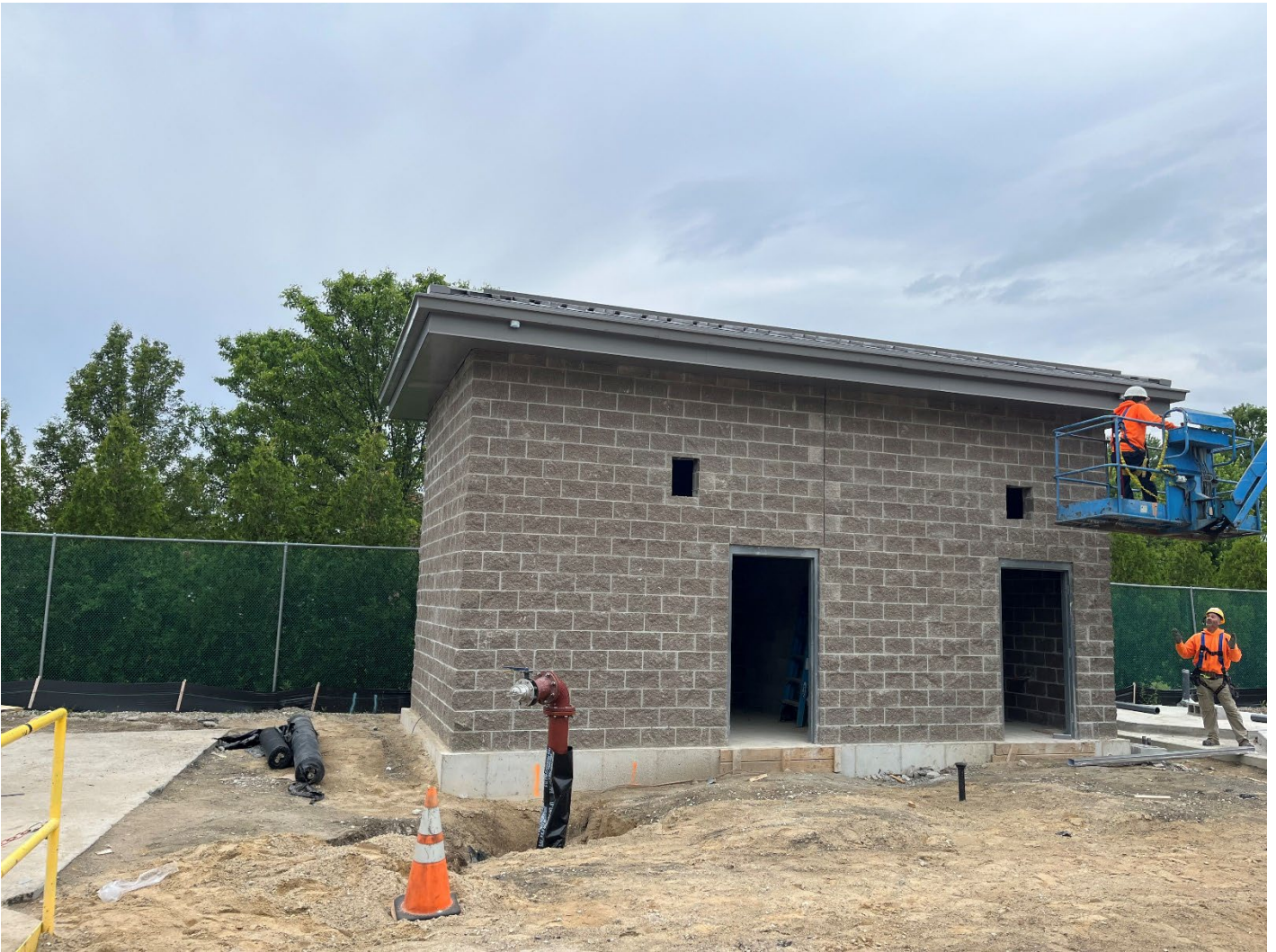
Figure 15 – NGI PS Odor & Corrosion Equipment Building – Gutter & Soffit Work
