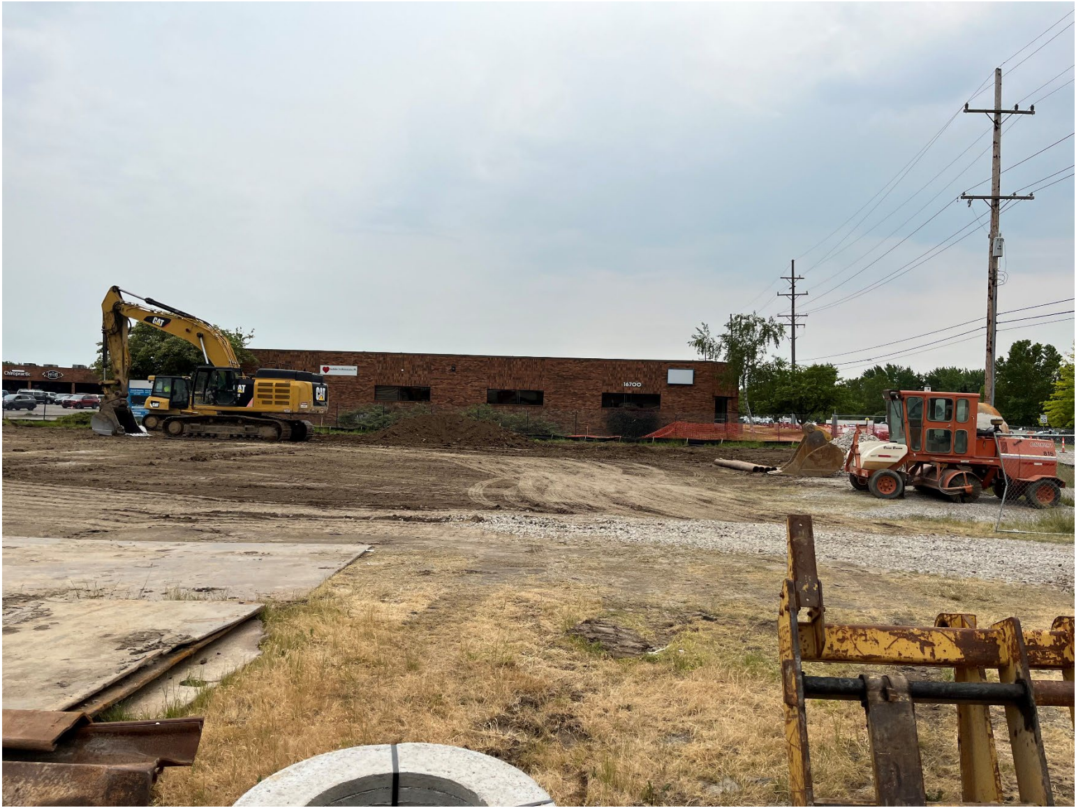
Figure 19 – Site Preparation at 21 Mile & Garfield
