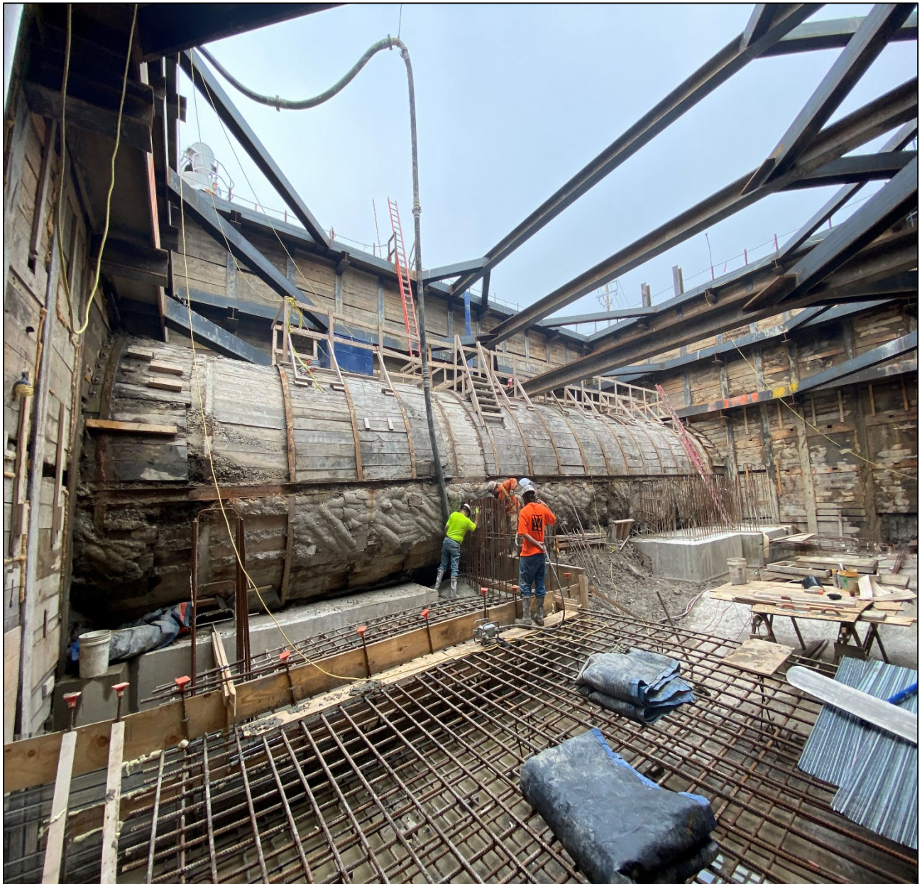
Figure 8 – Placing Concrete Foundation via Pump @ East Wall of Beaconsfield Shaft
