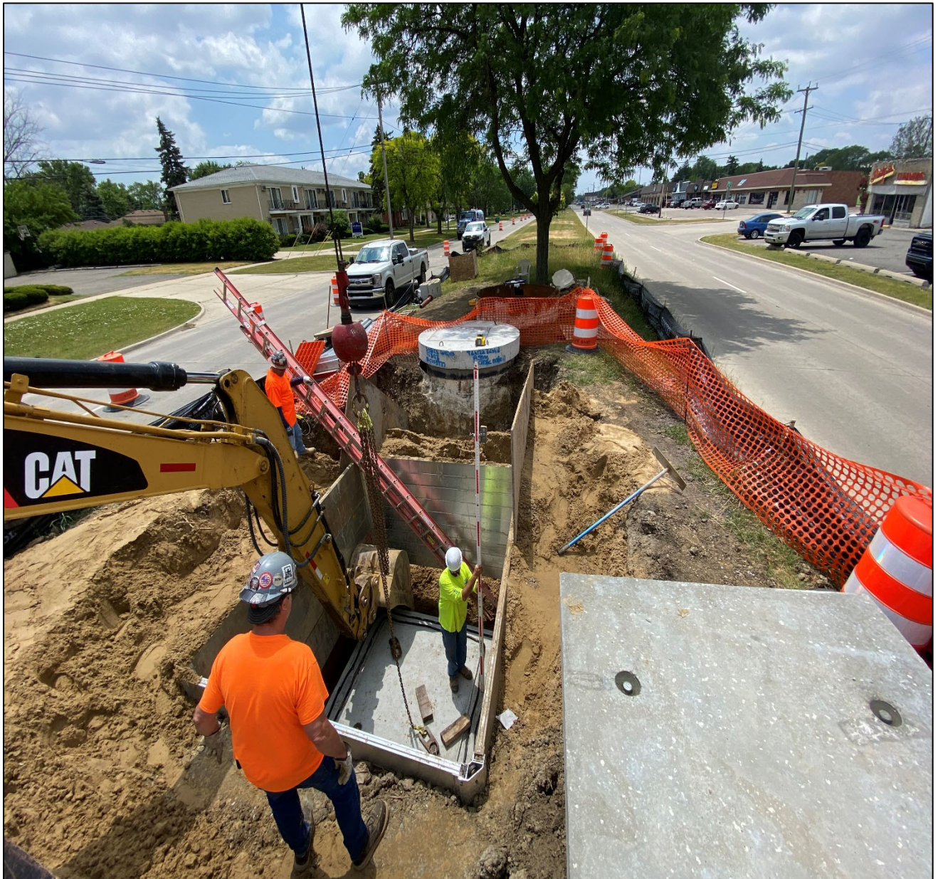
Figure 2 – Odor Control Vault Installation @ Kelly Rd.
