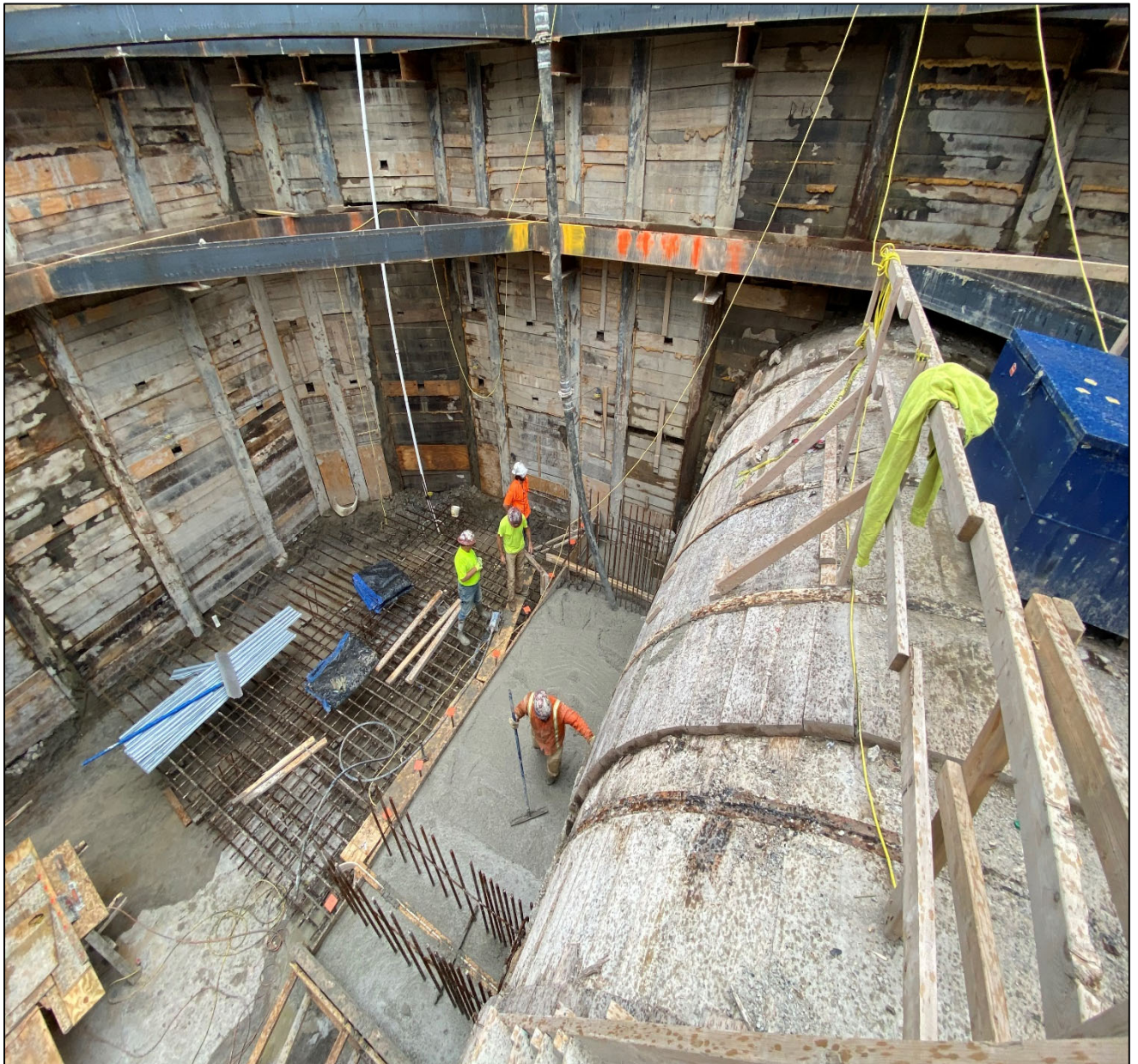
Figure 9 – Placing Concrete Foundation via Pump @ East Wall of Beaconsfield Shaft
