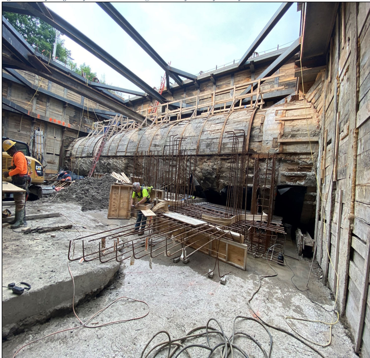
Figure 6 – Reinforcing Steel for New Foundation @ West Wall of Beaconsfield Shaft
