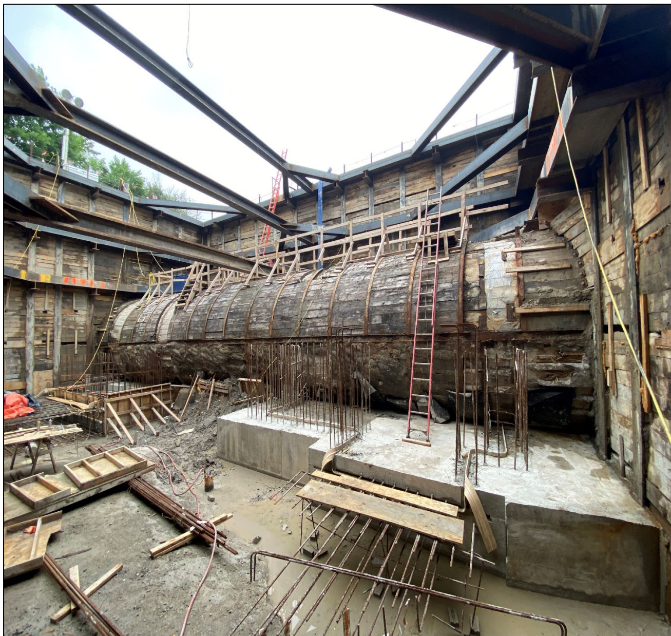
Figure 7 – New Concrete Foundation Support @ West Wall of Beaconsfield Shaft
