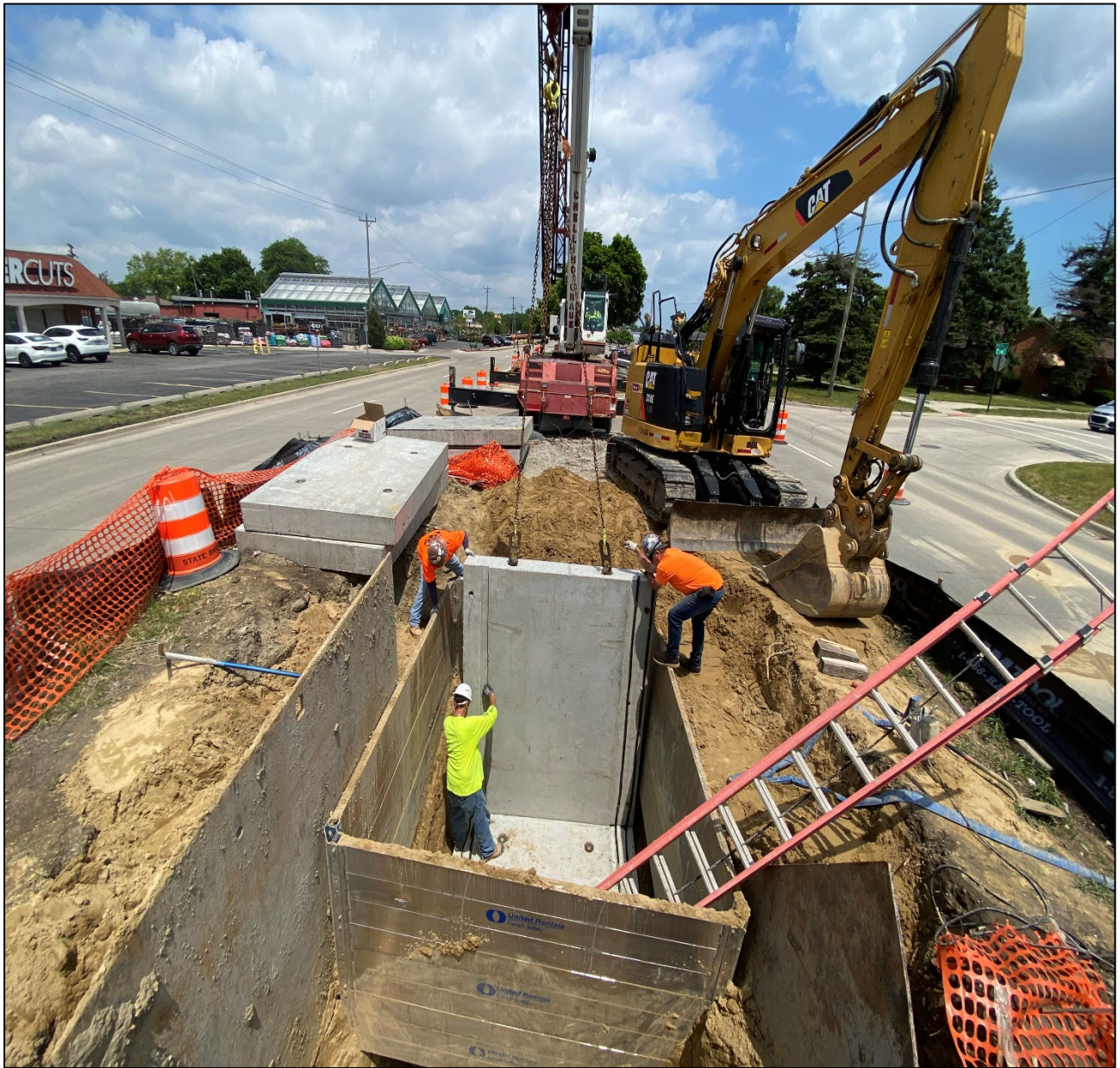
Figure 3 – Odor Control Vault Installation @ Kelly Rd.
