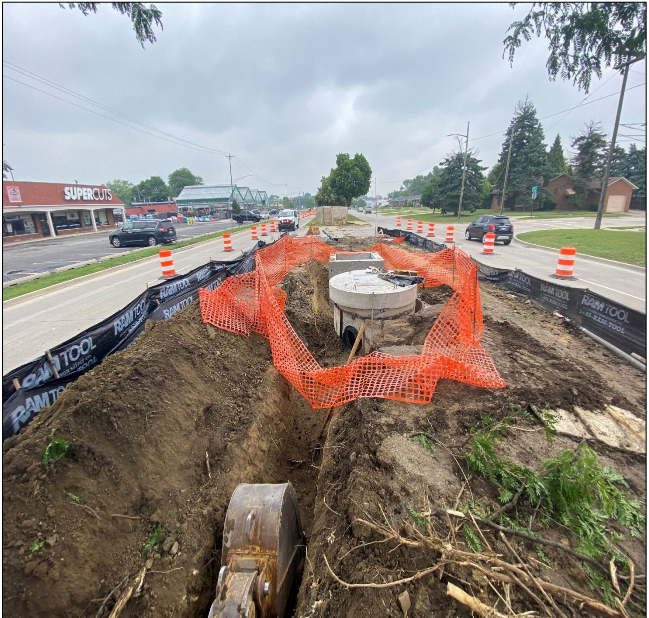
Figure 4 – Odor Control Vent Pipe Excavation @ Kelly Rd.
