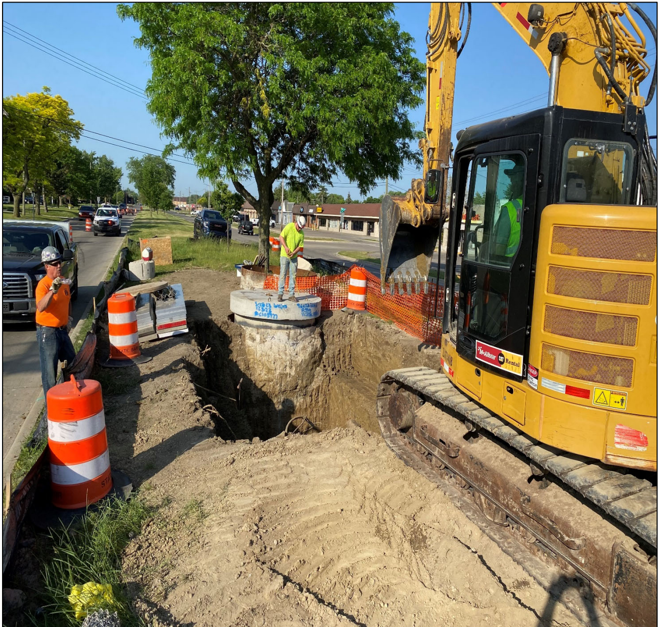
Figure 1 – Odor Control Vault Excavation @ Kelly Rd.
