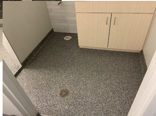
Figure 3 – Mezzanine Bathroom epoxy floor
