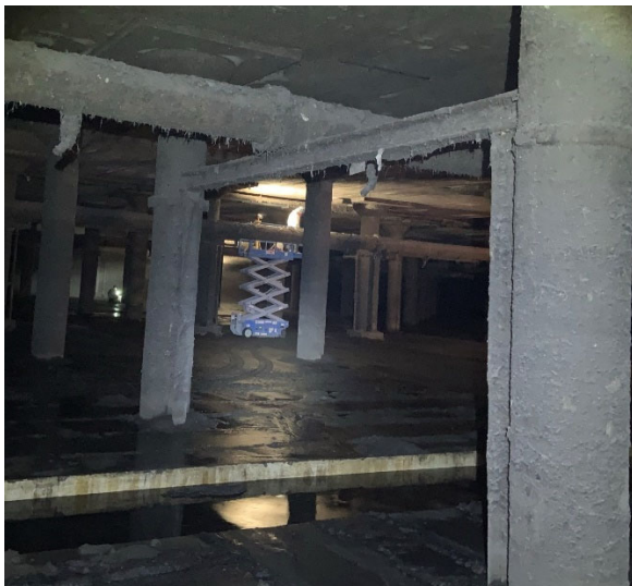
Figure 6 – Crew working on ceiling demolition
