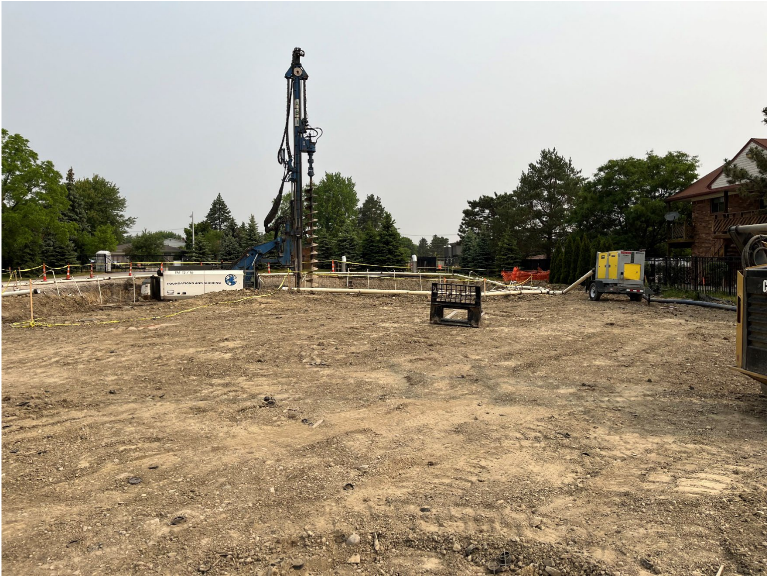
Figure 16 – Fraser Bio-Filter Foundation Drilling
