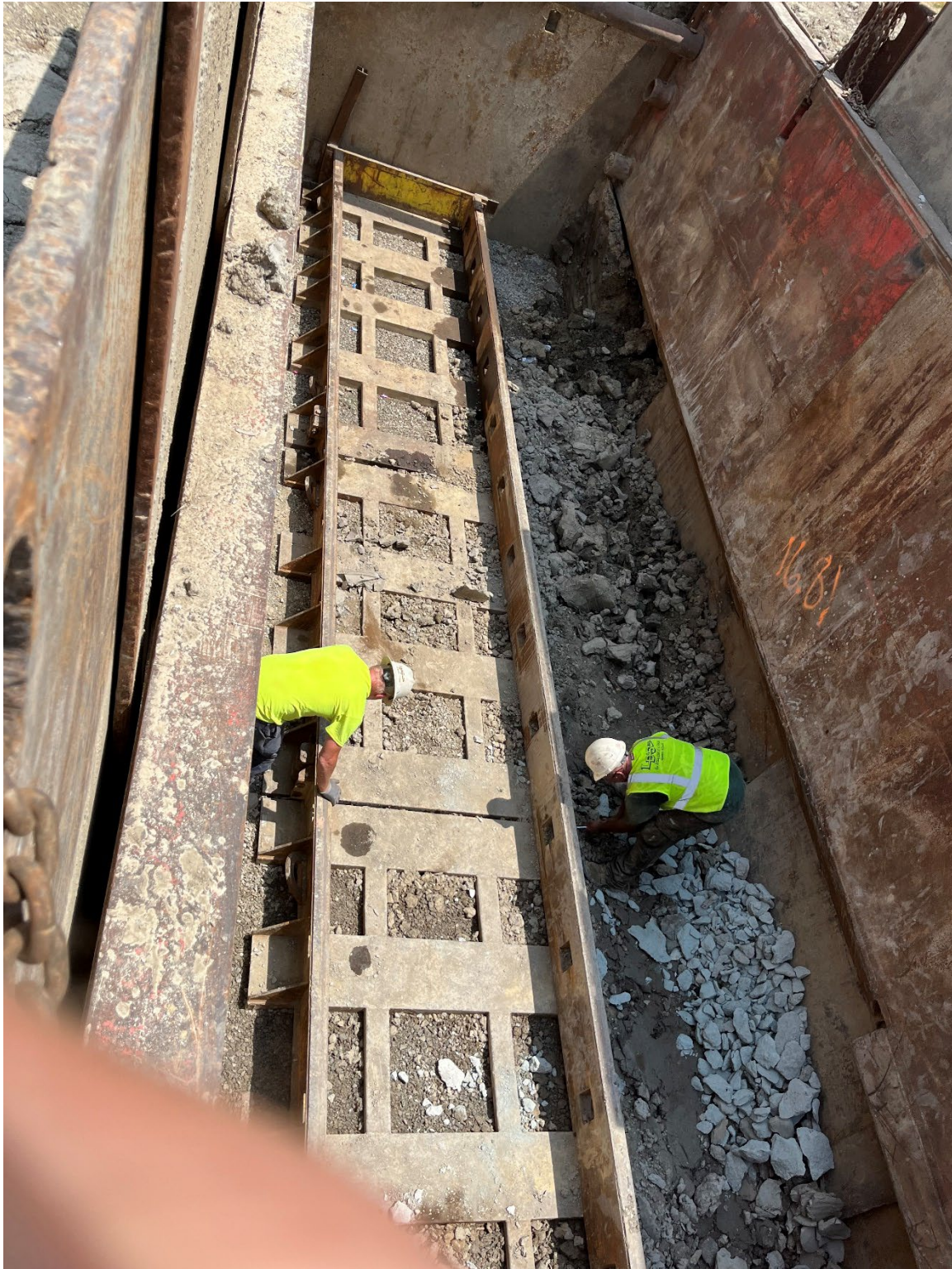
Figure 15 – Setting up rails for Jack & Bore Equipment
