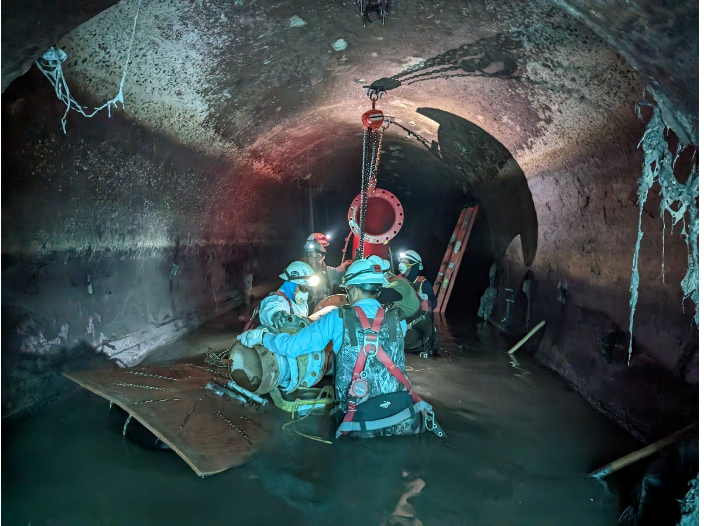
Figure 4 – Temp Pump for Dewatering to Remove Flume
