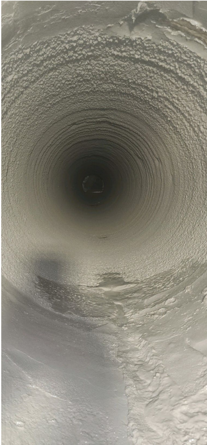
Figure 11 – SY-S-3 West Side) After Pipe Lining
