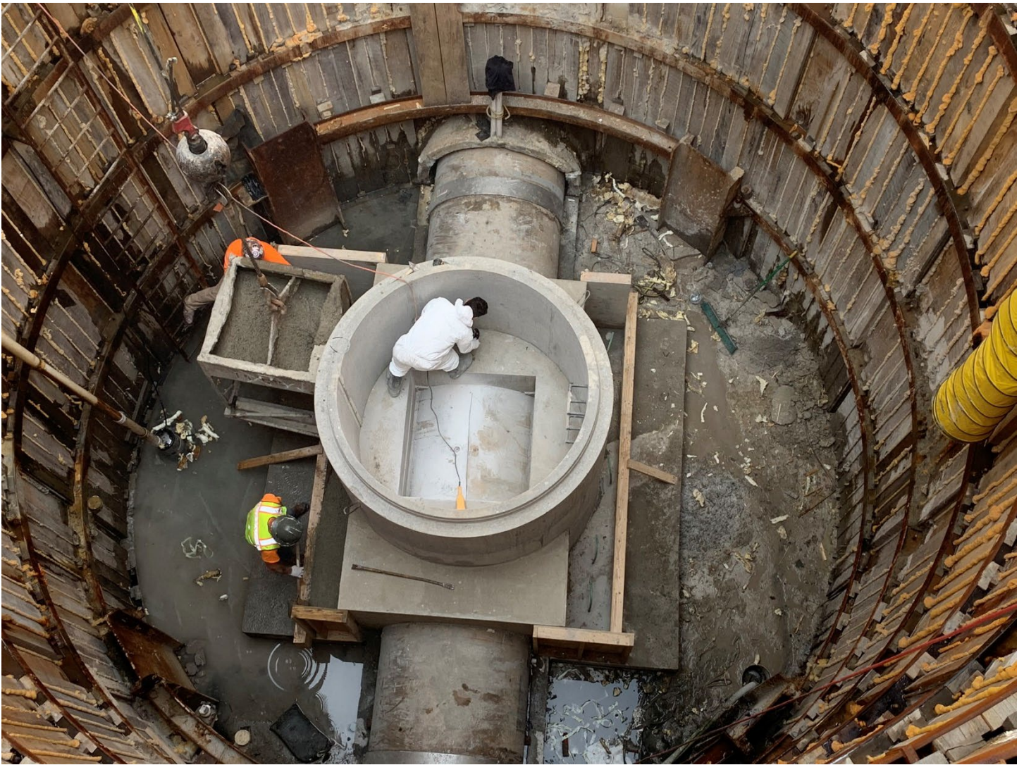
Figure 8 – Constructing Manhole at Lining Shaft
