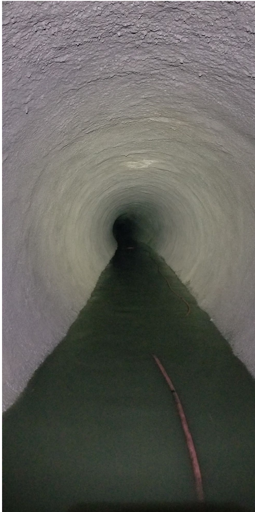
Figure 2 – Spray-Lined Section of 8-foot Pipe
