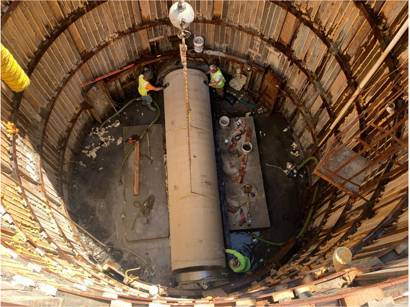
Figure 7 – Setting Final Section of 54-inch HOBAS
