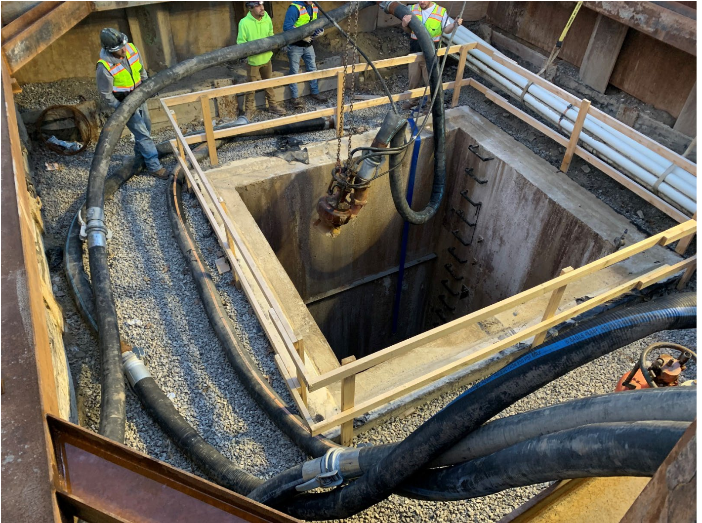
Figure 6 – Lowering Pump into CS-2 for Dewatering
