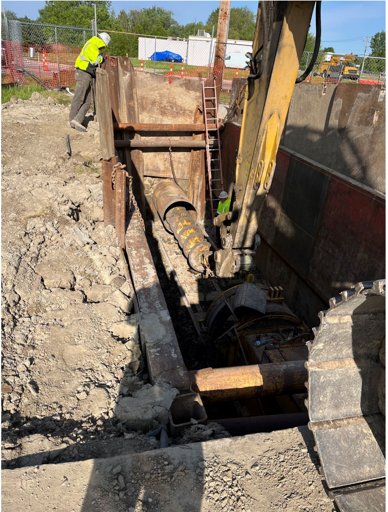
Figure 14 – 21 & Garfield – Jack & Bore for FAD
