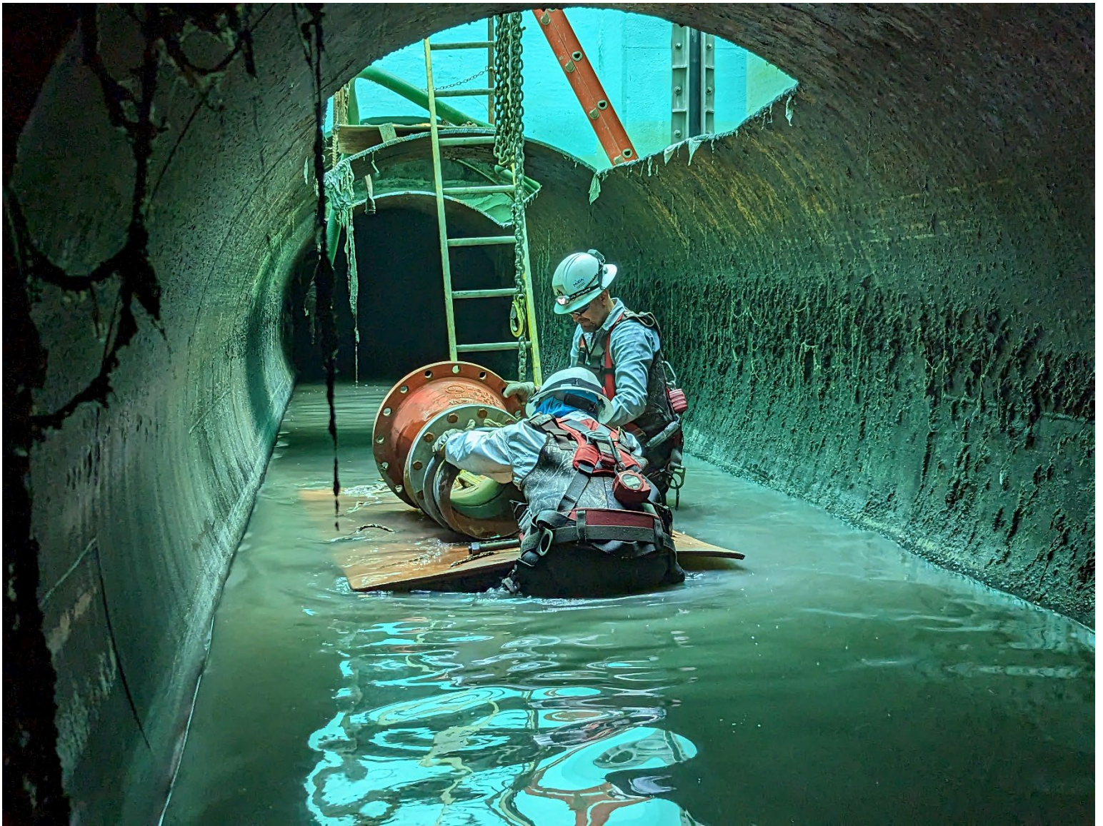
Figure 3 – Temp Pump to Dewater for Flume Removal
