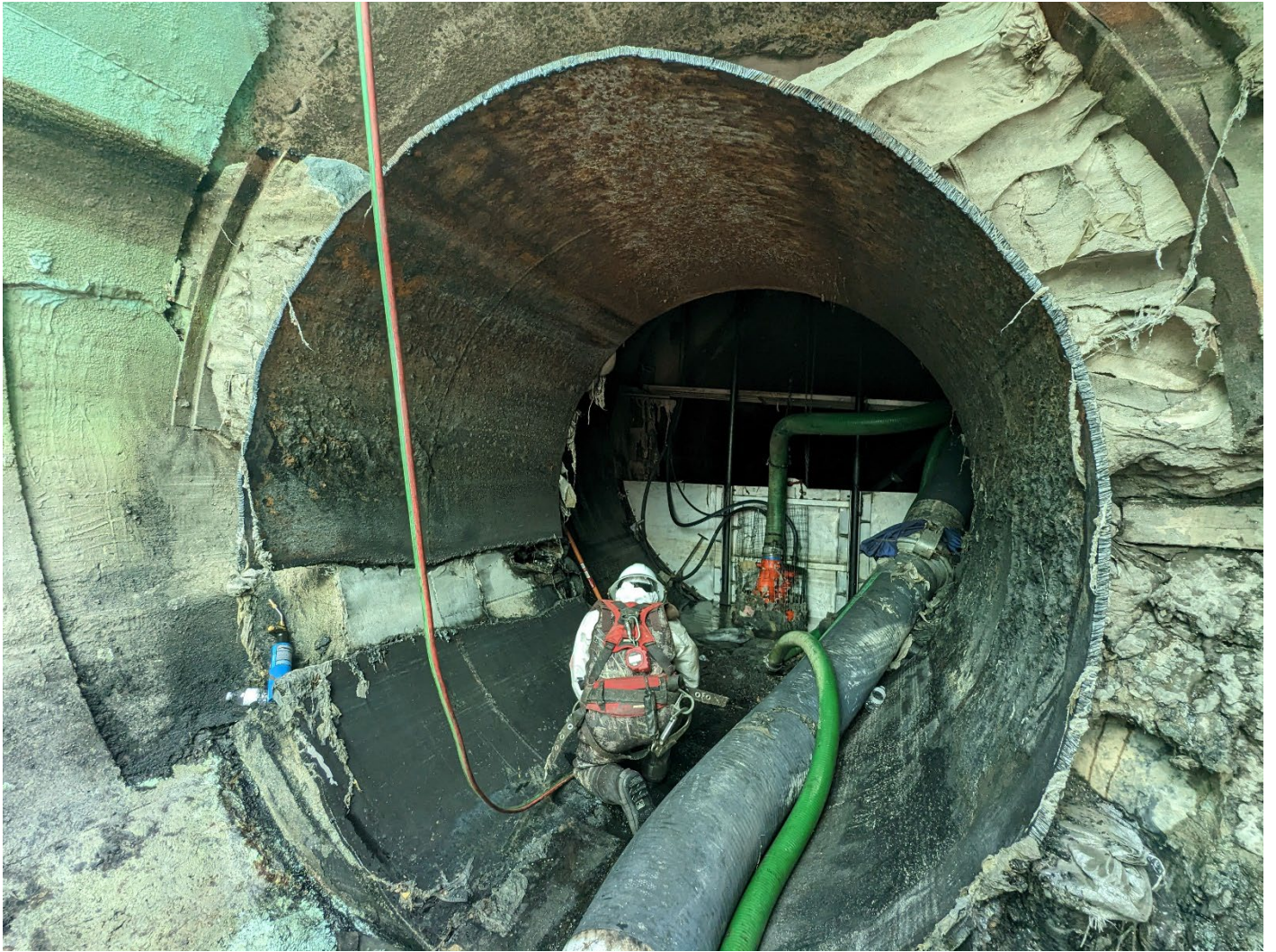
Figure 5 – Temporary Flume Removal
