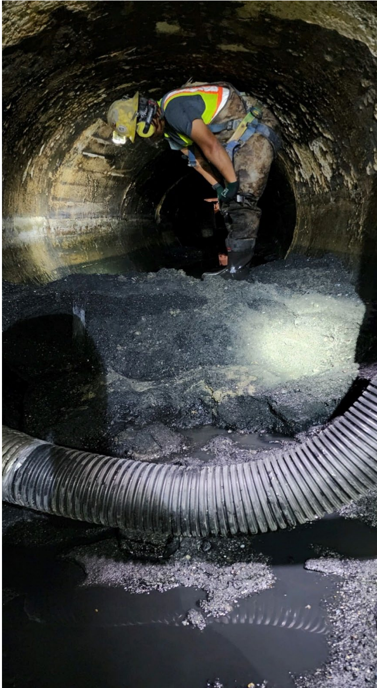
Figure 9 – MA-S-2 (East Side) Sediment Removal
