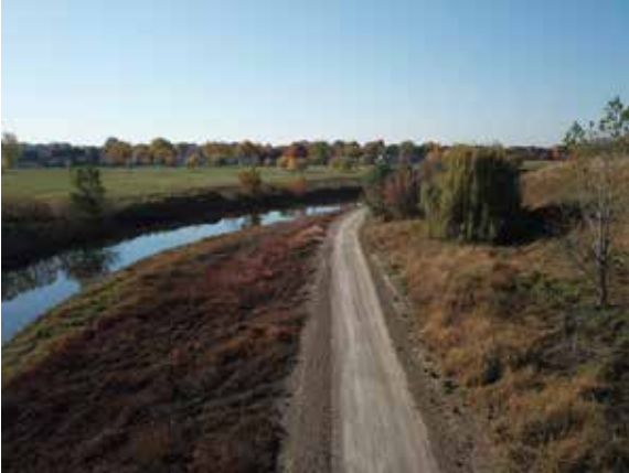
The completed hike/bike trail along the Red Run Drain portion of the 1.35-mile path
