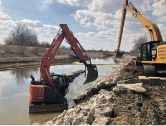
Construction of “j-hooks” in the red run drain
