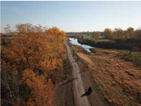
The completed hike/bike trail along the Sterling Relief Drain portion of the 1.35-mile path
