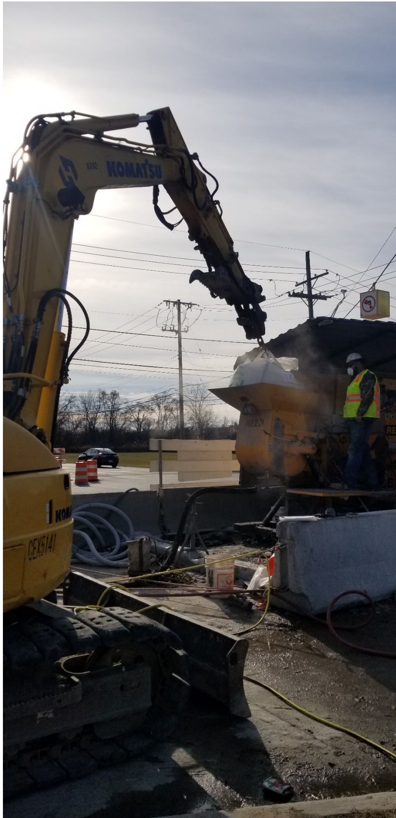
Figure 7 – CT-S-7 Spray-Lining – Mixing GeoKrete
