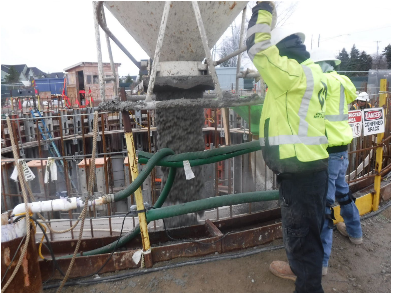
Figure 2 - CS-12 Concrete Placement
