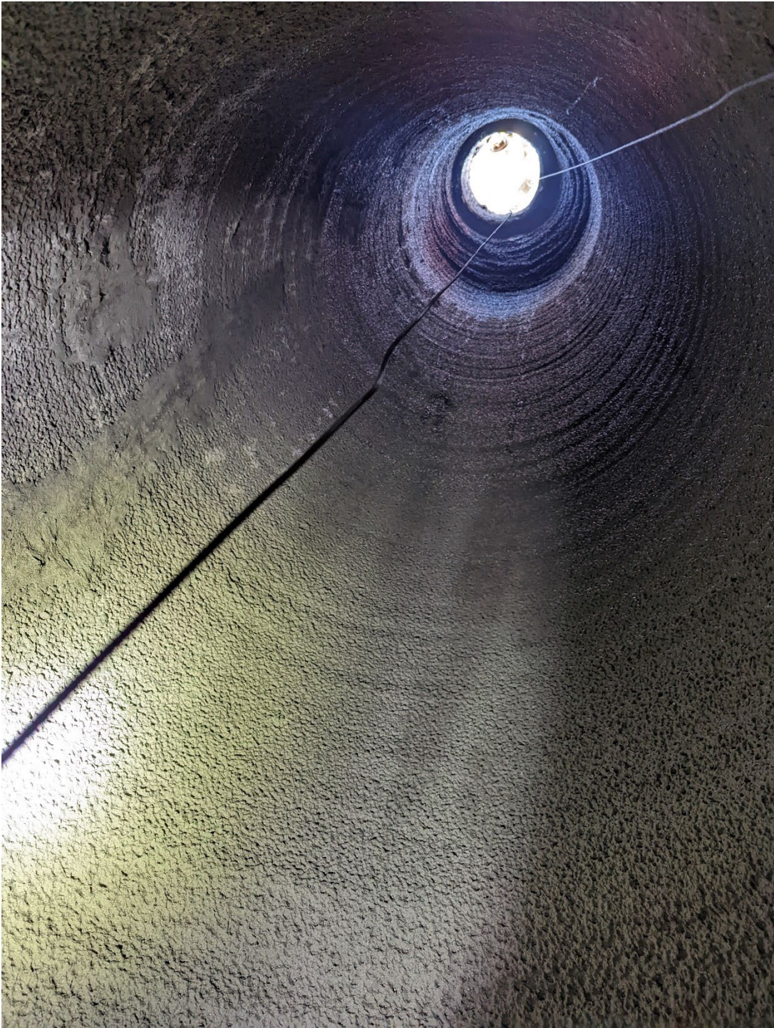
Figure 6 – CT-S-7 Drop Manhole Spray-Lining
