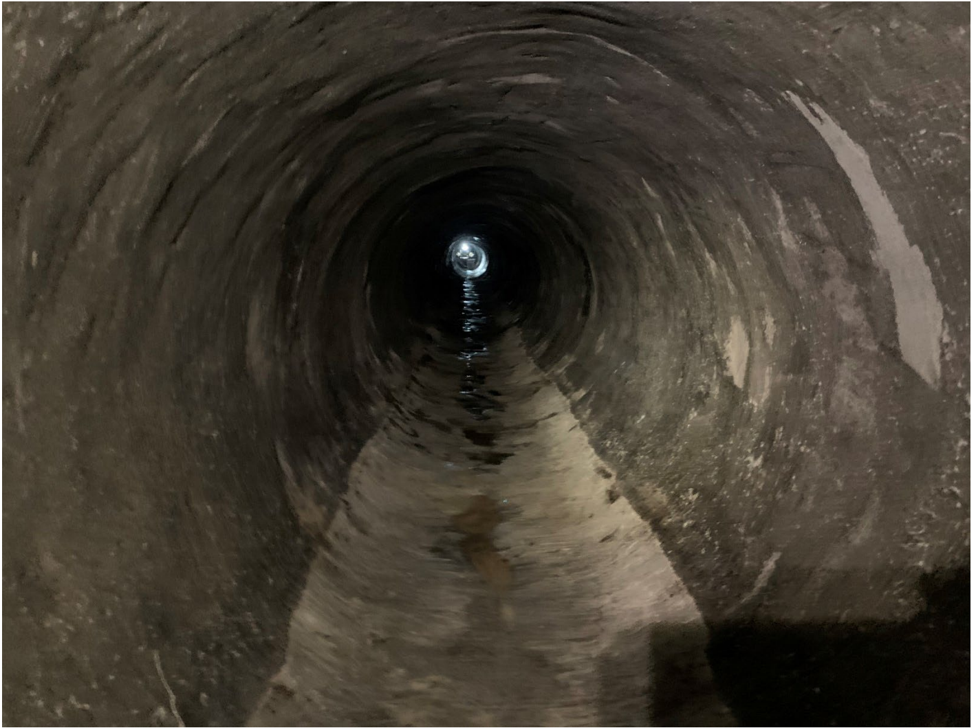
Figure 12 – FR-S-1 Connecting Sewer Pre-Spray-Lining
