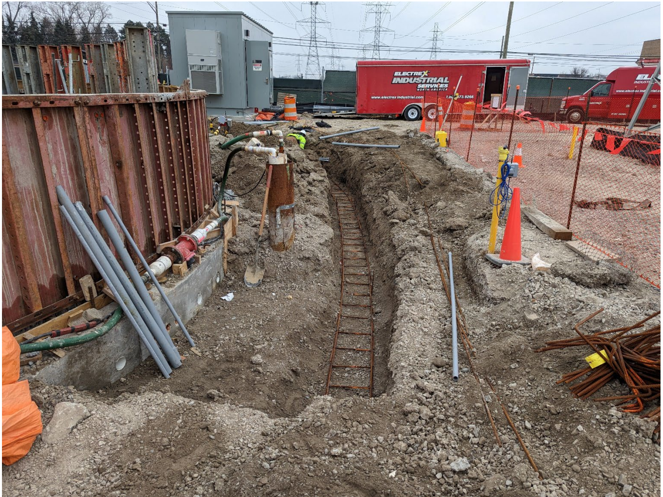
Figure 5 - CS-12 Electrical Conduit Installation for Pumps
