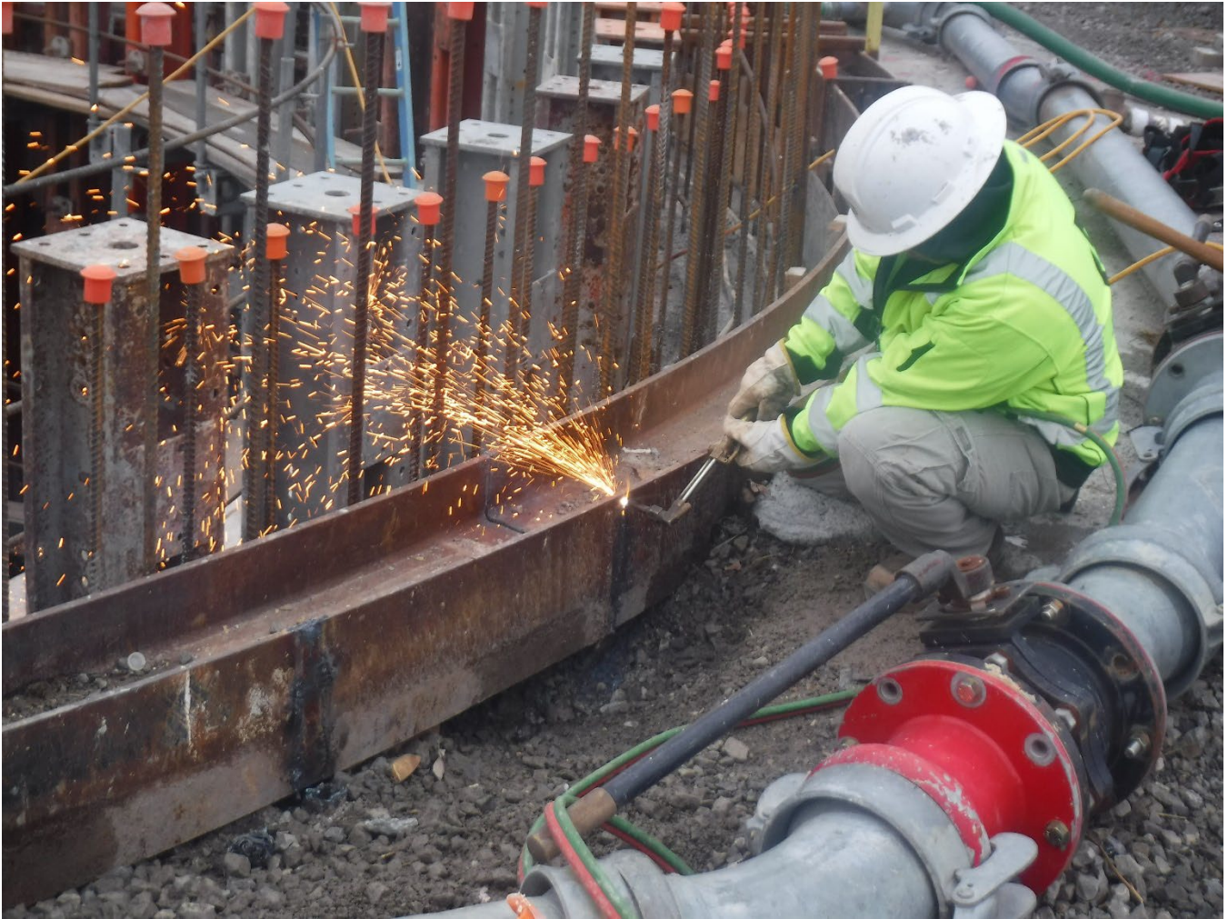
Figure 4 - CS-12 Upper TERS Removal
