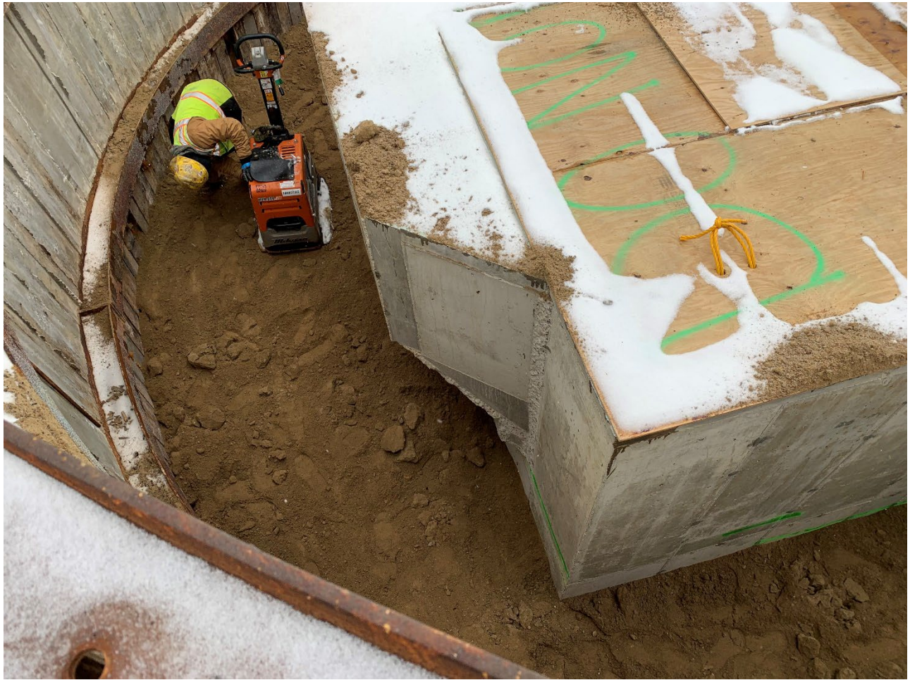
Figure 14 – CS-13 Sand Back-fill Operation
