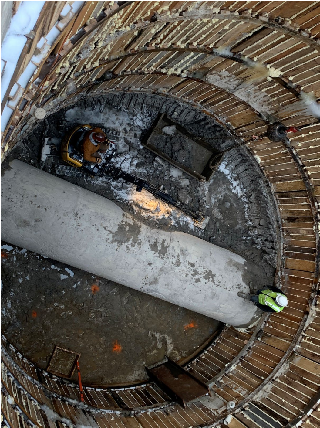
Figure 10 – Lining Completion Shaft Excavation
