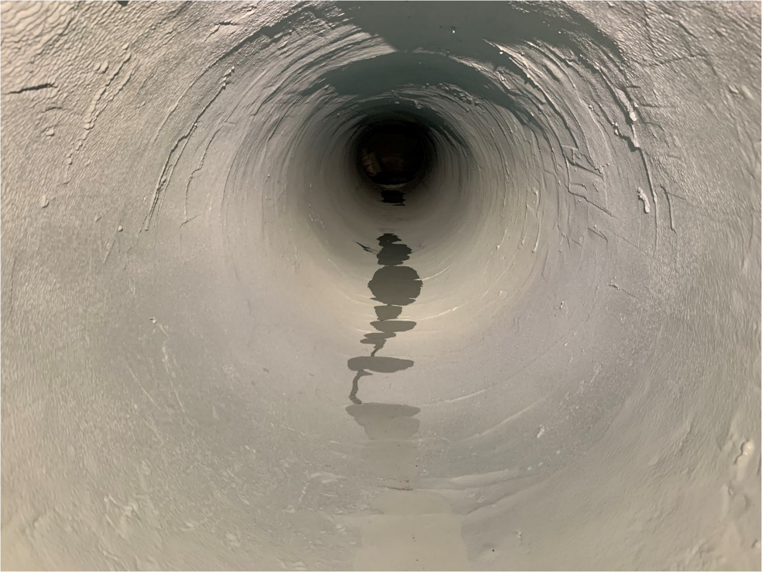
Figure 13 – FR-S-1 Connecting Sewer Post-Spray-Lining
