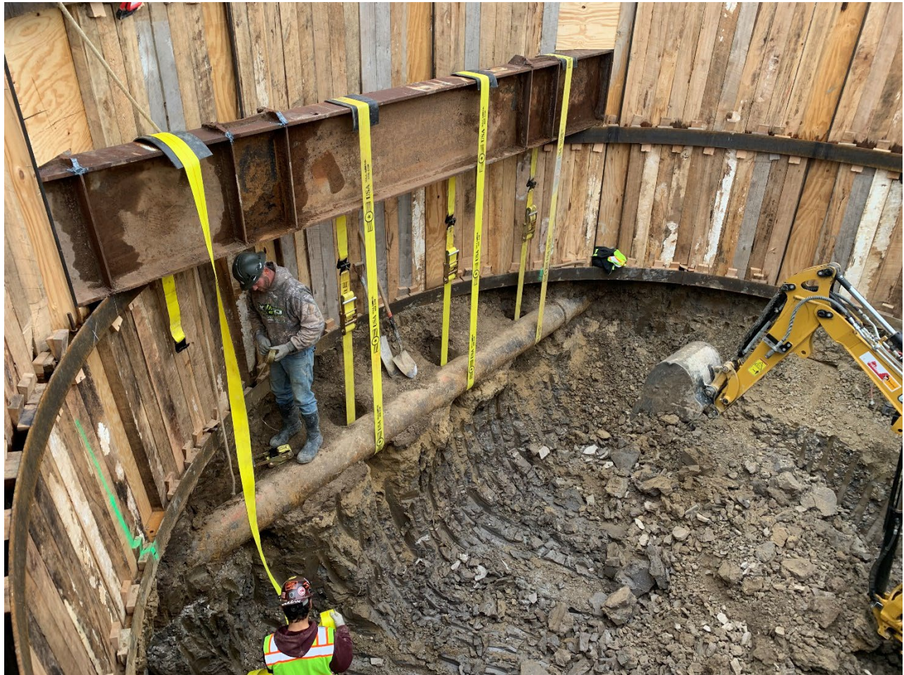
Figure 8 – Lining Completion Shaft Excavation – Supporting an Existing Watermain
