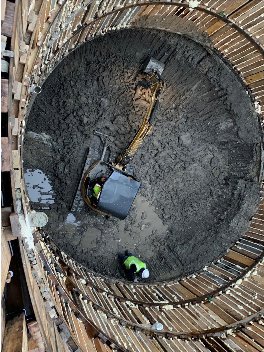
Figure 9 – Lining Completion Shaft Excavation
