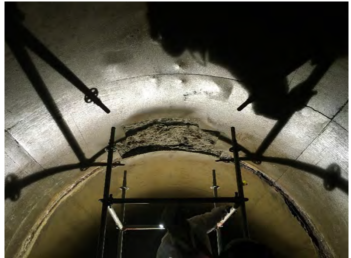
Figure 2 – 8.5 Mile Drain – Ceiling and Leaking Joint Repairs
