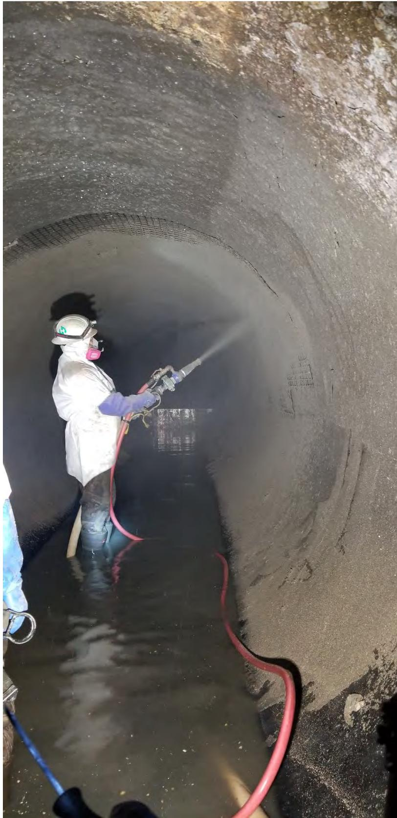
*Figure 9 - Spray-Lining Outer Layer*
