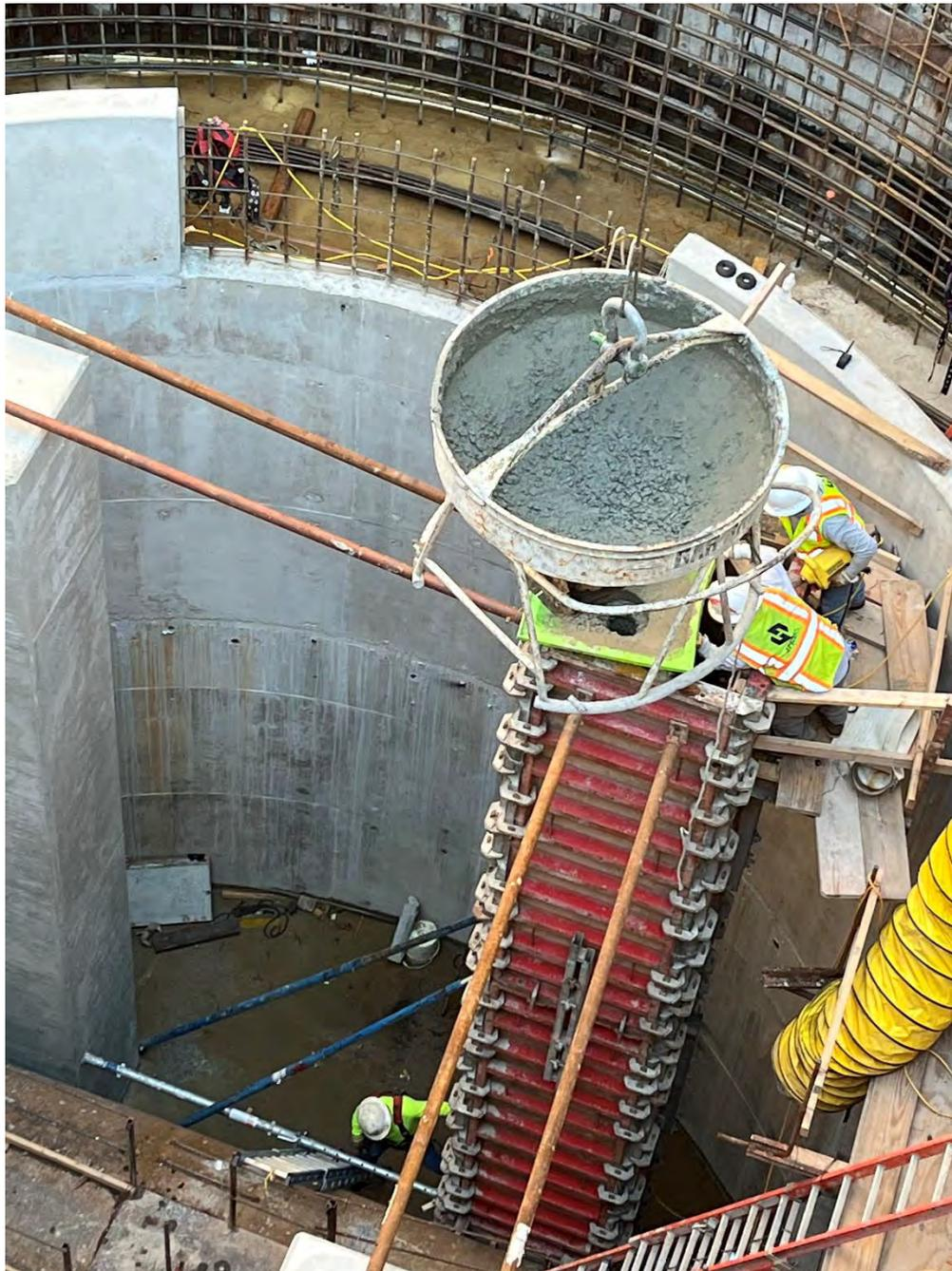
*Figure 2 - CS-12 Concrete Placement for Column 4*
