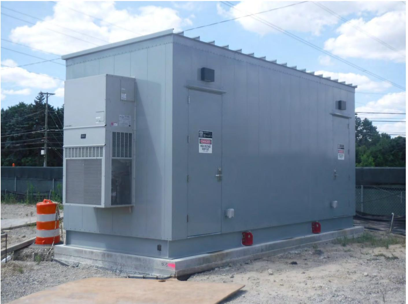
*Figure 13 - CS-12 Pump Station MCC Enclosure*
