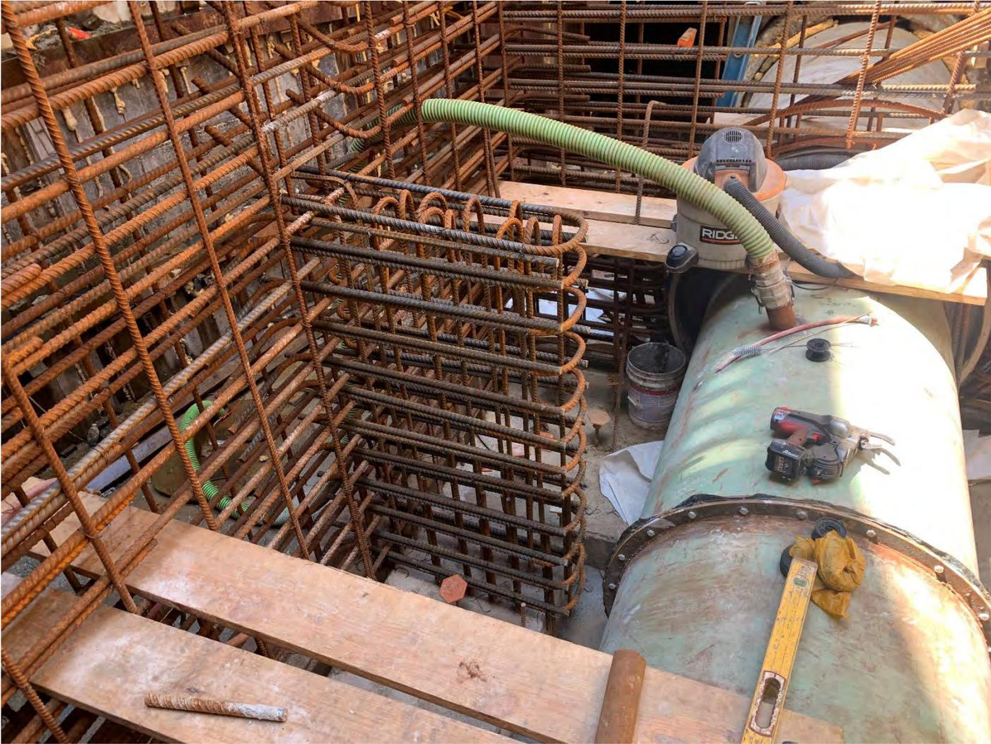
*Figure 16 - CS-13 Construction - Wall Lift #1 Rebar Installation*
