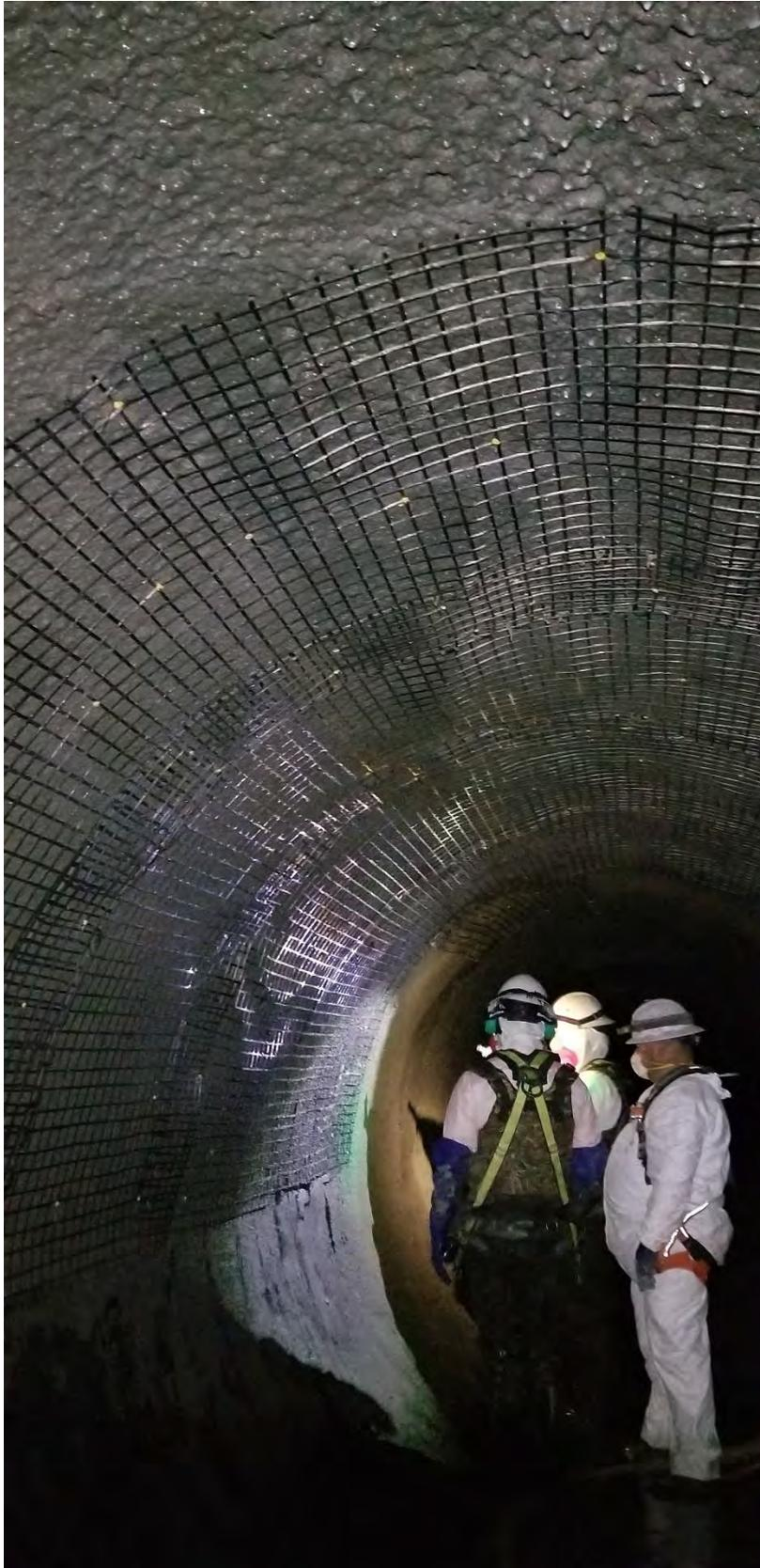
*Figure 8 - Installation of C-Grid*
