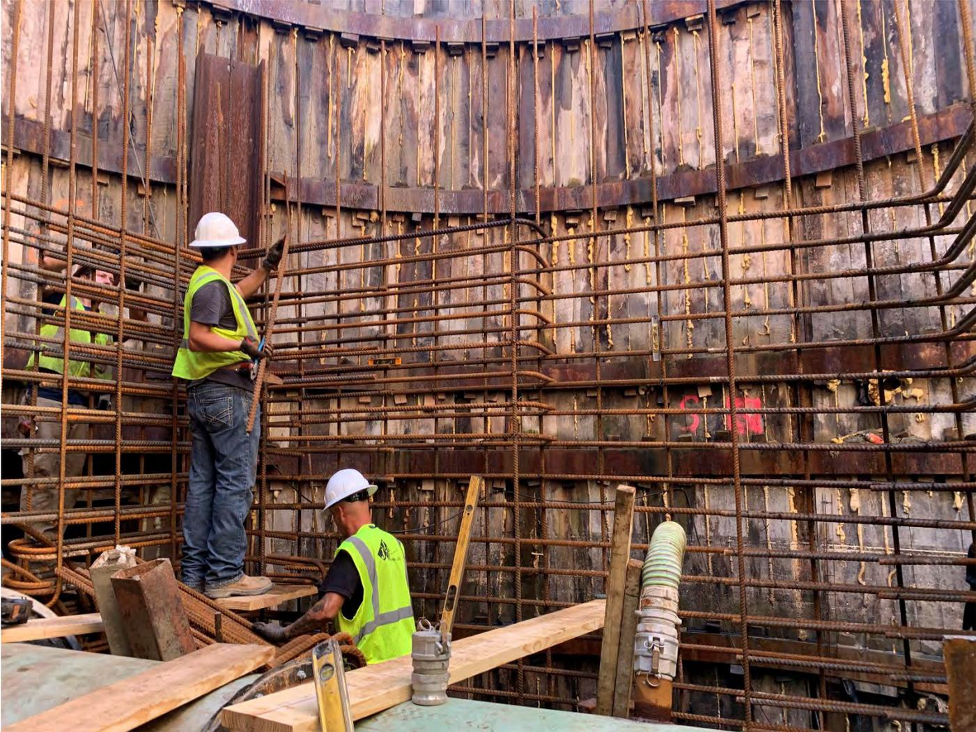
*Figure 15 - CS-13 Construction - Wall Lift #1 Rebar Installation*
