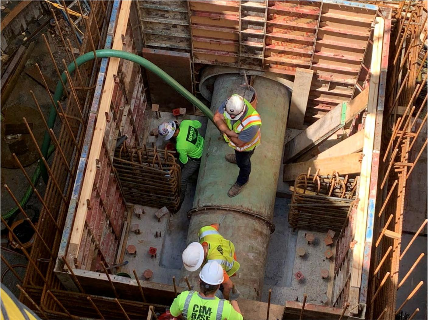
*Figure 17 - CS-13 Construction - Wall Lift #1 Concrete Formwork*
