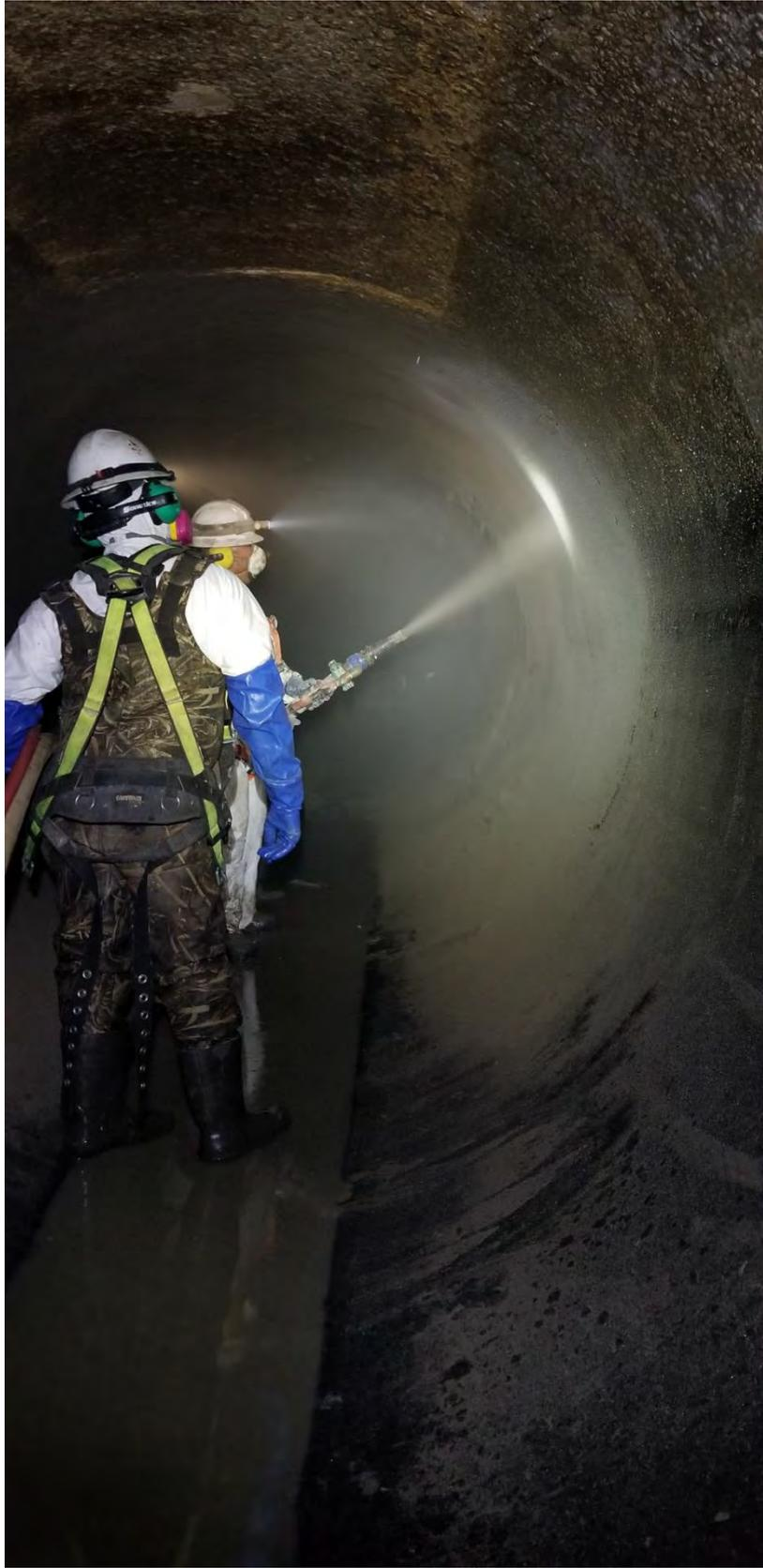
*Figure 7 - Spray-Lining Base Layer*
