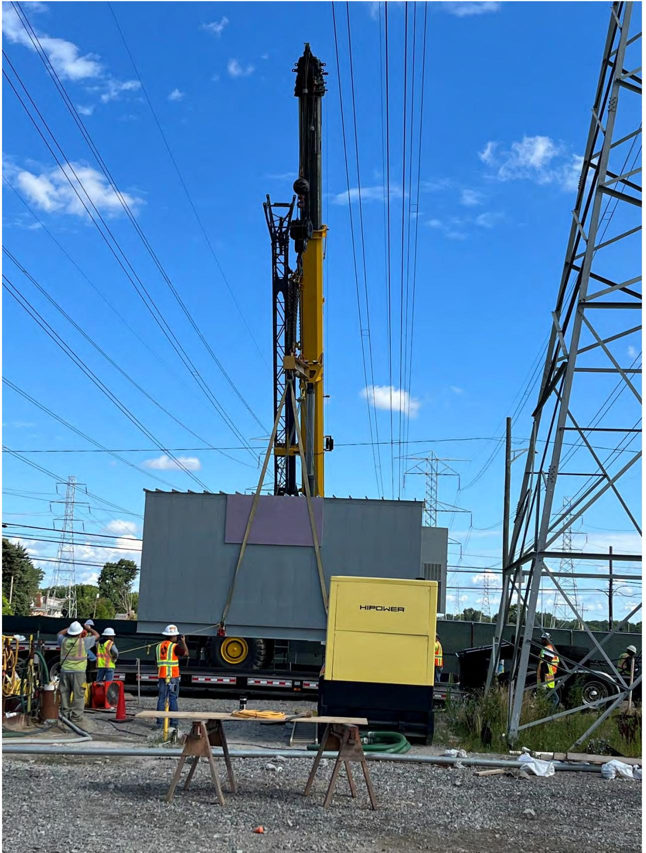
*Figure 12 - CS-12 Pump Station MCC Enclosure*
