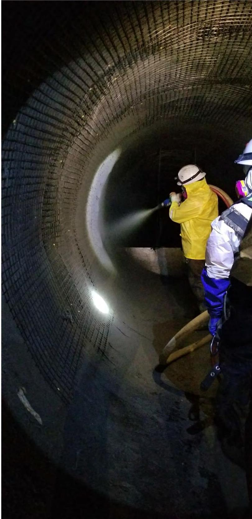
*Figure 10 - Spray-Lining Outer Layer*
