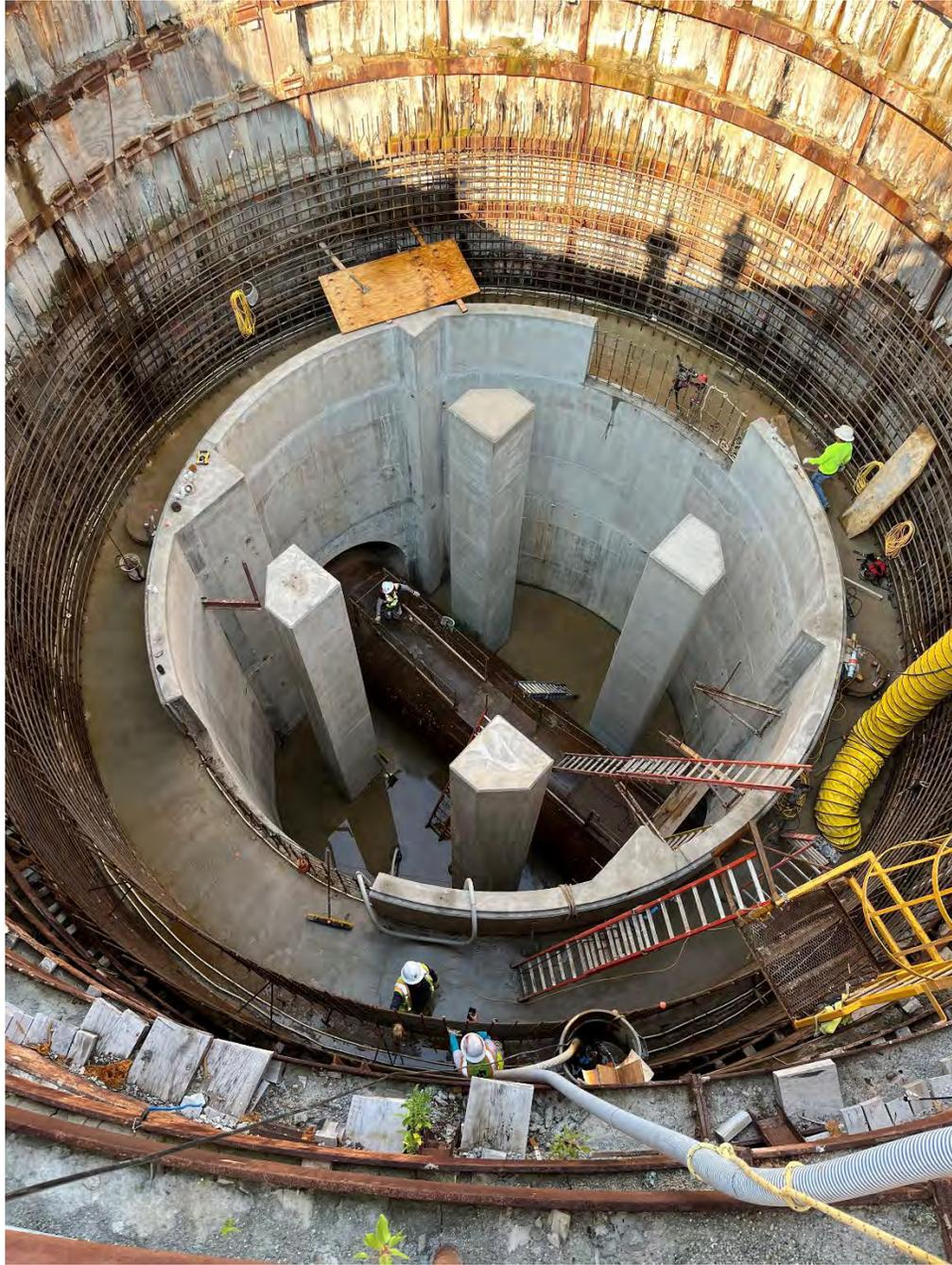
*Figure 3 – CS-12 Post Column 4 Form Removal*
