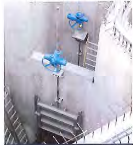
Gate installation at control structure
