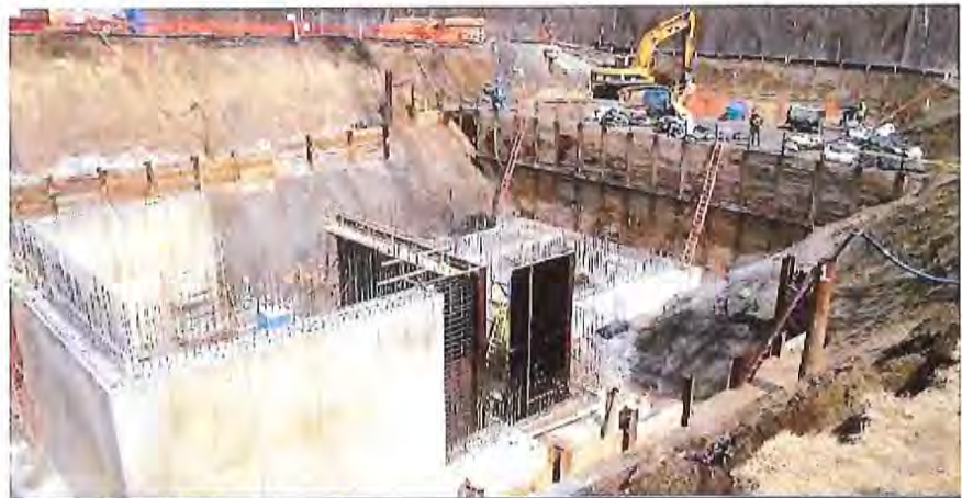
Construction of the Perry Street Pump Station, Oakland County, MI
