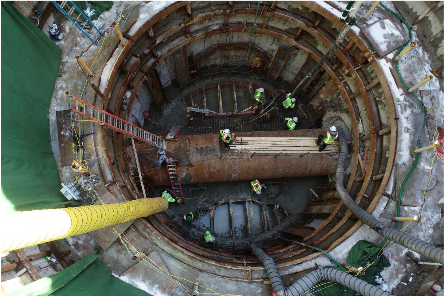
Figure 8 - Finishing Concrete Base Slab in CS-12
