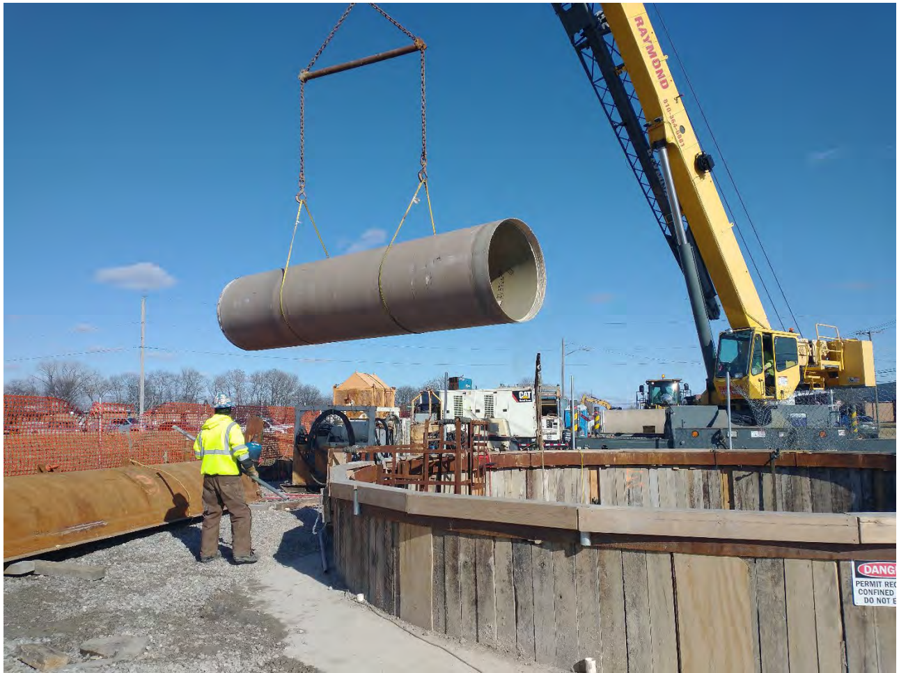
Figure 13 – Hoisting HOBAS into CS-13 Shaft
