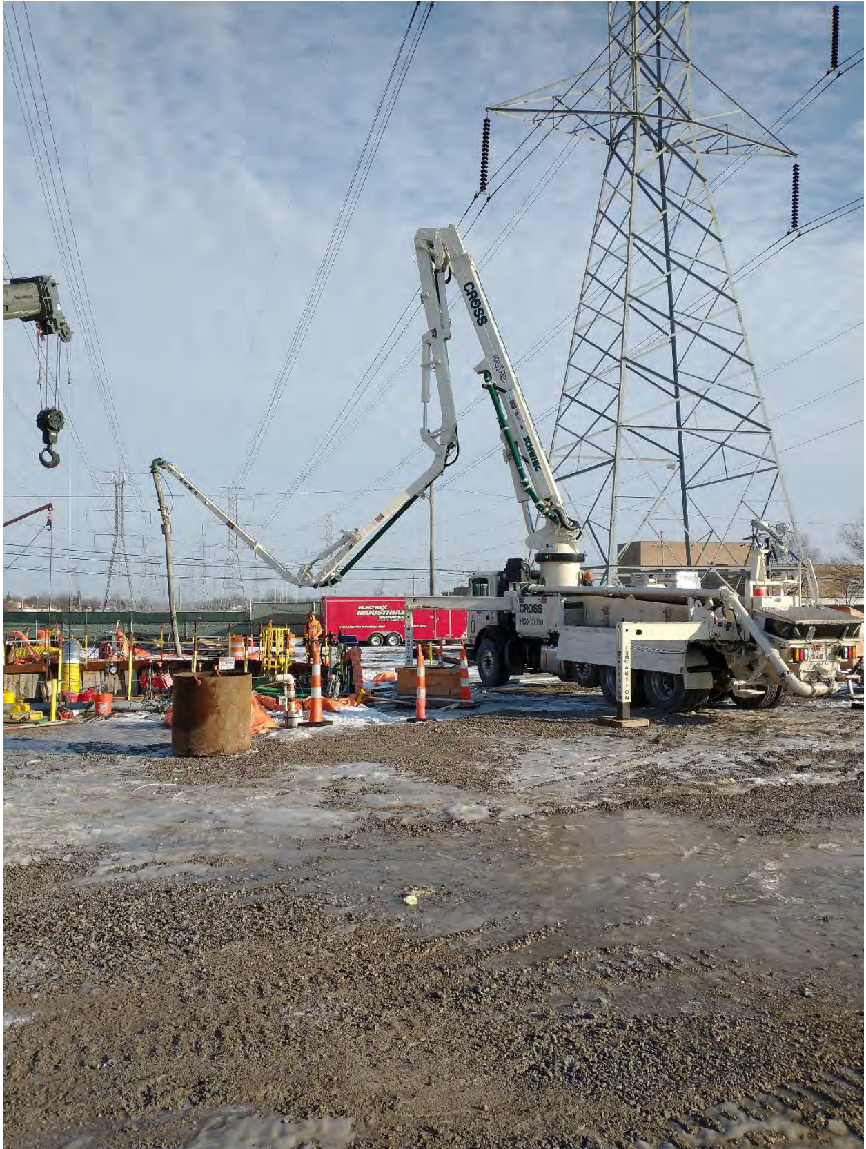
Figure 5 – Concrete Pump Truck
