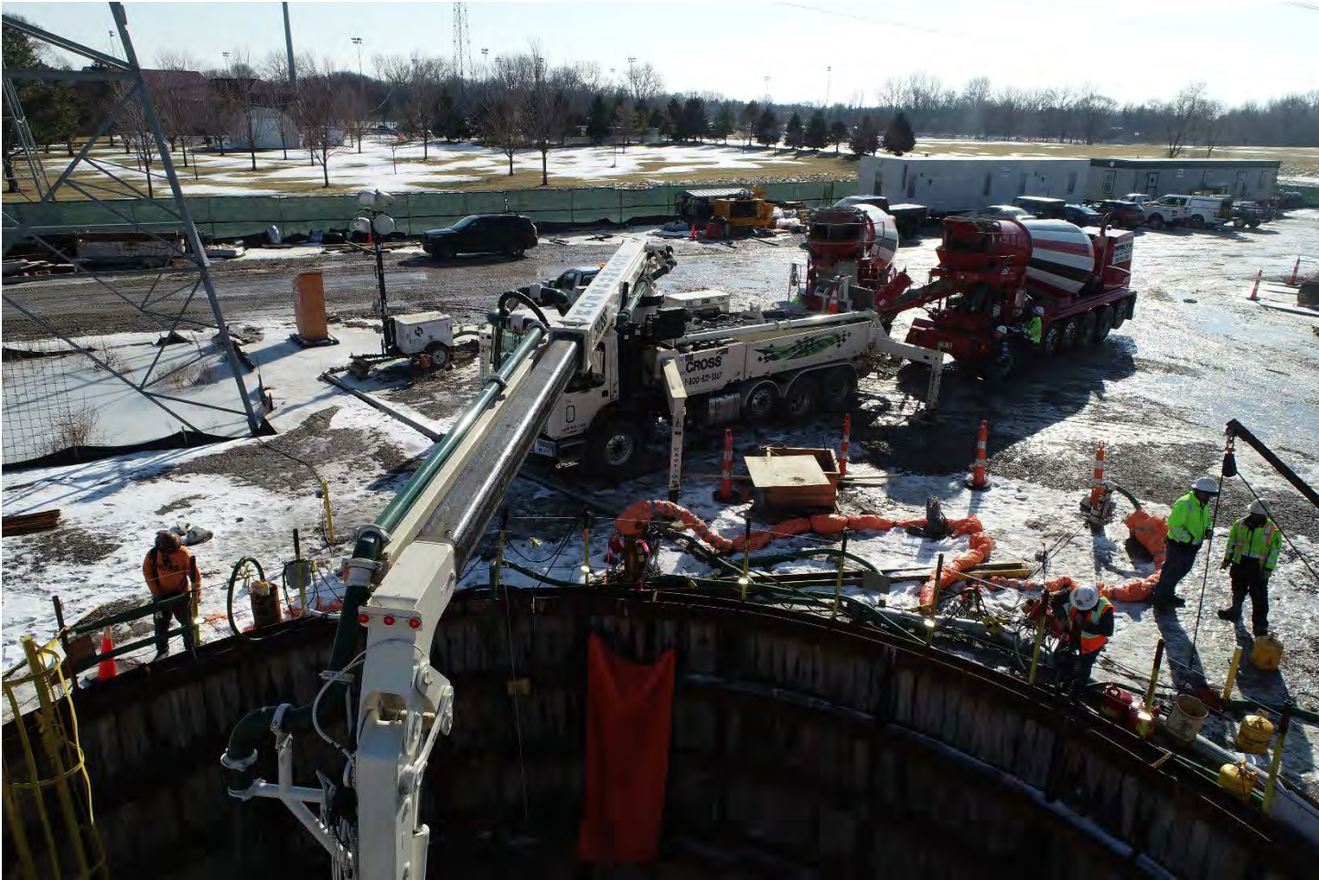
Figure 7 - Aerial View of Concrete Pump Truck
