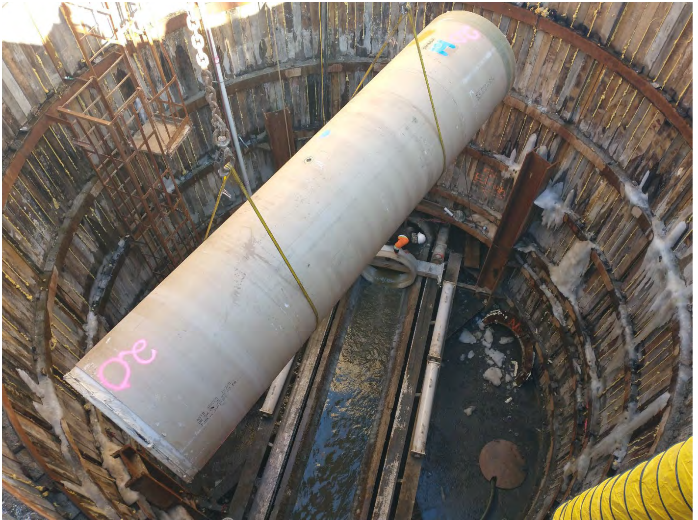
Figure 14 – Hoisting HOBAS into the CS-13 Shaft
