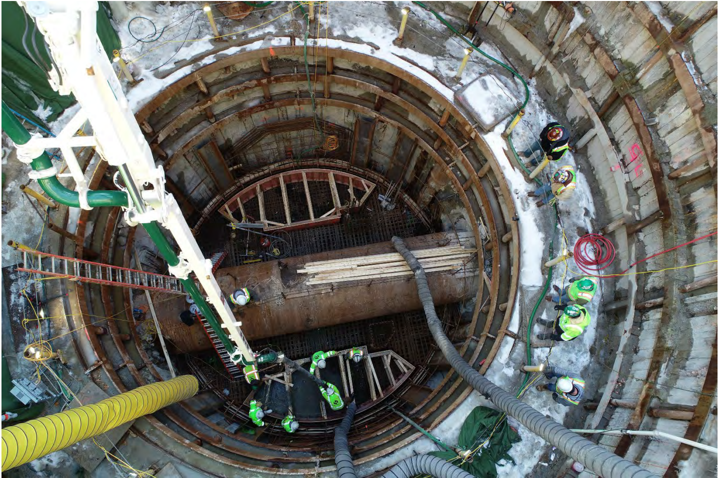
Figure 6 - Aerial View of CS-12 Base Slab Concrete Placement
