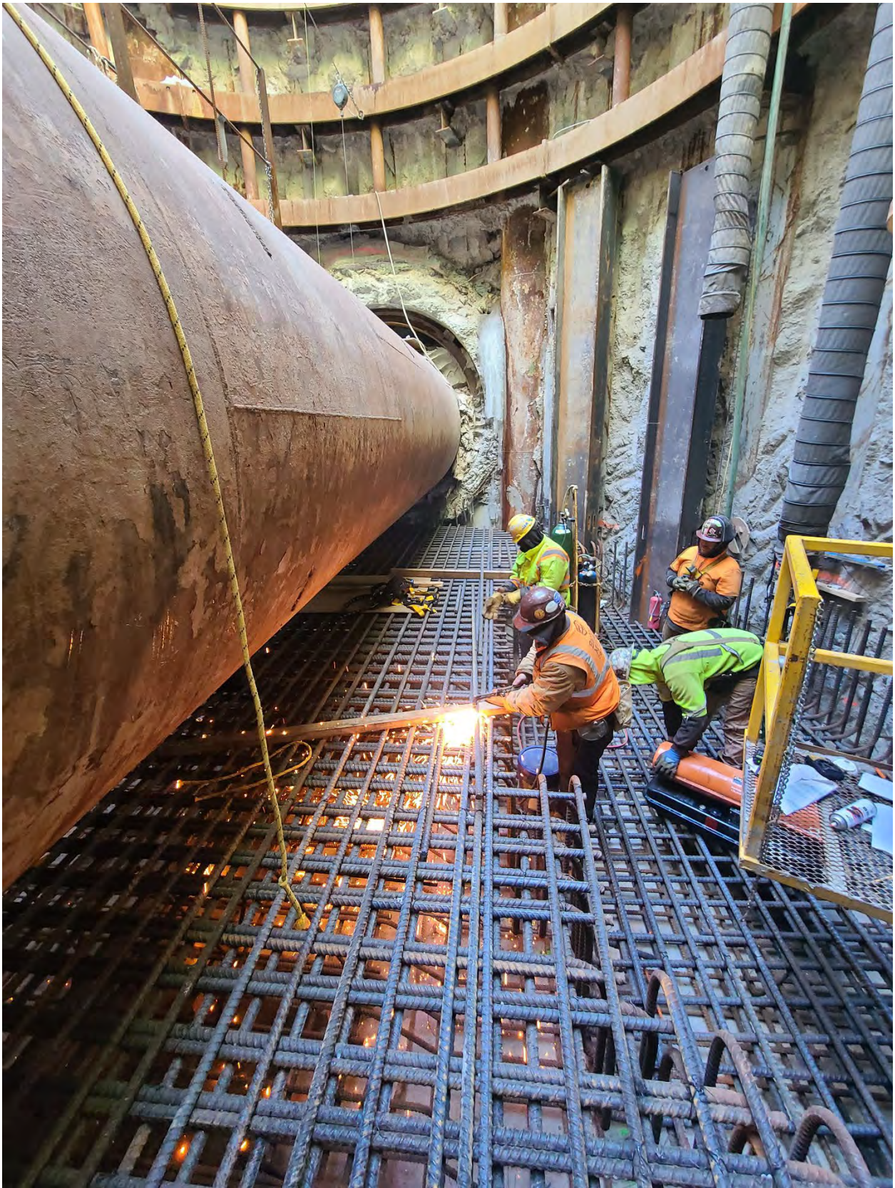
Figure 1 – Rebar Installation for the CS-12 Base Slab
