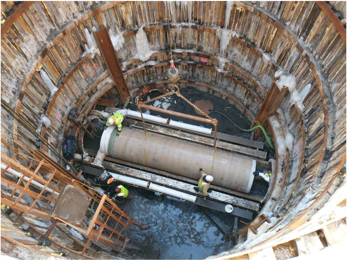
Figure 16 – Jacking HOBAS into the Interceptor
