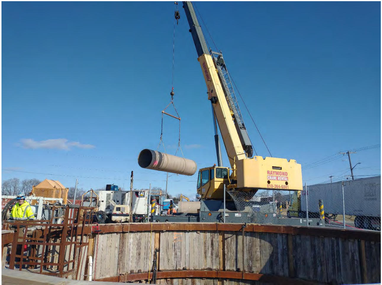
Figure 12 - Hoisting HOBAS into CS-13 Shaft
