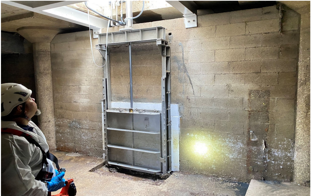
Figure 2 - Installed New Flushing Gates to Intermediate Basin Wall
