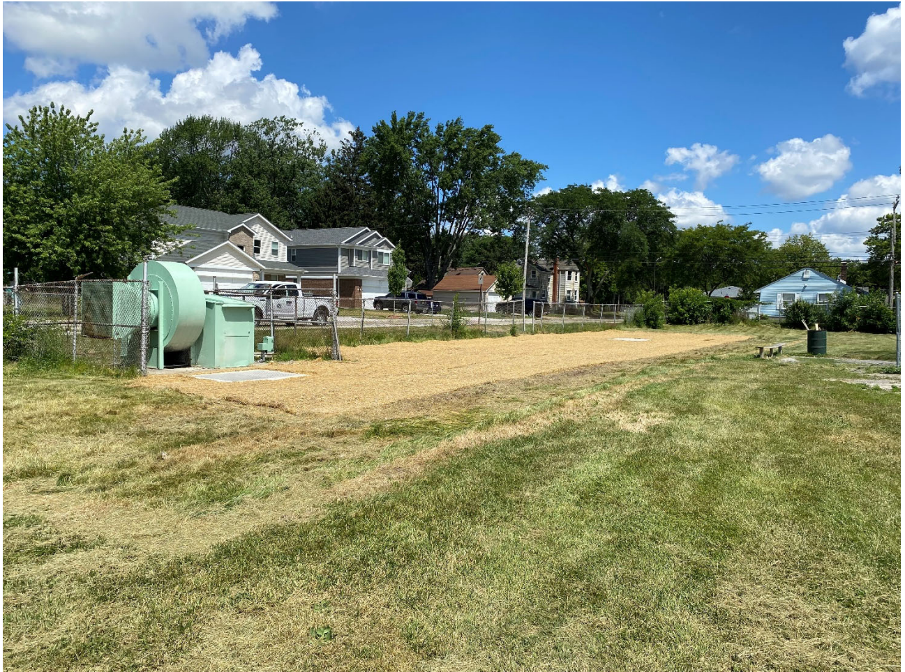
Figure 4 – Placed Topsoil and Straw Seed Blankets
