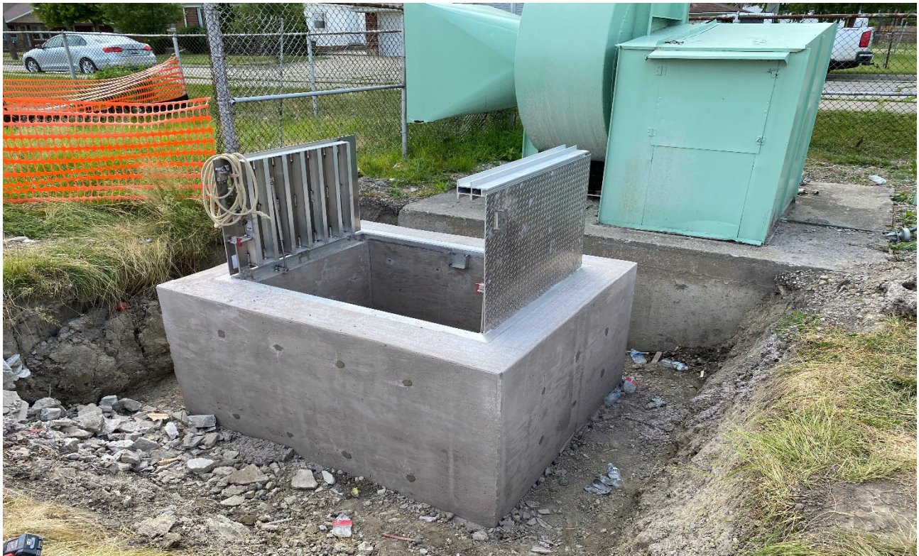
Figure 1 – New Basin Access Hatches and Concrete Risers
