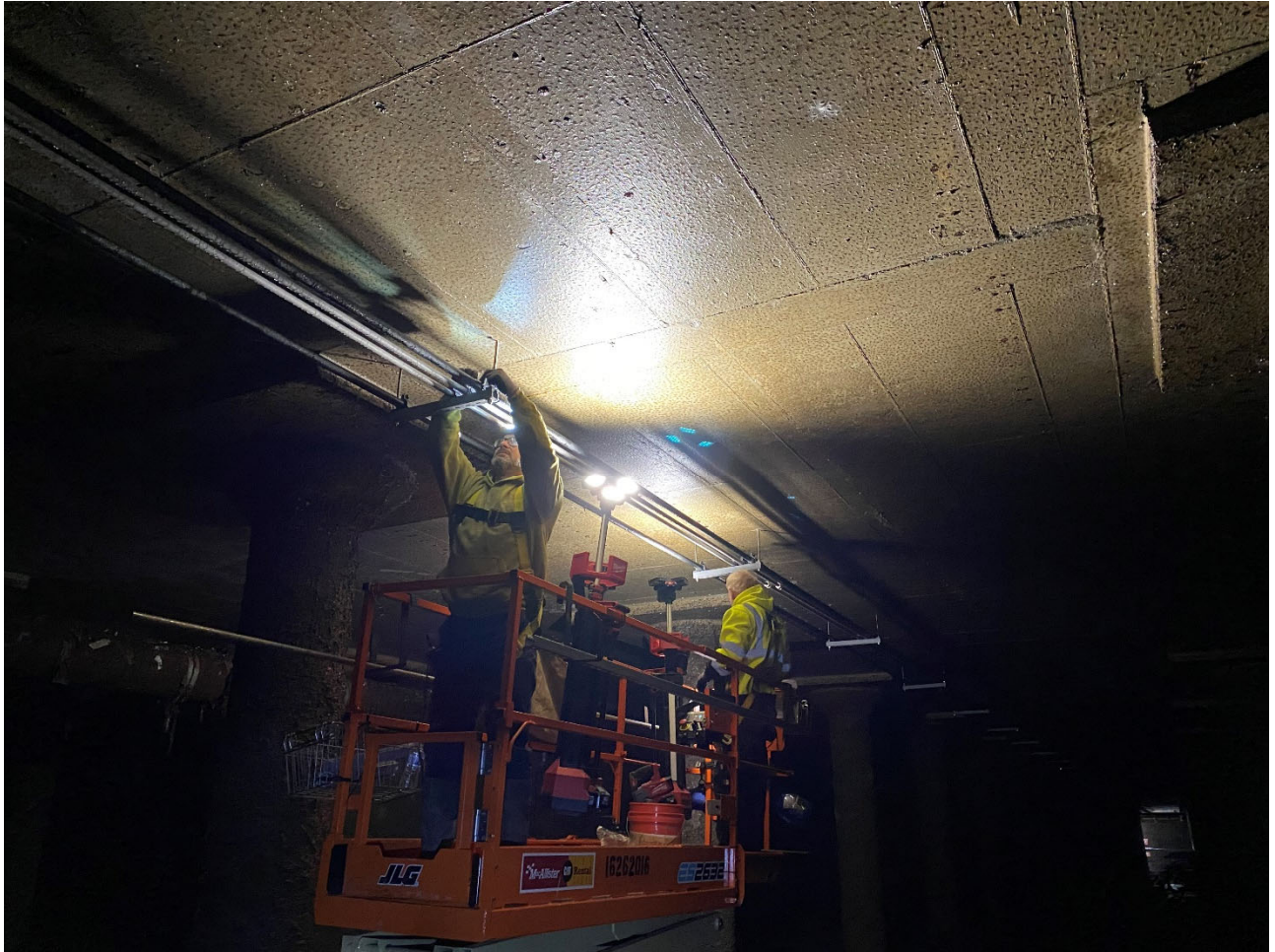
Figure 2 - LDS Installing Hydraulic Lines
