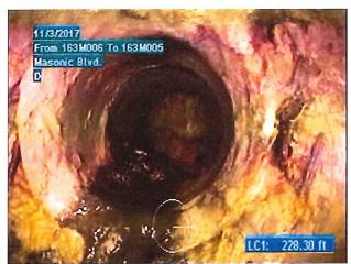
i. Pipe Segment 163M006-163M023:SRV at break-in tap located approximately 234 feet upstream of Manhole 163M023.
