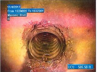
g. Outfall 1637001: Heavy rock and debris removal at Outfall Structure 163Z001.
