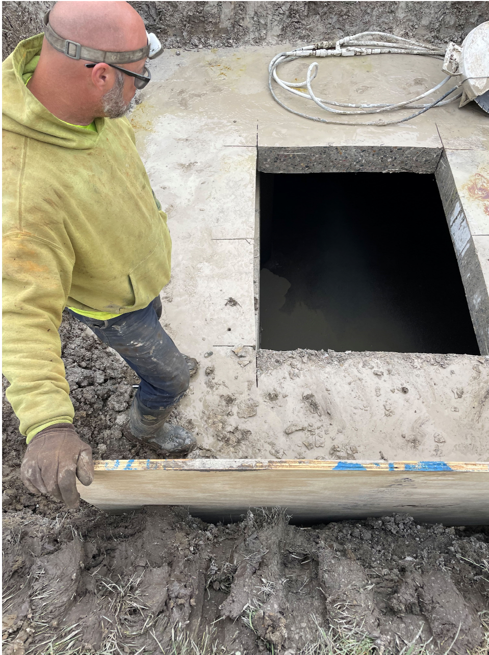
Figure 3 – New access in RTB roof for gate installation
