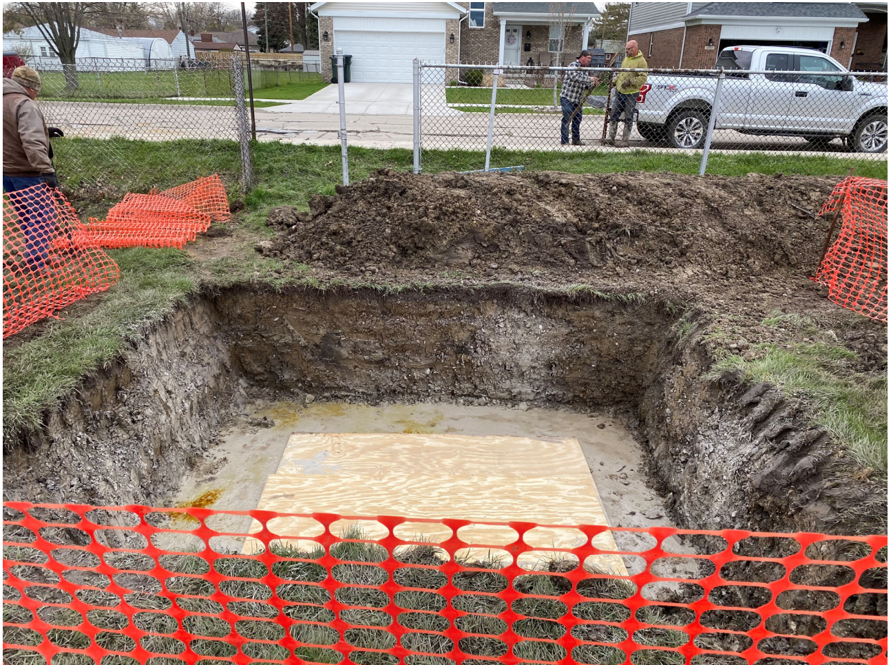
Figure 4 – Excavation to RTB roof and plywood over cutout holes
