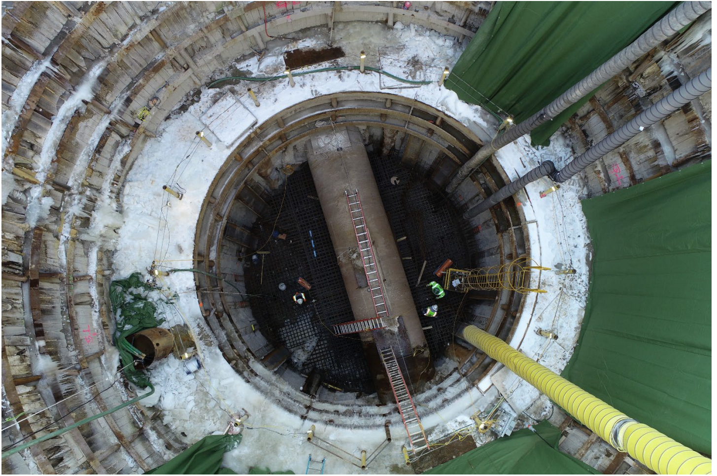
Figure 6 - Aerial View of Rebar Installation
