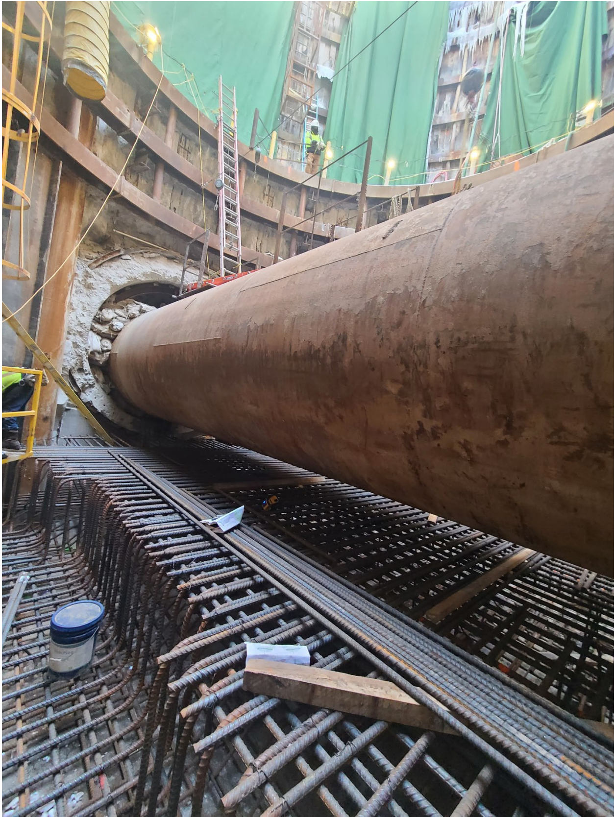
Figure 5 - Installation of Rebar for the Base Slab of the Finished Structure
