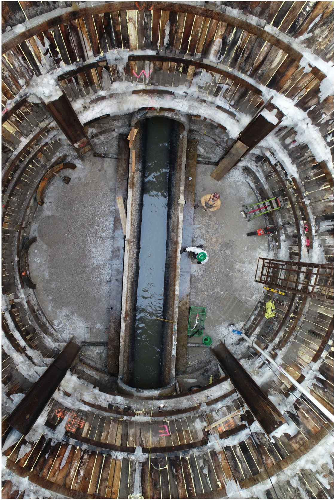
Figure 7 – CS-13 Shaft after the Interceptor Top is Removed
