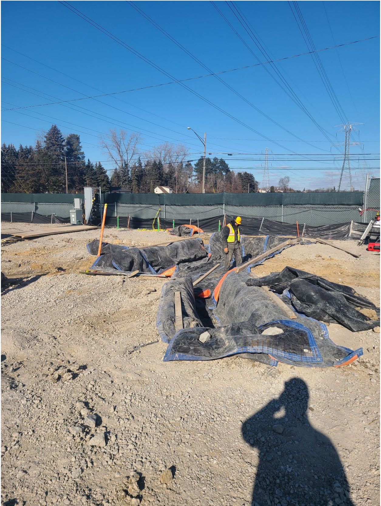
Figure 1 – Excavation for Electrical Pad & Conduit Runs
