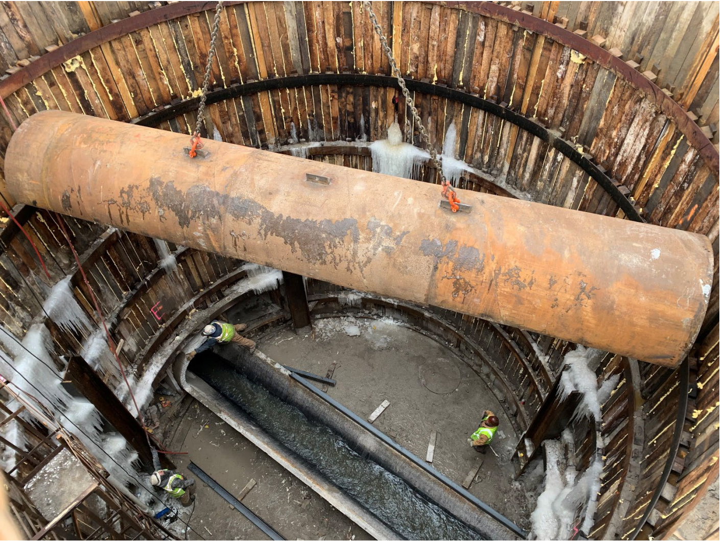
Figure 11 - Temporary Cover for Interceptor
