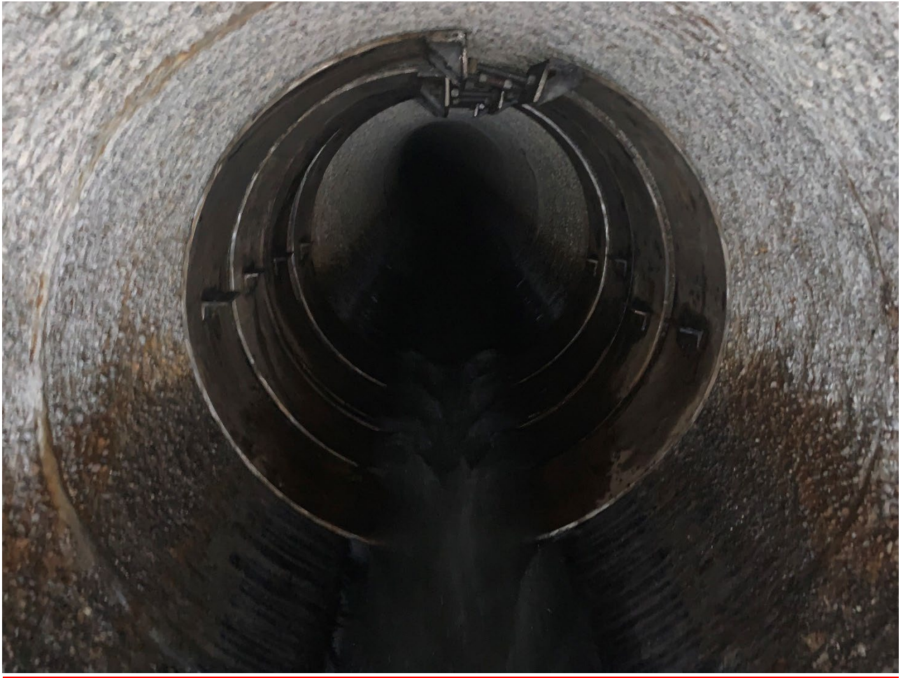
Figure 8 – Steel Internal Bracing prior to Saw Cutting the Interceptor
