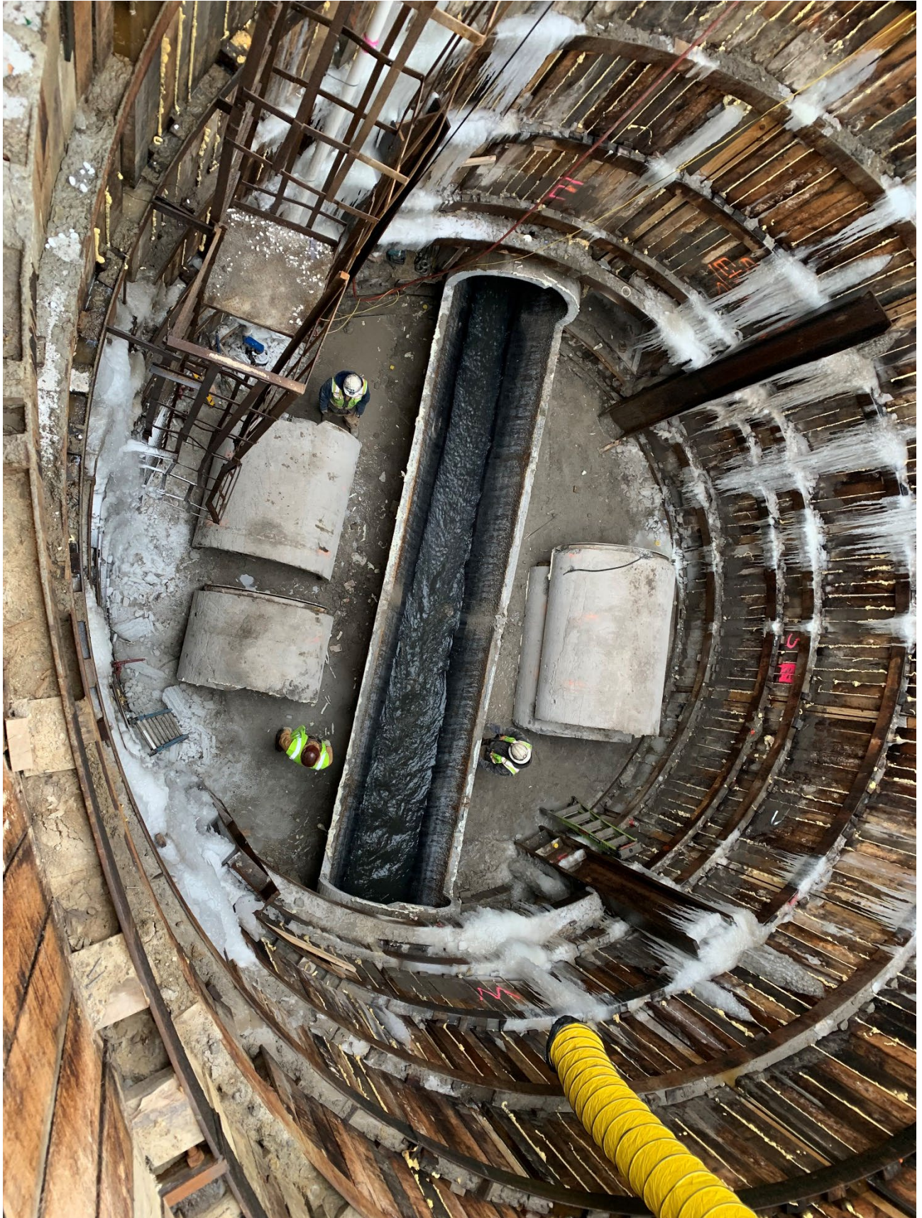
Figure 10 - Interceptor Demolition
