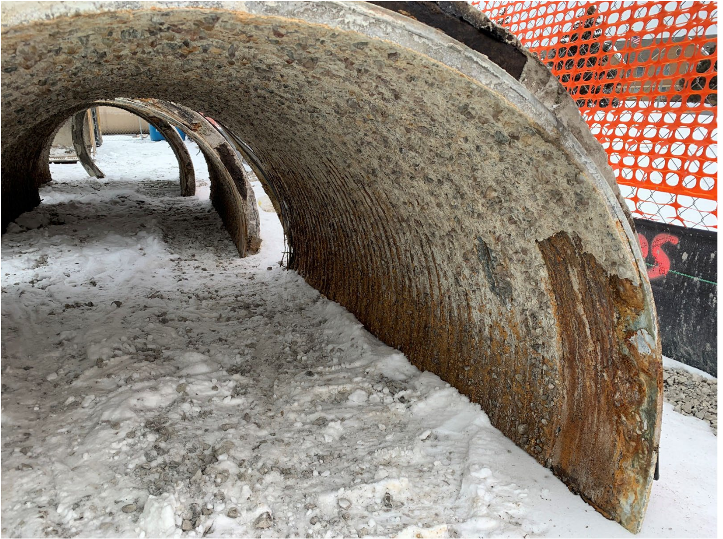
Figure 9 - Removed Section of Interceptor
