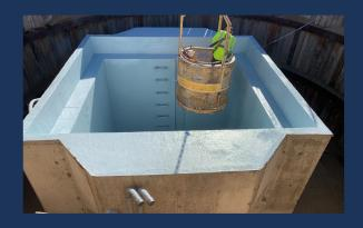
Rehabilitation and spray-lining of the control structure facilities. These concrete structures have been damaged by corrosive hydrogen sulfide gas over time and need repair.
