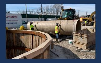
Cleaning and slip-lining 110 segments of large, impervious HOBAS pipe along 15 Mile Road, east of Garfield.
