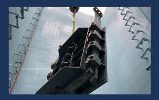
Installation of a new gate control structure on the 15 Mile Interceptor. This will allow for the rehabilitation of a manhole structure and provide future options to store sanitary sewage flow within that interceptor.
