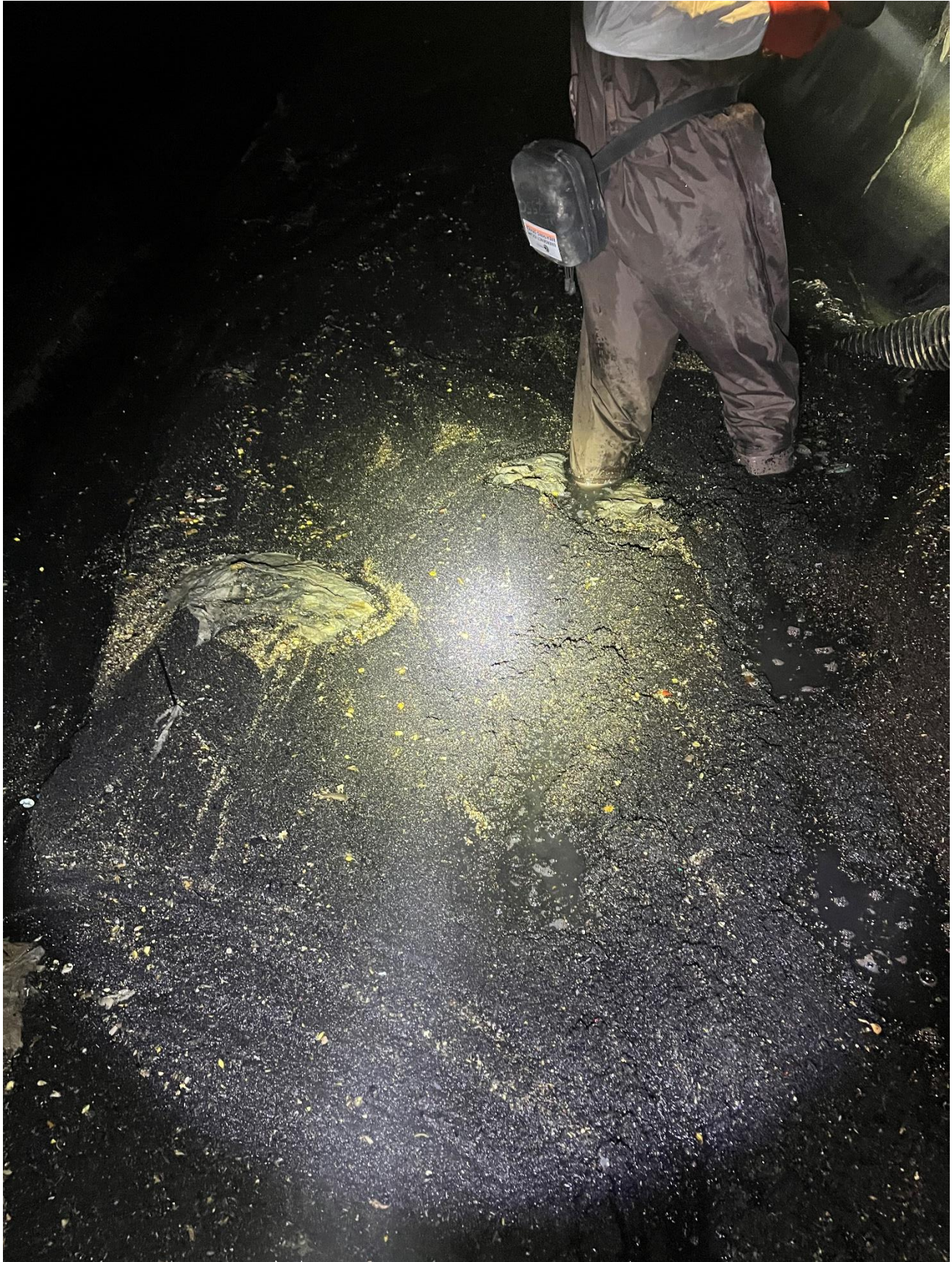
Figure 11 – Viscous Sludge between CS-2 and 15-Mile Interceptor Tap
