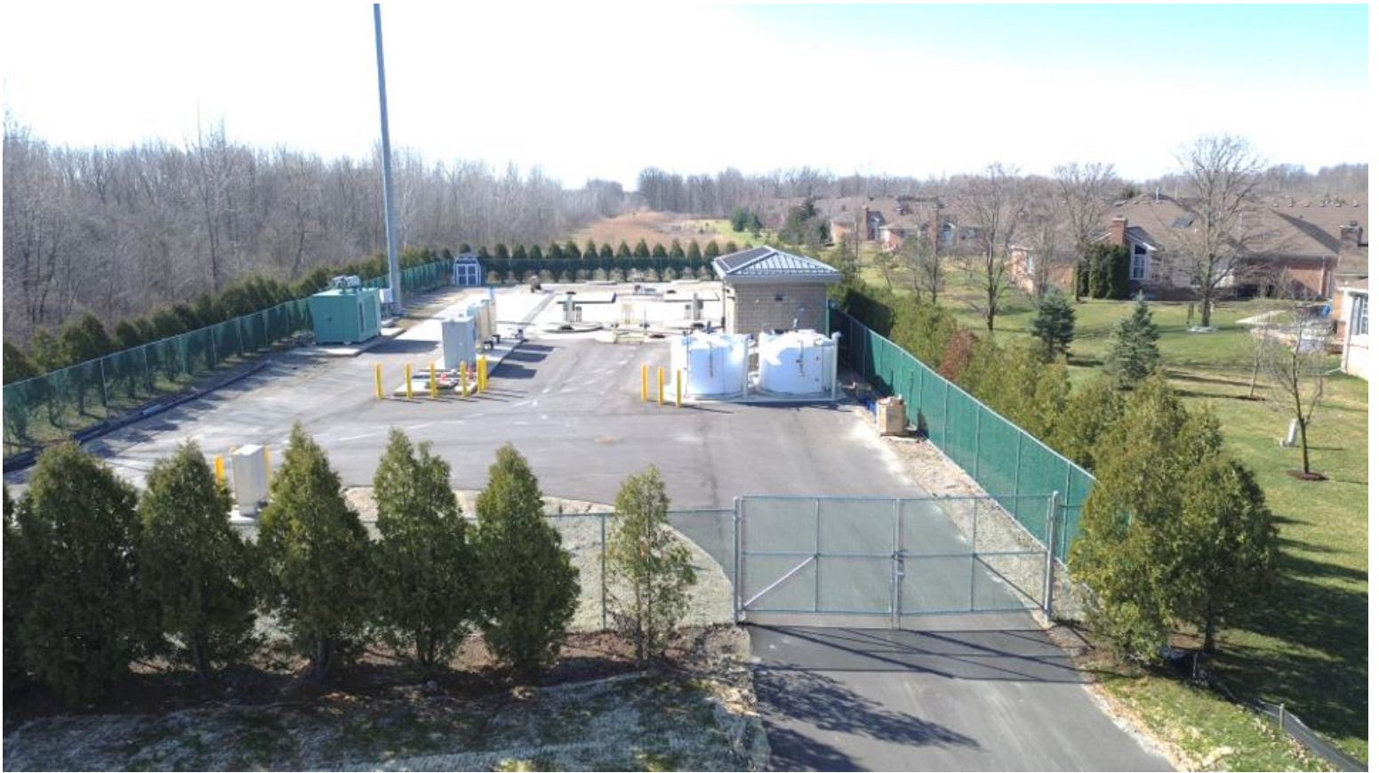
Figure 14 – Aerial View of the NGI Chemical Injection Facility
