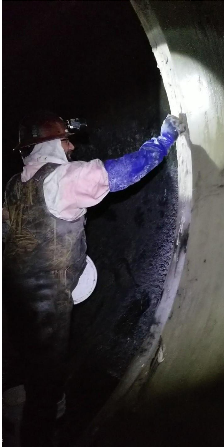
Figure 4 – Applying Joint Soap to the HOBAS
