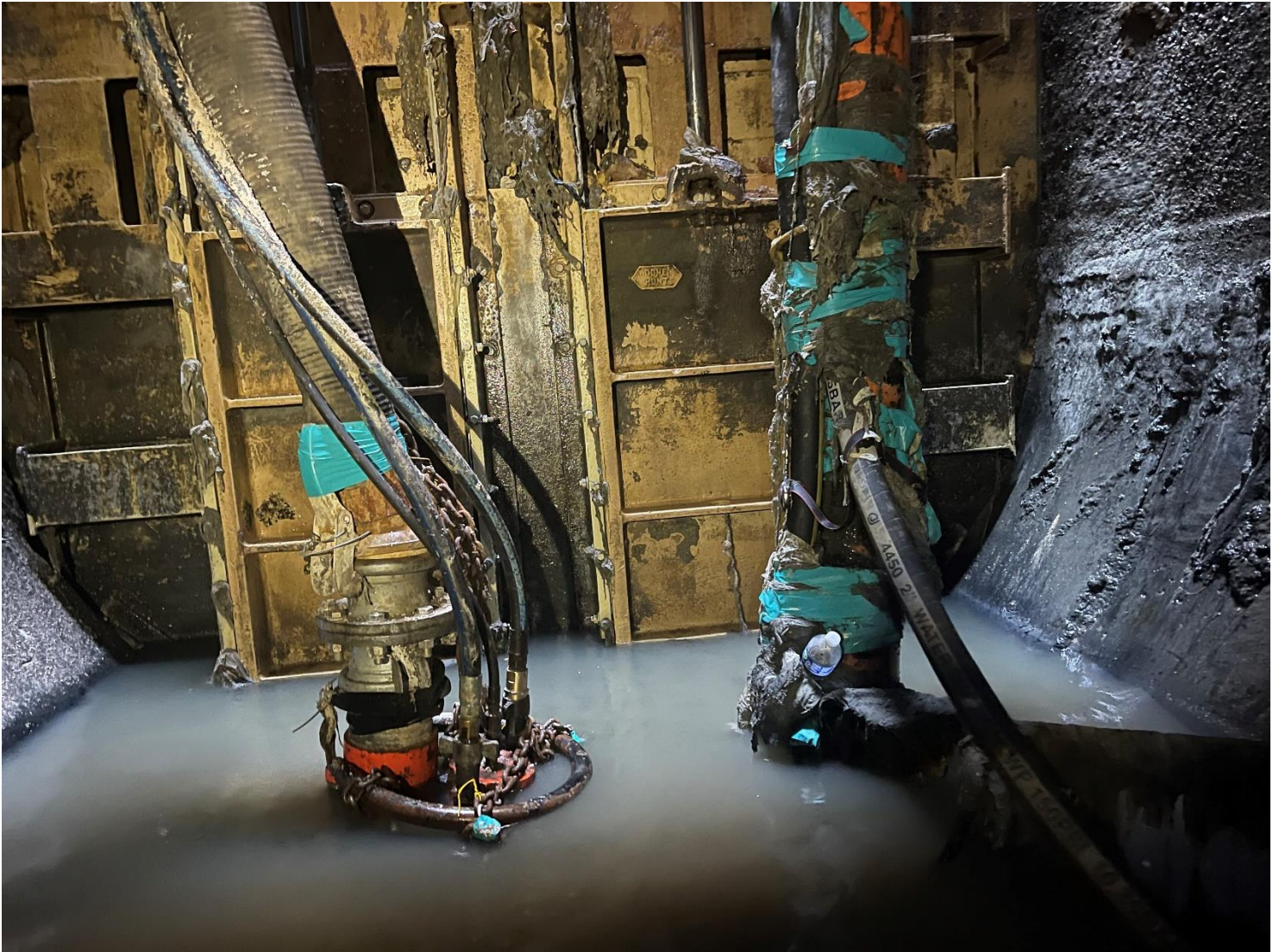
Figure 9 – Dewatering Pump and Vac Line at CS-3
