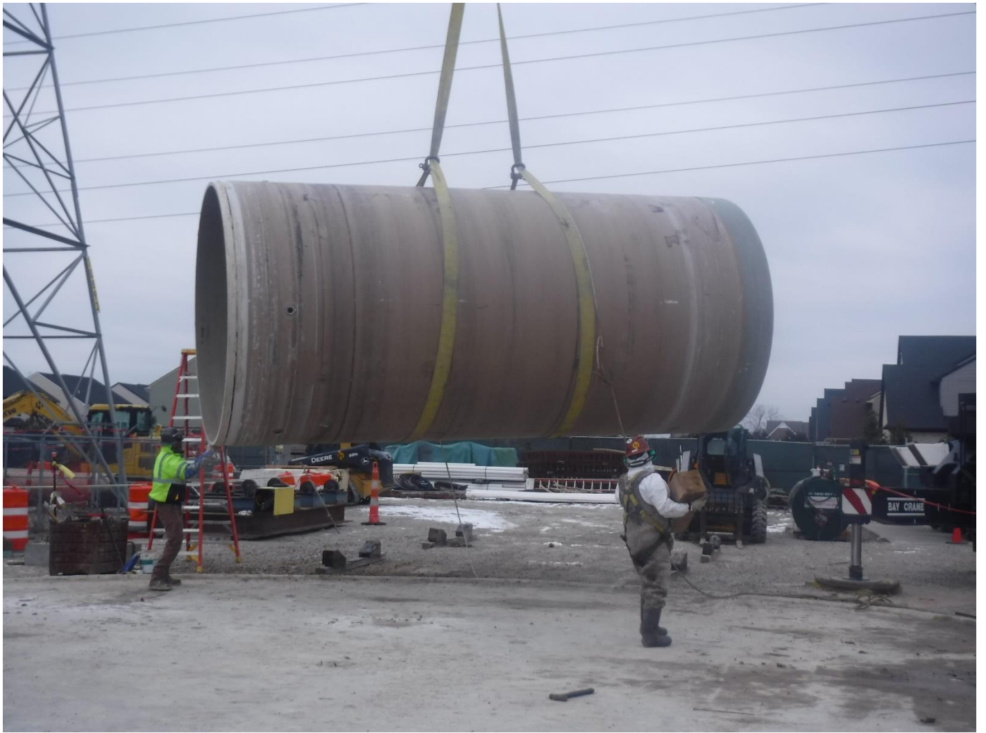
Figure 2 – Hoisting HOBAS Pipe into CS-12 (daily operation for while slip-lining)
