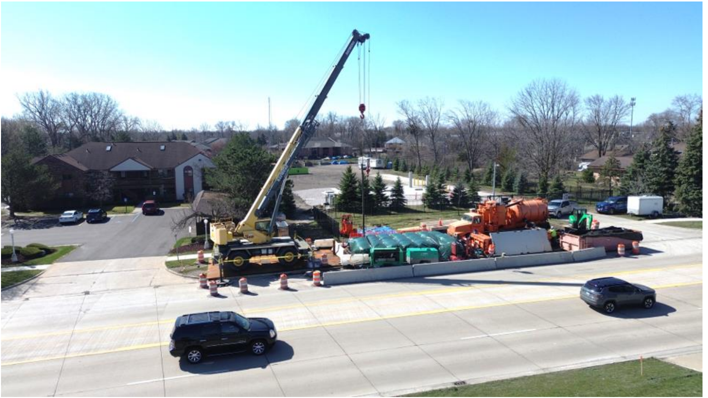
Figure 8 – Debris Removed Setup at CS-3 – Facing South
