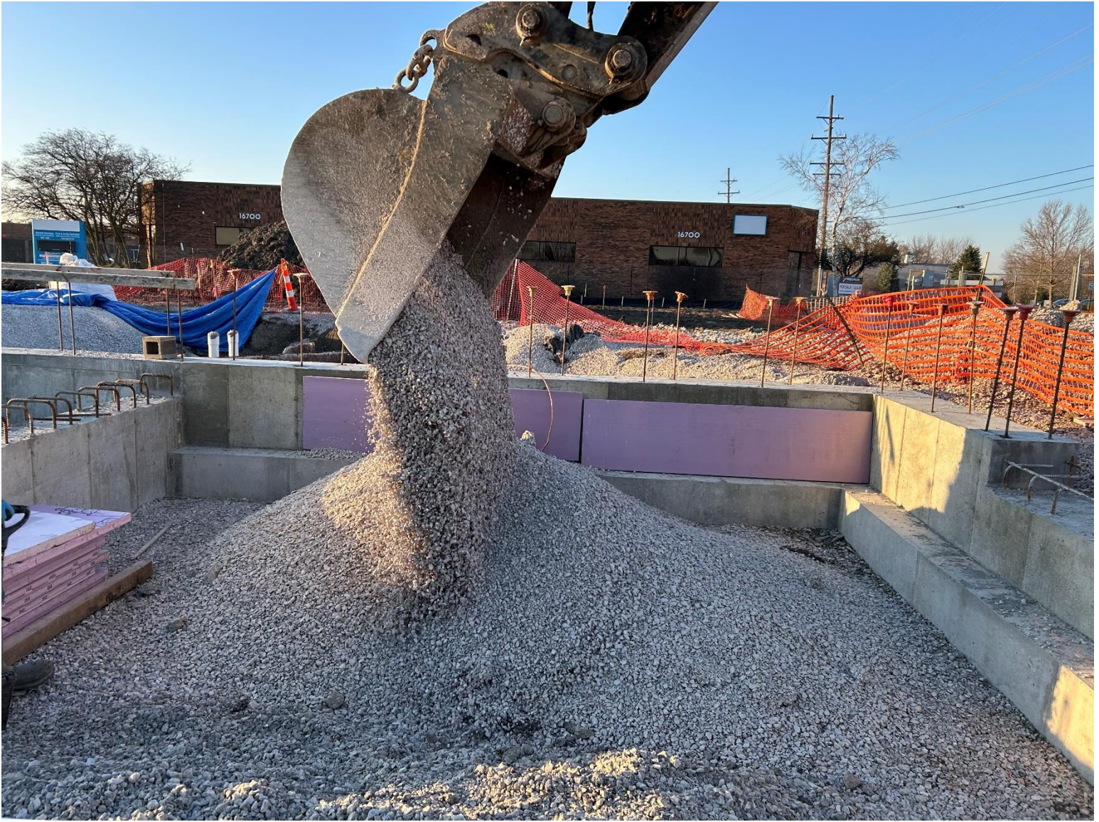
Figure 20 – Macomb Township Bio-Filter Back-Filling at Utility Building
