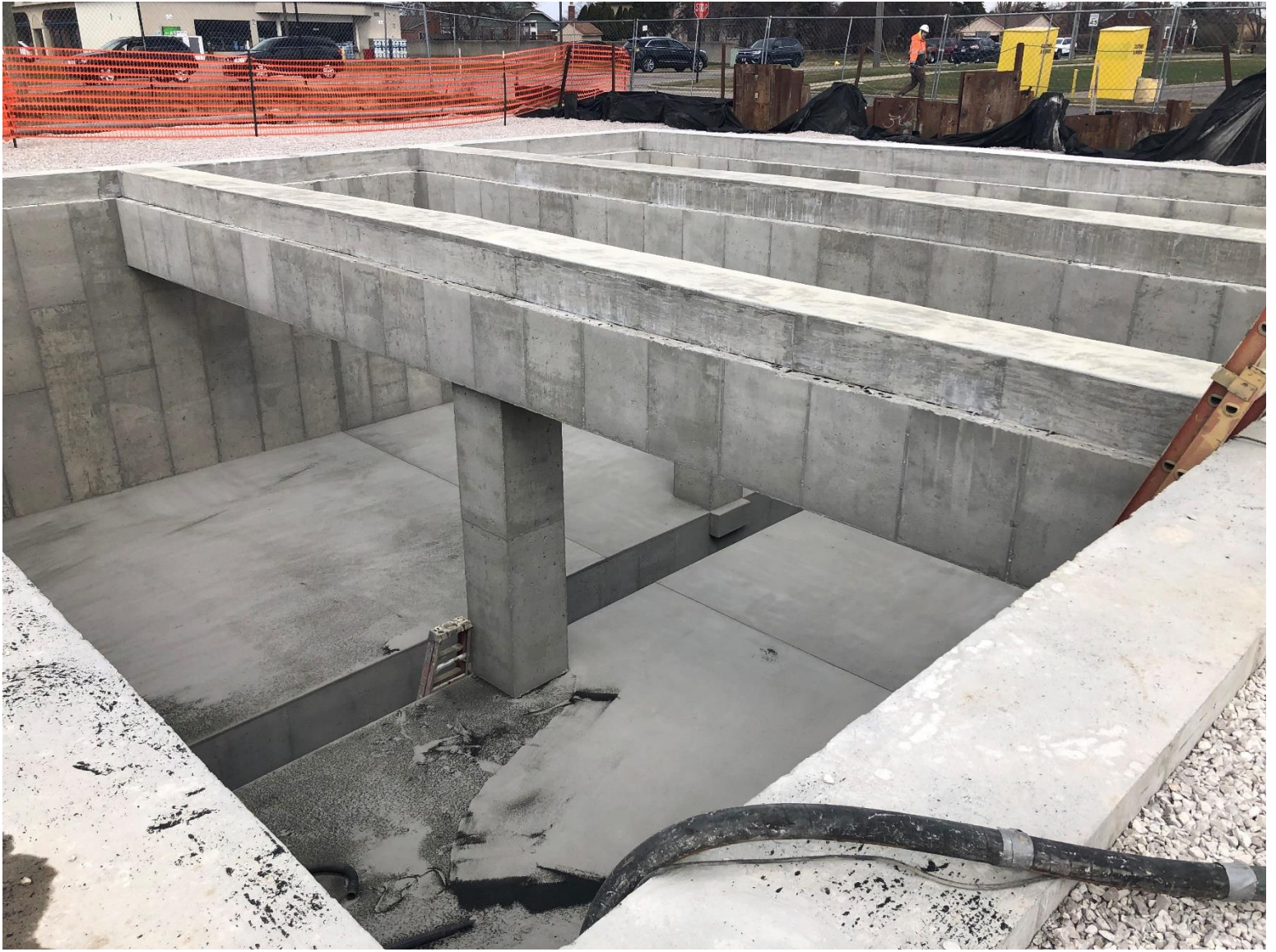
Figure 15 – Macomb Township Bio-Filter Media Chamber Sandblasting
