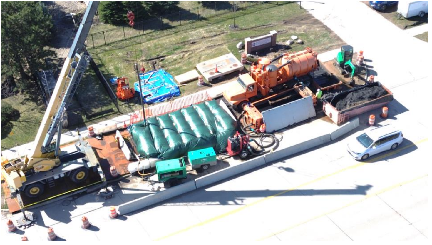
Figure 7 – Aerial View at CS-3 of Debris Removal Equipment
