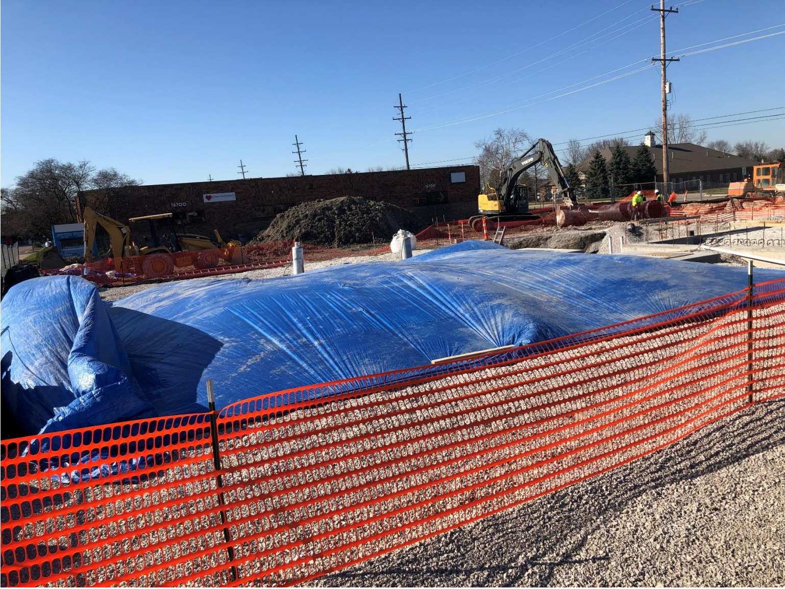
Figure 17 – Macomb Township Bio-Filter Media Temporary Tarp Installation
