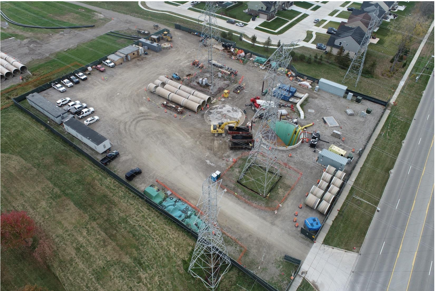
Figure 1 – CS-12 Pump Station, Construction Yard
