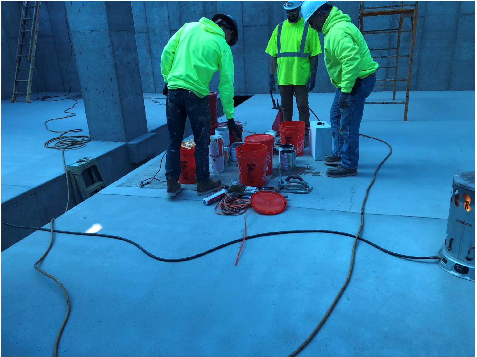
Figure 18 – Macomb Township Bio-Filter Media Chamber Crack Repair & Surface Preparation
