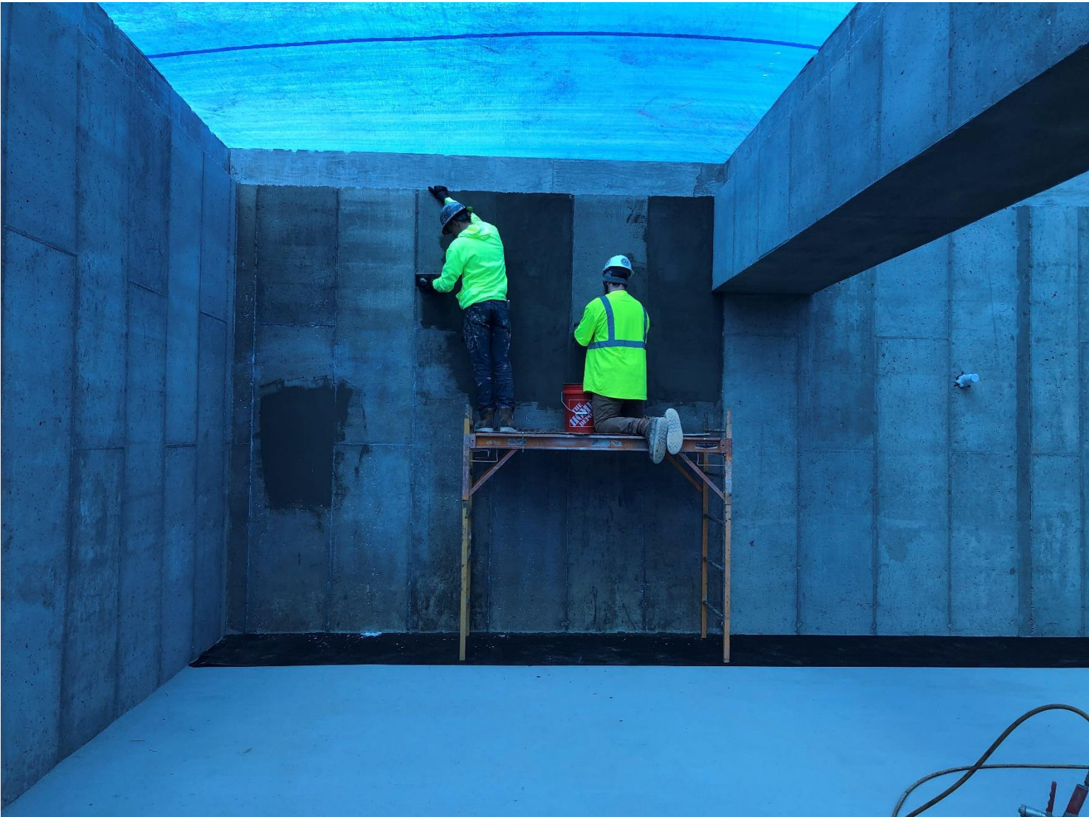
Figure 19 - Macomb Township Bio-Filter Media Chamber Crack Repair & Surface Preparation
