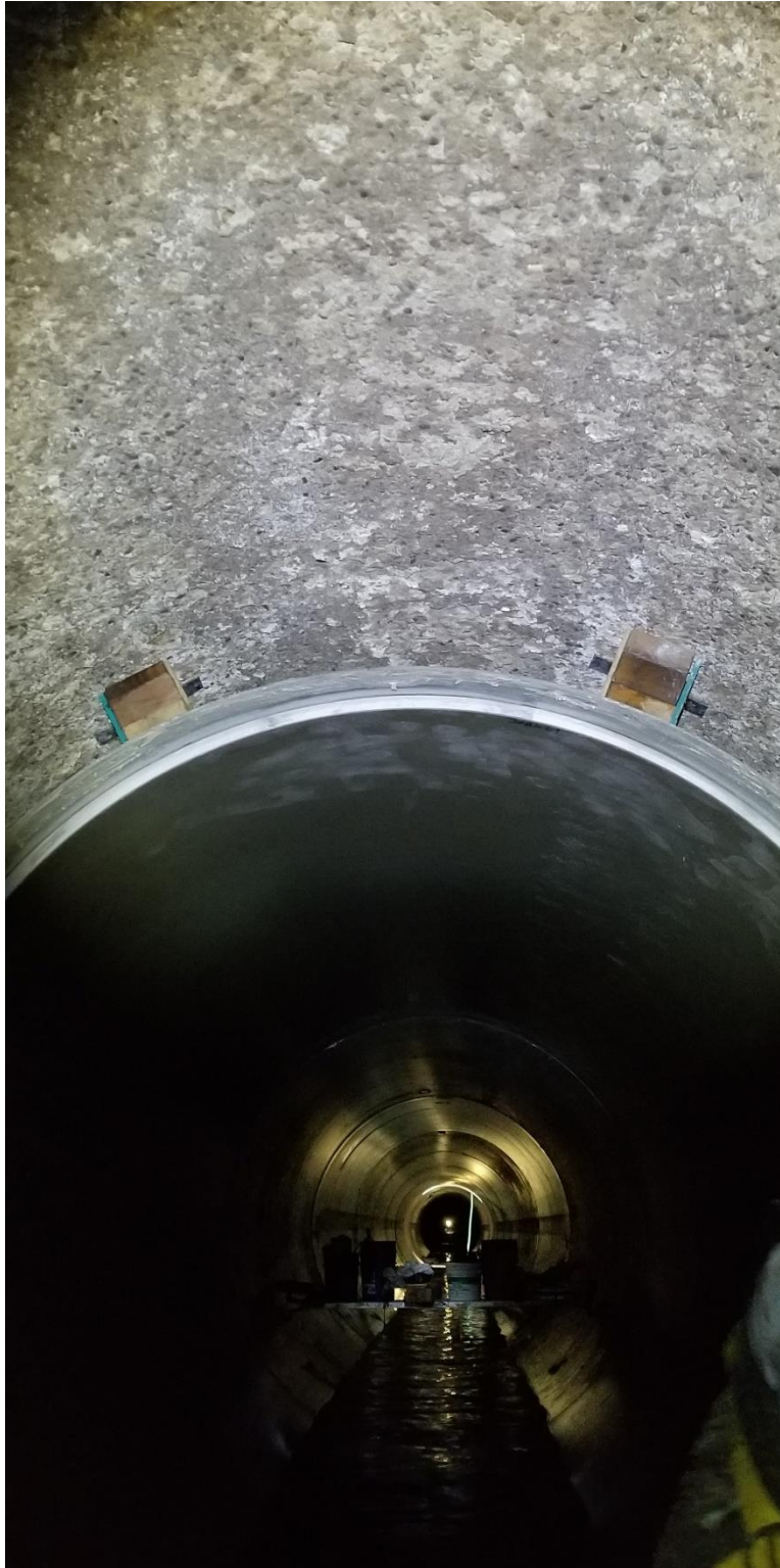
Figure 6 – Wood Blocking on the Crown of the Pipe
