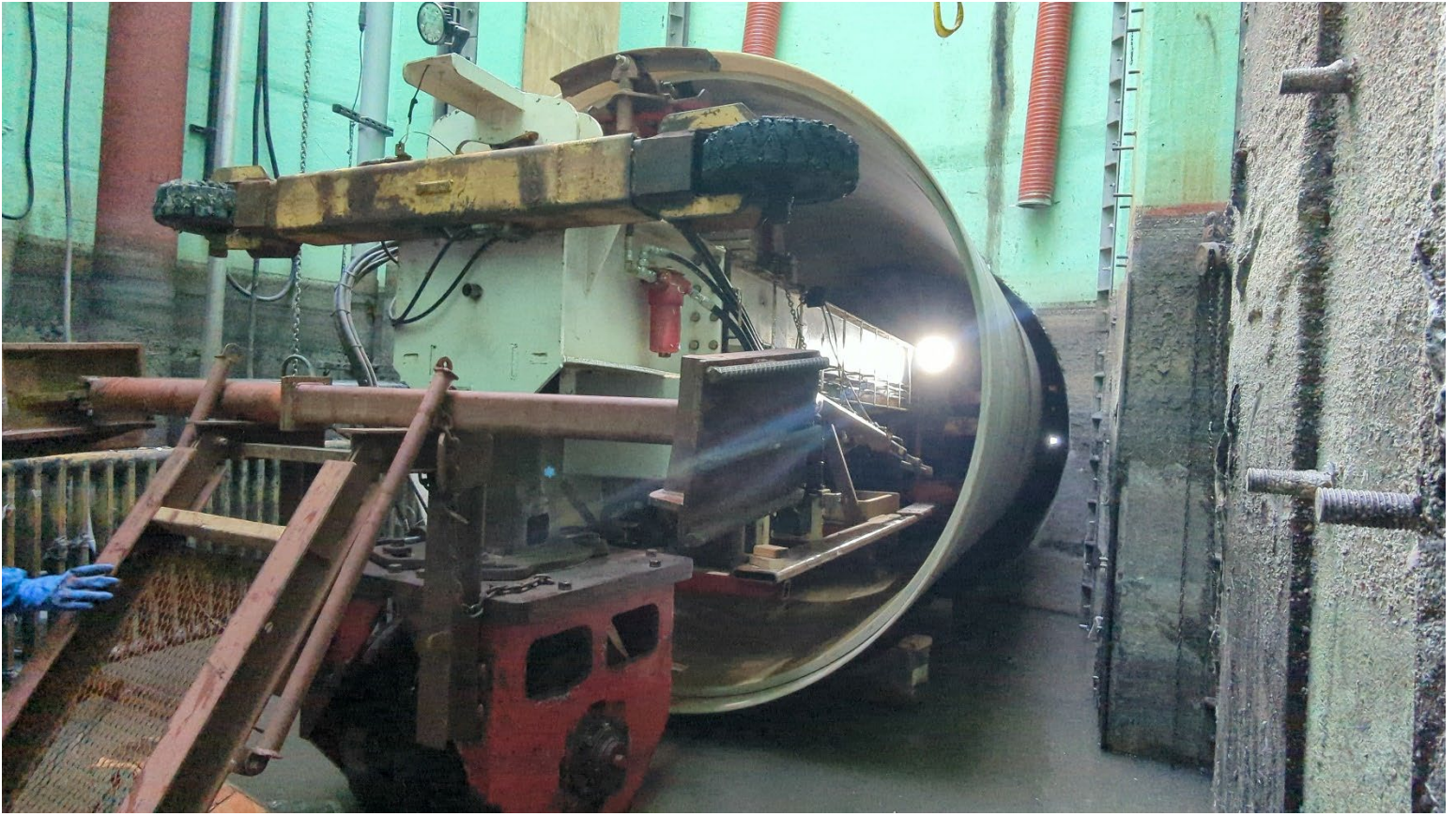
Figure 3 – Pipe Carrier Testing with HOBAS
