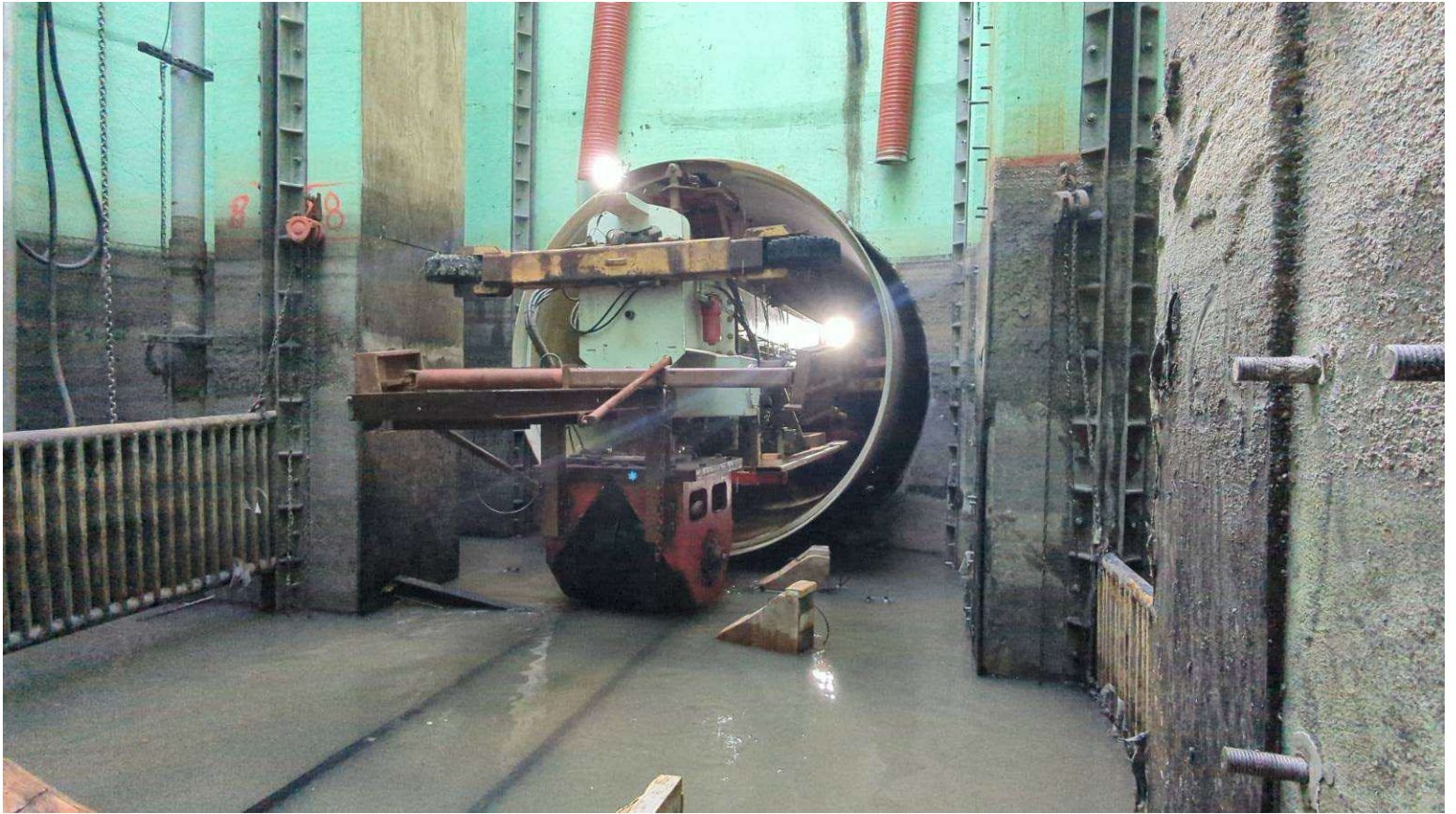
Figure 4 – Pipe Carrier Testing with HOBAS
