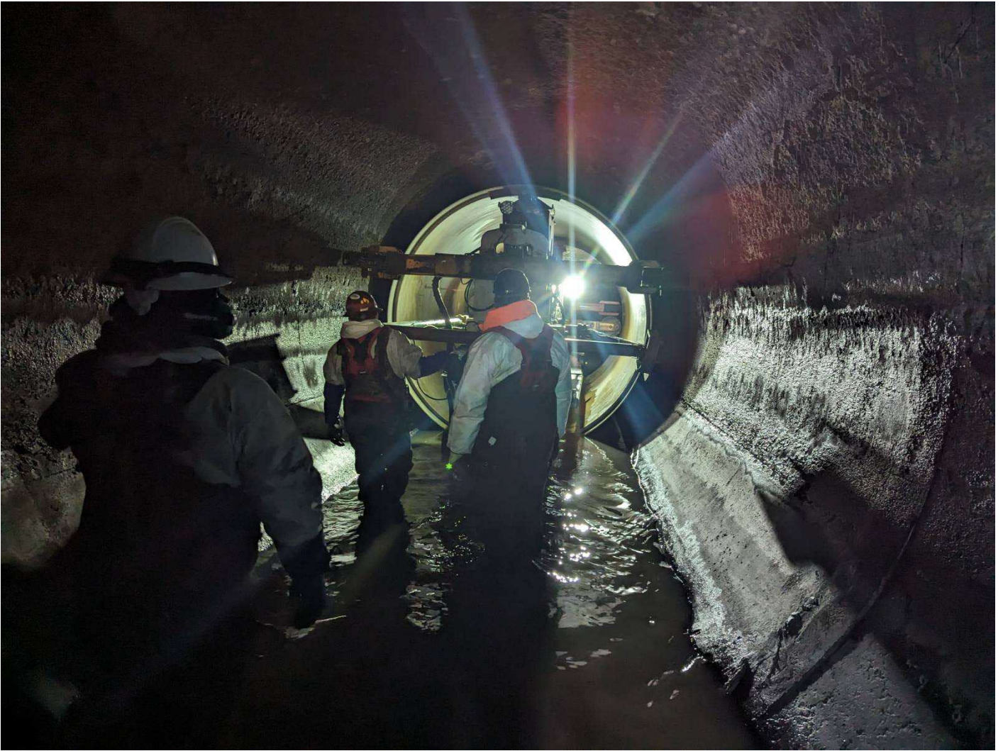
Figure 5 – Pipe Carrier Testing with HOBAS Pipe
