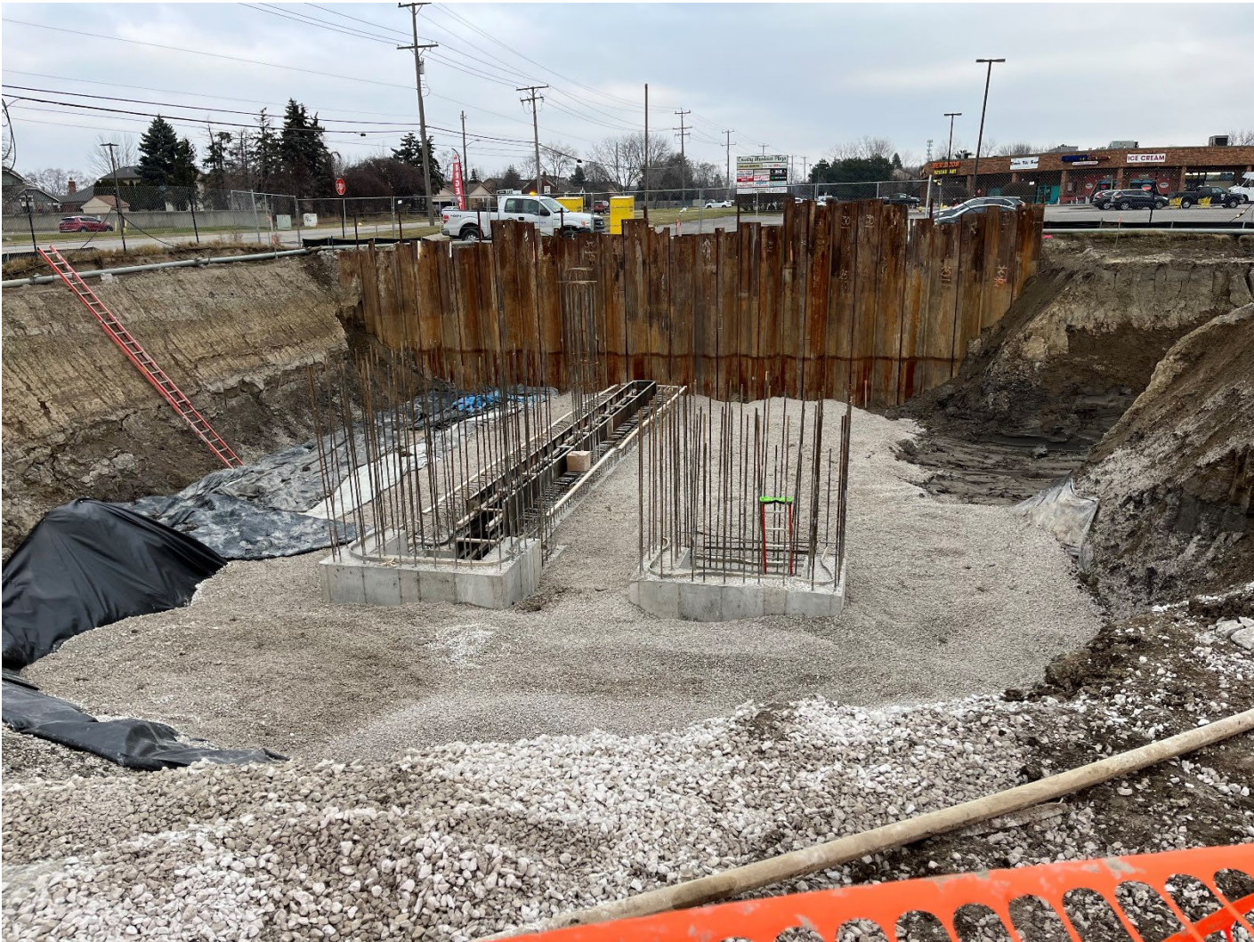
Figure 14 – Macomb Twp. Foundation Construction
