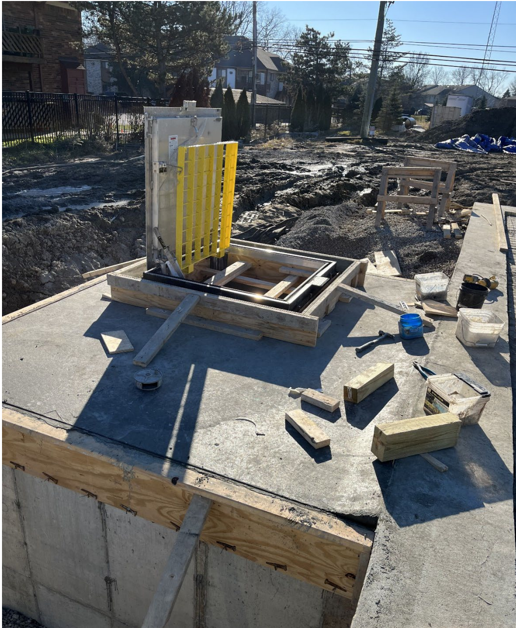
Figure 12 – Fraser Bio-Filter Access Hatch Installation
