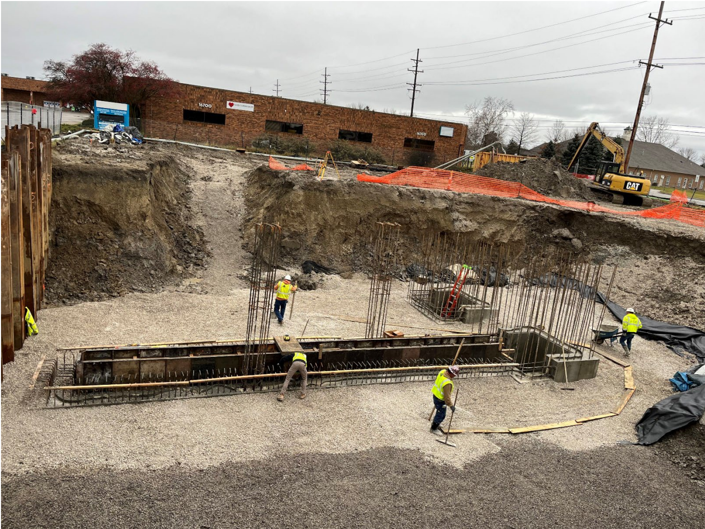
Figure 16 – Macomb Twp. Foundation Construction
