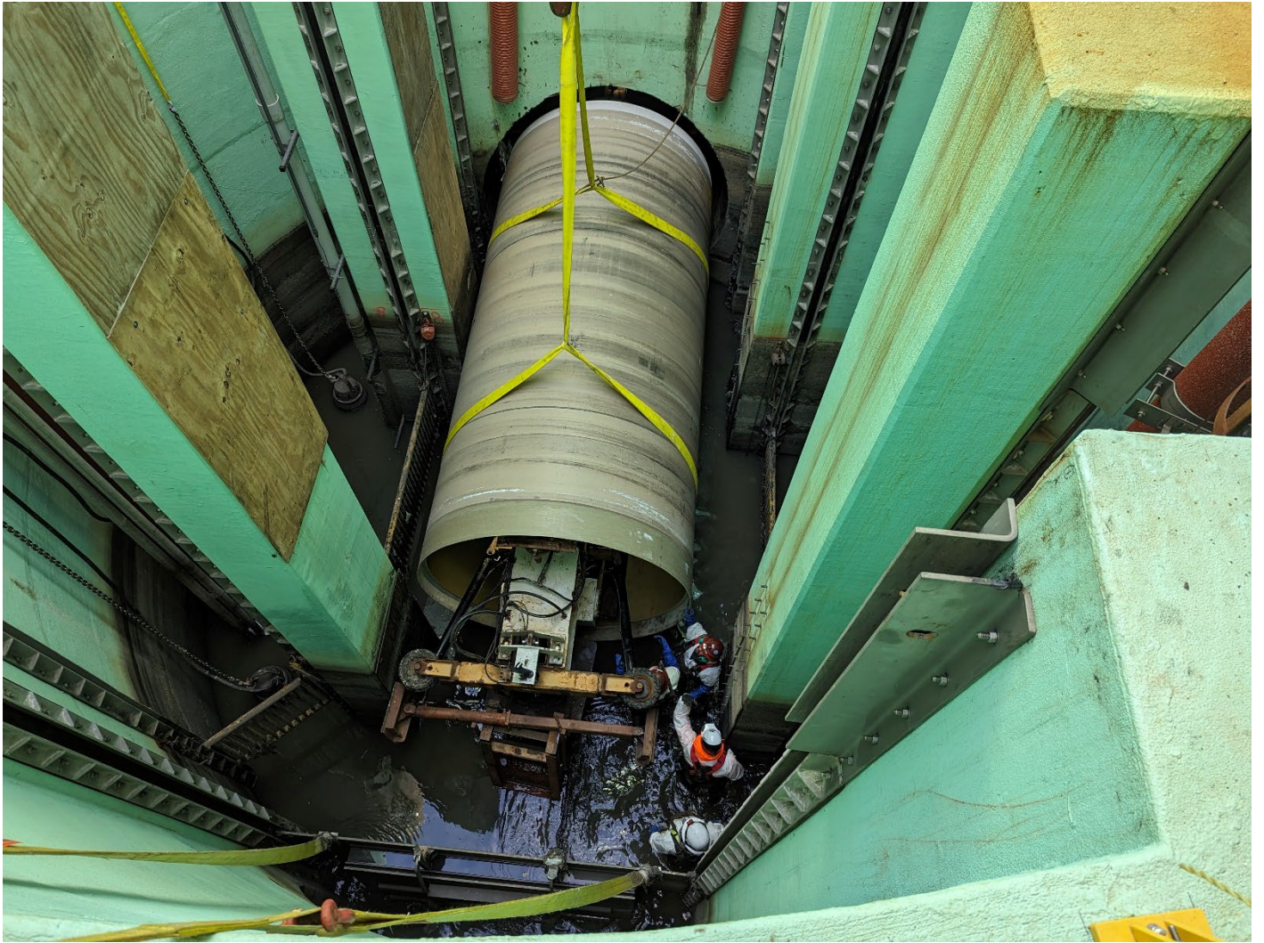
Figure 2 – Pipe Carrier Testing with HOBAS
