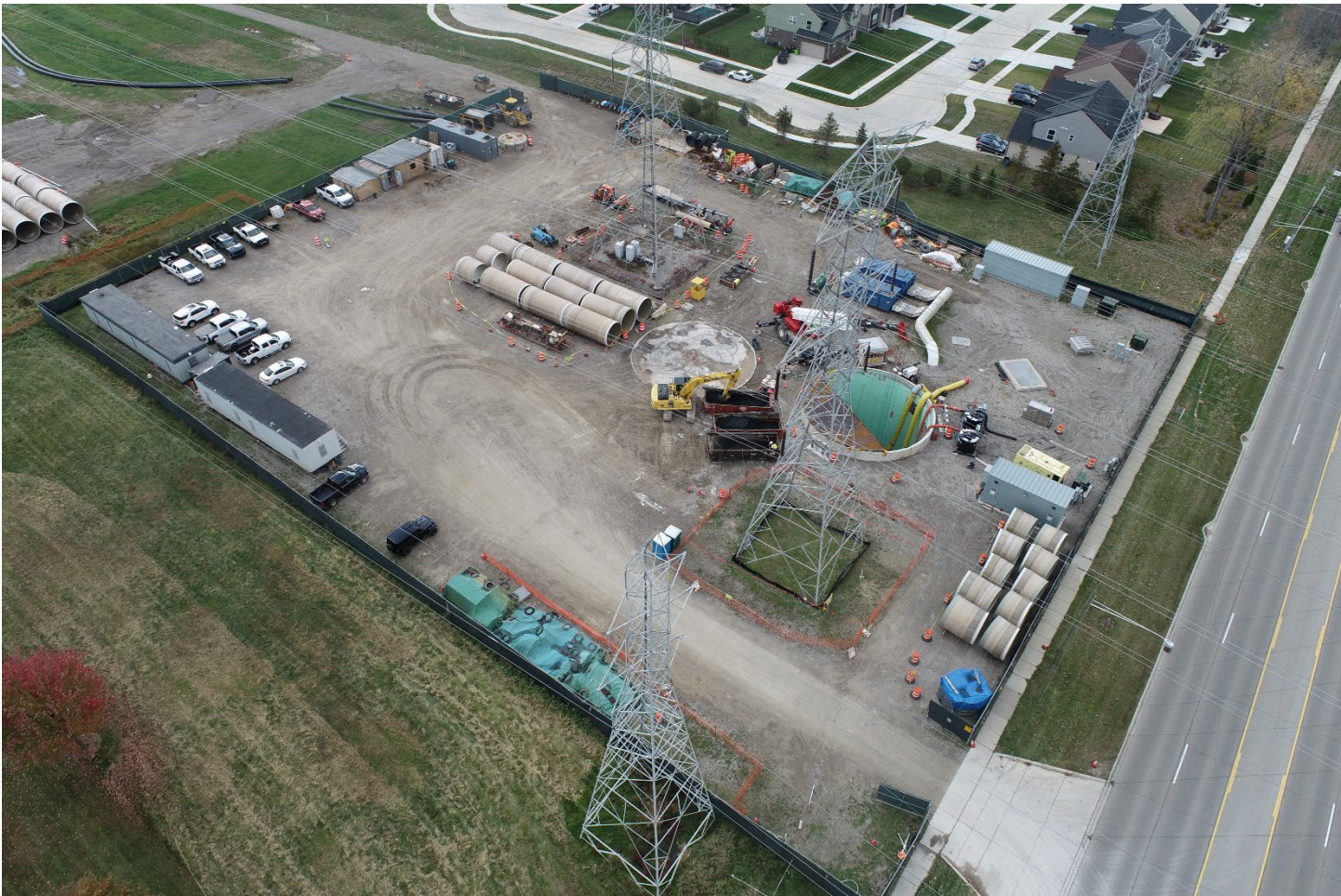
Figure 1 – CS-12 Pump Station, Construction Yard
