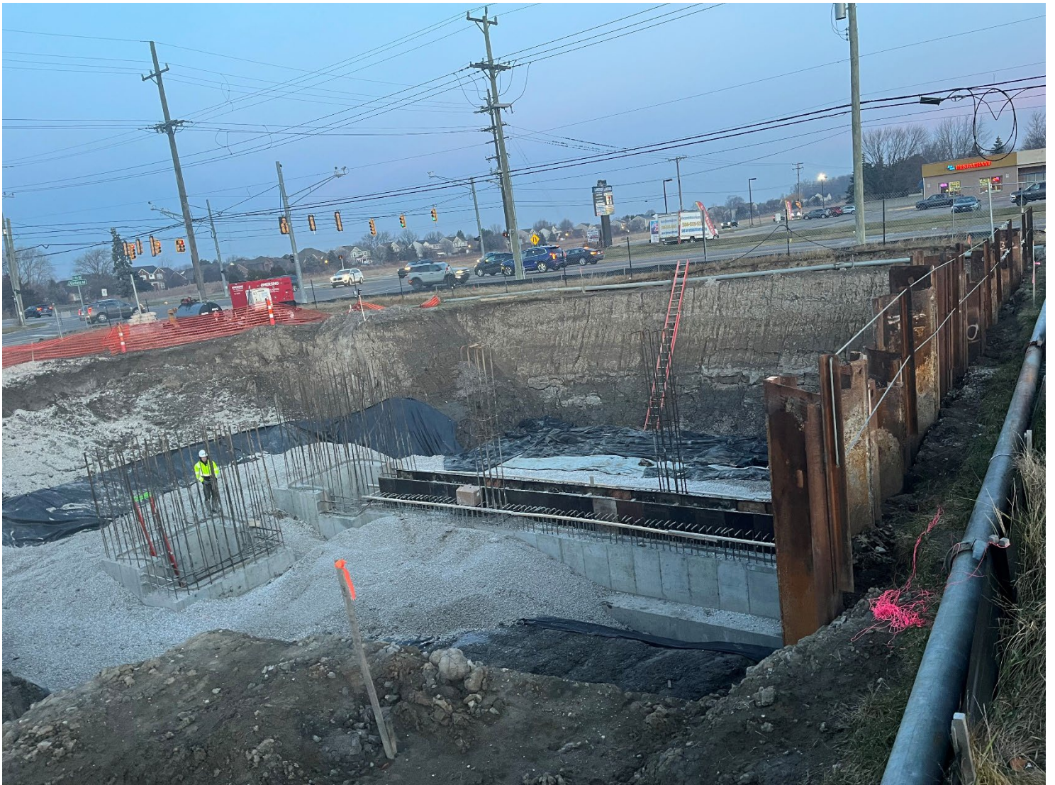
Figure 15 – Macomb Twp. Foundation Construction
