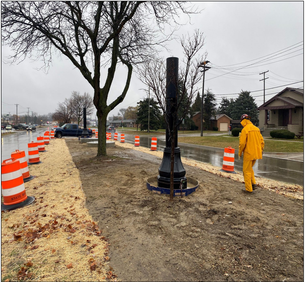
Figure 8 – Installing Lampstand Vents @ Kelly Rd. Blvd.
