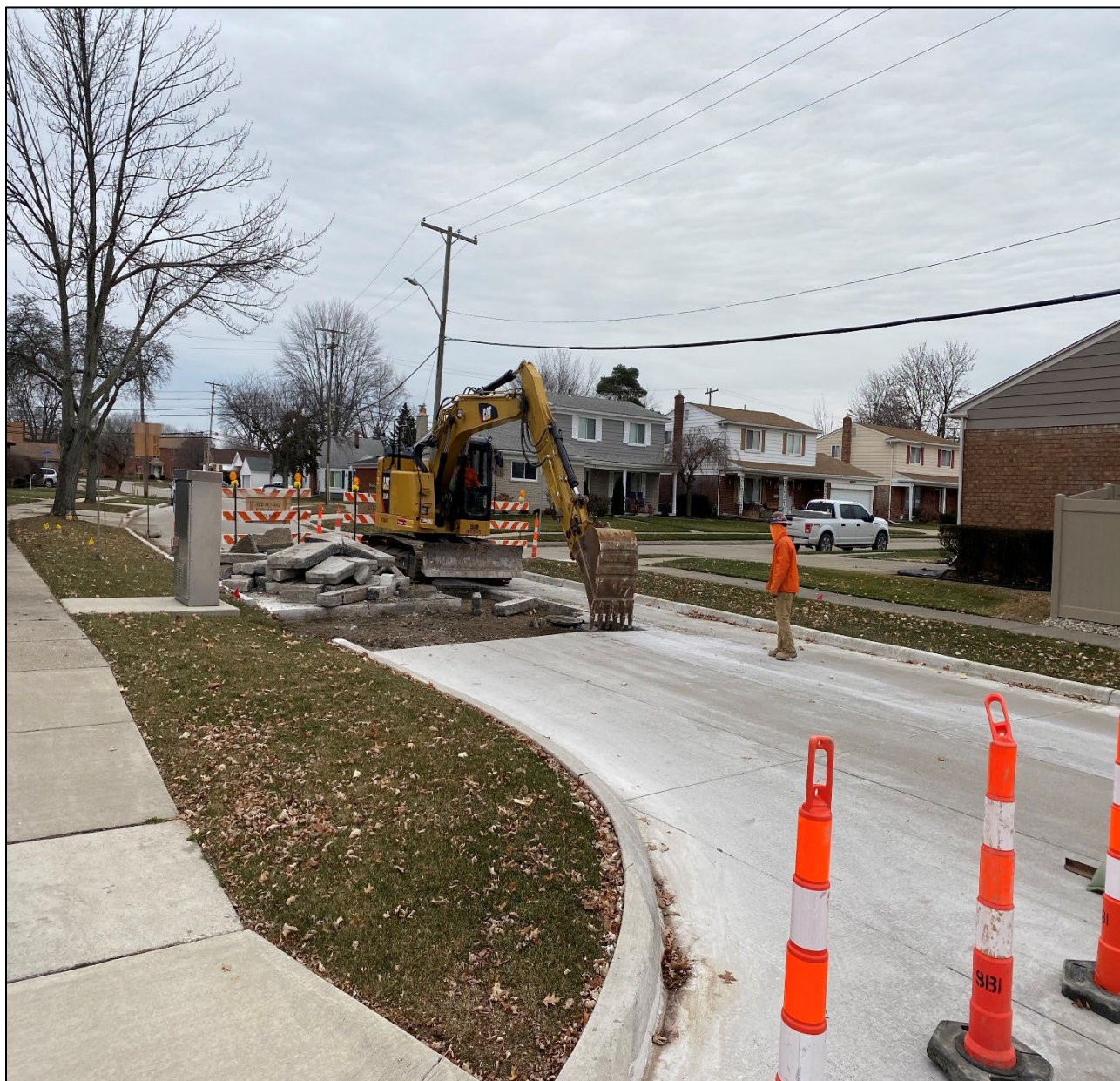
Figure 10 –Removing Concrete @ Malvern Street
