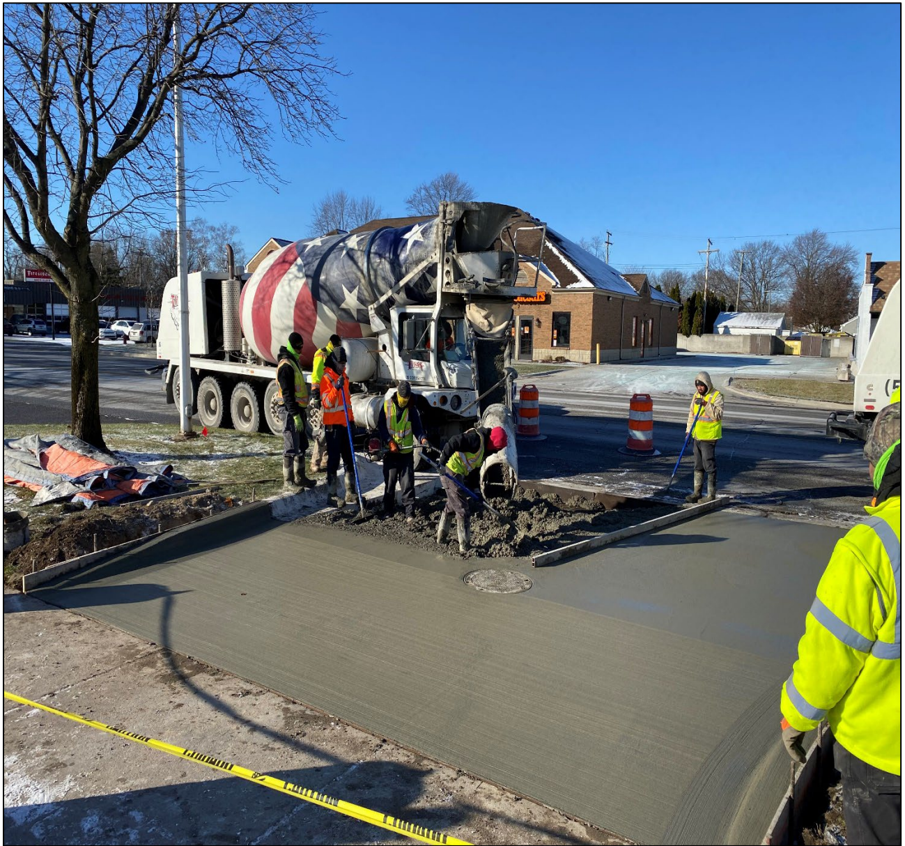
Figure 9 – Placing Concrete @ Greater Mack Road
