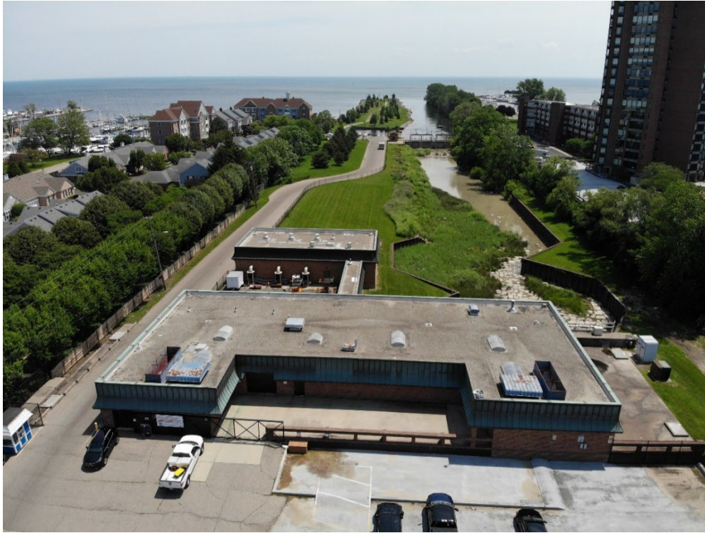
Figure 21 – Drone Aerial at 100 FT Facing East (Baseline)
