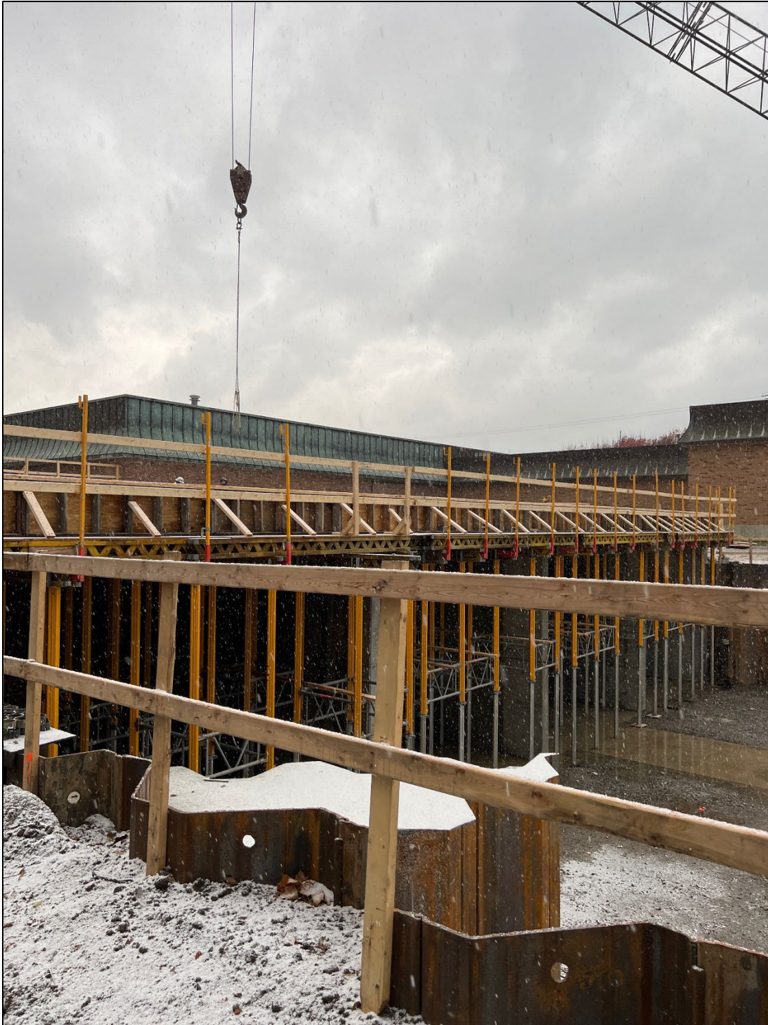
Figure 15 – Screening Structure top slab forms
