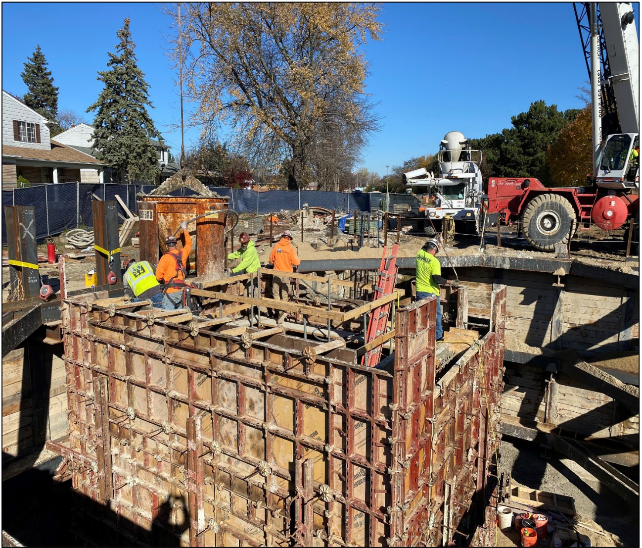
Figure 4 – Placing Wall Concrete for West Access @ Beaconsfield Shaft
