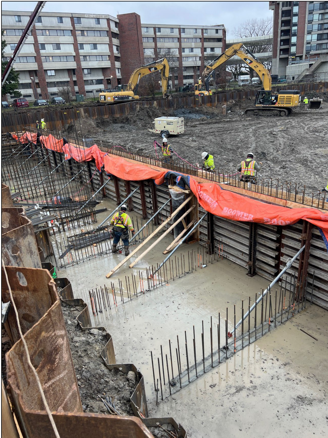
Figure 17 – Outfall Structure wall pour (N-s) + divider wall steel (E-W)
