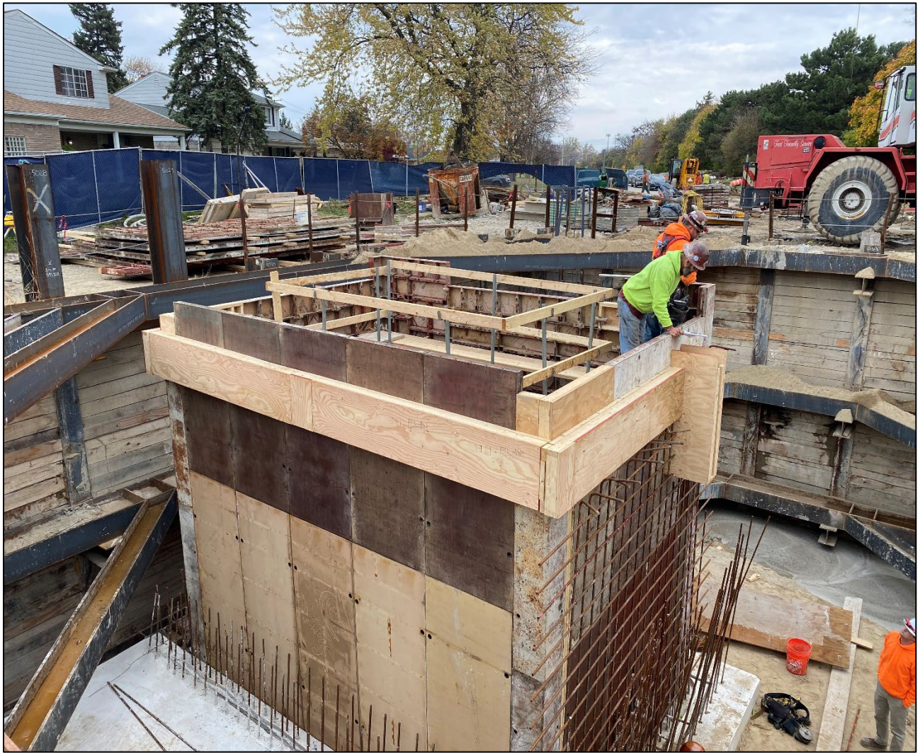
Figure 3 – Installing Concrete Wall Forms @ Beaconsfield Shaft
