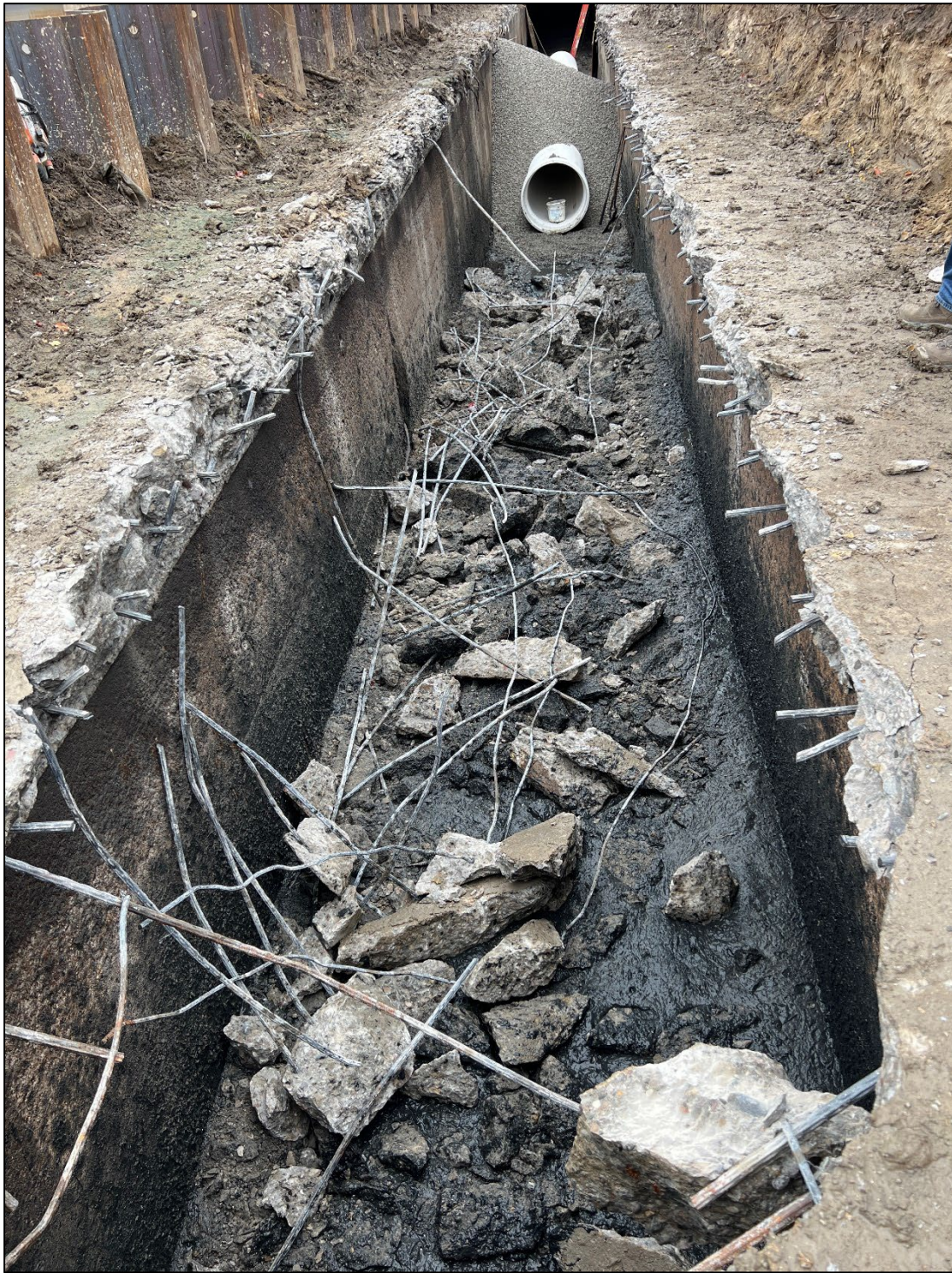
Figure 20 – 36” dia. Storm sewer installed within north box of abandoned 9-Mile Drain.
