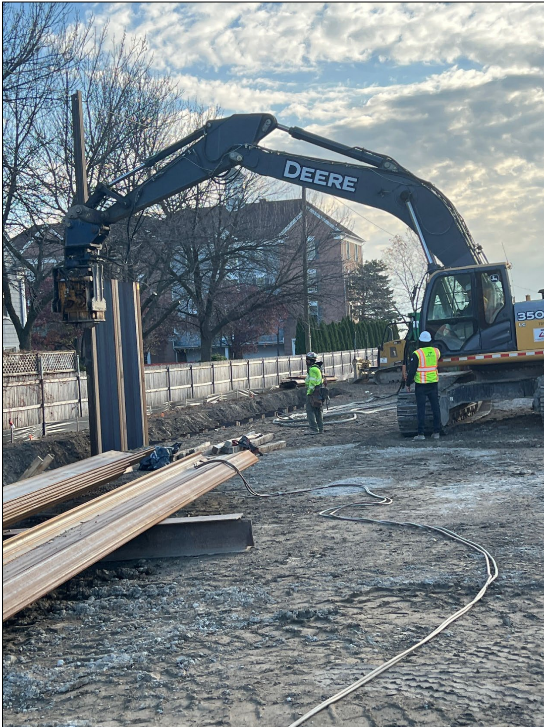
Figure 19 – Row of tieback sheeting along northerly property line
