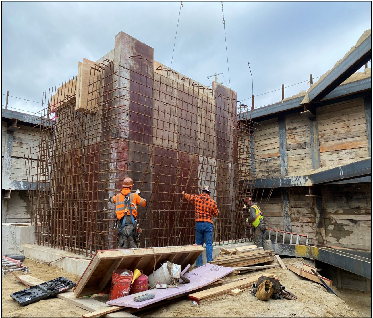
Figure 2 – Placing Reinforcing Steel @ Beaconsfield Shaft
