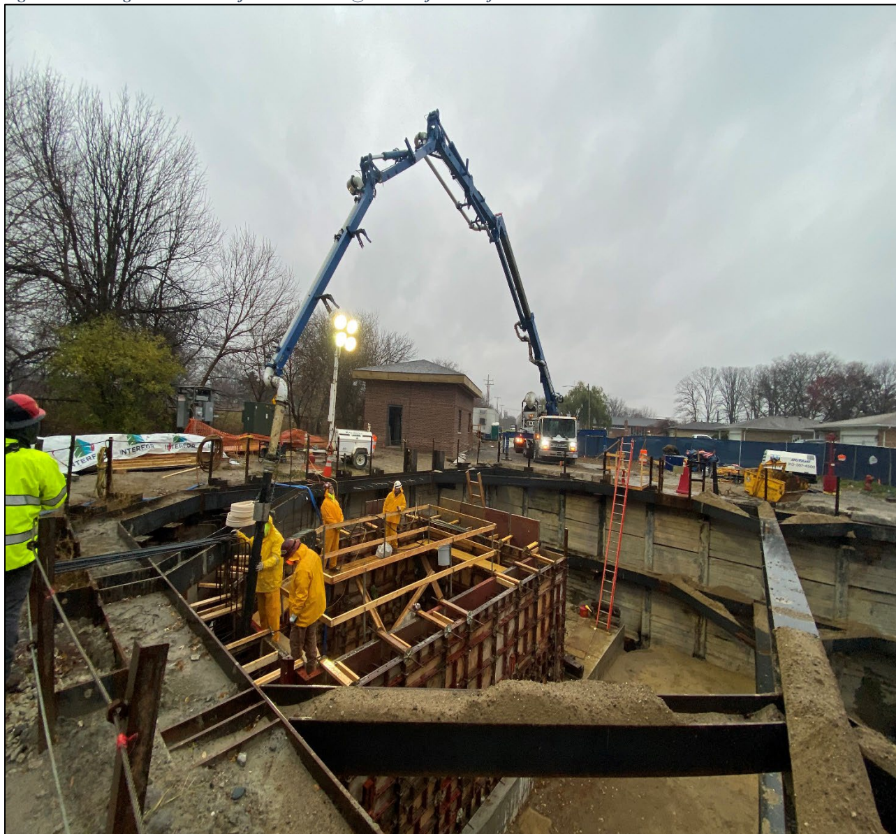
Figure 6 – Placing Wall Concrete for East Access @ Beaconsfield Shaft
