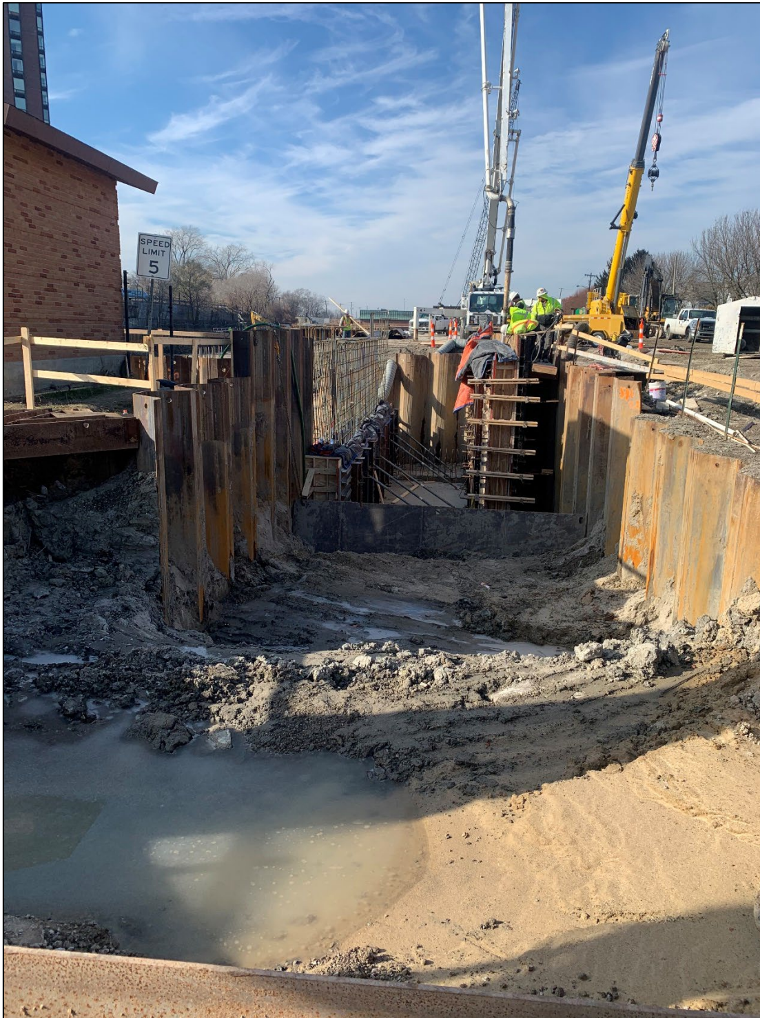
Figure 18 – Cofferdam and deep foundation for future outfall building
