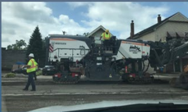
Rehabilitation and resurfacing
