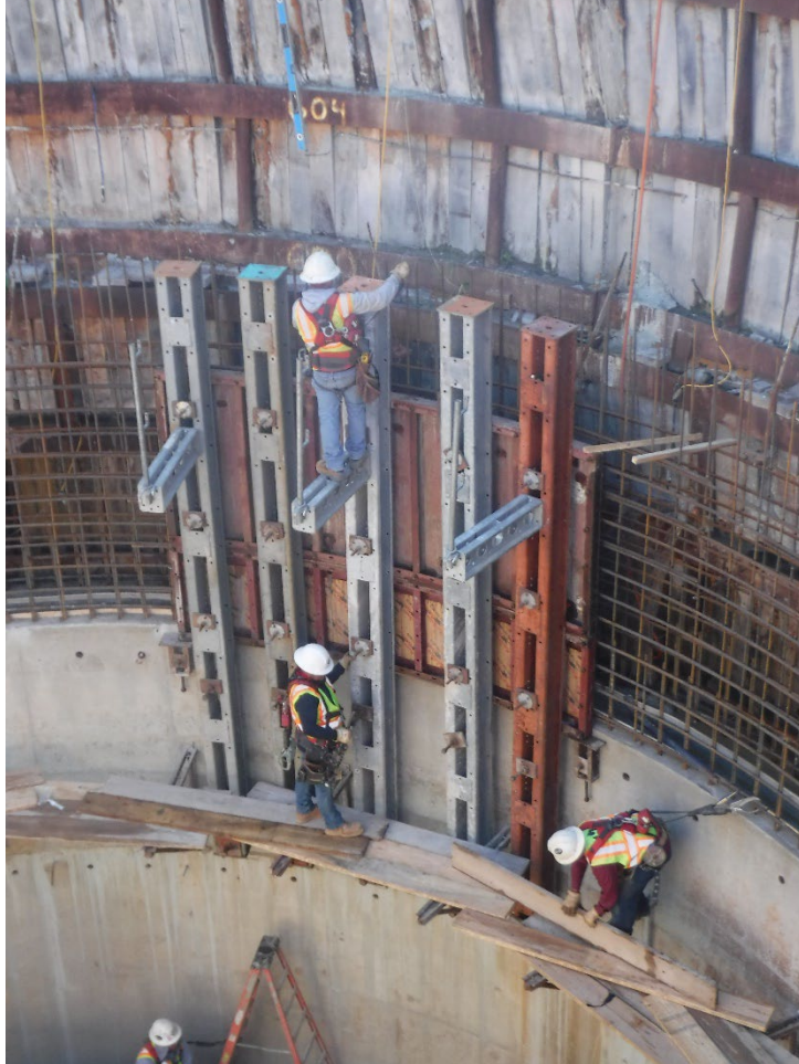
Figure 4 - CS-12 Wall Formwork Installation
