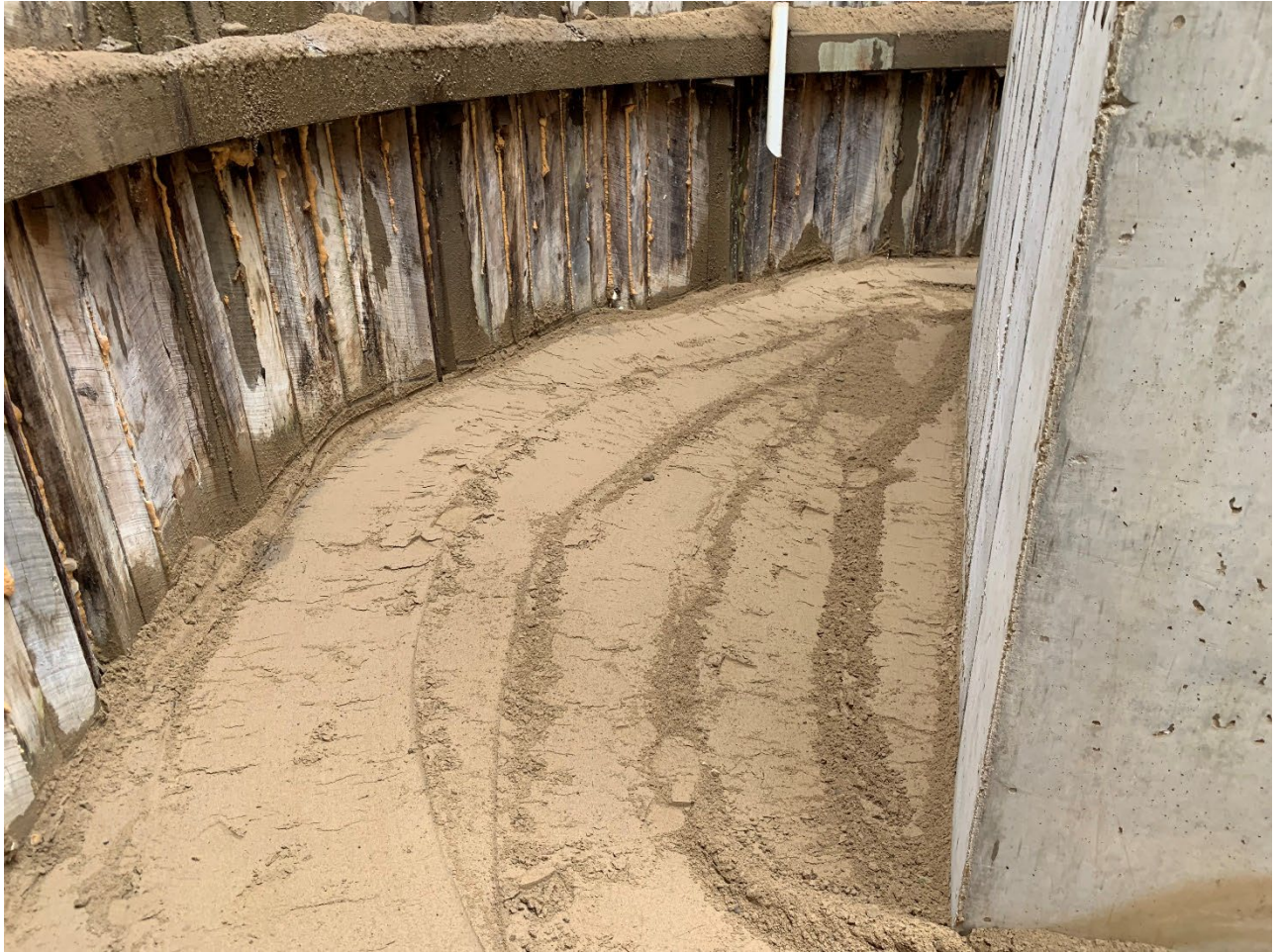
Figure 12 – CS-13 Sand Back-fill
