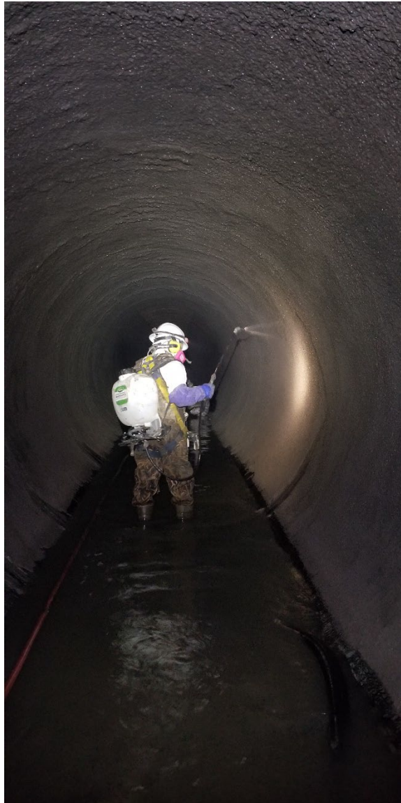
Figure 1 – Application of Geo-polymer Curing Agent PCI-37
