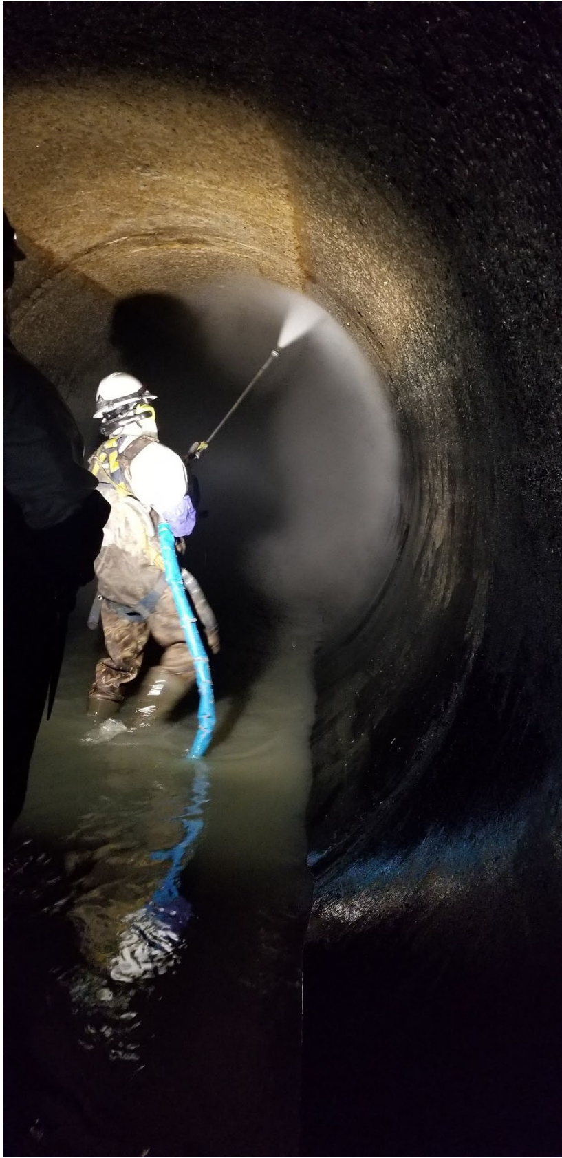
Figure 6 - PCI-37 Power Washing
