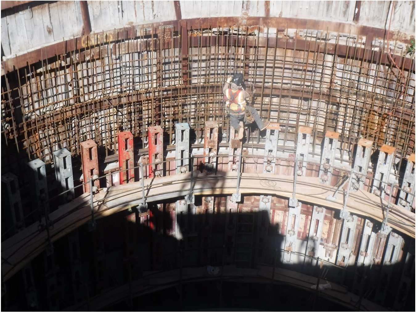
Figure 2 - CS-12 Rebar Installation
