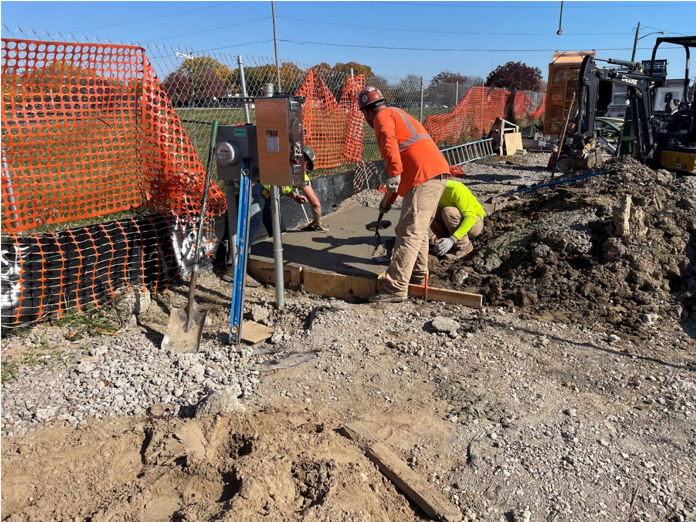
Figure 11 - CS-13 Equipment Pad Concrete Placement
