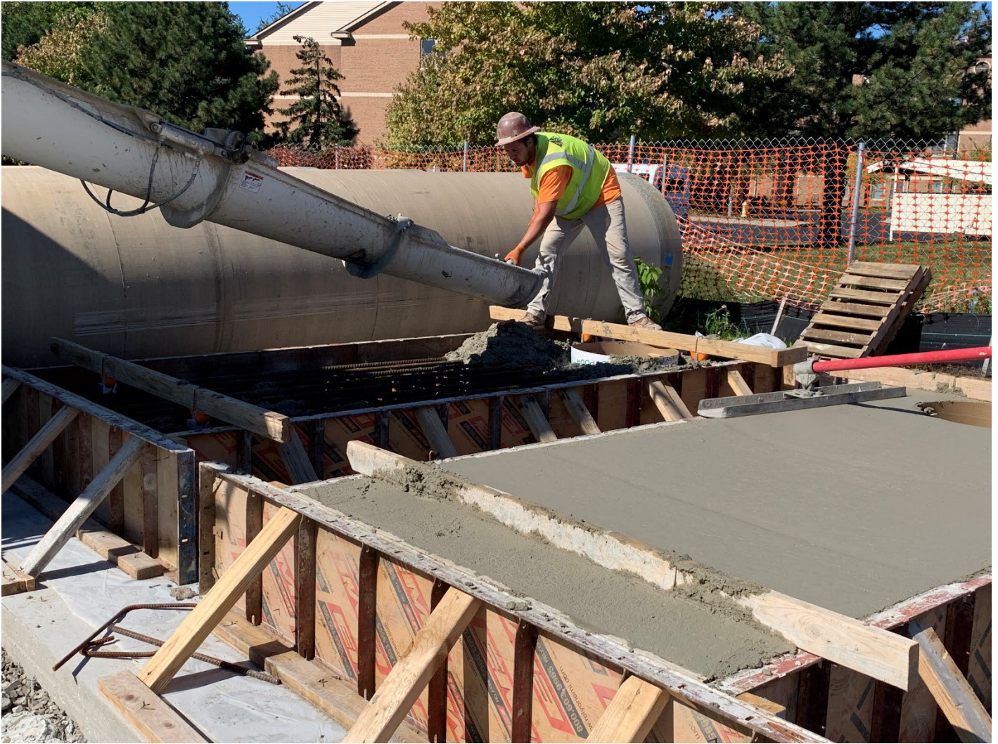
Figure 9 - CS-13 Concrete Top Placement
