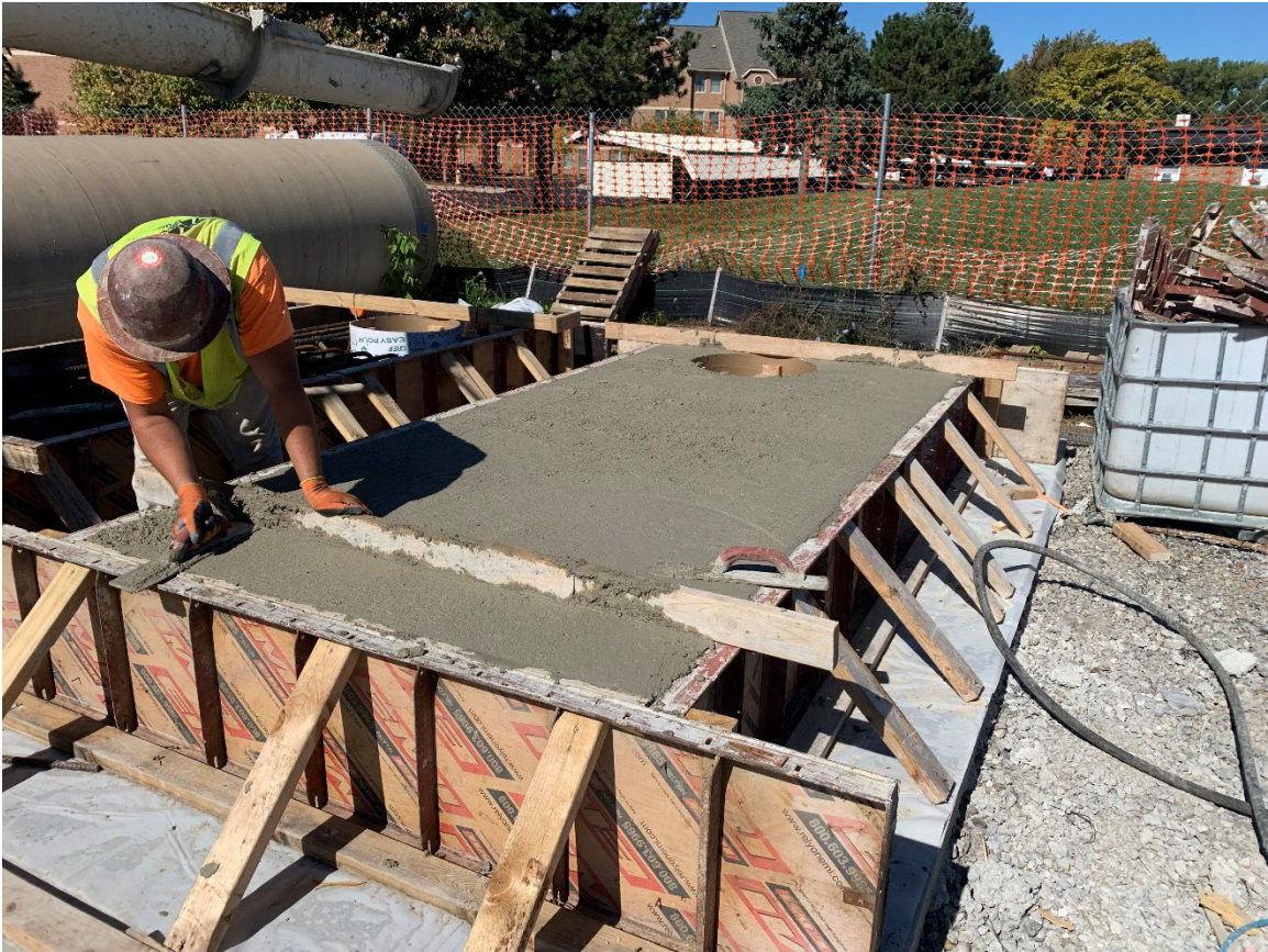
Figure 8 - CS-13 Concrete Top Placement
