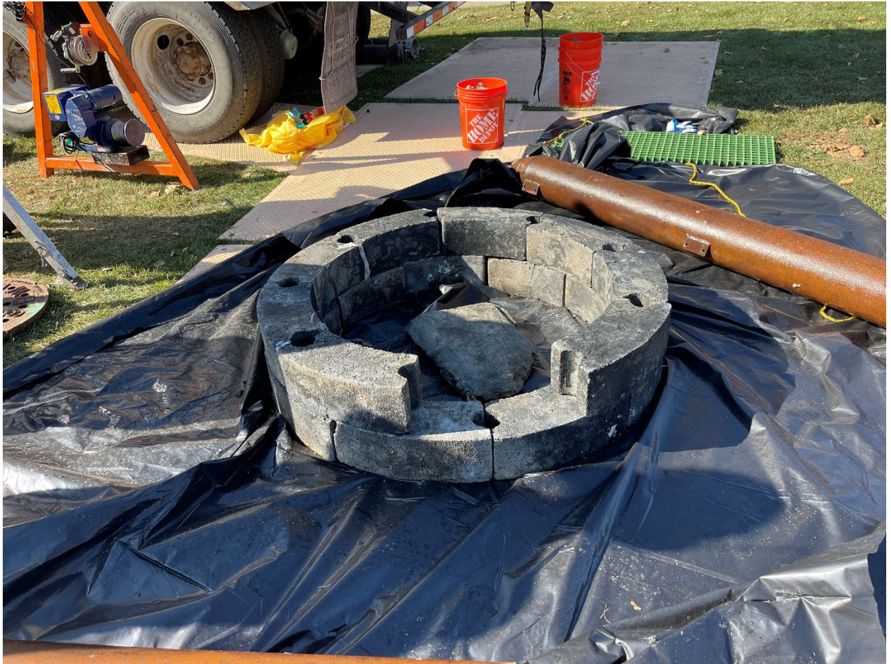
Figure 14 – Blocks and Debris Removed from the Garfield Interceptor
