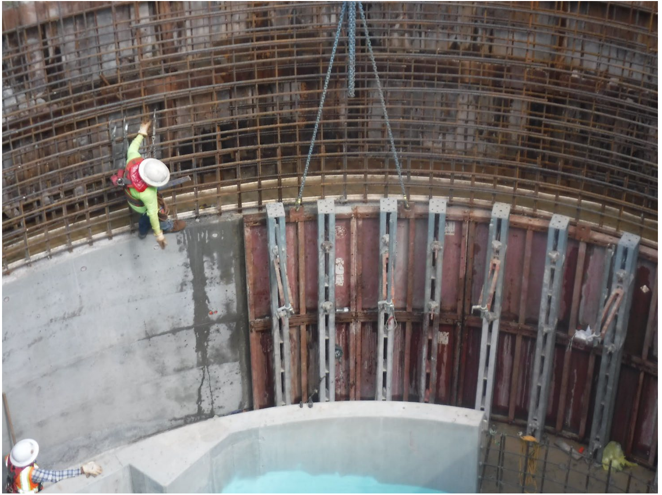
Figure 5 - CS-12 Wall Formwork Removal
