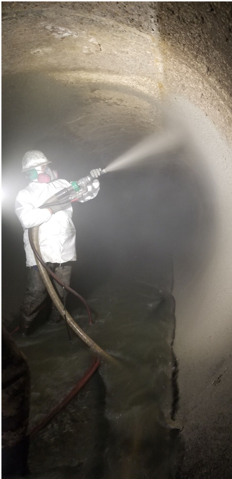
Figure 7 - PCI-37 Spray Lining Application
