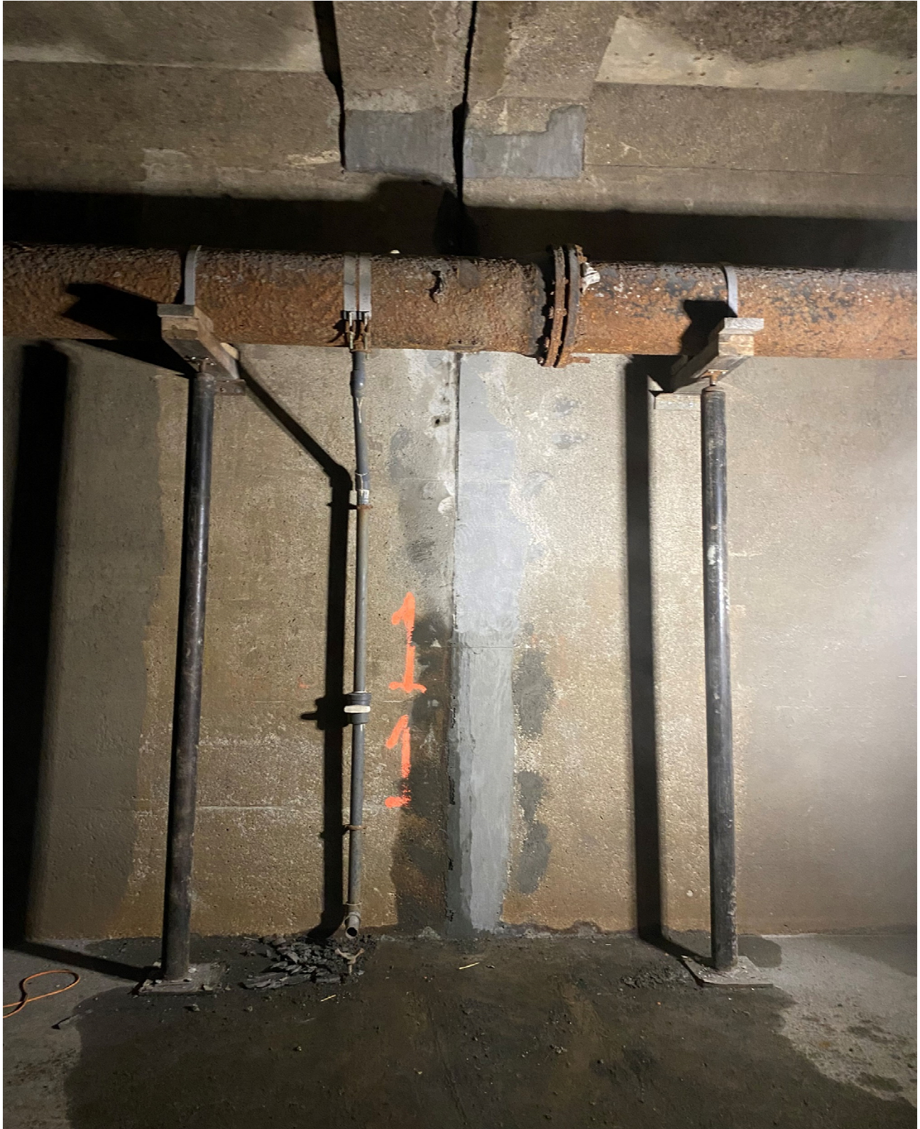
Figure 4 - Concrete Patch Repair
