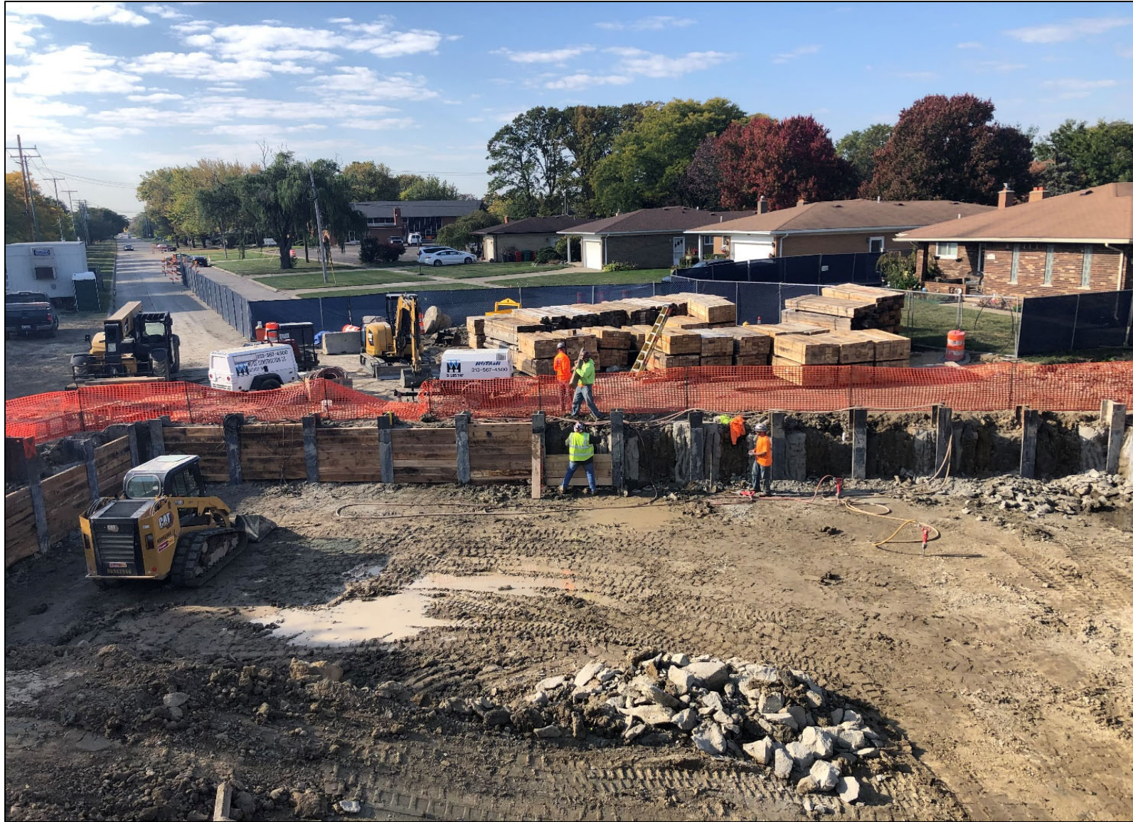
Figure 2 – Installing Timber Retaining Walls
