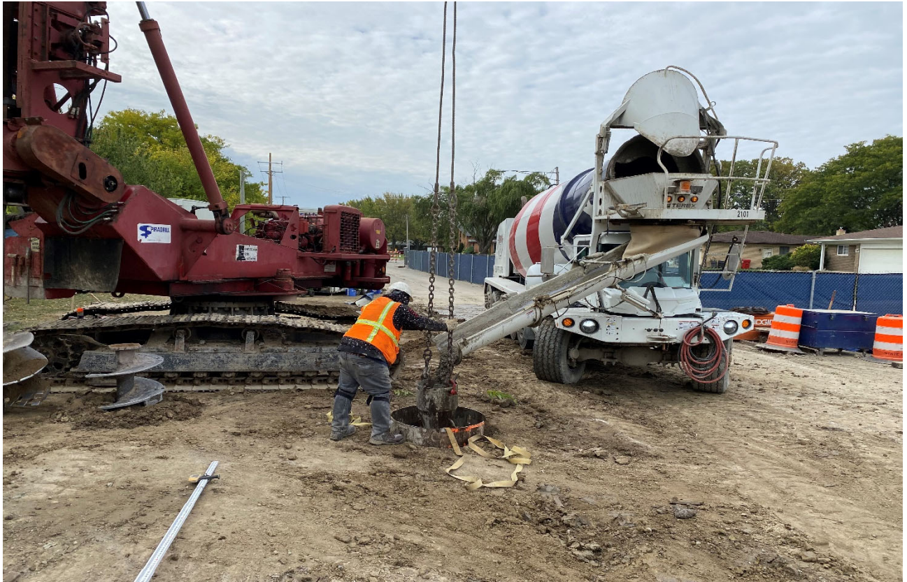
Figure 3 – Encasing Piers in Concrete
