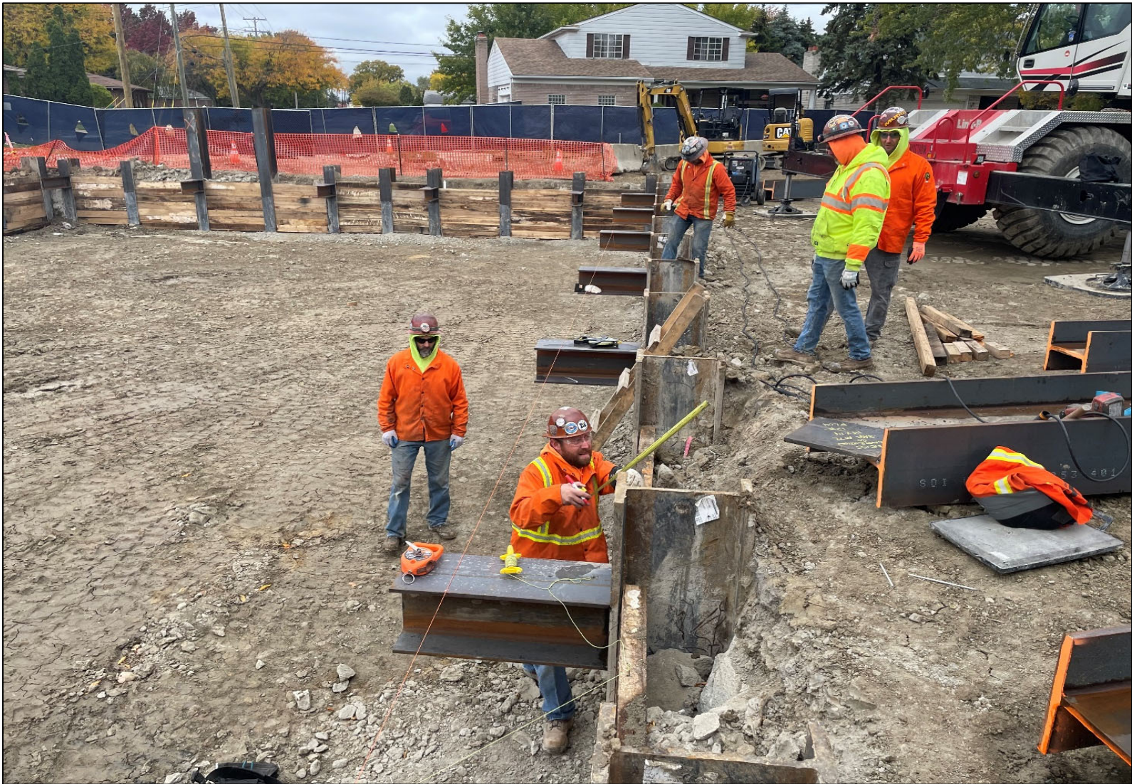
Figure 3 – Top Tier Bracing and Support Layout
