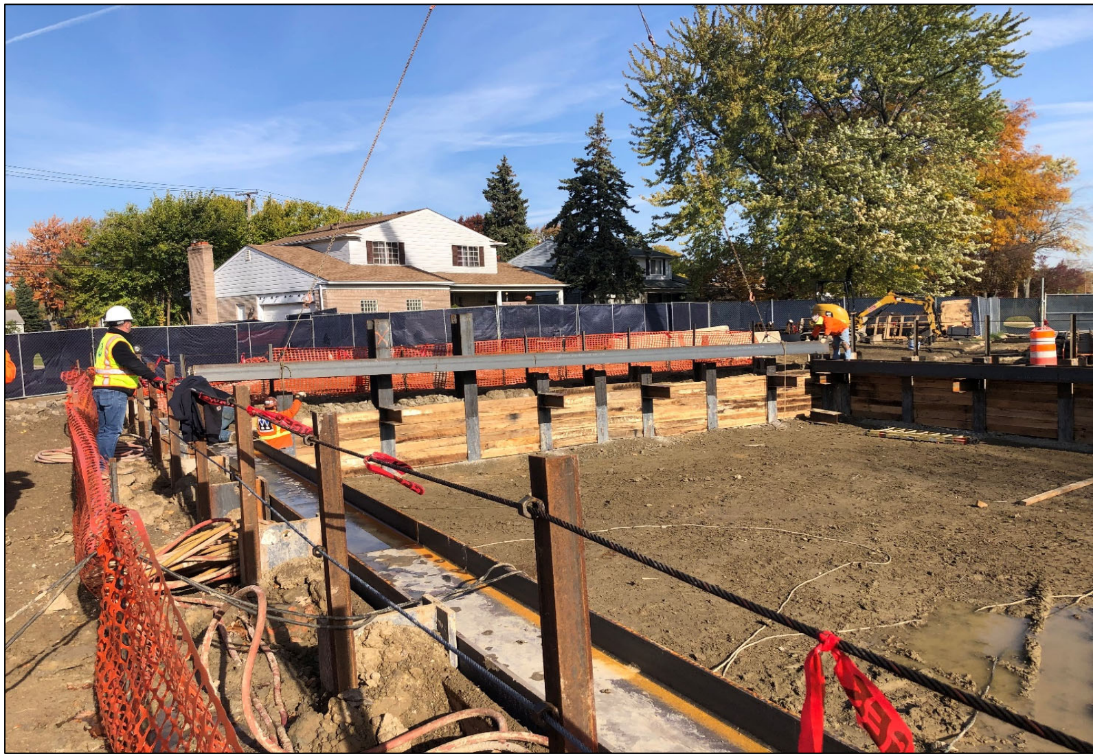
Figure 4 – Installed Safety Railing
