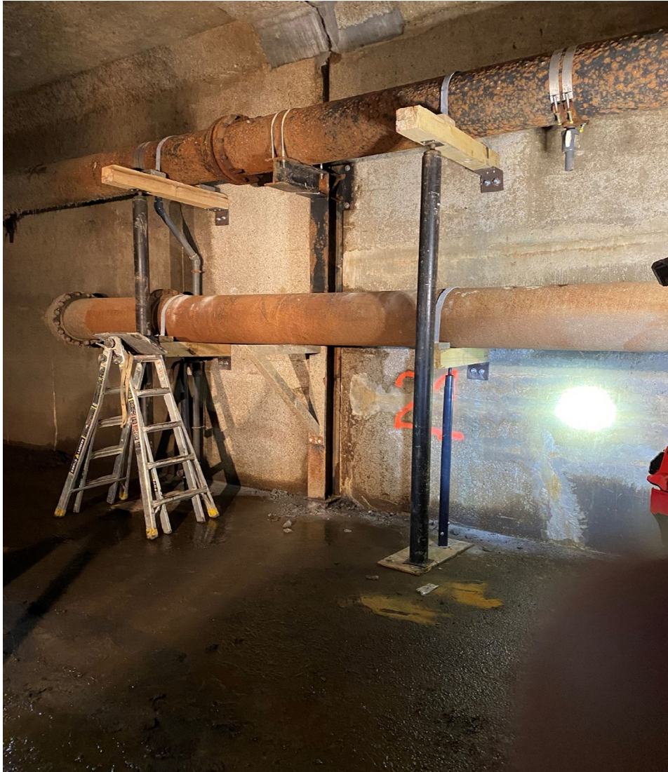
Figure 1- Temporary Pipe Supports
