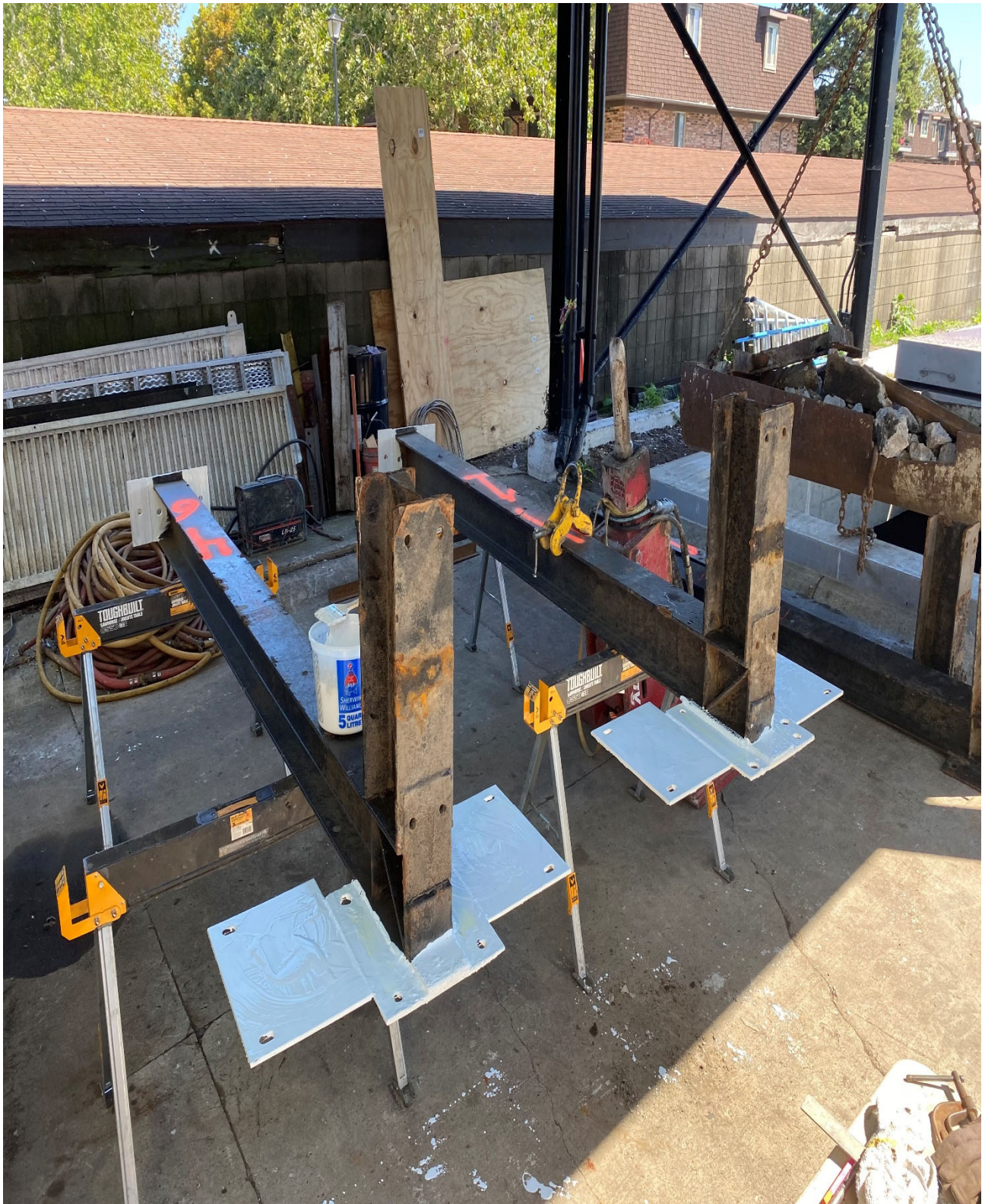
Figure 3 – Fabricating Flushing Pipe Support Beams
