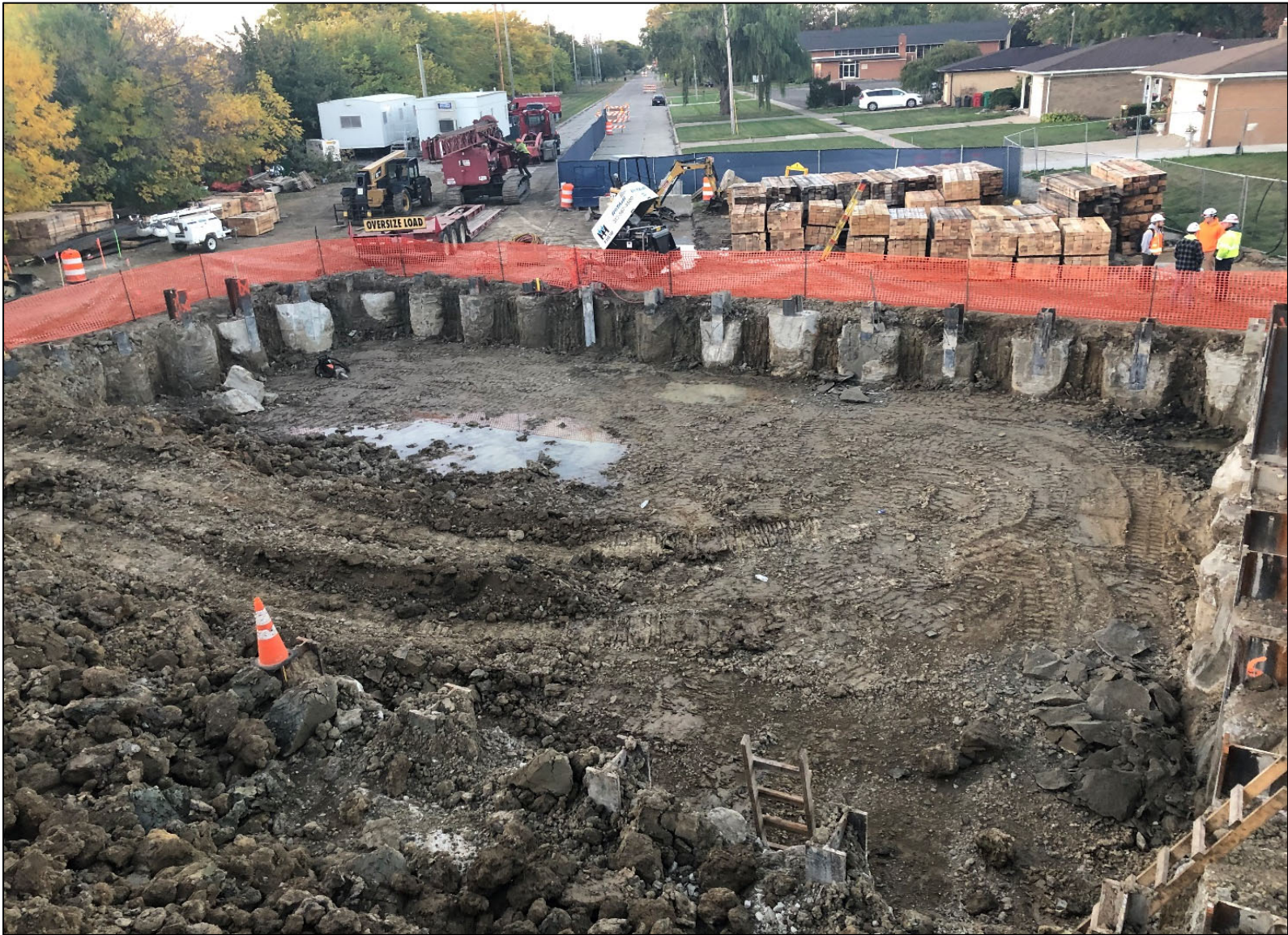
Figure 1 – Beaconsfield Shaft Excavation
