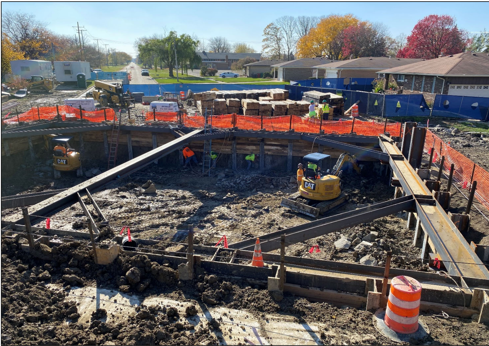
Figure 6 – Shaft Excavation @ Approx. 10ft
