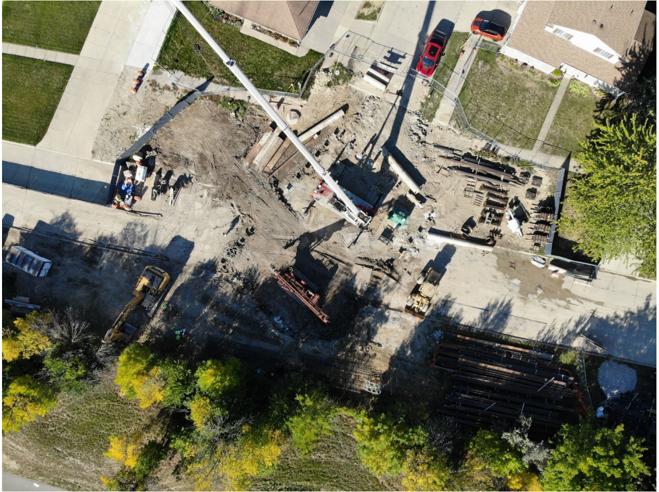
Figure 5 – Aerial Drone Image Showing Soldier Piles Being Installed
