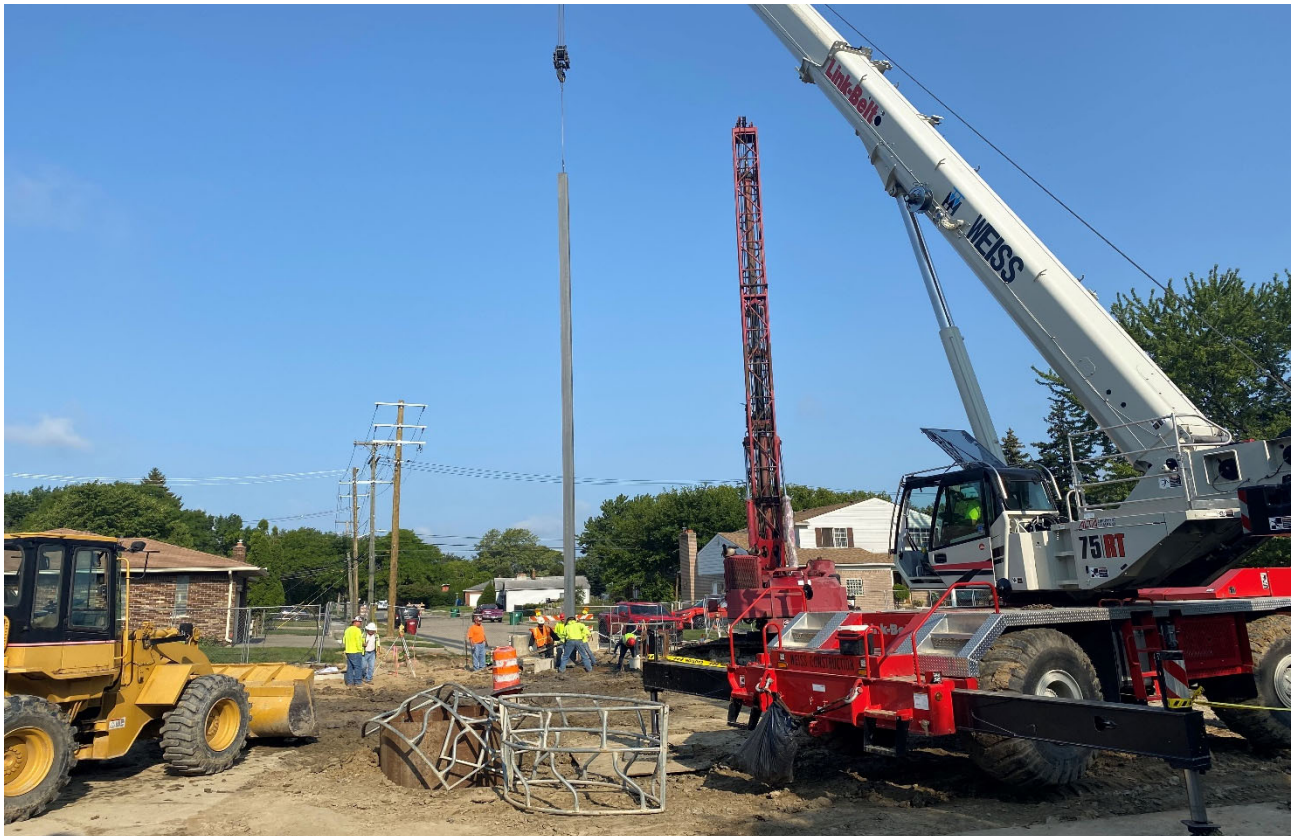
Figure 2 – Lowering 55FT I-beam Pier into Drilled Hole
