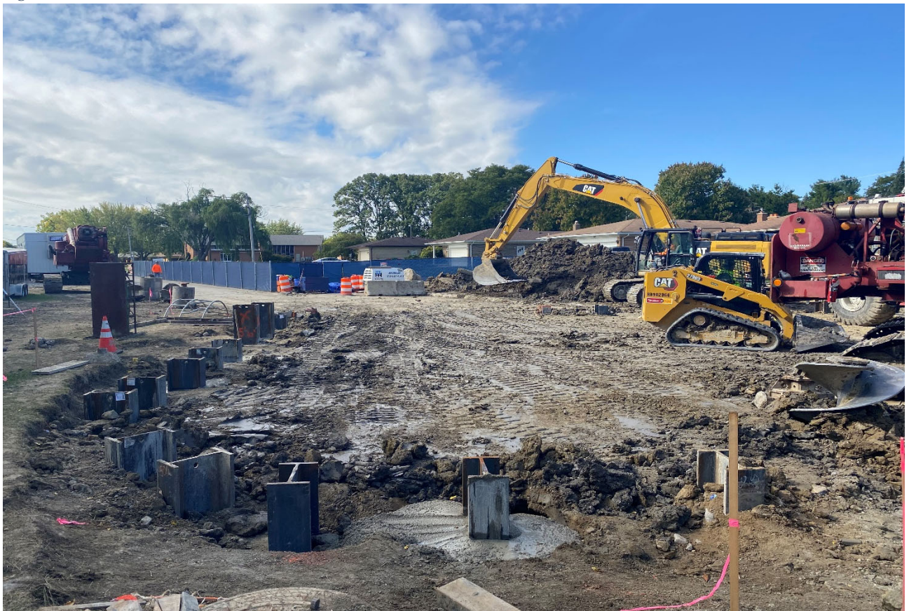
Figure 4 – Installed Steel I-beam Piers
