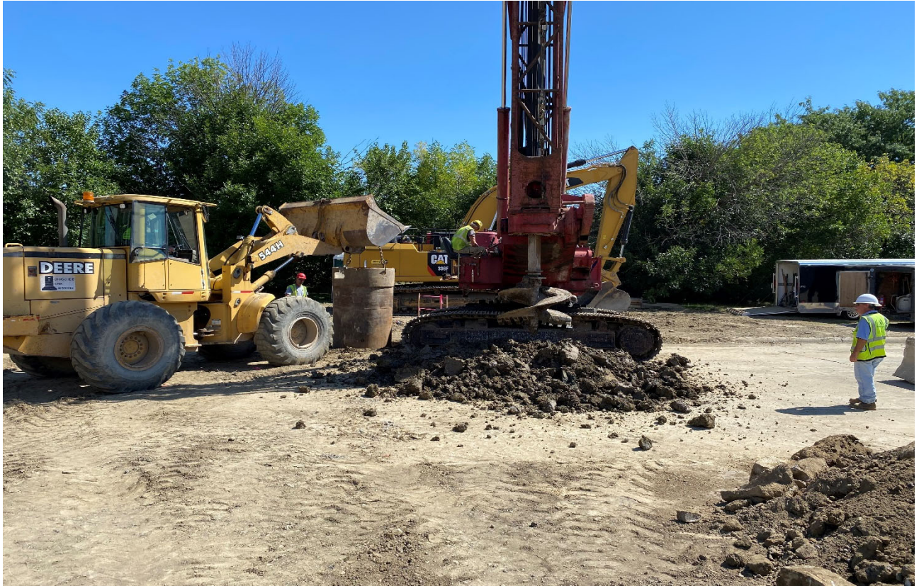
Figure 1 – Drilling Hole for I-Beam Pier
