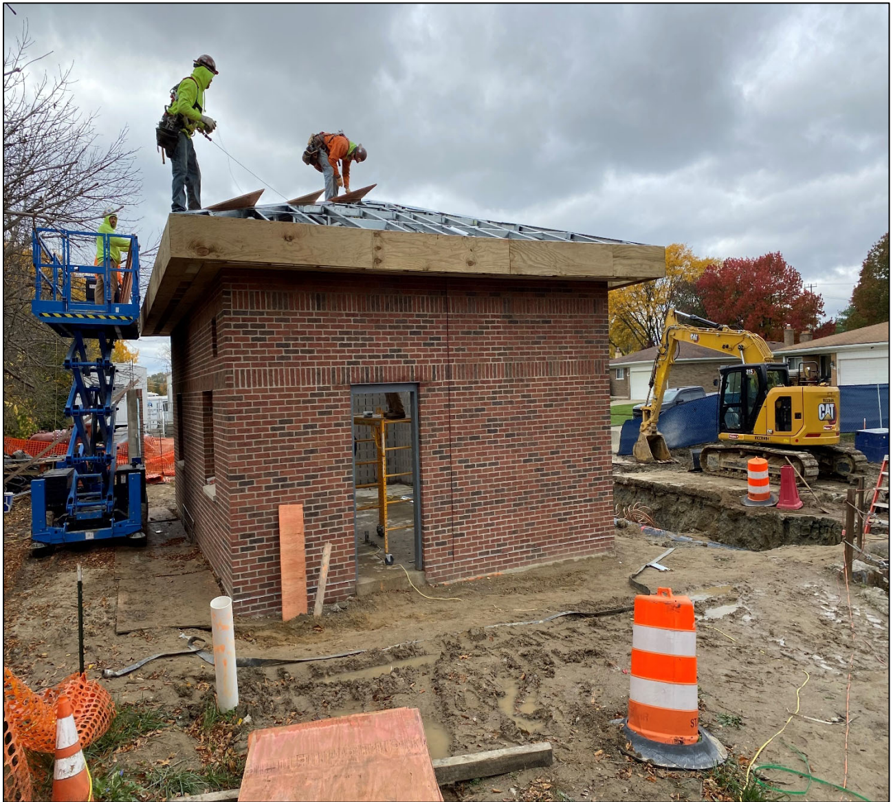
Figure 10 – Installing Roof Sheeting & Overhang @ Beaconsfield Control Bldg.
