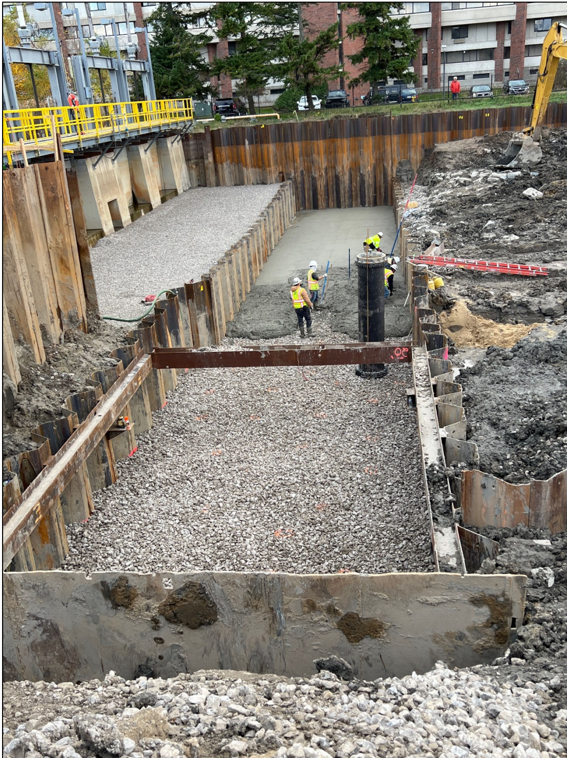
Figure 17 – Pouring concrete mudmat for Outfall Structure
