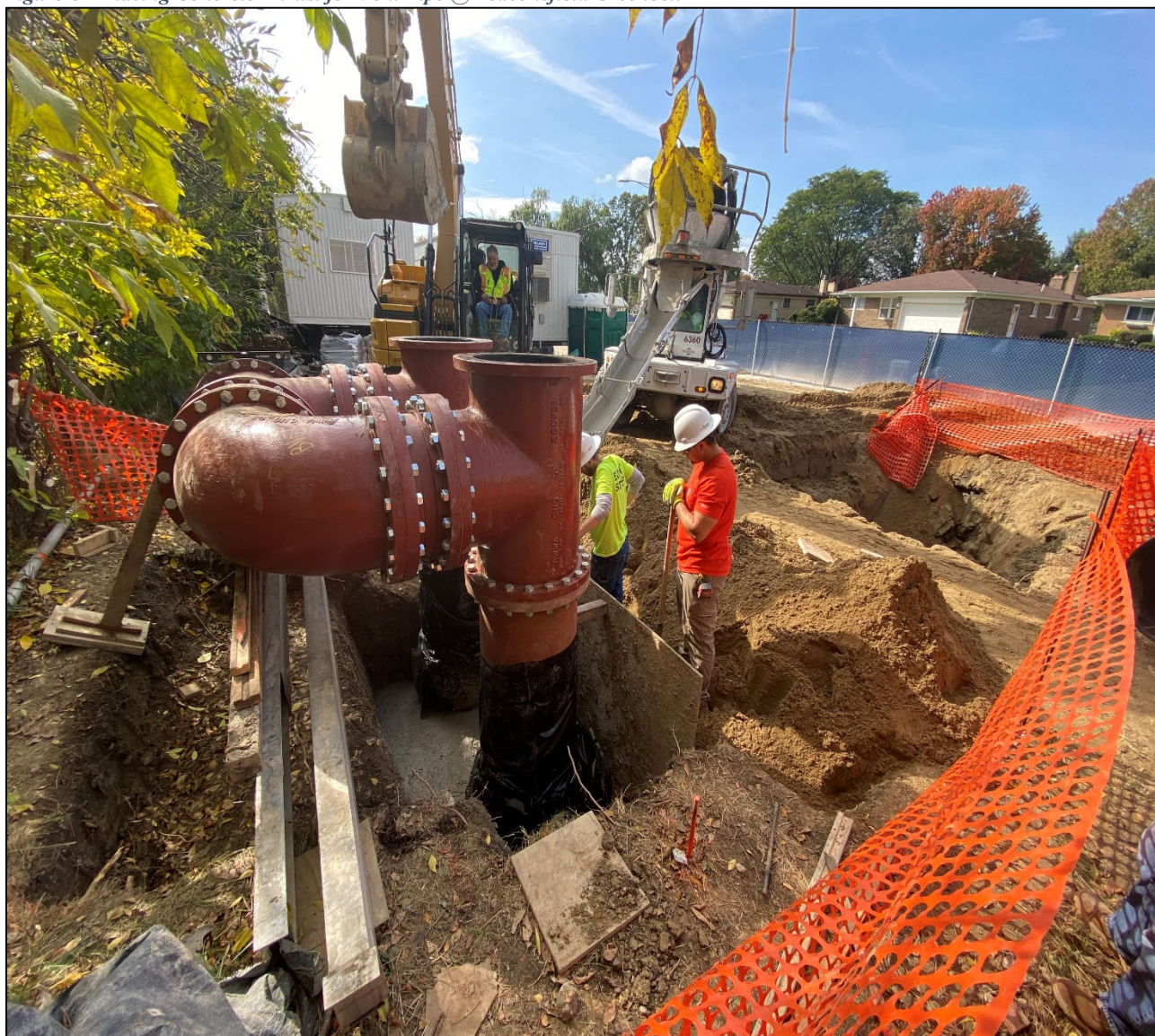
Figure 6 – Placing Concrete Thrust for Vent Pipe @ Beaconsfield Greenbelt
