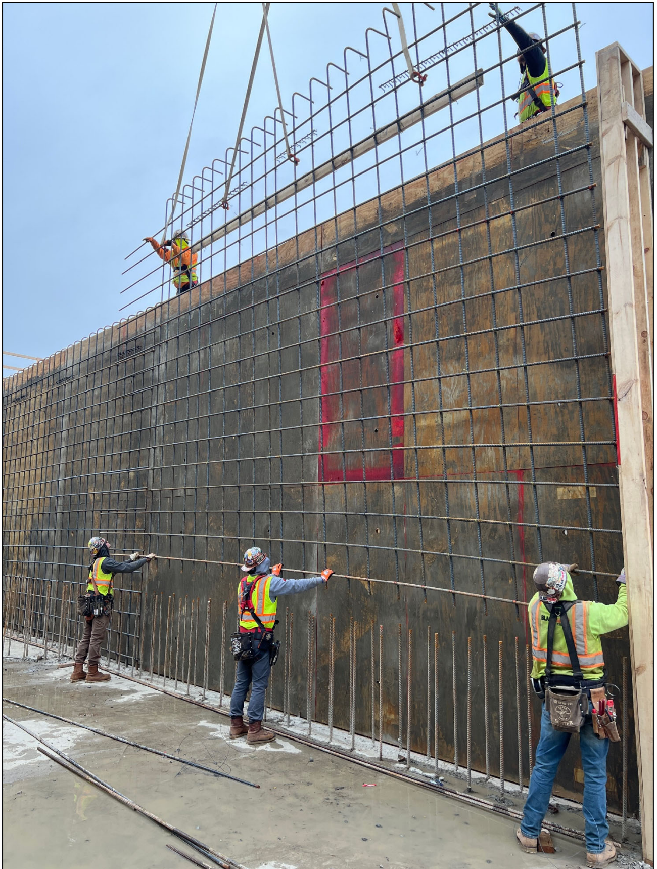
Figure 13 – Lowering pre-assembled reinforcement into place for divider wall
