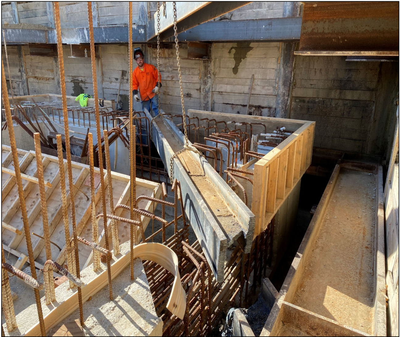
Figure 1 – Removing Steel I-Beams @ Beaconsfield Shaft
