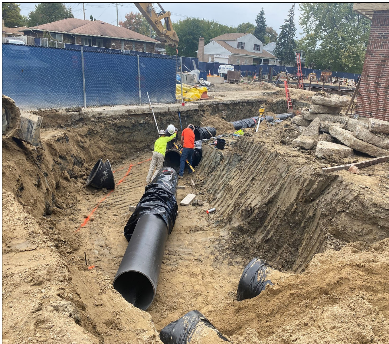
Figure 5 – Installing 24in Vent Pipe @ Beaconsfield Road
