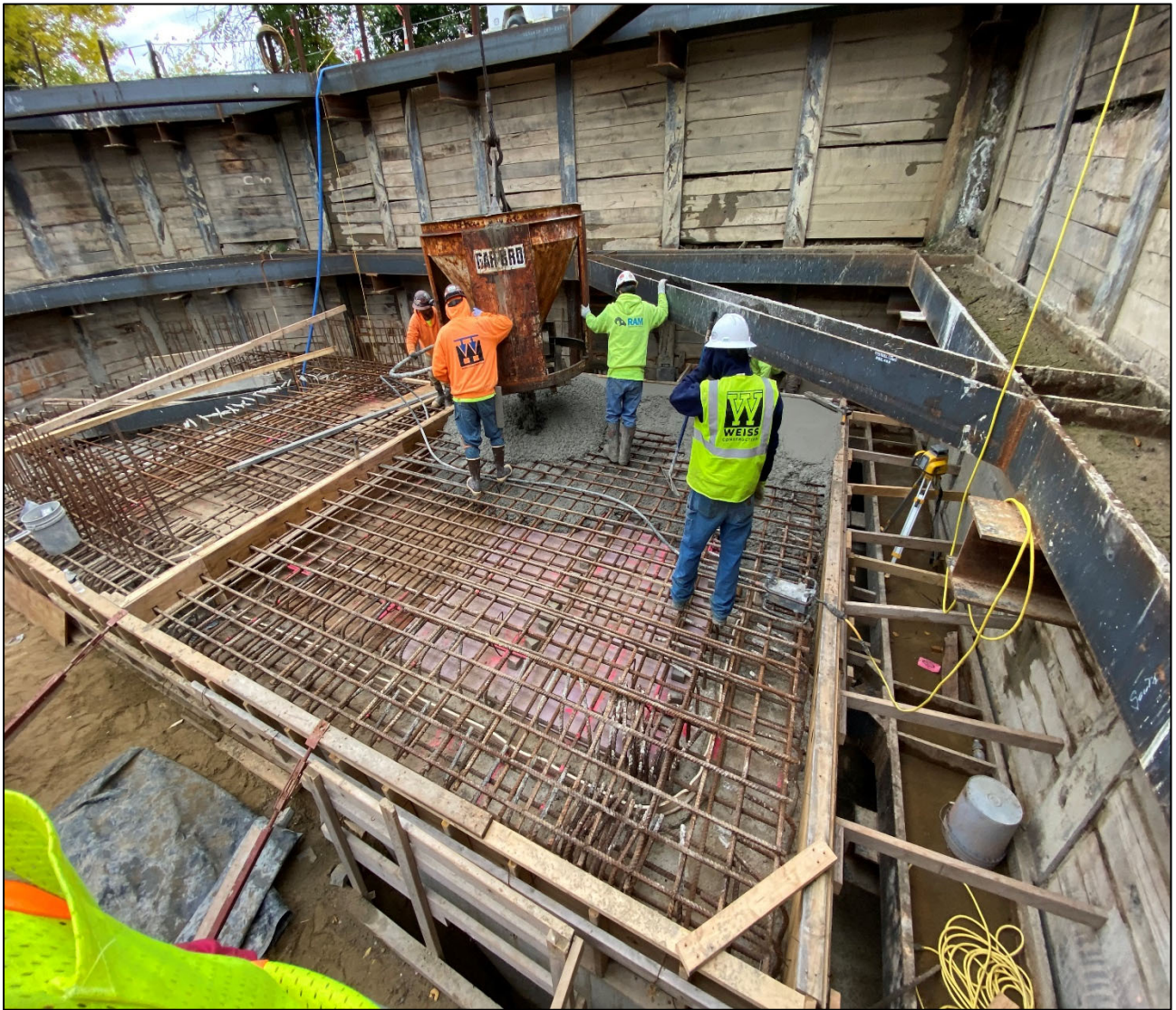
Figure 4 – Placing Mechanical Room Concrete Floor @ Beaconsfield Shaft
