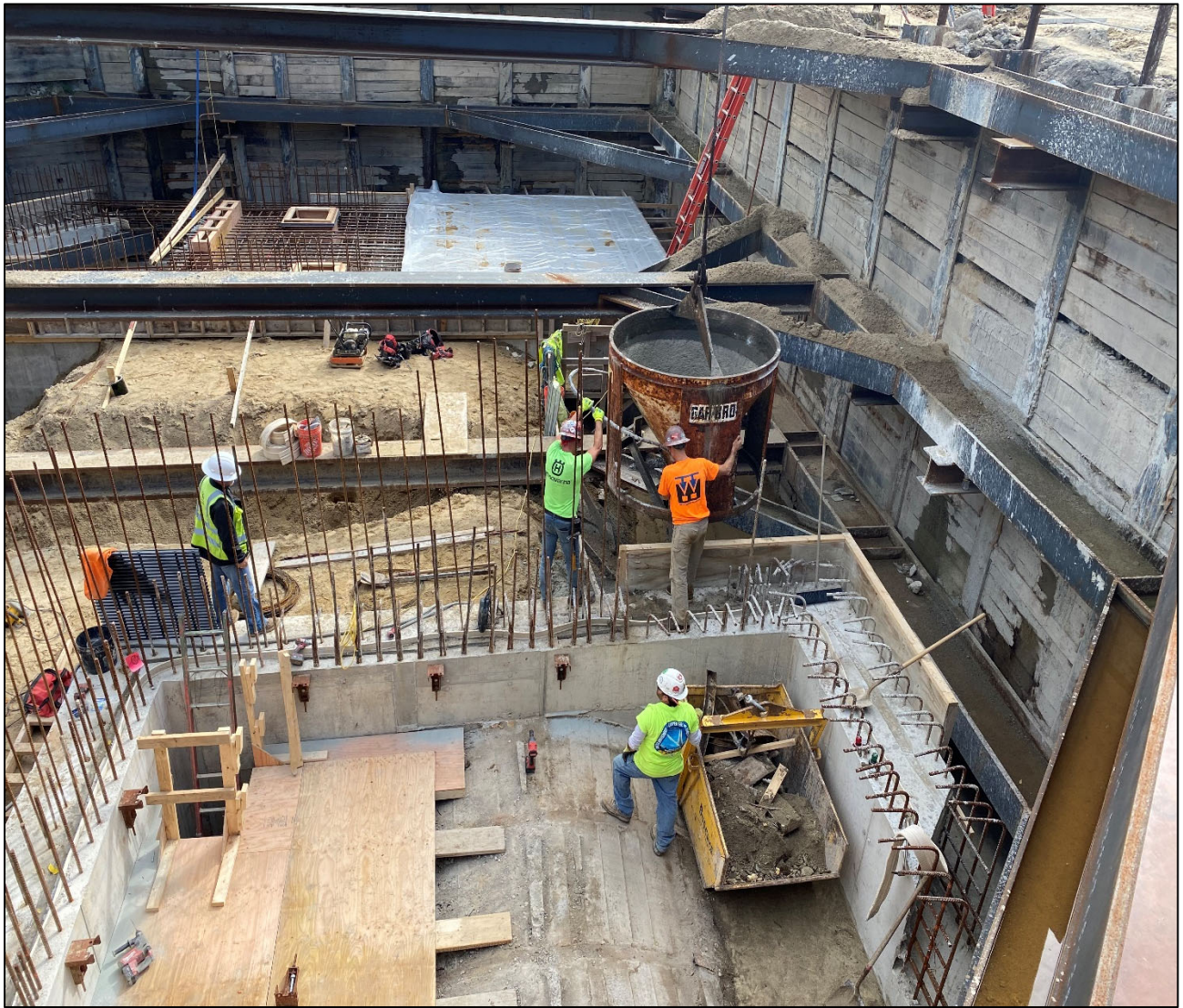
Figure 2 – Placing Concrete Backfill @ Beaconsfield Shaft
