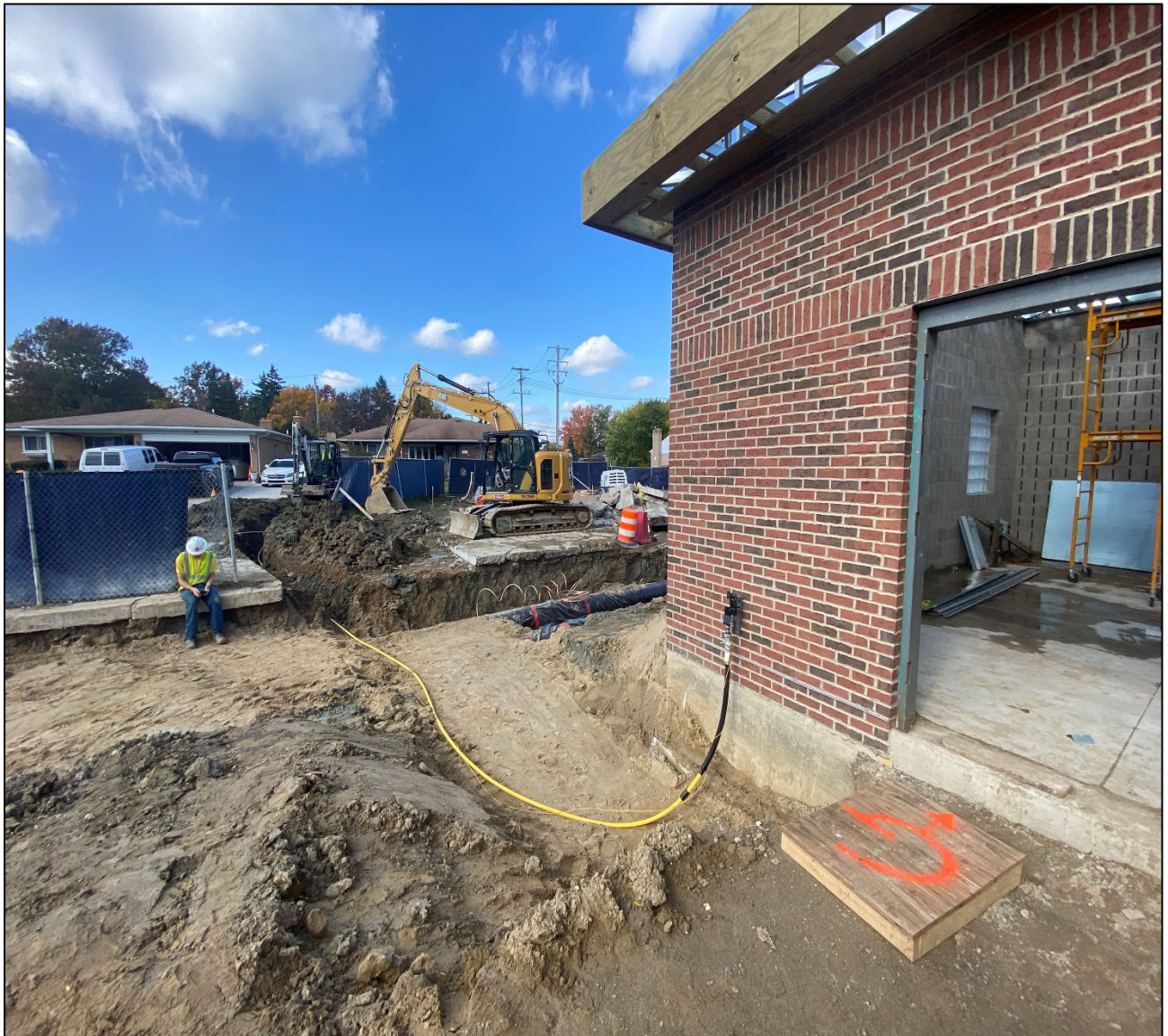
Figure 8 – New Gas Line @ Beaconsfield Control Bldg.
