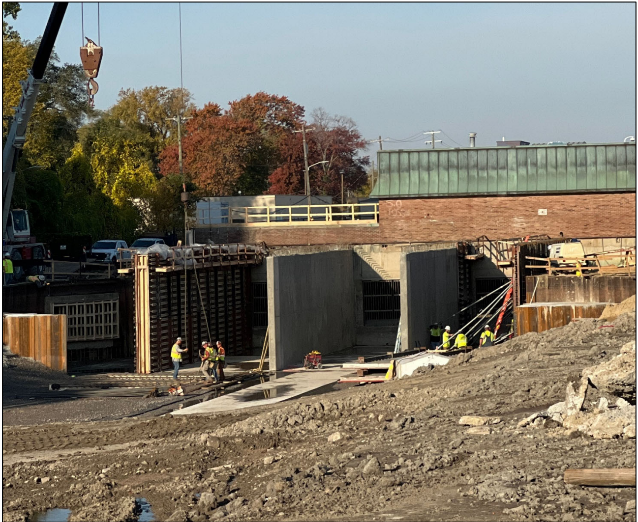
Figure 12 – Screening Structure divider walls in various stages of construction
