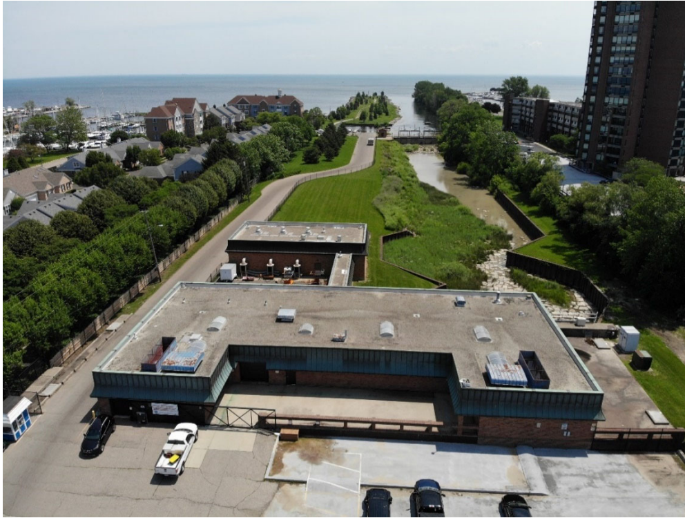
Figure 19 – Drone Aerial at 100 FT Facing East (Baseline)
