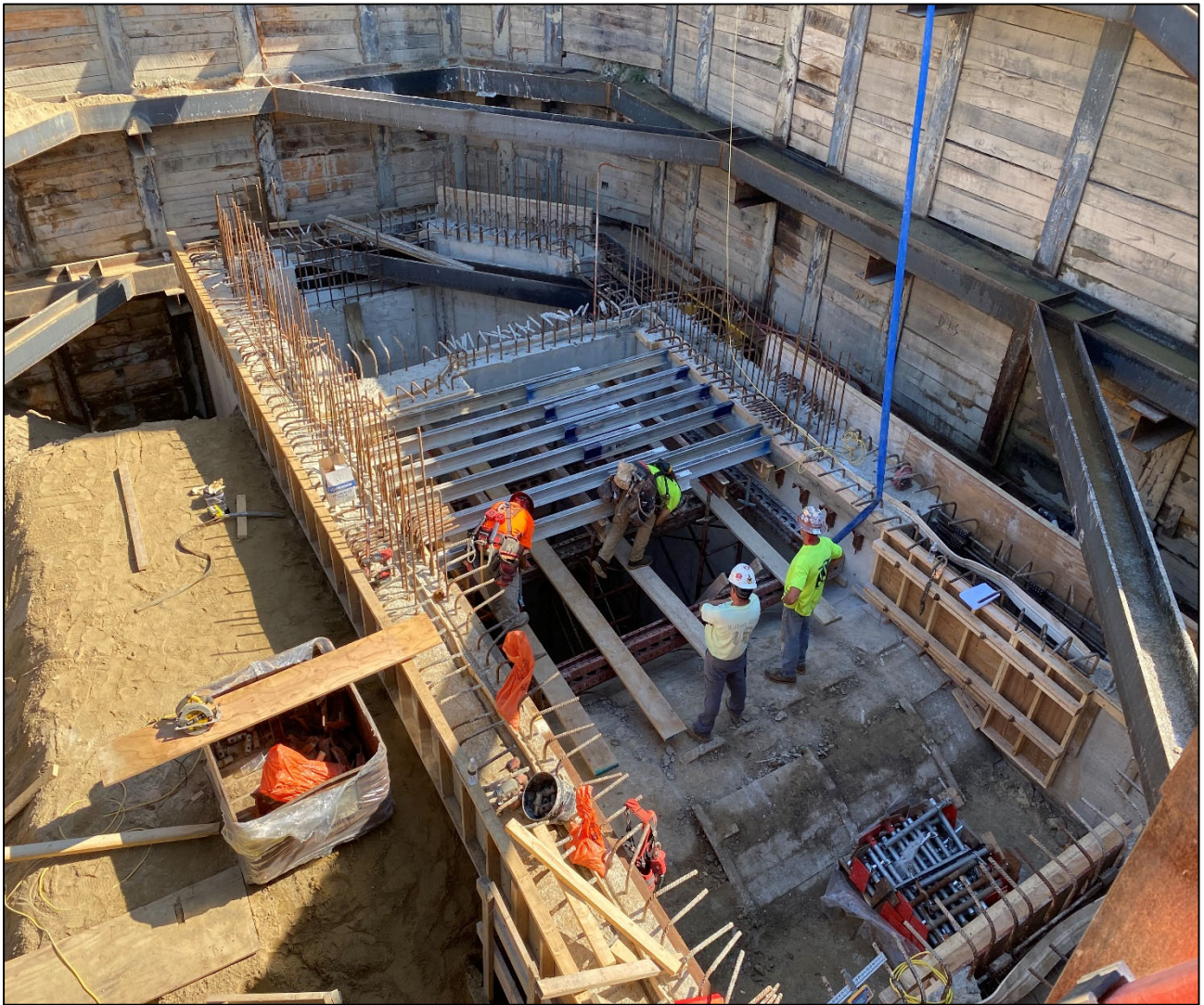
Figure 3 – Installing Supports for Mechanical Room Floor @ Beaconsfield Shaft
