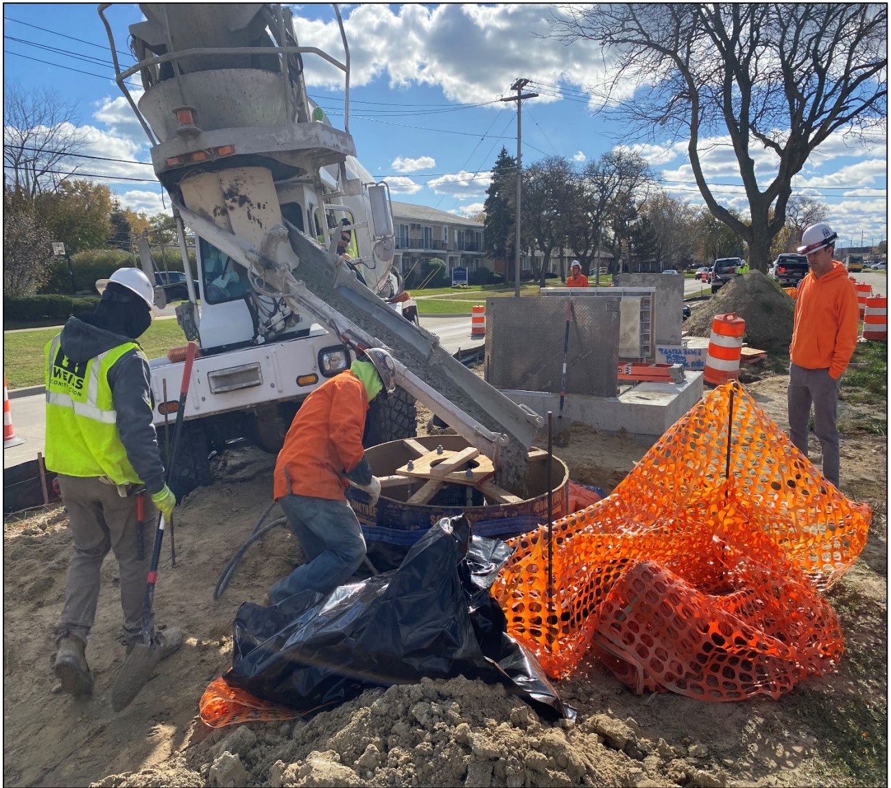
Figure 7 – Placing Concrete Lampstand Bases @ Kelly Rd. Blvd.
