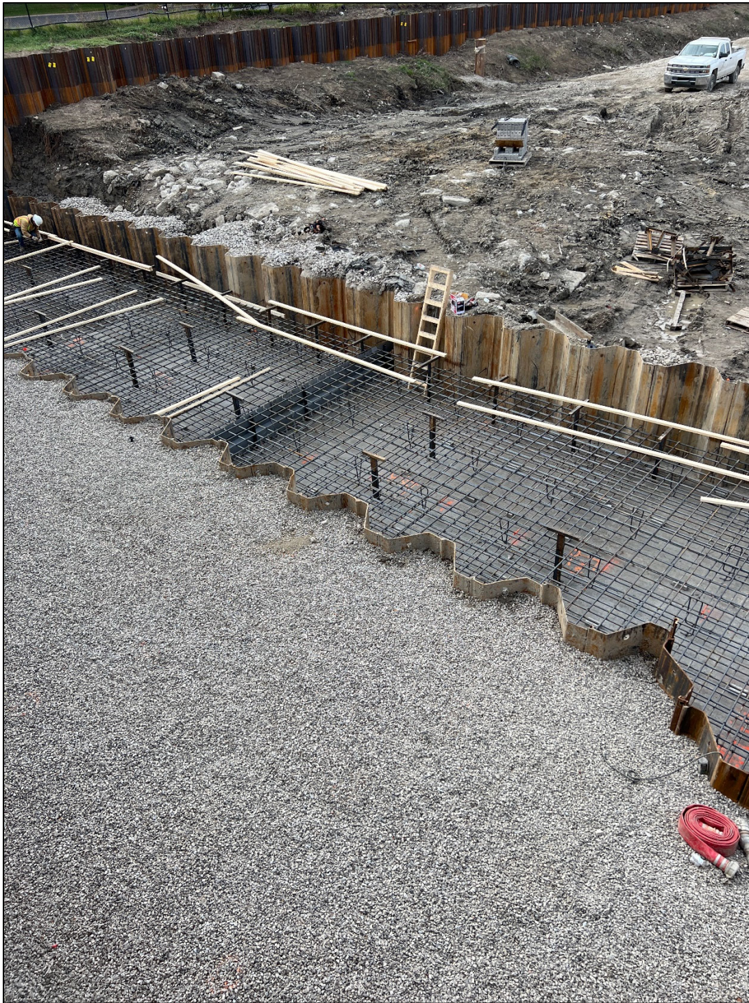
Figure 18 – Steel reinforcement for Outfall Structure base slab
