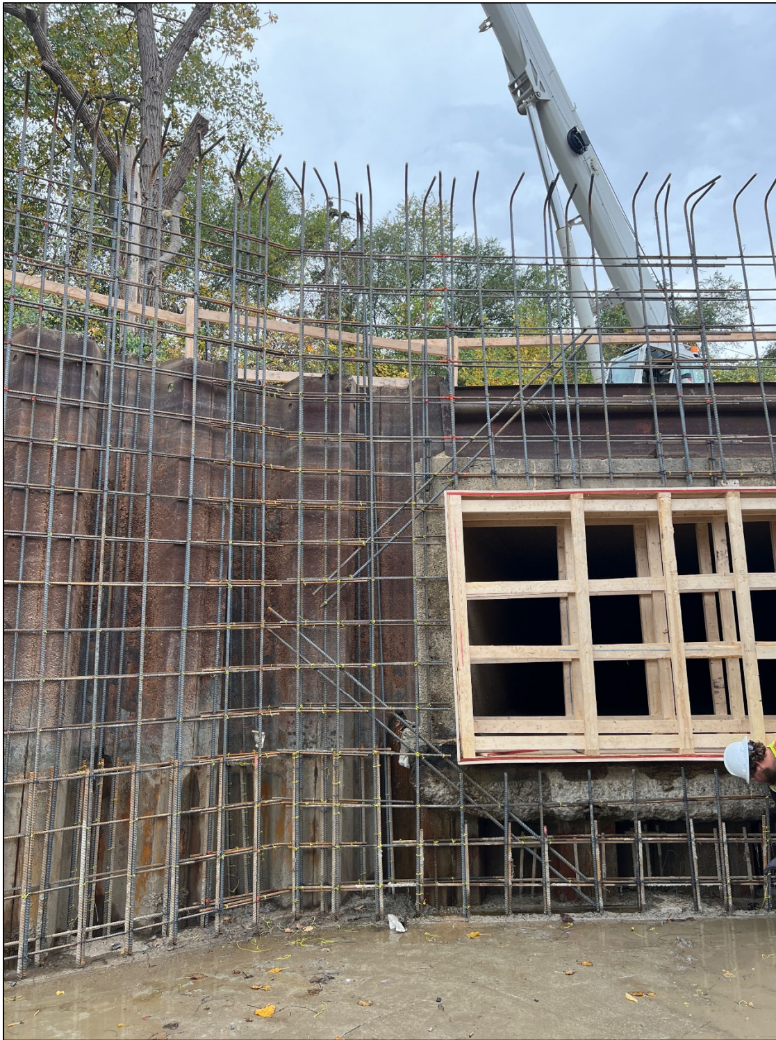
Figure 14 – Reinforcement for southerly wall of Screening Structure with boxout for 9EB
