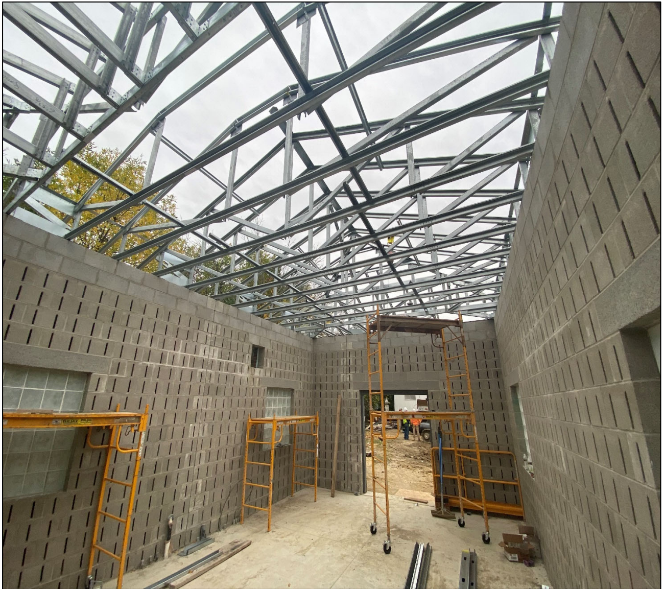
Figure 9 – Installing Roof Trusses @ Beaconsfield Control Bldg.
