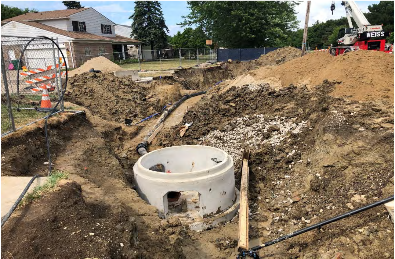
Figure 3 – New Water Main and Gate Well Valve
