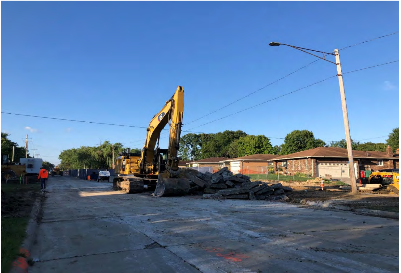
Figure 5 – Removed Concrete at Oak & Beaconsfield Intersection
