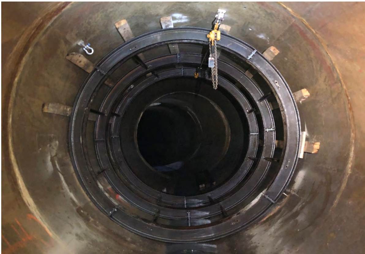
Figure 4 – Installed Steel Bracing Ribs in 11FT Tunnel
