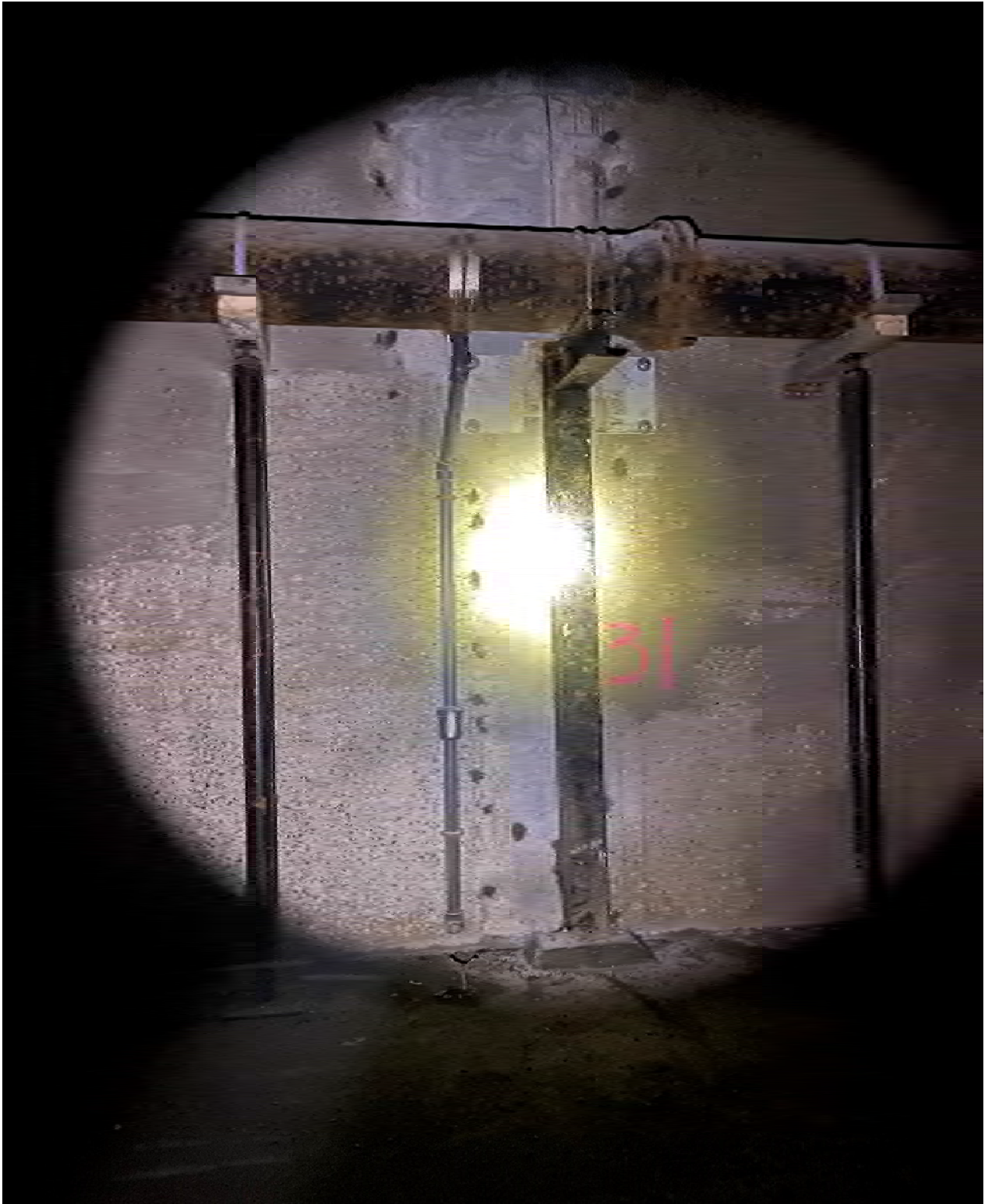
Figure 5 – Installed Slotted Beams
