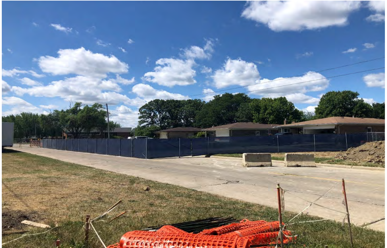
Figure 2 – Fencing Installed at Construction Site
