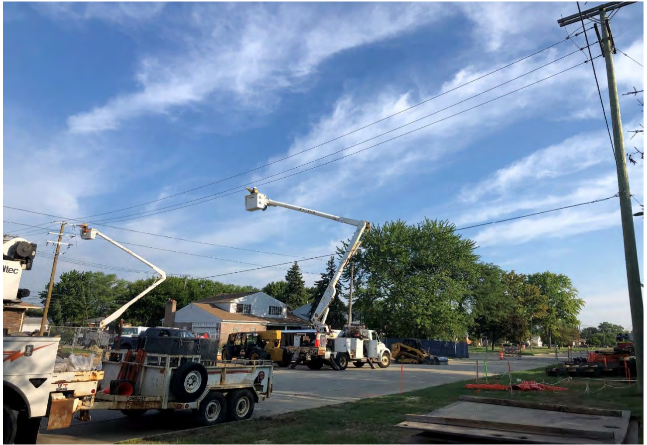
Figure 1 – Relocating Existing Power Lines
