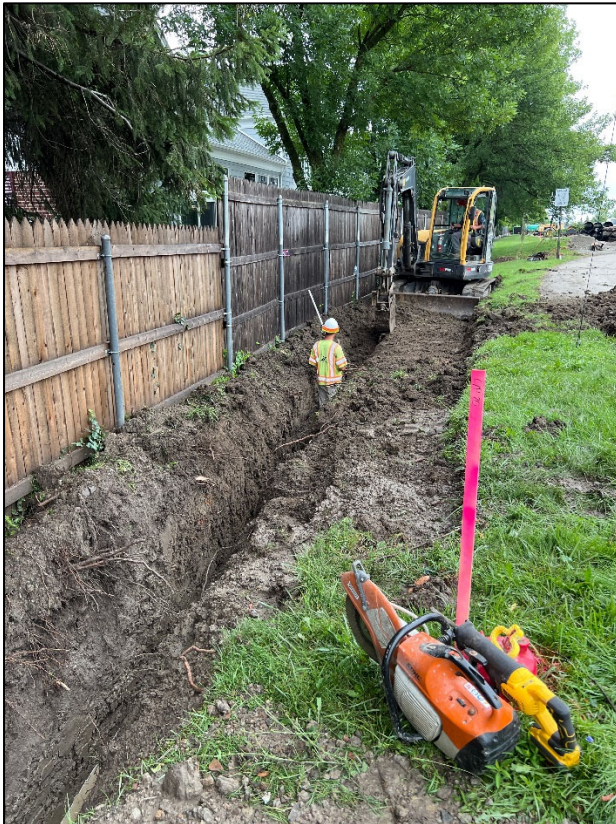
Figure 11 – Temporary Utility Trench
