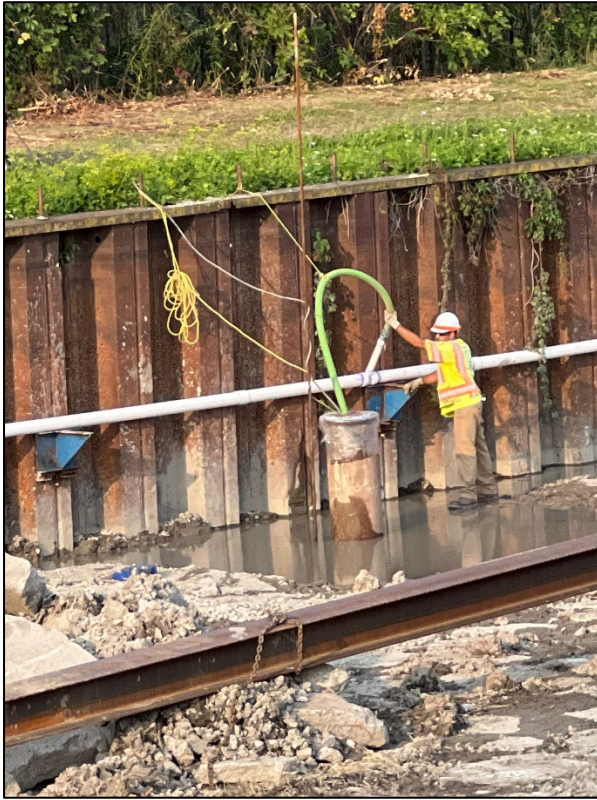
Figure 10 – Dewatering Well and Discharge Header
