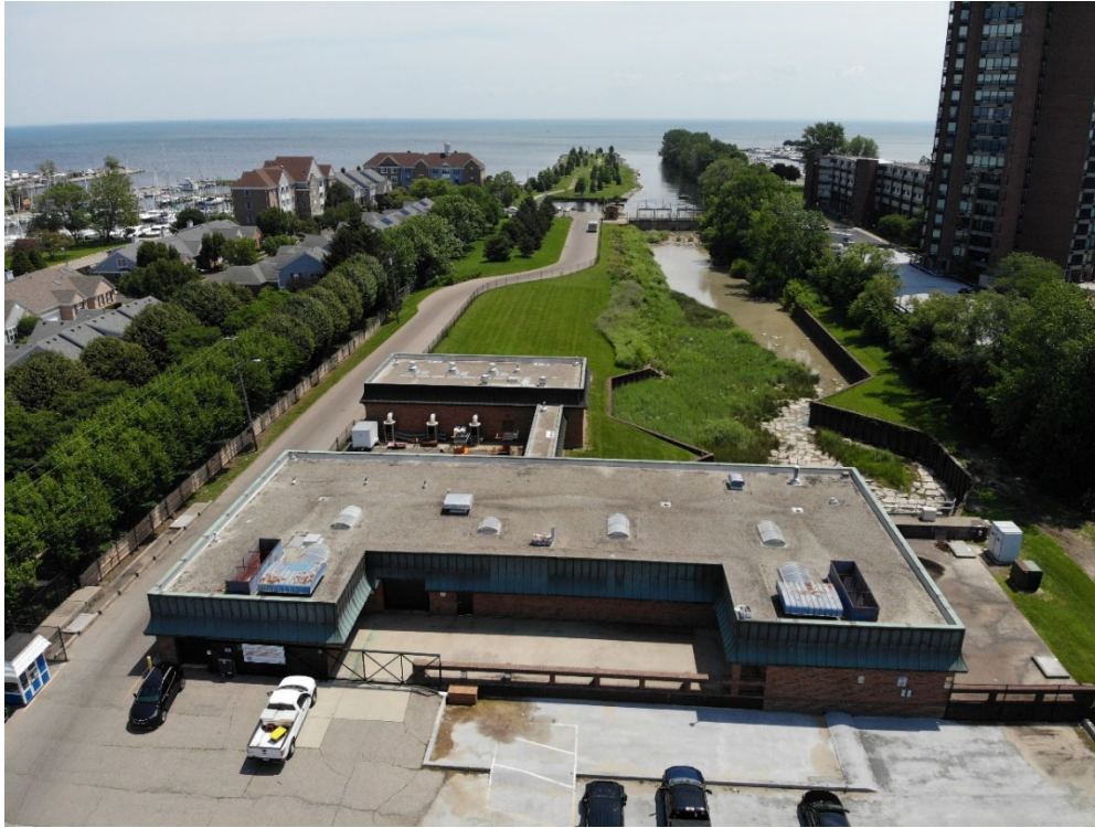
Figure 13 – Drone Aerial at 100 FT Facing East (Baseline)
