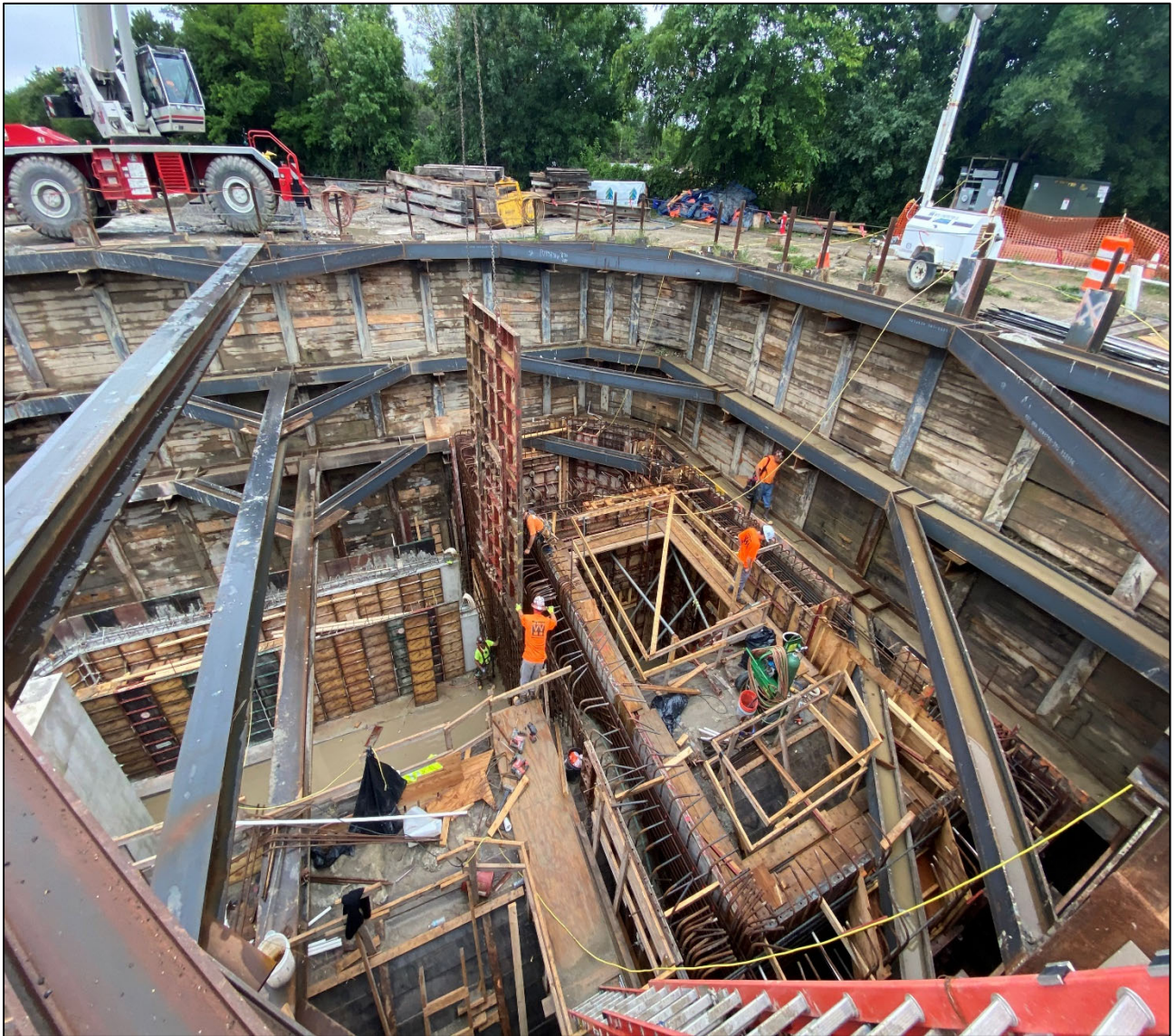
Figure 5 – Installing Wall Forms @ East Wall of Beaconsfield Shaft
