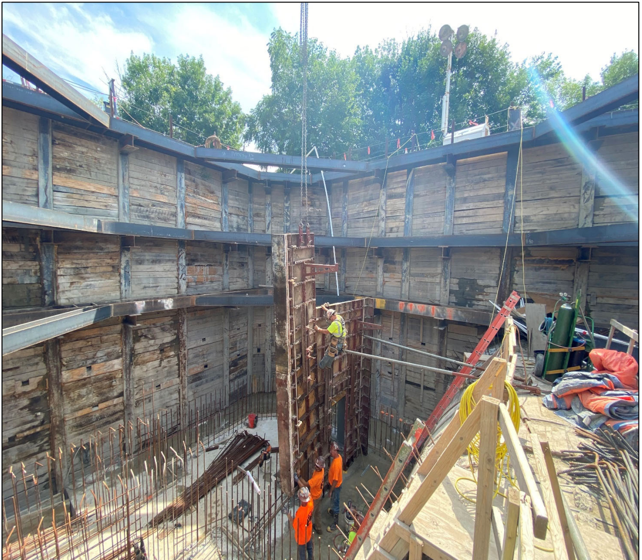
Figure 3 – Setting Concrete Wall forms @ East side of Beaconsfield Shaft
