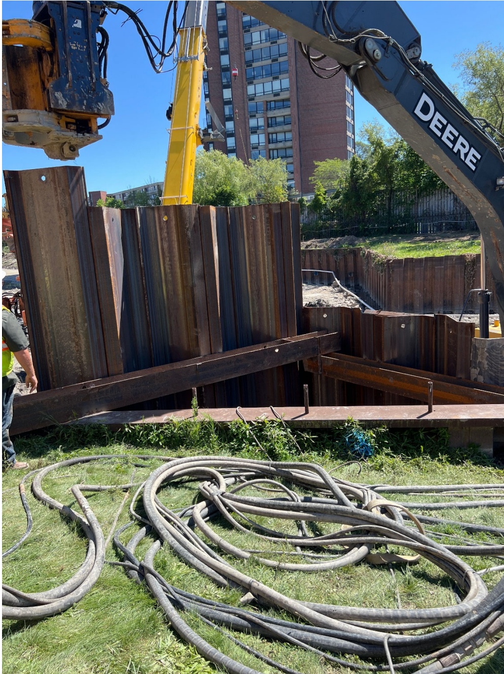
Figure 12 – North Side Sheeting: New, Existing, Template
