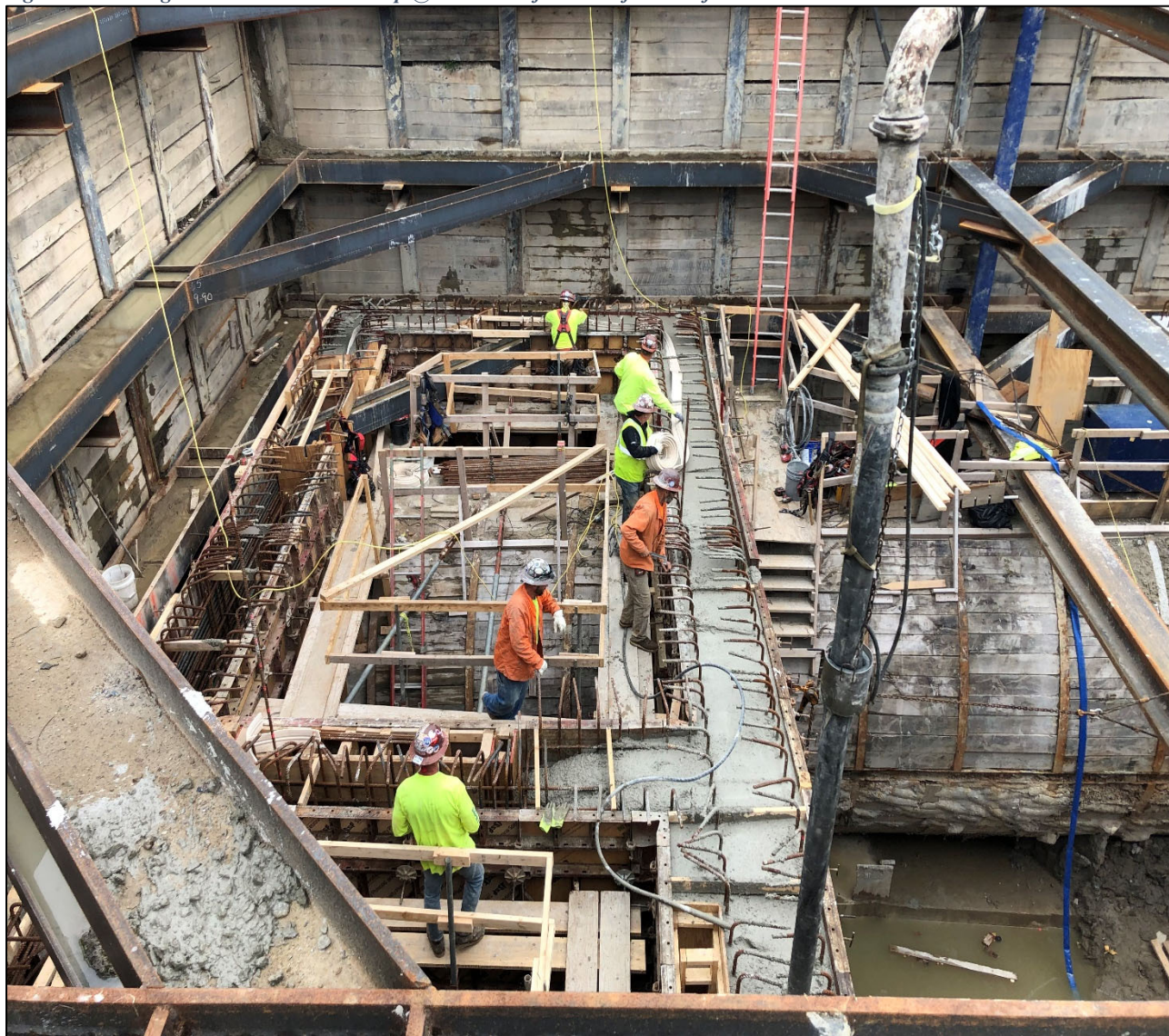
Figure 6 – Placing Concrete Walls via Pump @ East End of Beaconsfield Shaft
