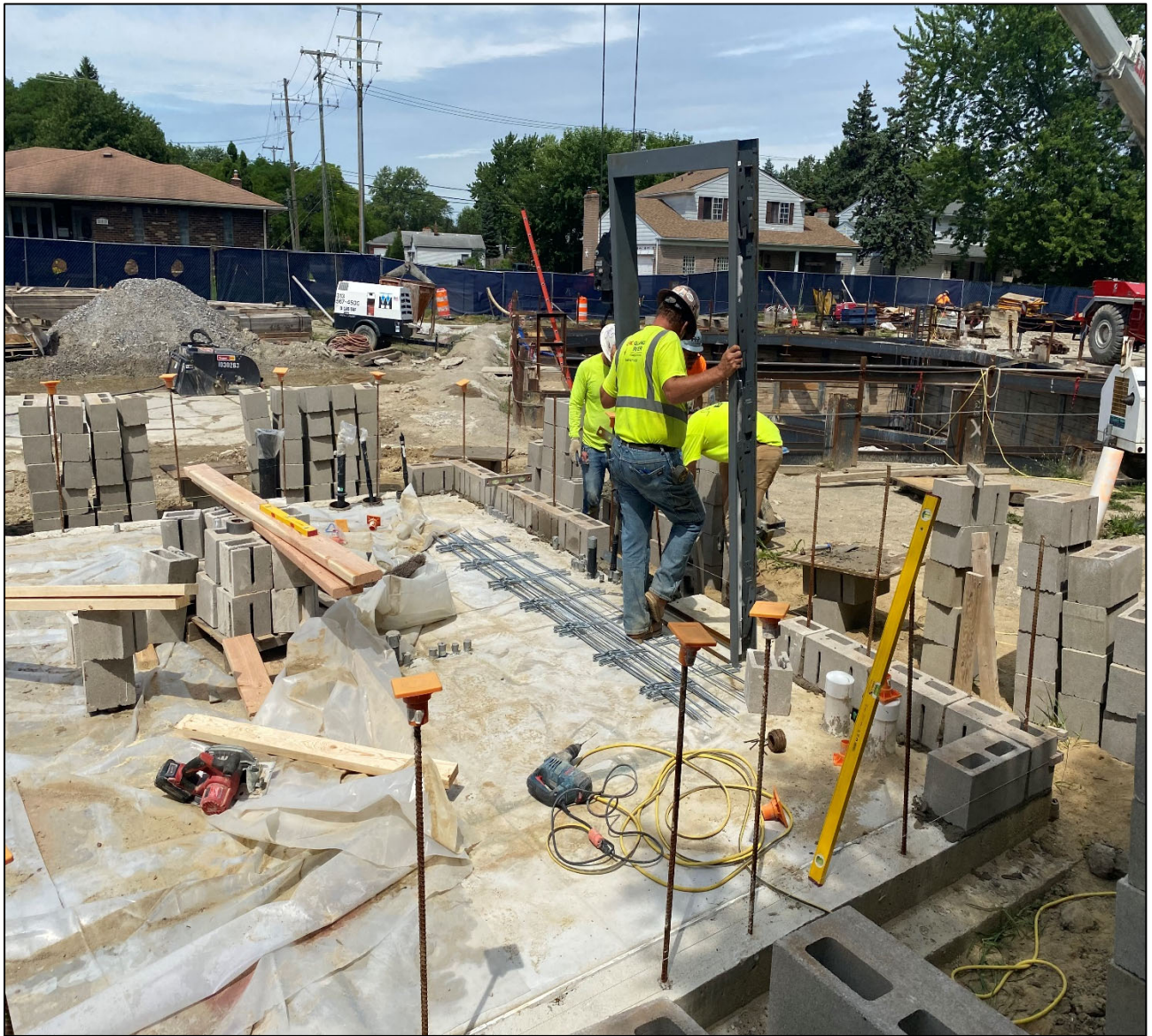
Figure 7 – Installing Door Jambs @ Beaconsfield Control Bldg.
