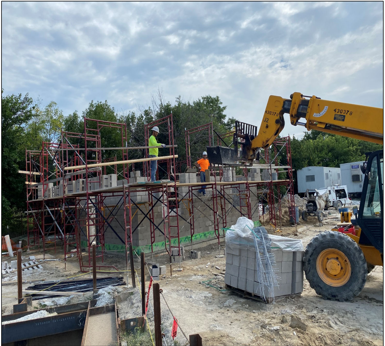
Figure 8 – Installing Concrete Masonry Blocks @ Beaconsfield Control Bldg.
