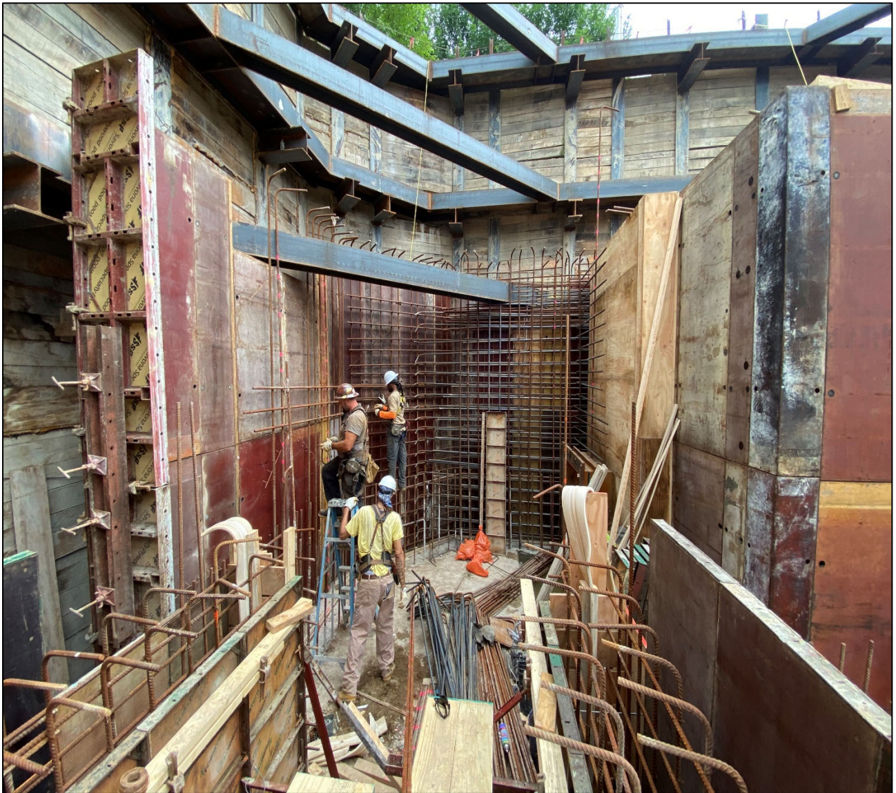
Figure 4 – Installing Reinforcing Steel @ East Wall of Beaconsfield Shaft
