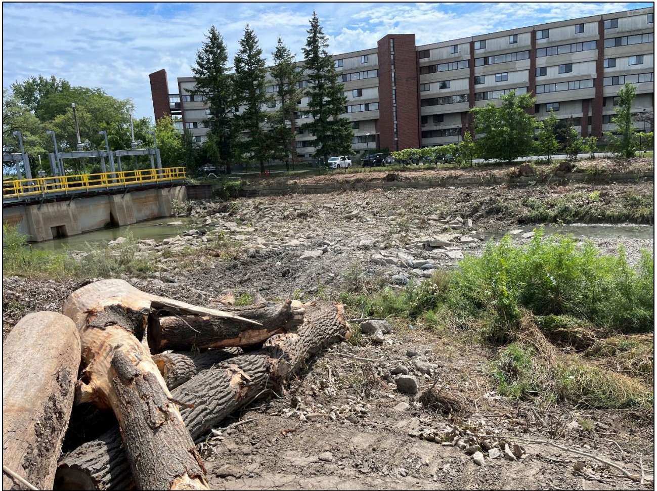
Figure 9 – South Side Tree Clearing
