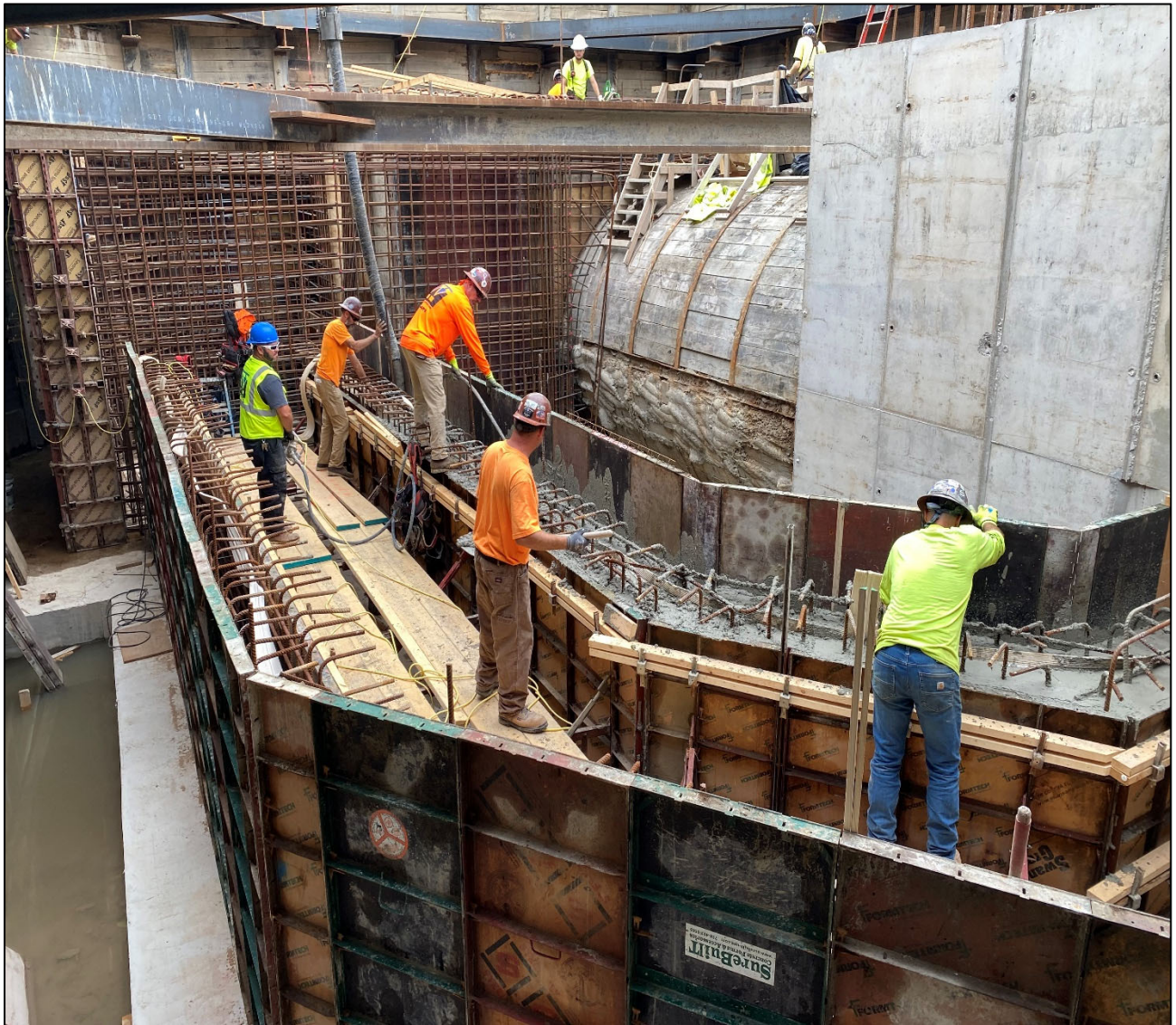
Figure 2 – Placing Concrete Walls for Tunnel Bypass @ Beaconsfield Shaft
