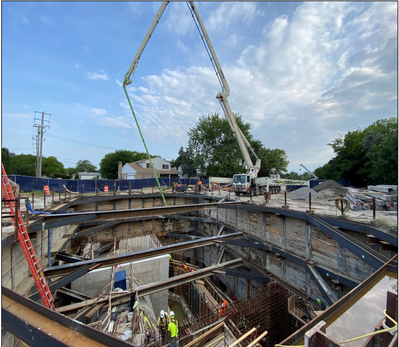
Figure 1 – Placing Concrete for Tunnel Bypass Walls via Pump @ Beaconsfield Shaft
