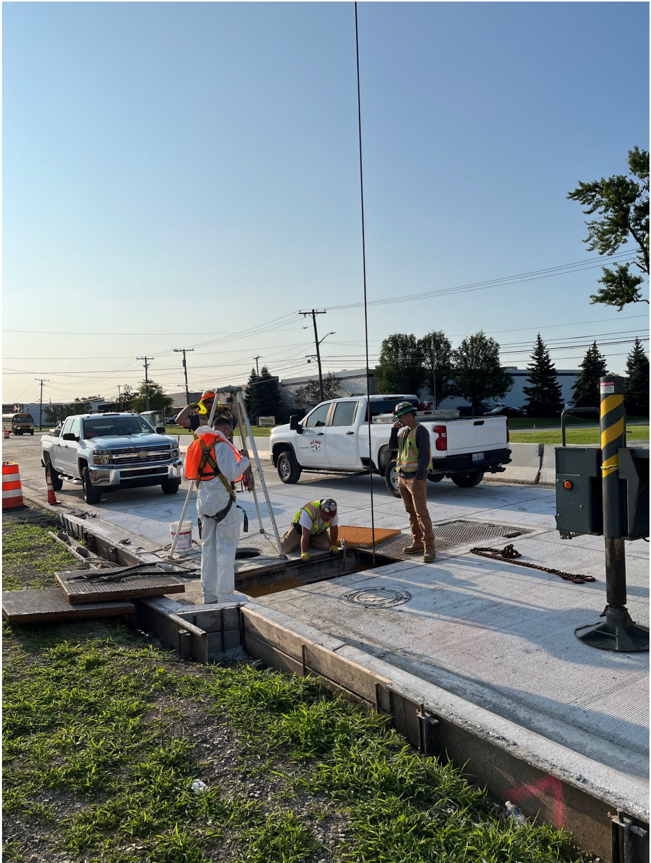
Figure 11 – Re-installation of the Hydraulic Cylinder at CS-13
