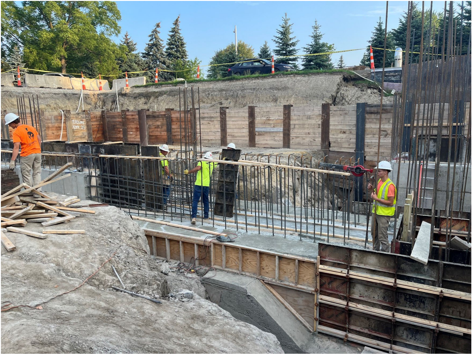
Figure 18 – Formwork Installation for Foundation Wall at Fraser Site
