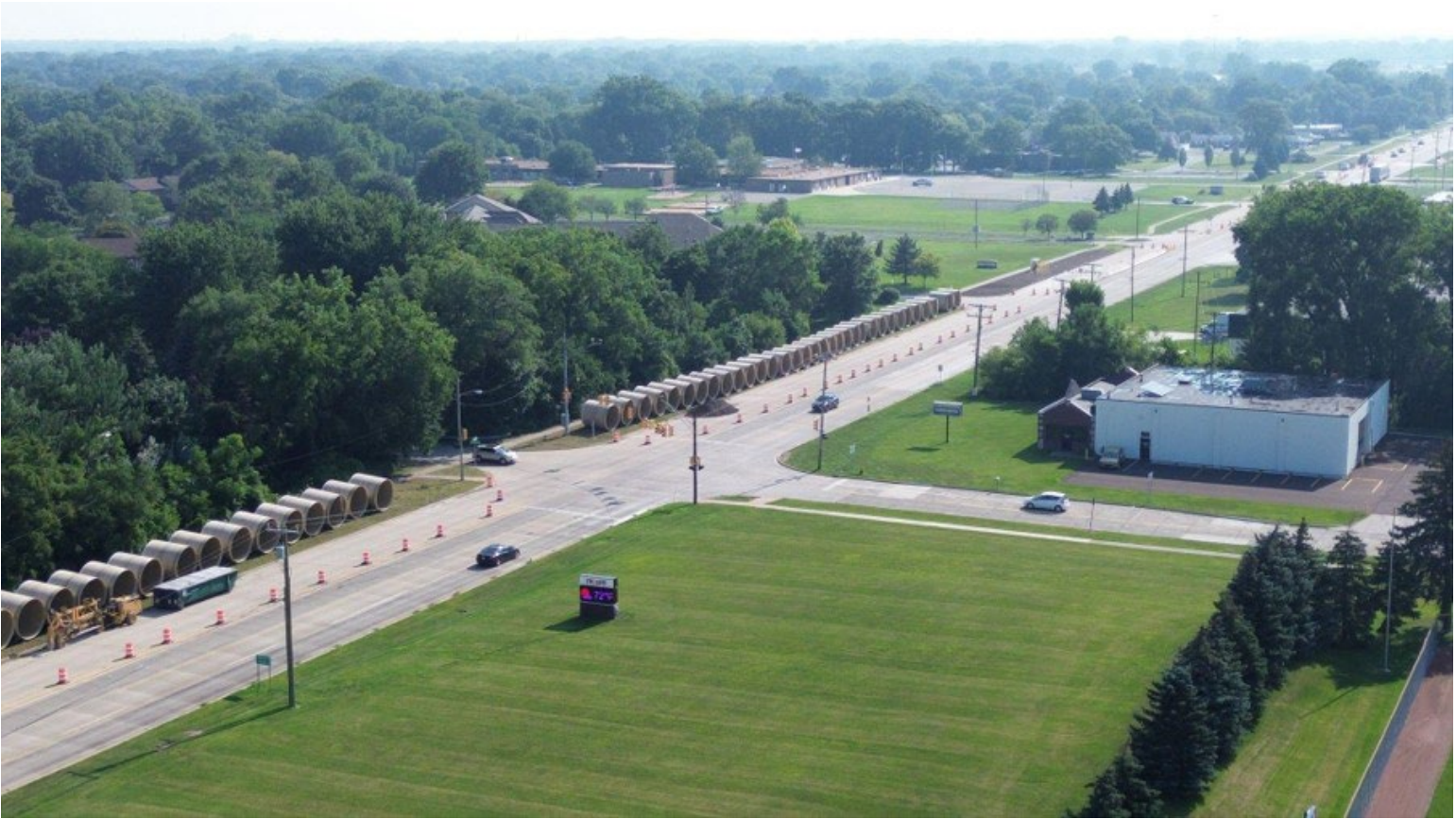
Figure 12 – Drone View of HOBAS along 15 Mile Road
