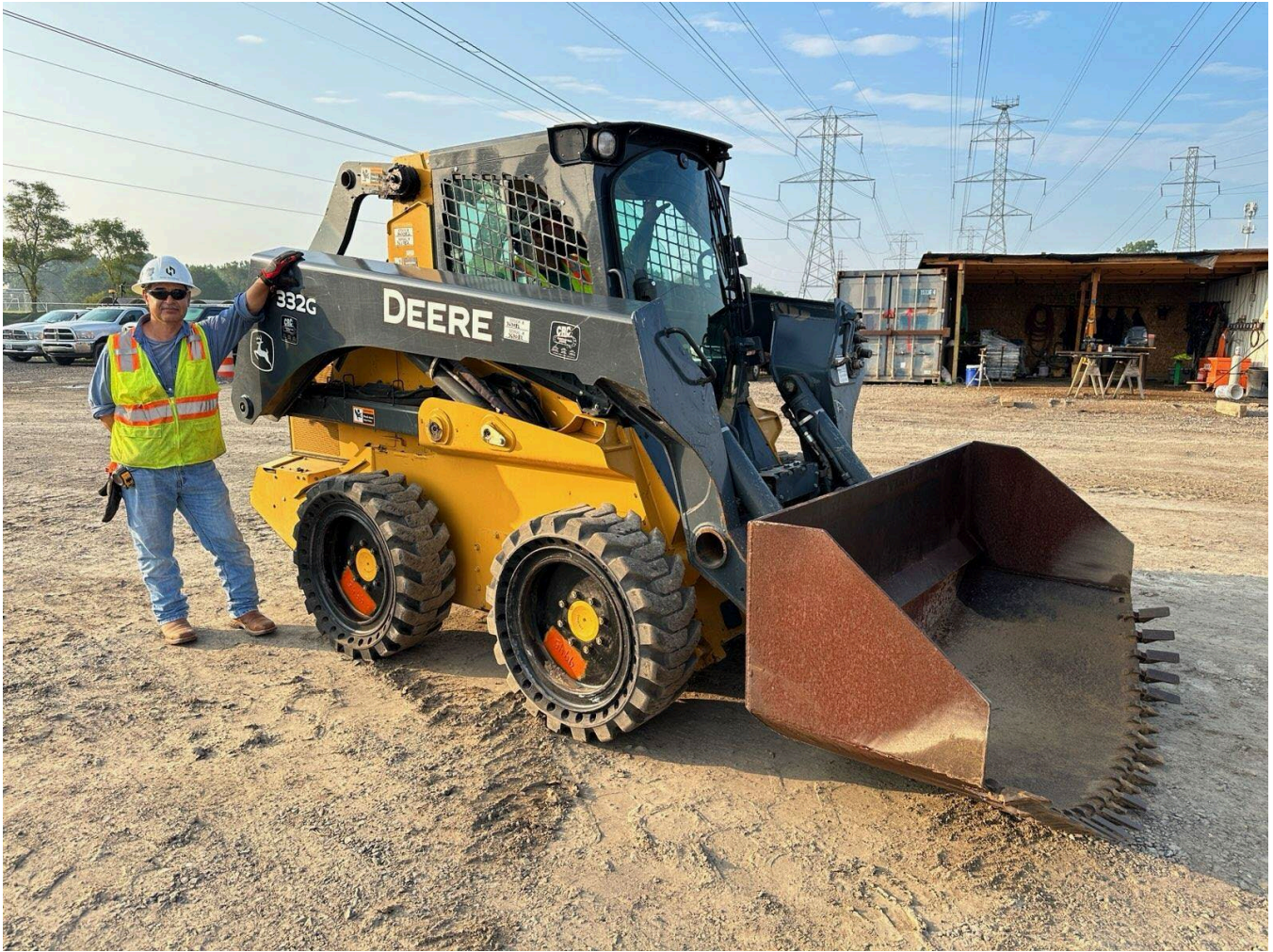
Figure 1 – Debris/Sediment Removal – Modified Skid-Steer
