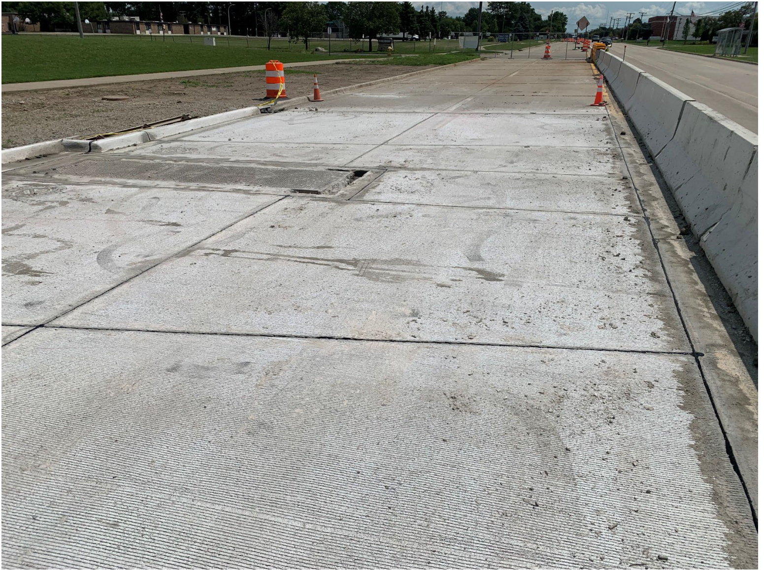
Figure 10 – 15 Mile Road Pavement Restoration at CS-13
