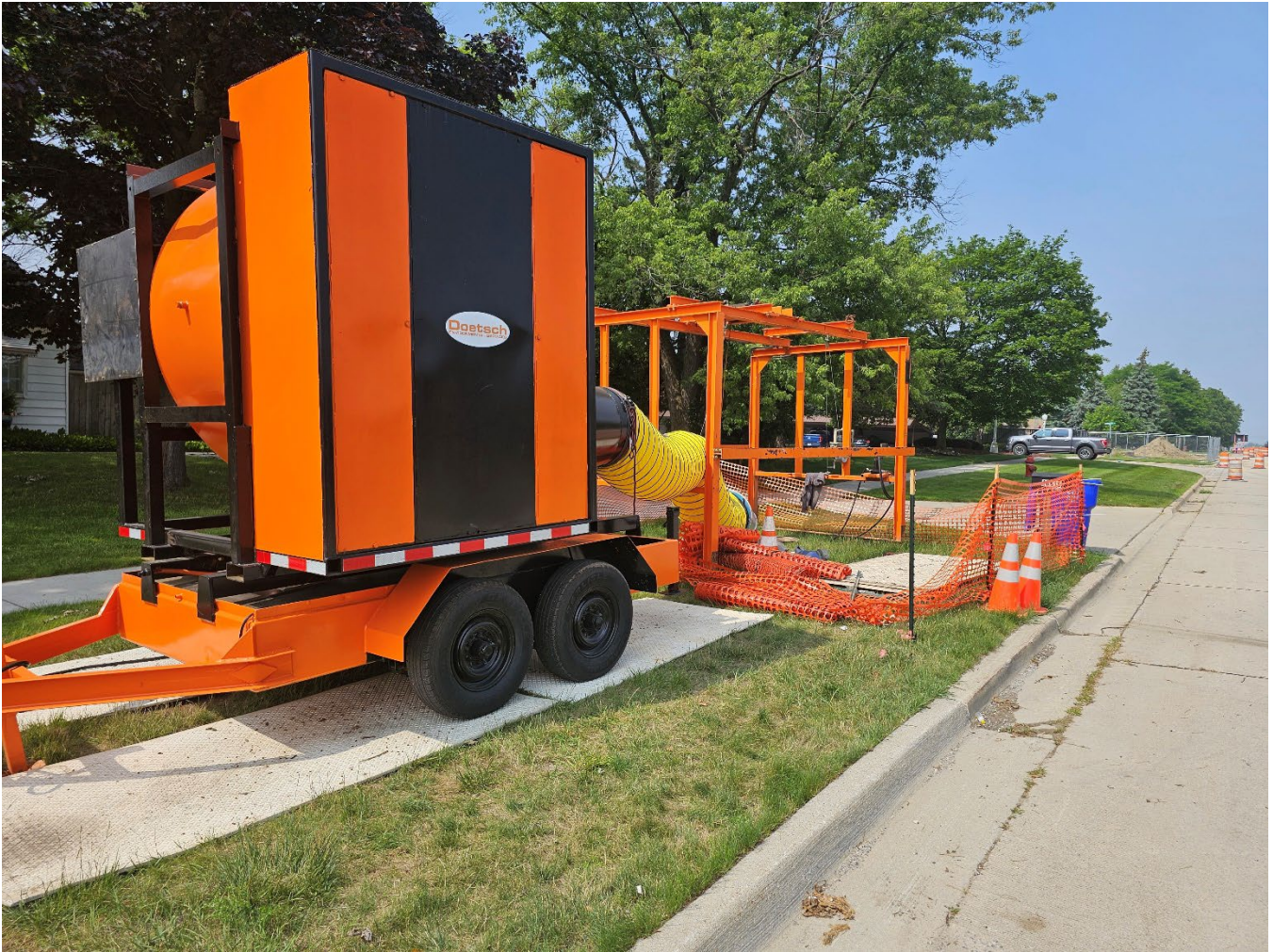
Figure 9 – Sediment/Debris Removal Ventilation Equipment at RAI-MH-10
