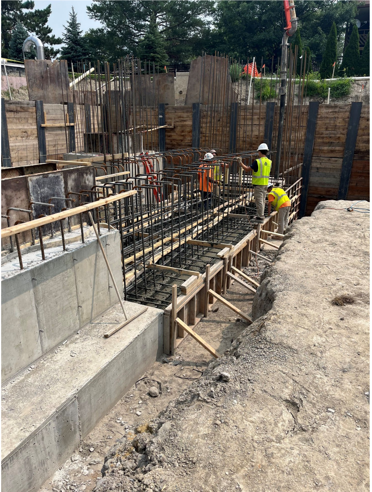
Figure 17 – Foundation Wall Rebar Installation at Fraser Site
