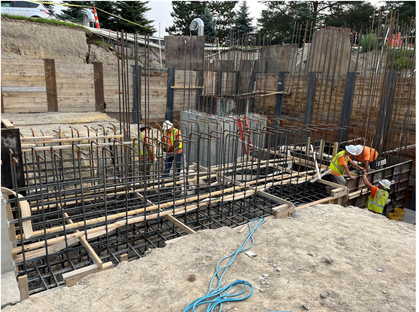
Figure 16 – Foundation Wall Rebar Installation at Fraser Site
