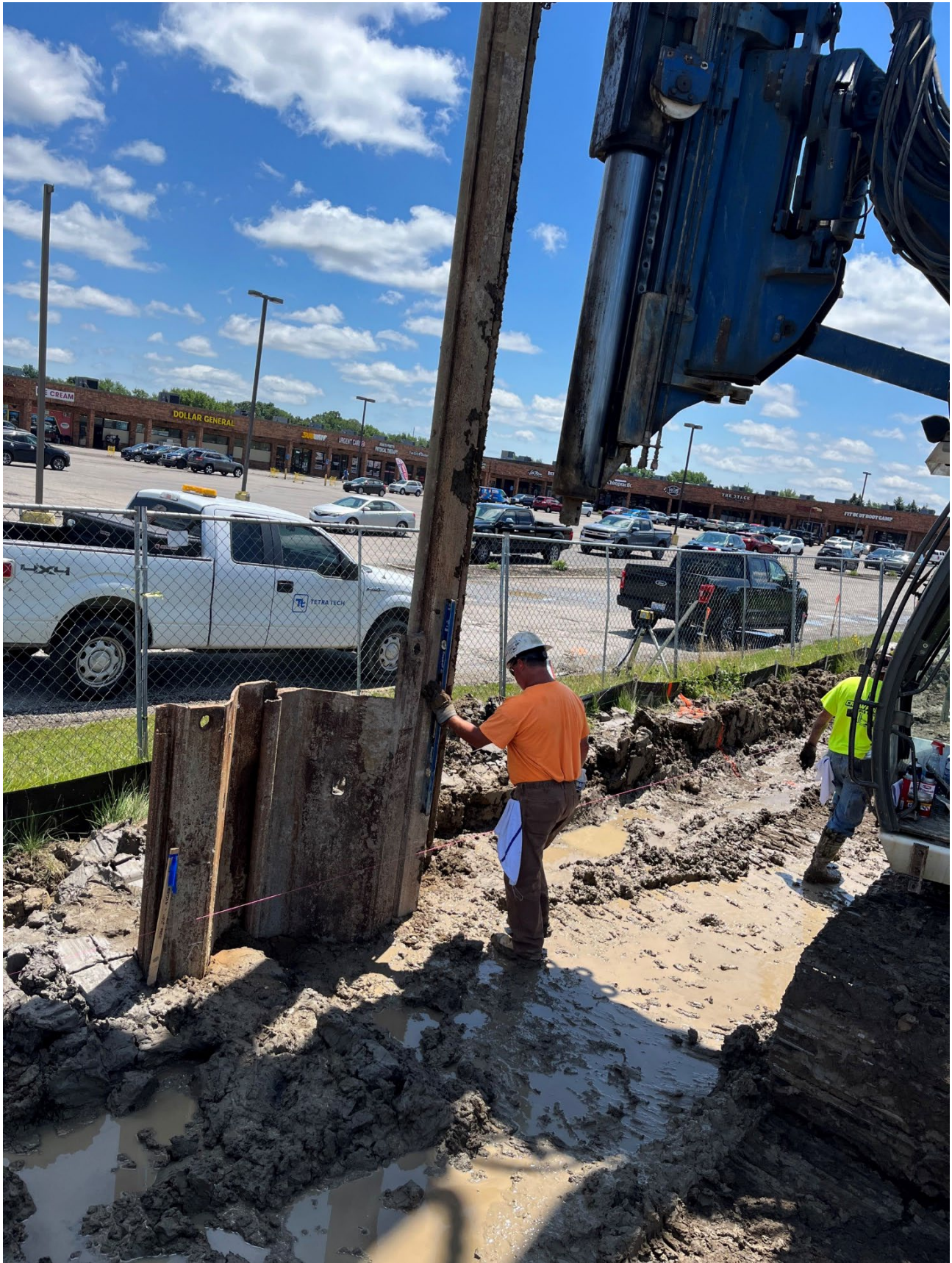
Figure 20 – Sheet piling Installation at 21 Mile & Garfield
