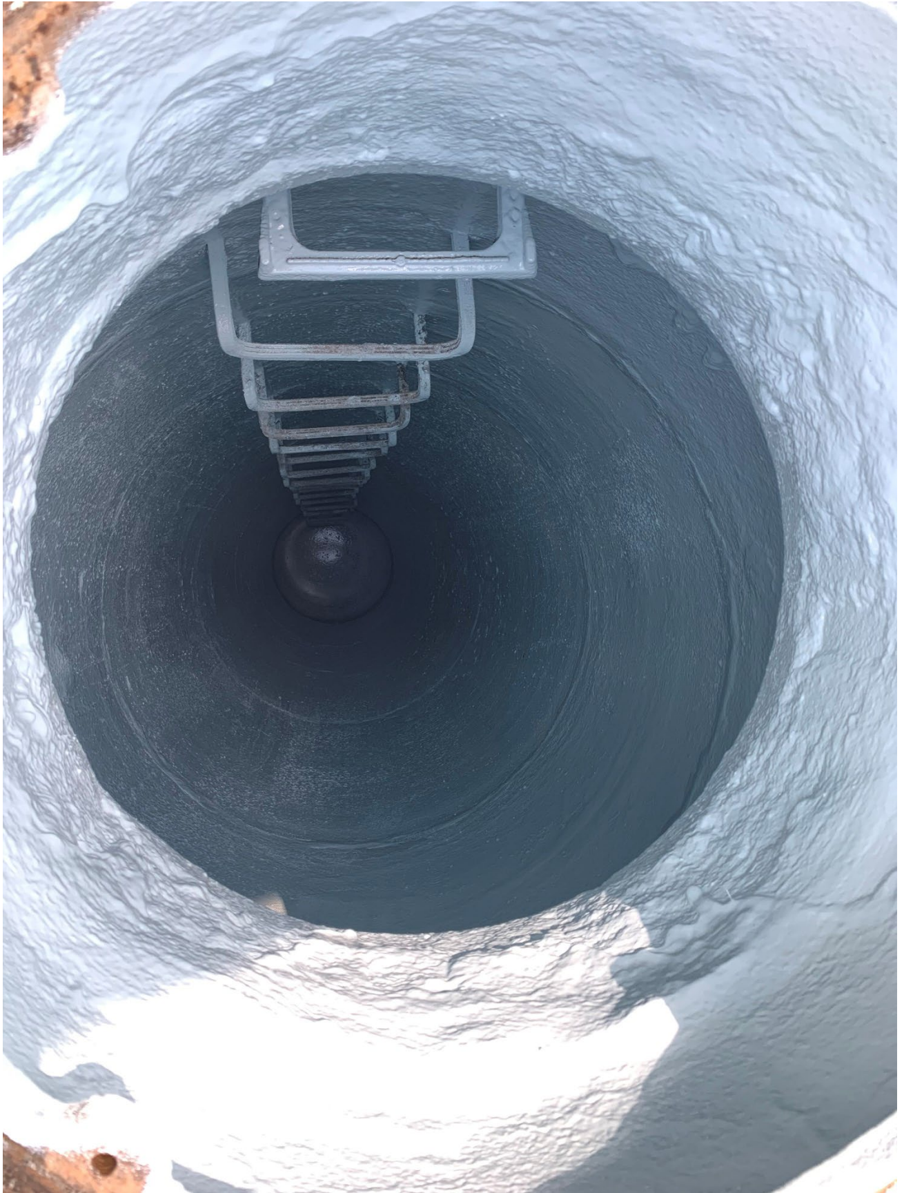
Figure 14 – 15 Mile Interceptor MH-04 – Post Epoxy Coating
