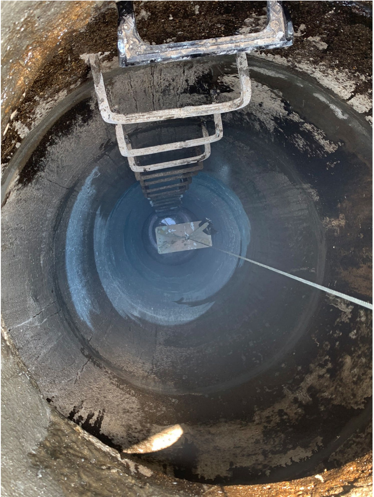
Figure 13 – 15 Mile Interceptor MH-04 – During Epoxy Coating
