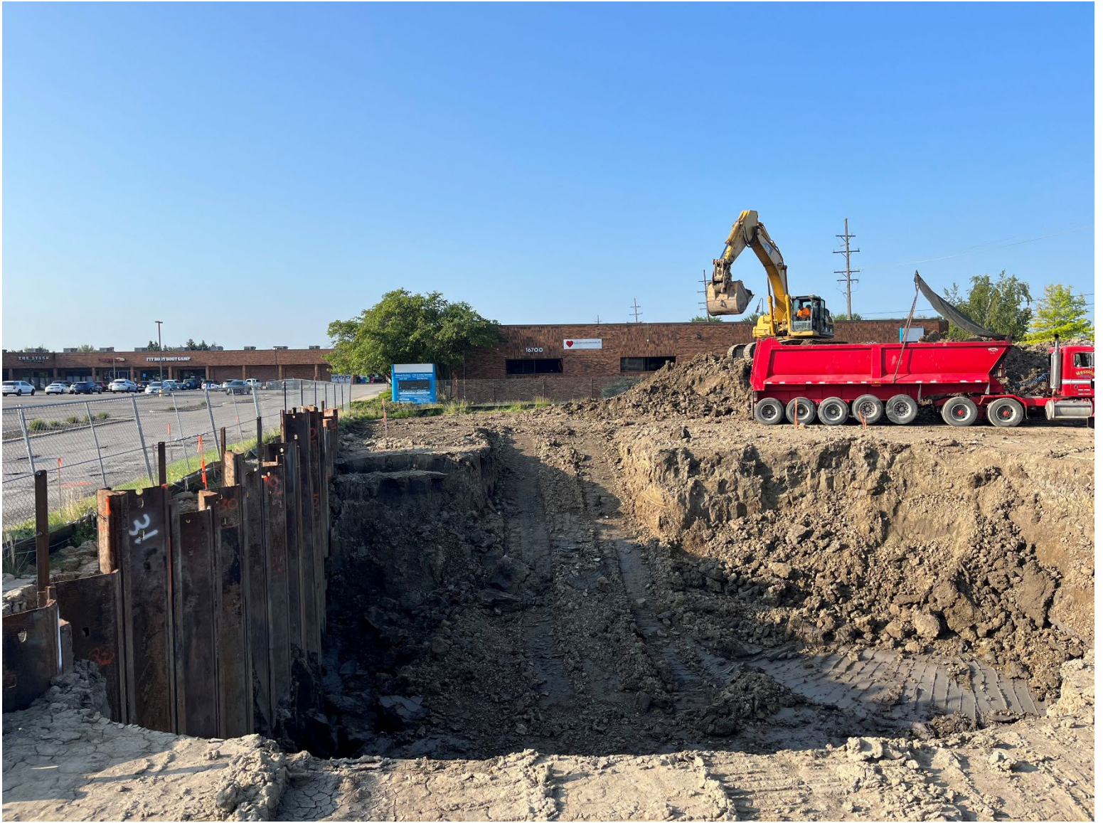
Figure 19 – Excavation & Sheet piling at 21 Mile & Garfield
