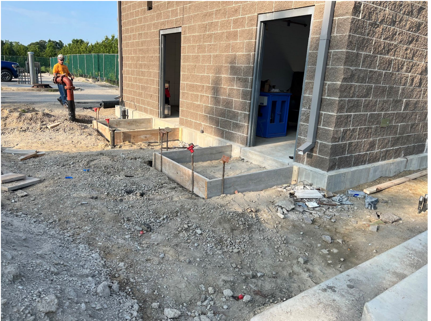
Figure 15 – NGI PS Odor & Corrosion Equipment Building – Prep for Concrete Stoops
