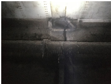
Figure 4 – Concrete ceiling repair
