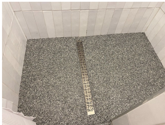
Figure 3 – Repaired epoxy floor in shower
