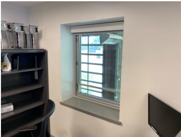
Figure 1 – New window in SCADA Control Room
