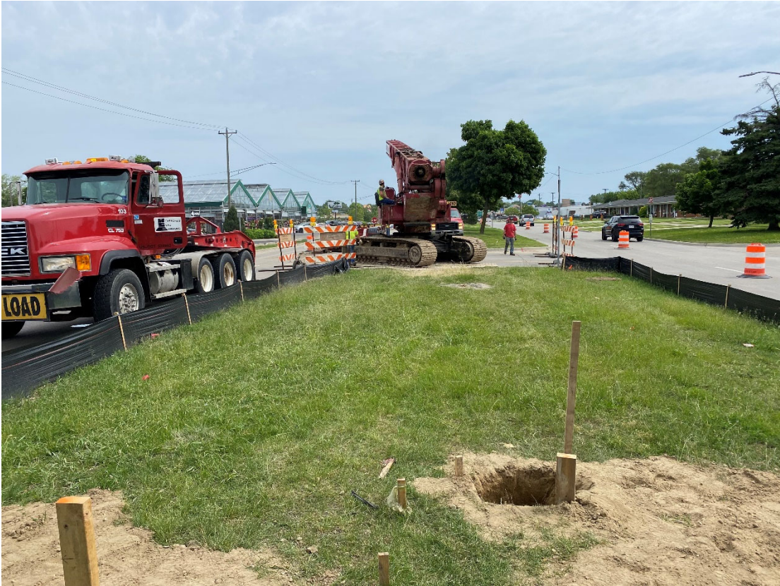
Photo of mobilizing drilling equipment at Kelly and Oak.
