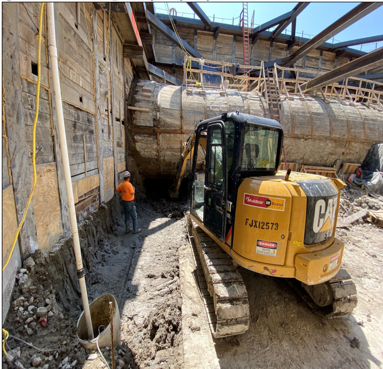
Figure 5 – Excavation under Tunnel @ East wall of Beaconsfield Shaft
