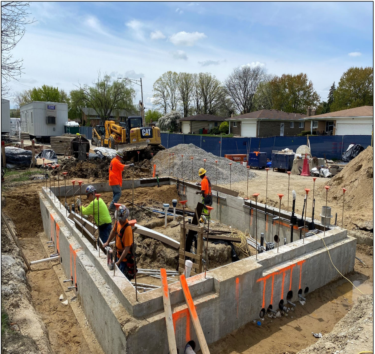
Figure 1 – Control Bldg. below Floor Electrical & Mechanical @ Beaconsfield
