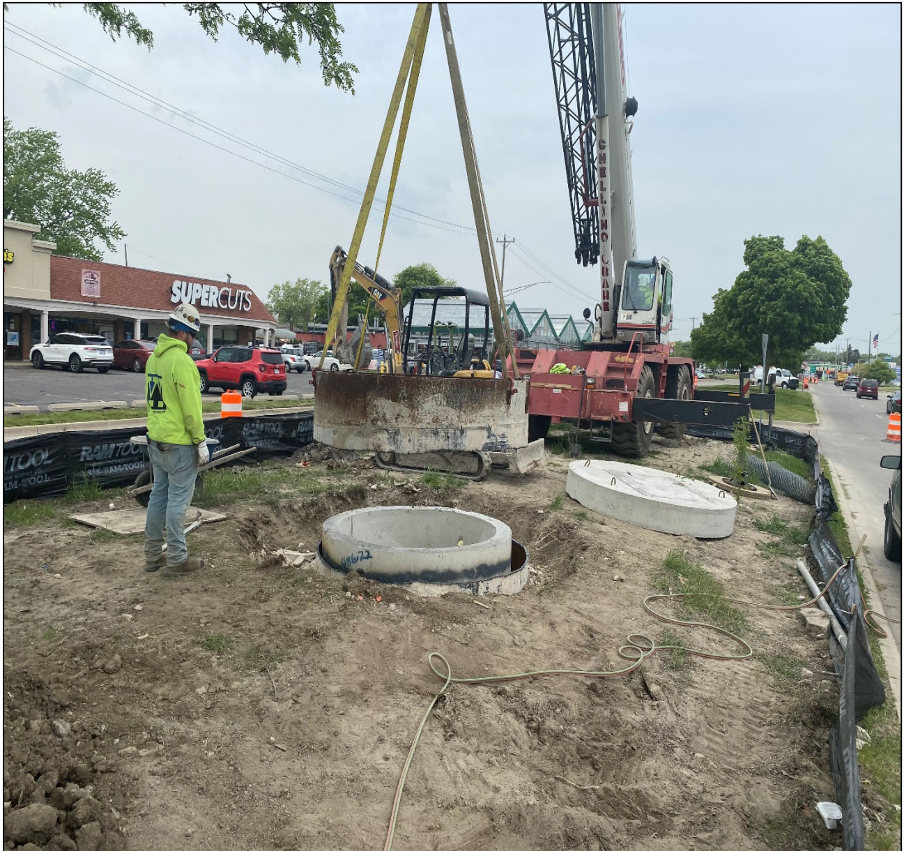
Figure 4 – Installing Access Structure @ Kelly Rd.
