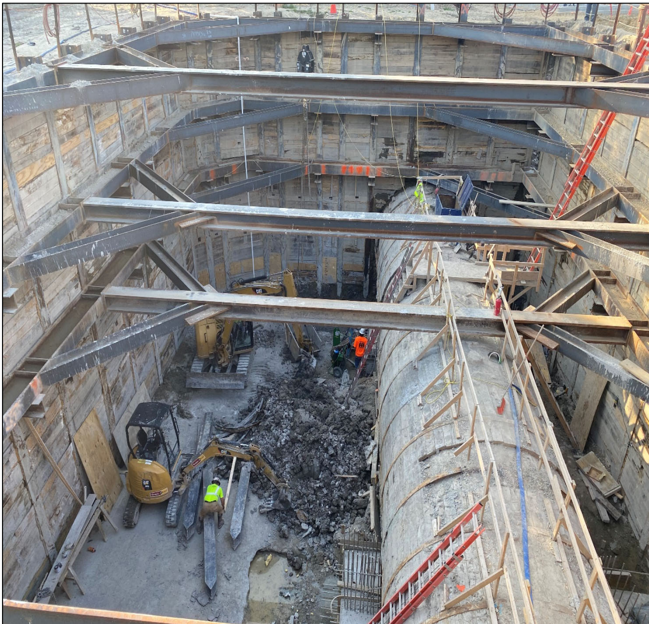
Figure 8 – 11FT Tunnel Facing East @ Beaconsfield Rd. Shaft
