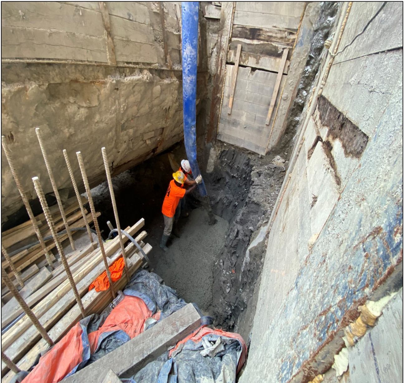
Figure 6 – Placing Concrete via Chute South side of Tunnel @ Beaconsfield
