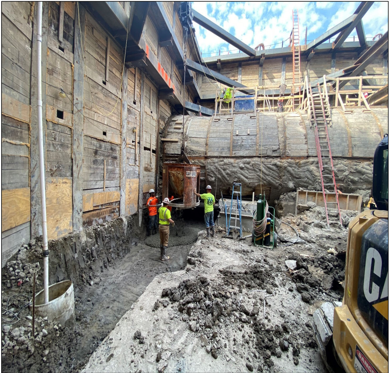
Figure 7 – Placing Concrete via Hopper at North side of Tunnel @ Beaconsfield
