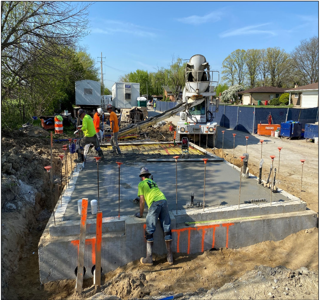
Figure 2 – Placing Concrete Control Bldg. floor @ Beaconsfield
