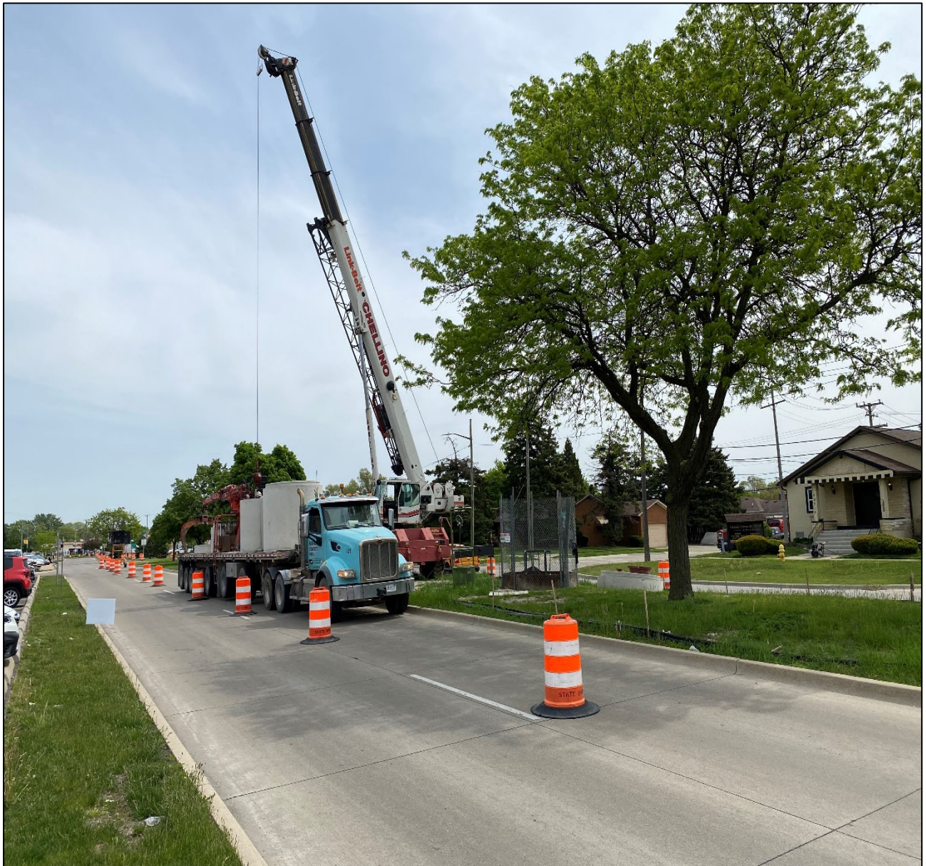
Figure 3 – Precast Access Structure Delivery @ Kelly Rd.
