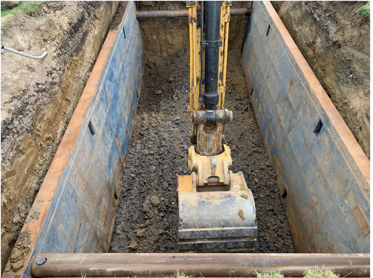
Figure 10 – FAD Bore Pit Excavation
