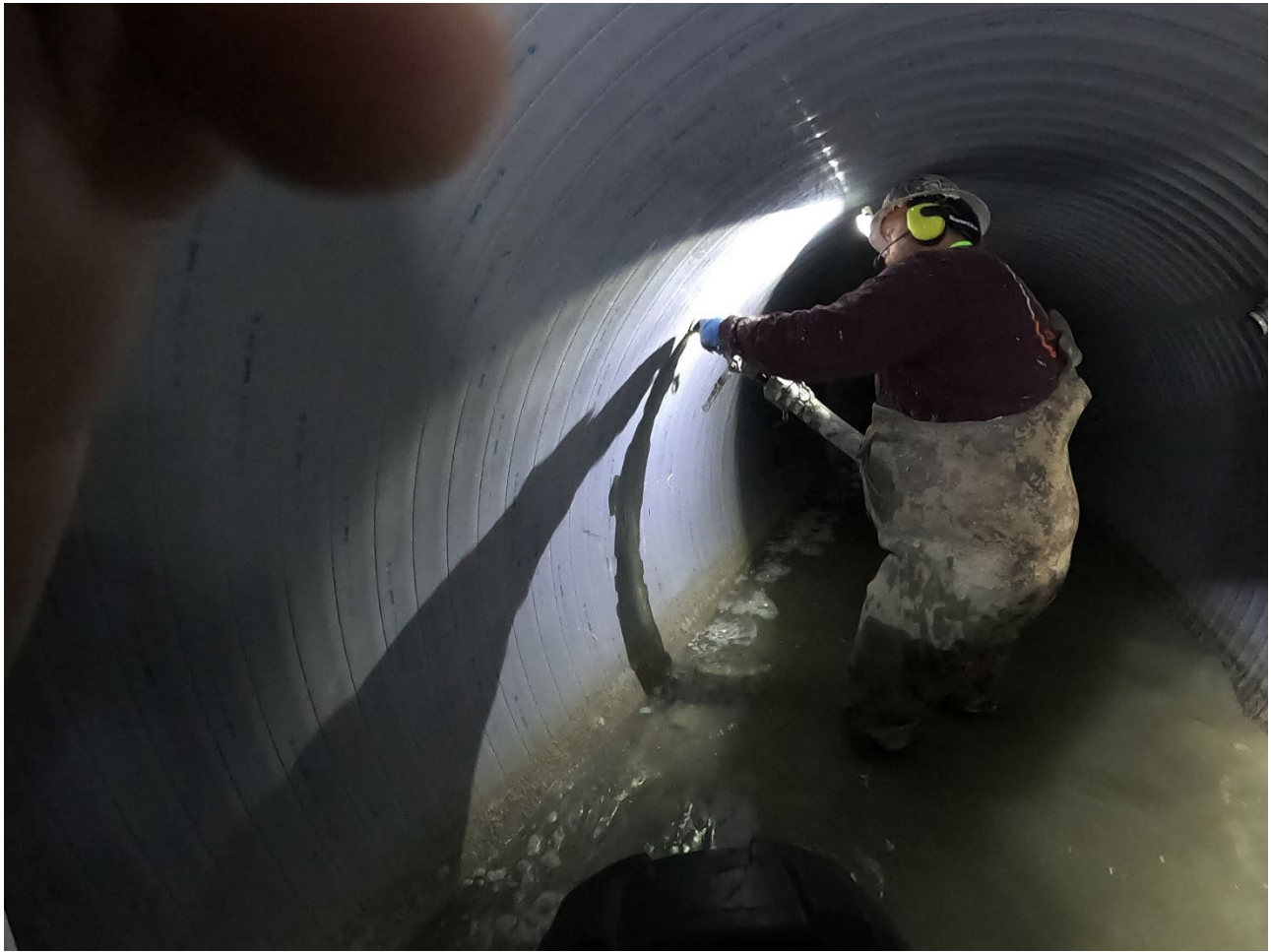
Figure 13 – Annular Grouting Operation through Grout Ports
