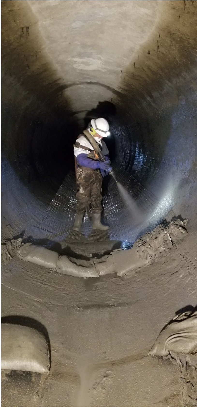
Figure 8 – Spray-Lining Invert of 8-foot Pipe
