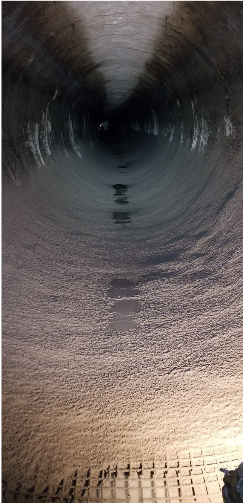
Figure 7 – Invert of 8-foot Pipe Post-Spray-Lining
