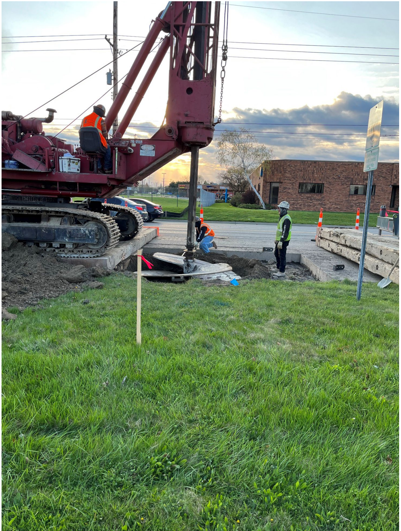
Figure 15 – 21 & Garfield – Drilling for 8-foot Caisson at Interceptor
