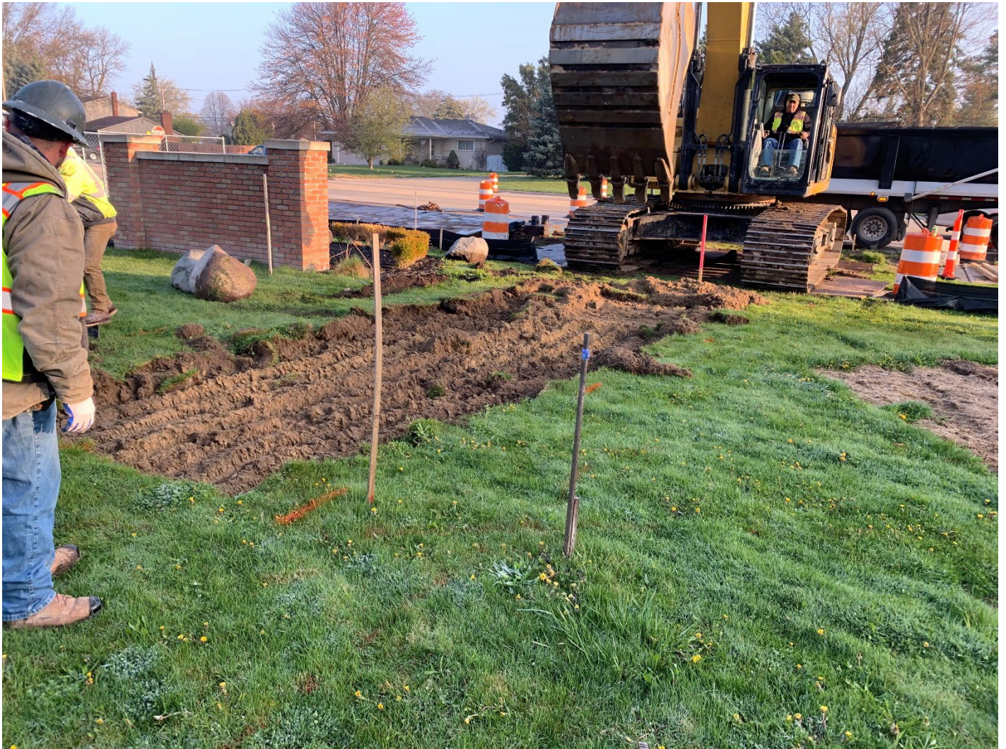
Figure 9 – FAD Bore Pit Excavation
