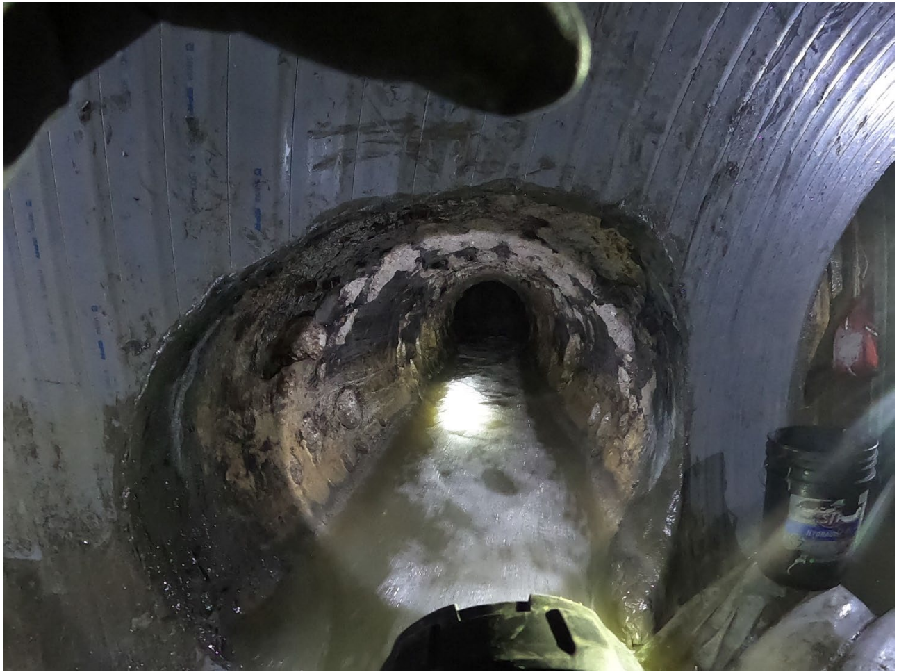
Figure 14 – Shelby Connection into Garfield Interceptor
