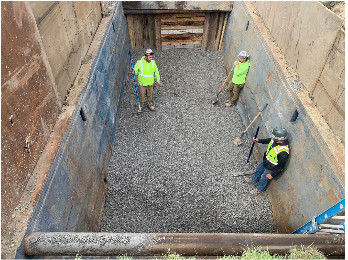
Figure 11 – FAD Bore Pit
