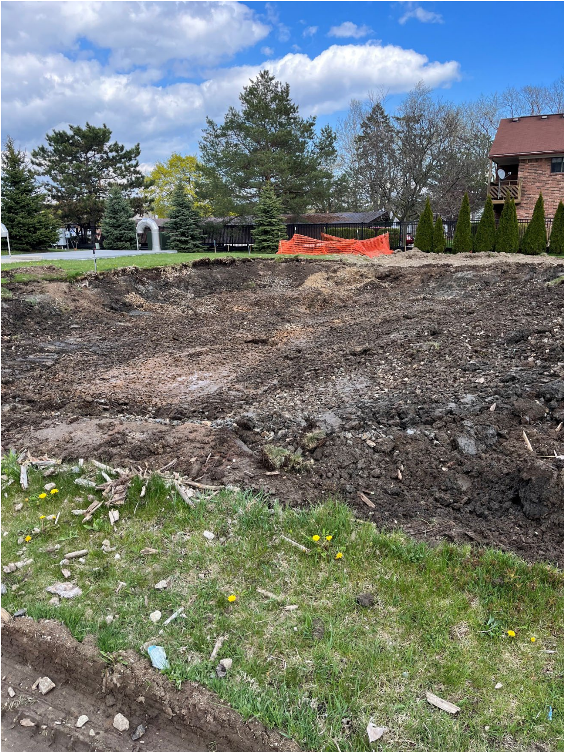
Figure 16 – Fraser – Bio-Filter Demolition
