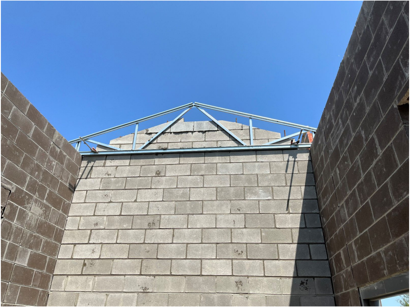
Figure 14 – NGI Building - Steel Truss Installation
