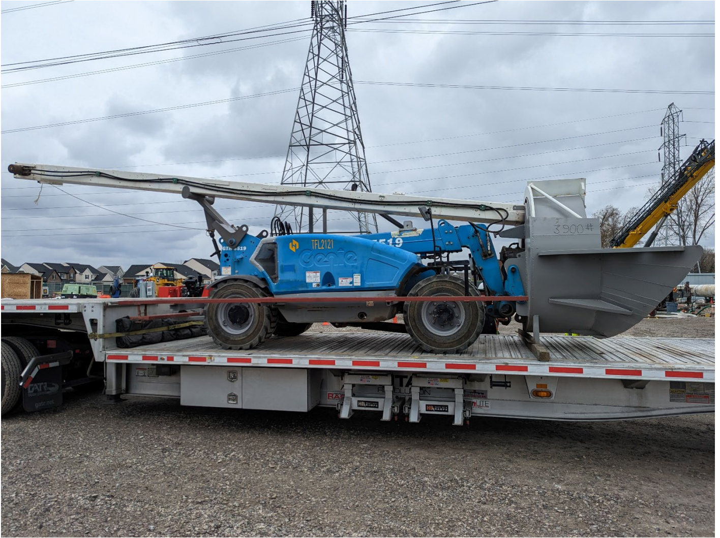
Figure 4 – Debris/Sediment Removal Equipment
