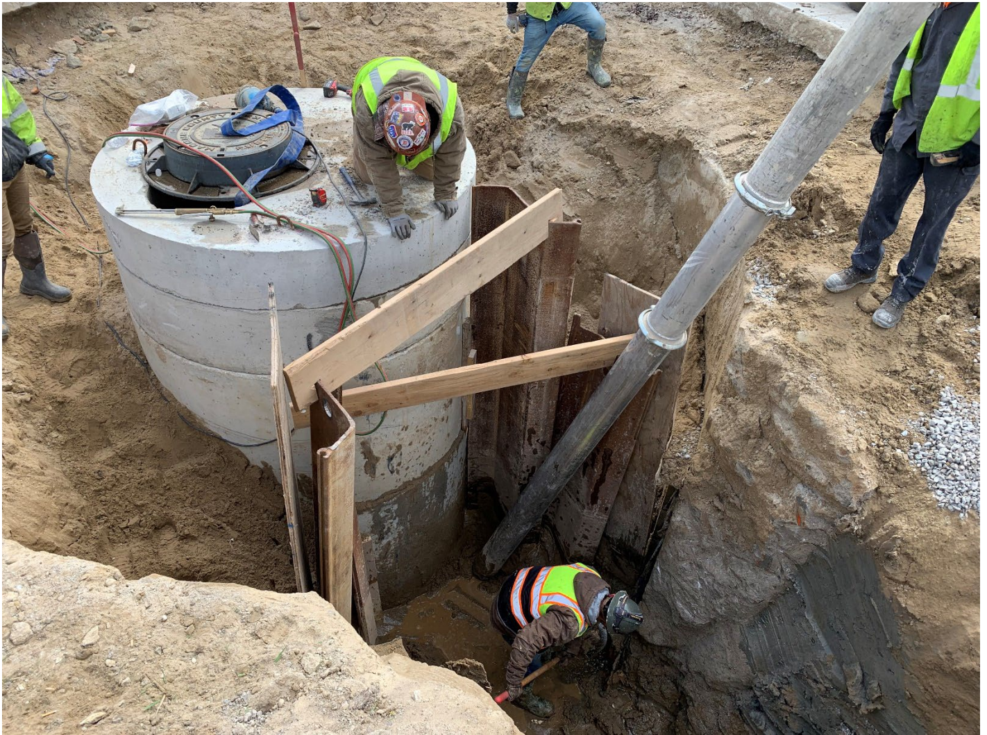
Figure 12 – FAD Excavation at MH-01
