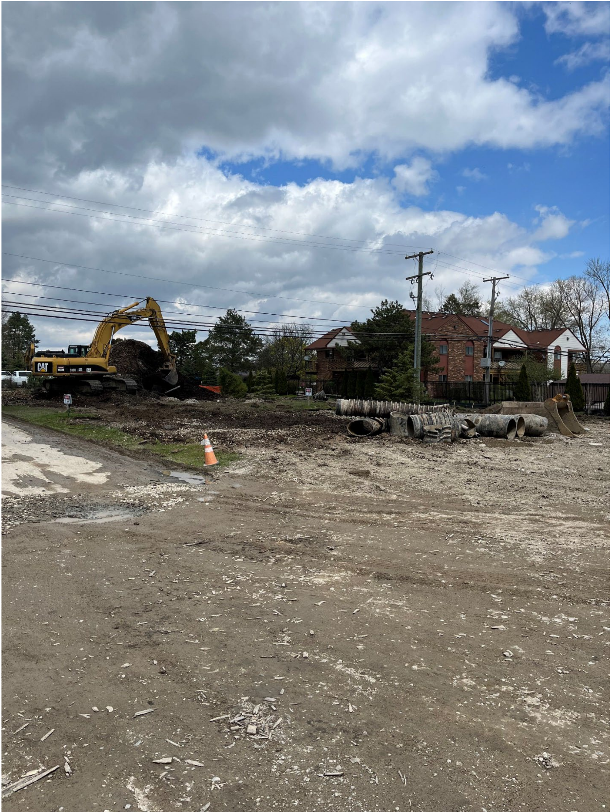
Figure 17 – Fraser Bio-Filter Demolition
