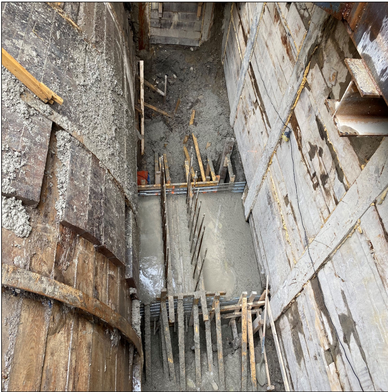
Figure 6 – New Concrete Foundation – South Side of Tunnel
