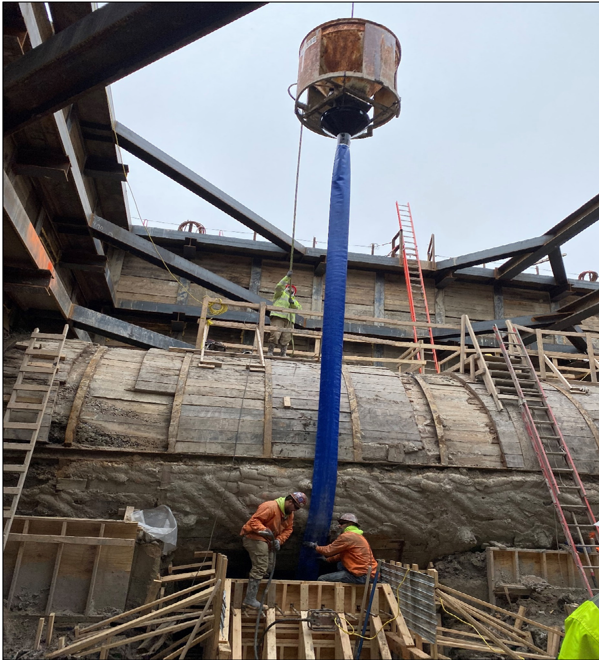
Figure 5 – Placing New Tunnel Foundation Concrete via Hopper
