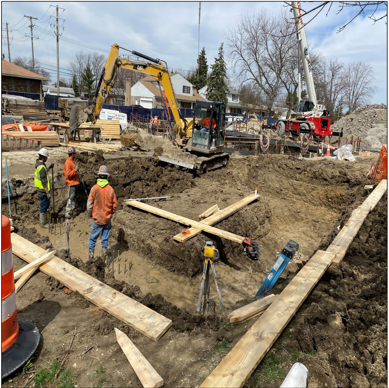
Figure 1 – Control Bldg. Foundation Excavation @ Beaconsfield
