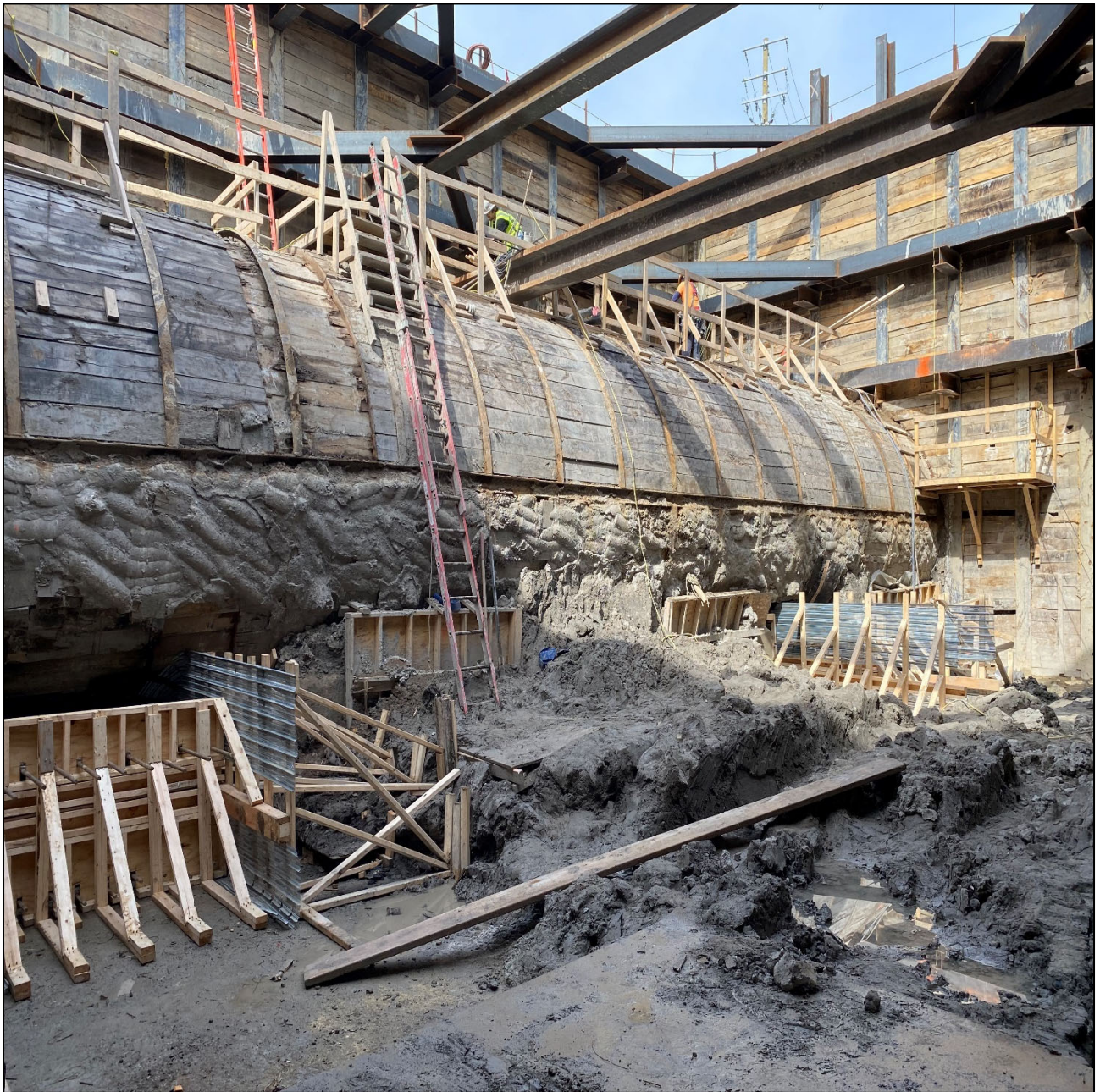
Figure 7 – Foundation Concrete Forms - North side of Tunnel
