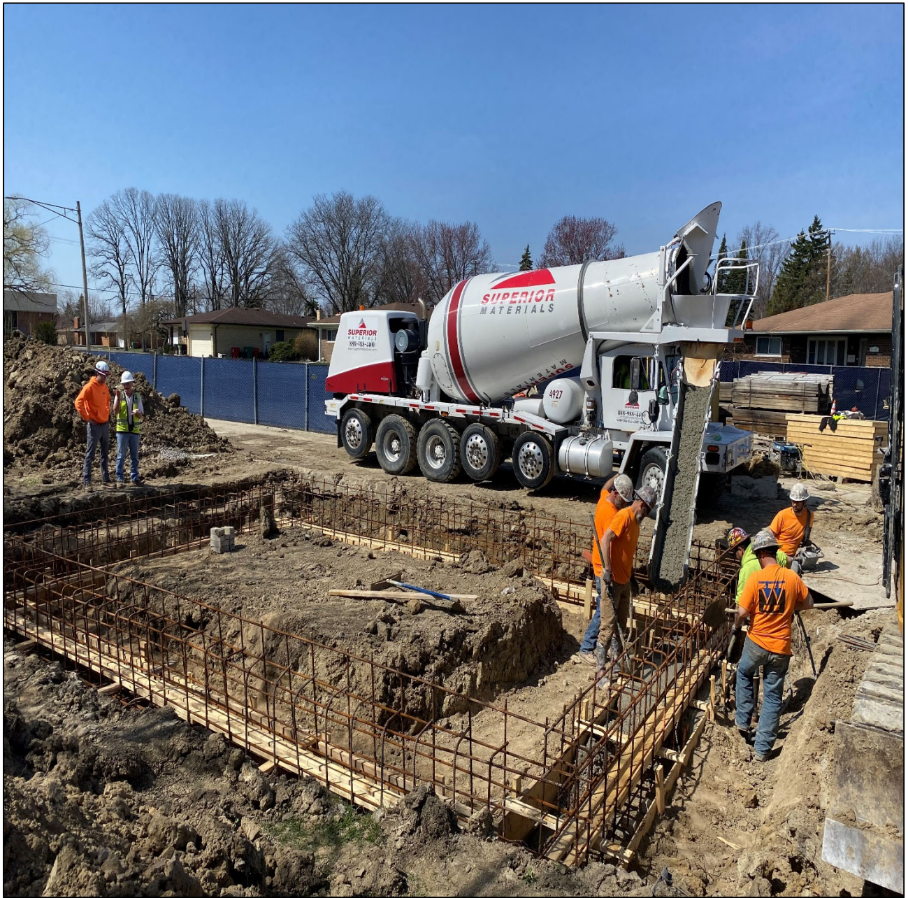
Figure 2 – Control Bldg. Concrete Spread Footing
