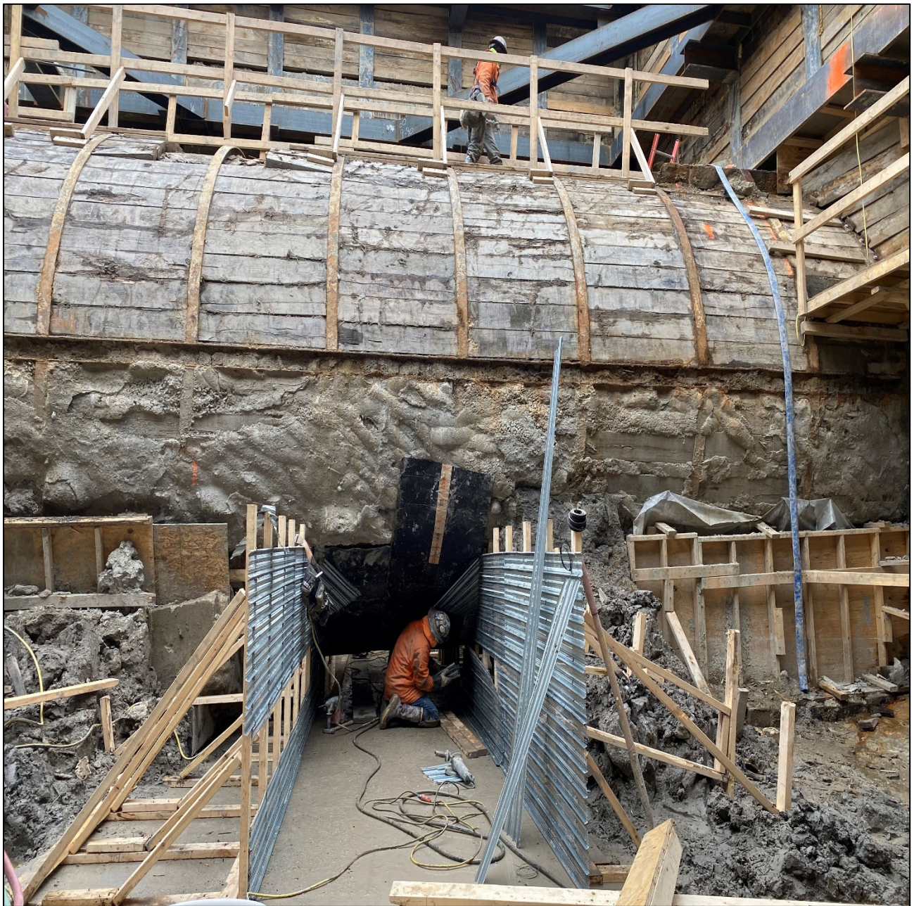
Figure 4 – Laying Out for New Concrete Support Foundations
