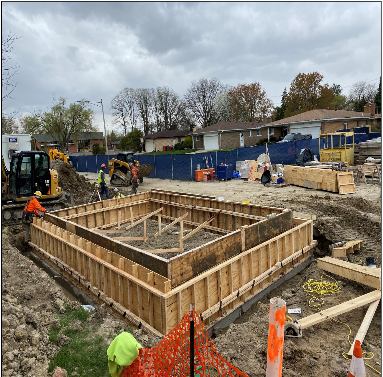
Figure 3 – Control Bldg. Foundation Walls
