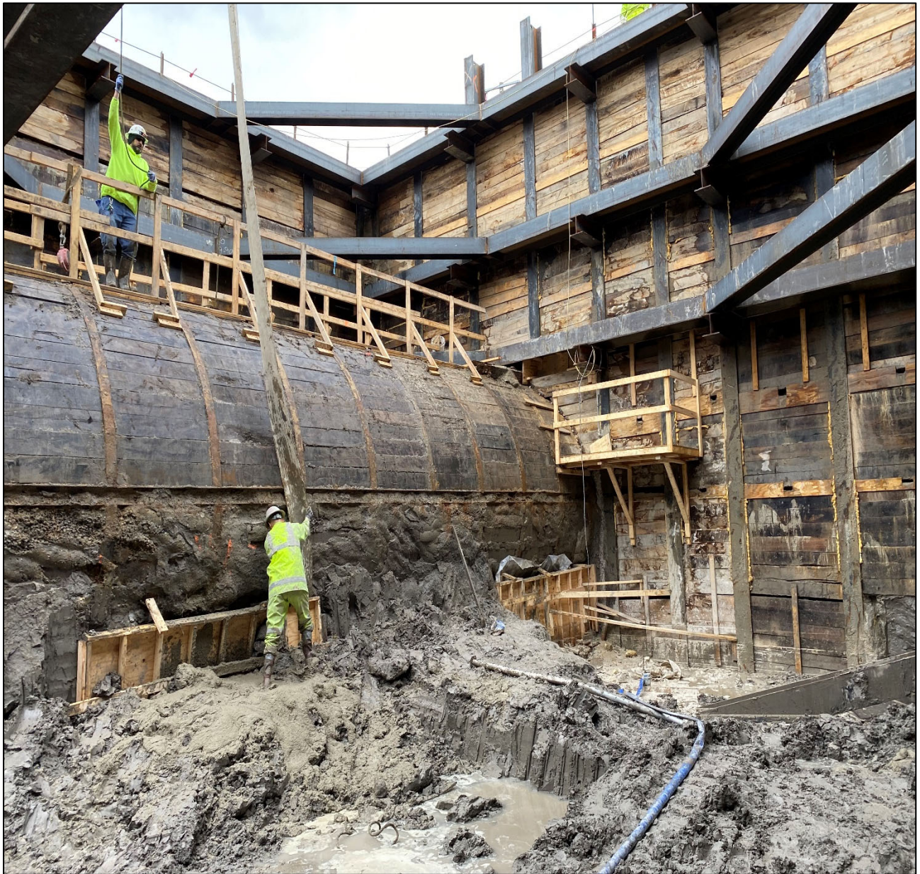
Figure 7 – Placing Flow Fill via Chute
