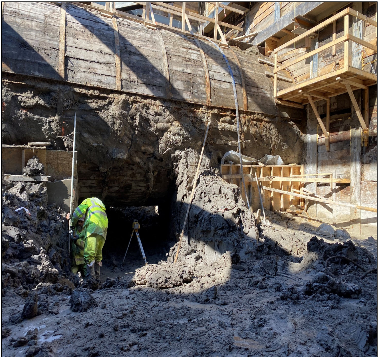
Figure 4 – Laying Out for New Concrete Support
