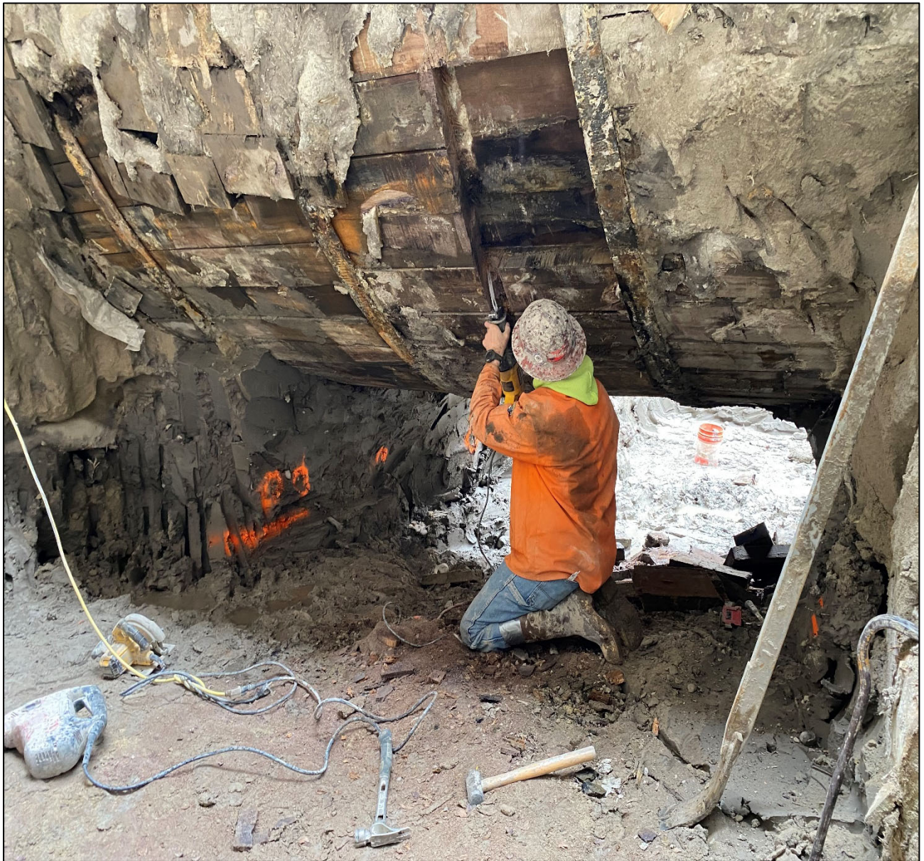
Figure 3 – Removing Existing Timber Forms
