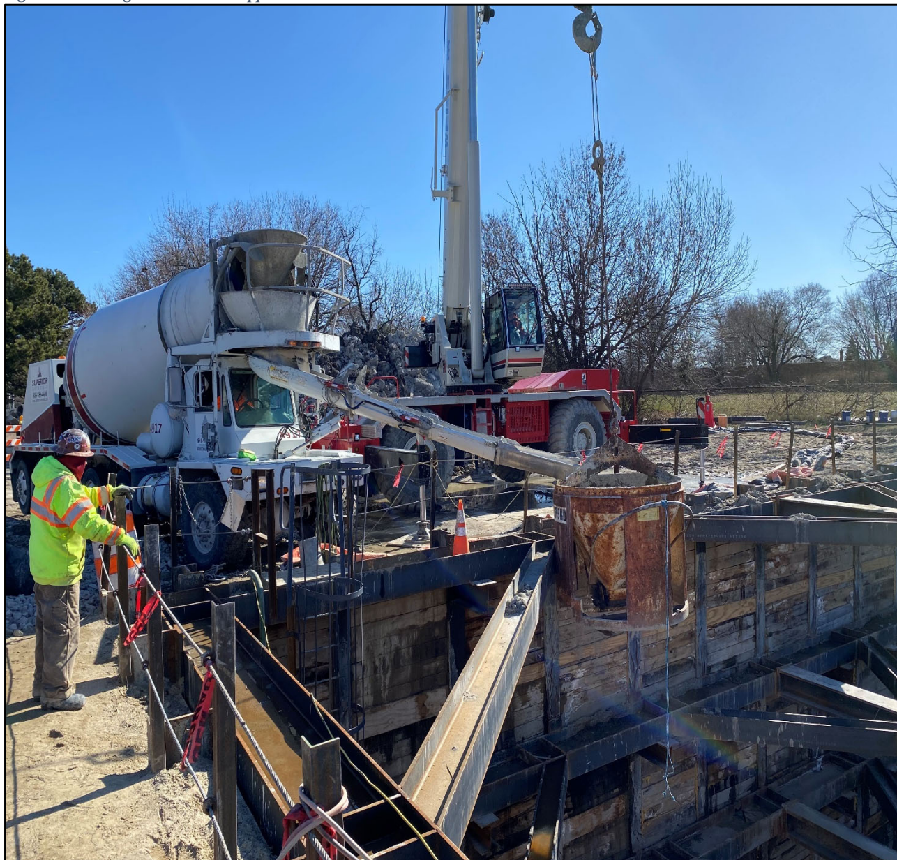
Figure 5 – Placing Concrete via Hopper
