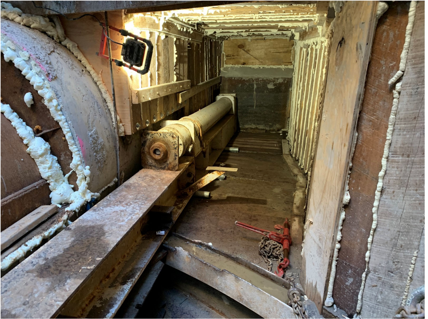
Figure 9 – Lining Completion Shaft – Tail-Tunnel w/ Hydraulic Jack
