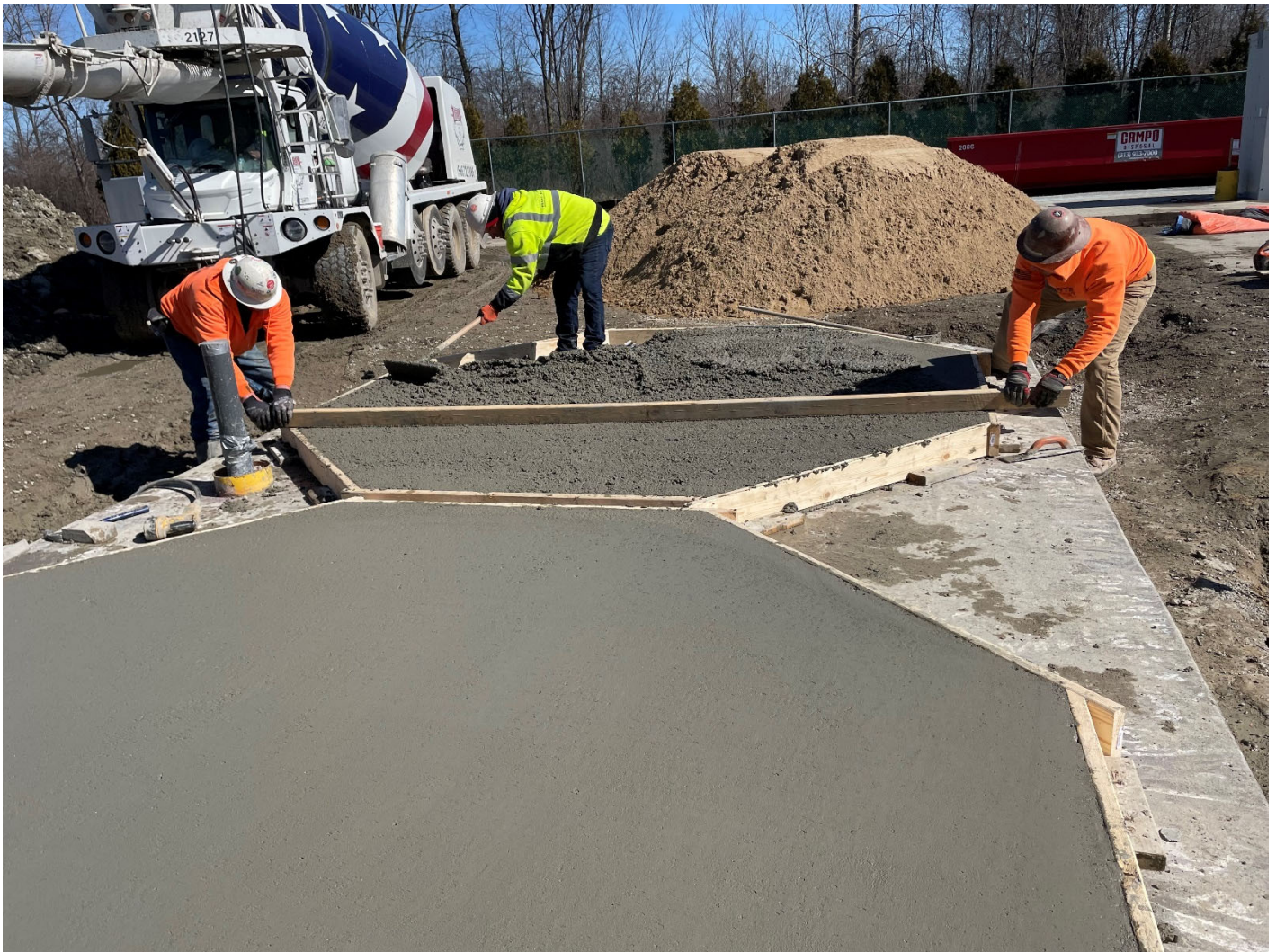
Figure 17 – Concrete Placement for Tank Pads at NGI
