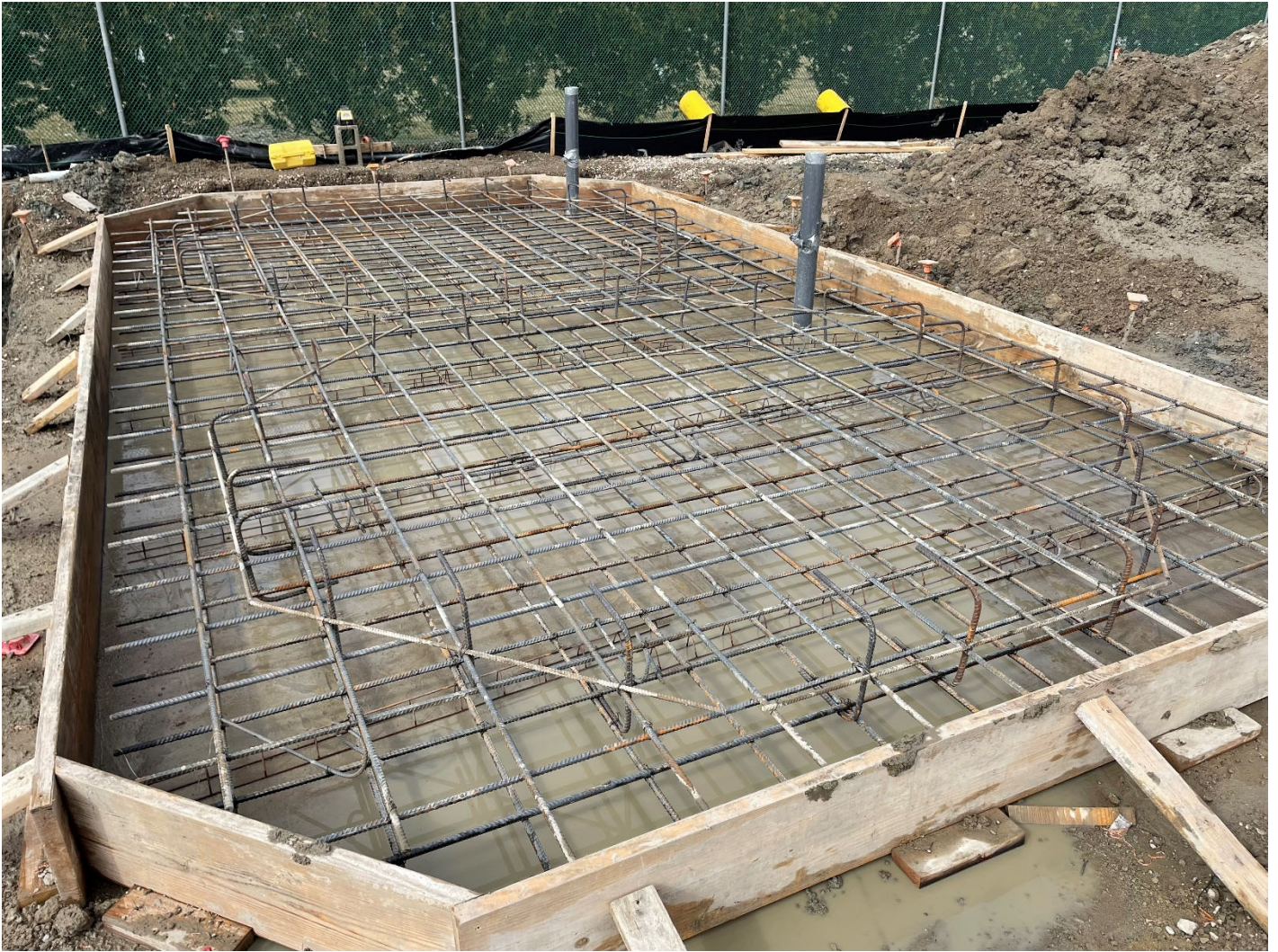
Figure 15 – Rebar for Tank Pad Foundation at NGI
