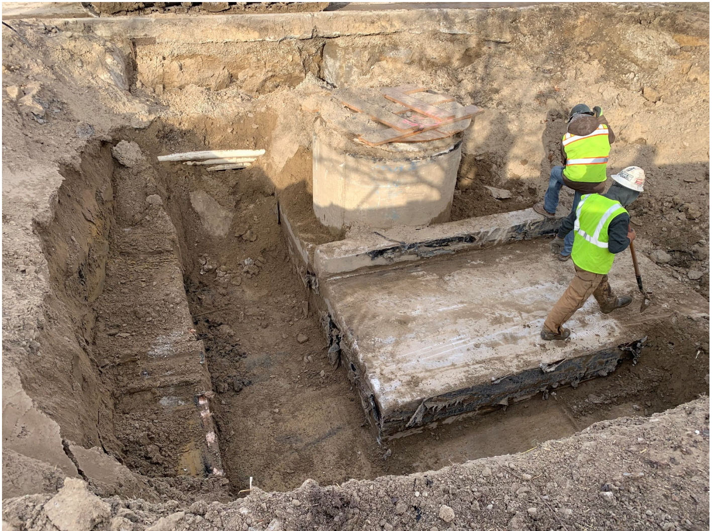
Figure 8 – Excavation to Expose CS-2
