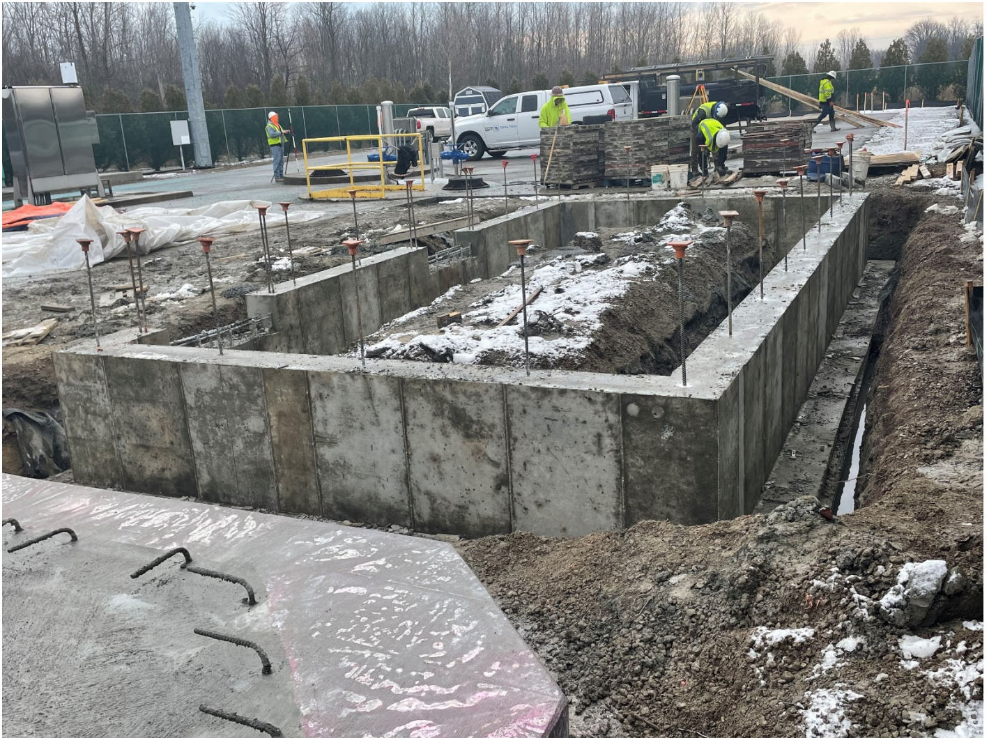
Figure 19 – NGI Building Foundation
