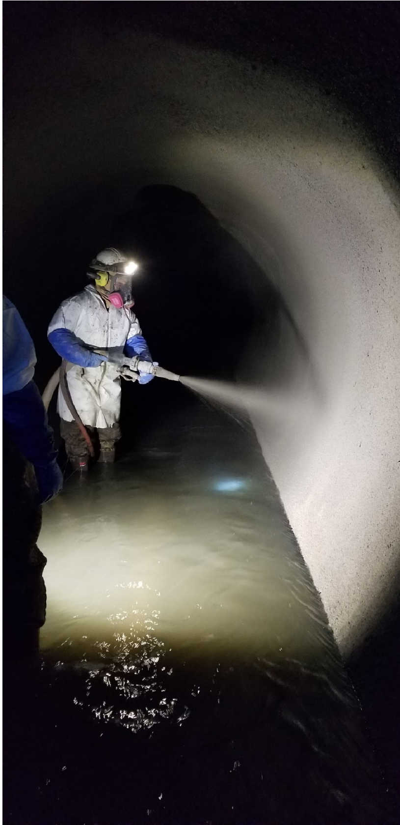
Figure 7 – Spray-Lining in the 8-foot Diameter section of Interceptor
