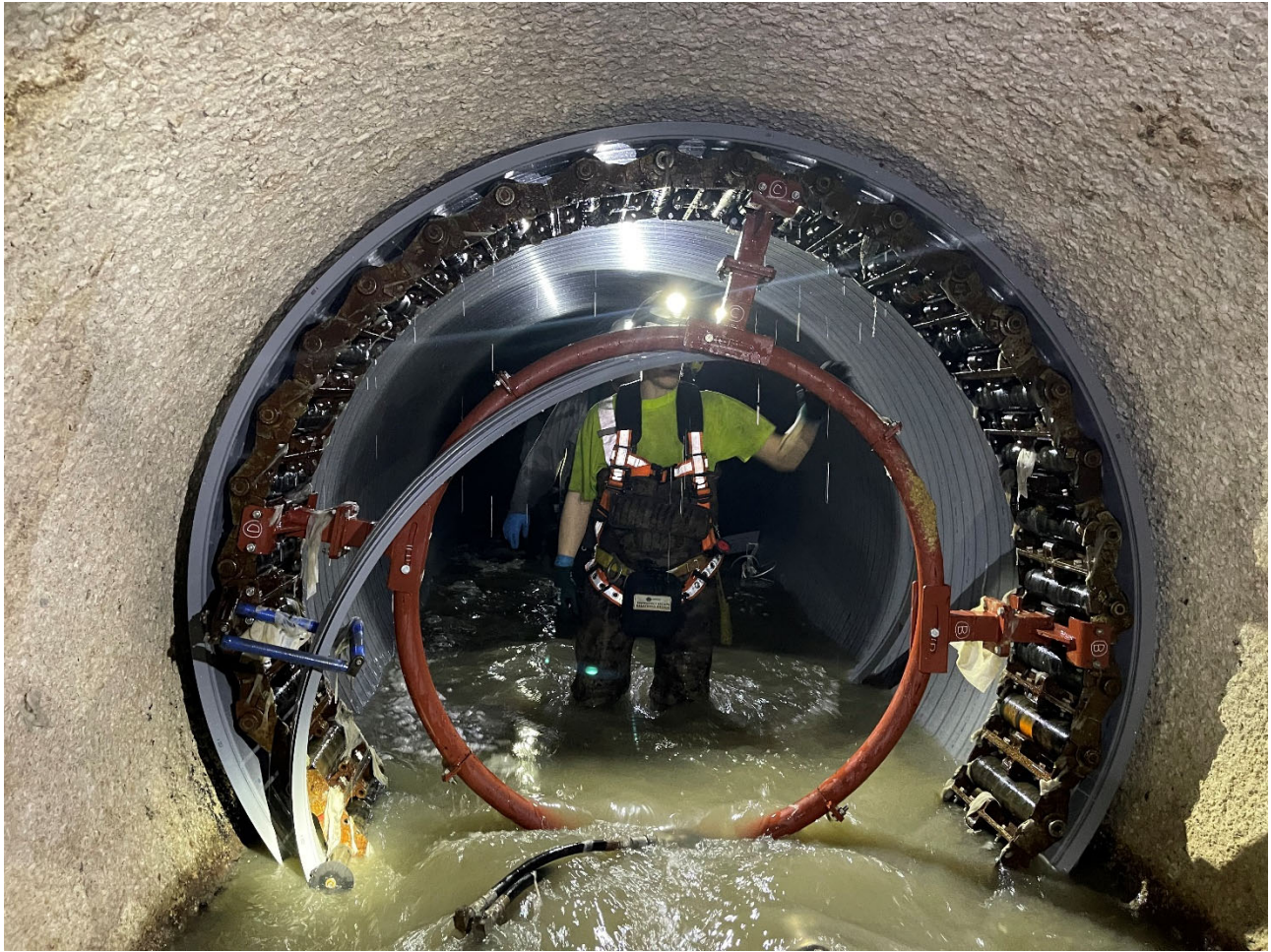
Figure 12 – Spiral Wound Lining Being Wound in the Pipe
