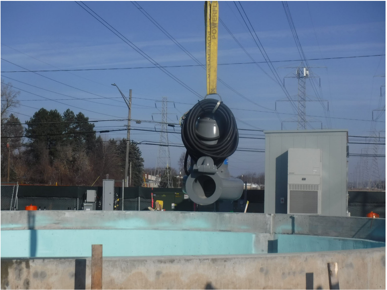
Figure 4 – Lowering in Pump for a Dry Fit at CS-12
