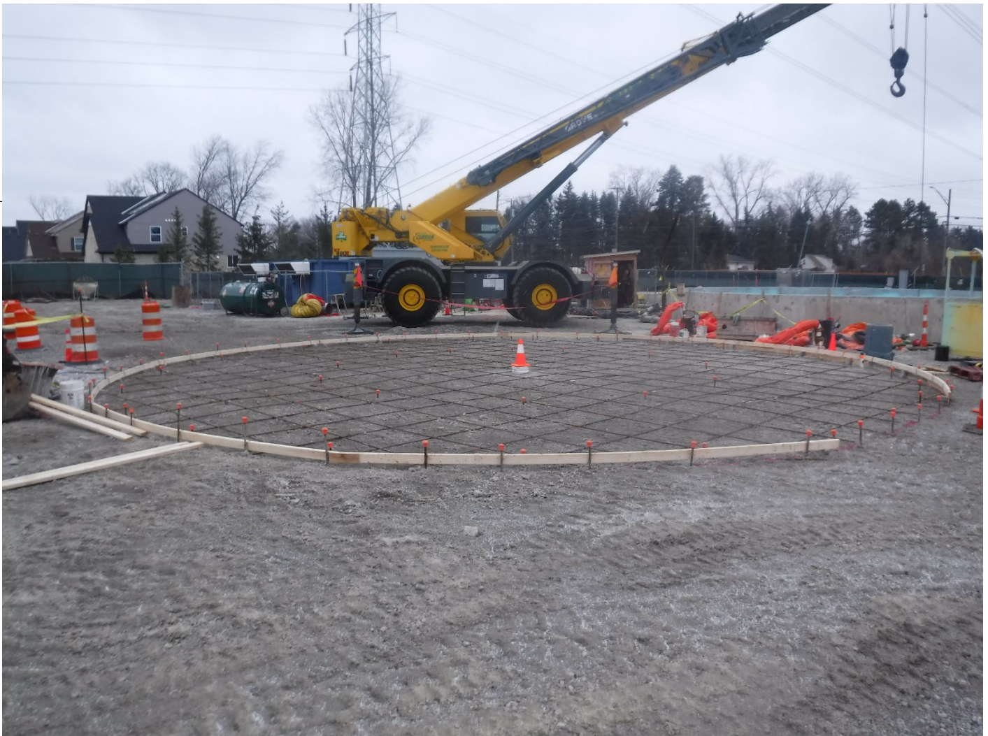
Figure 1 – Temporary Concrete Pad Prep at CS-12
