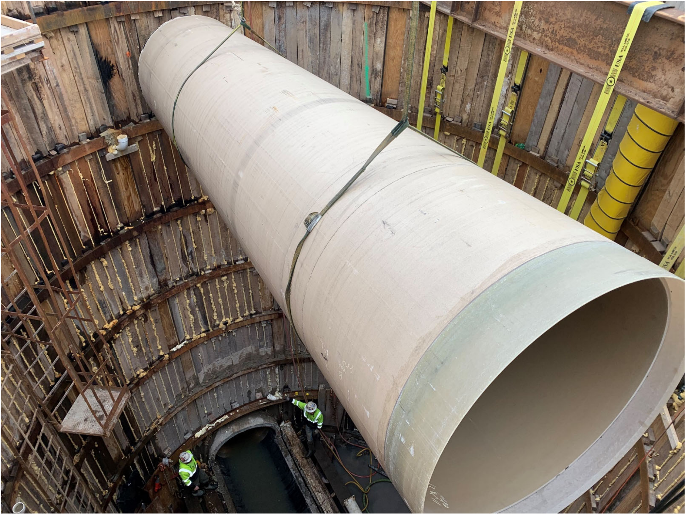
Figure 10 – Hoisting 5-foot diameter HOBAS into Access Shaft
