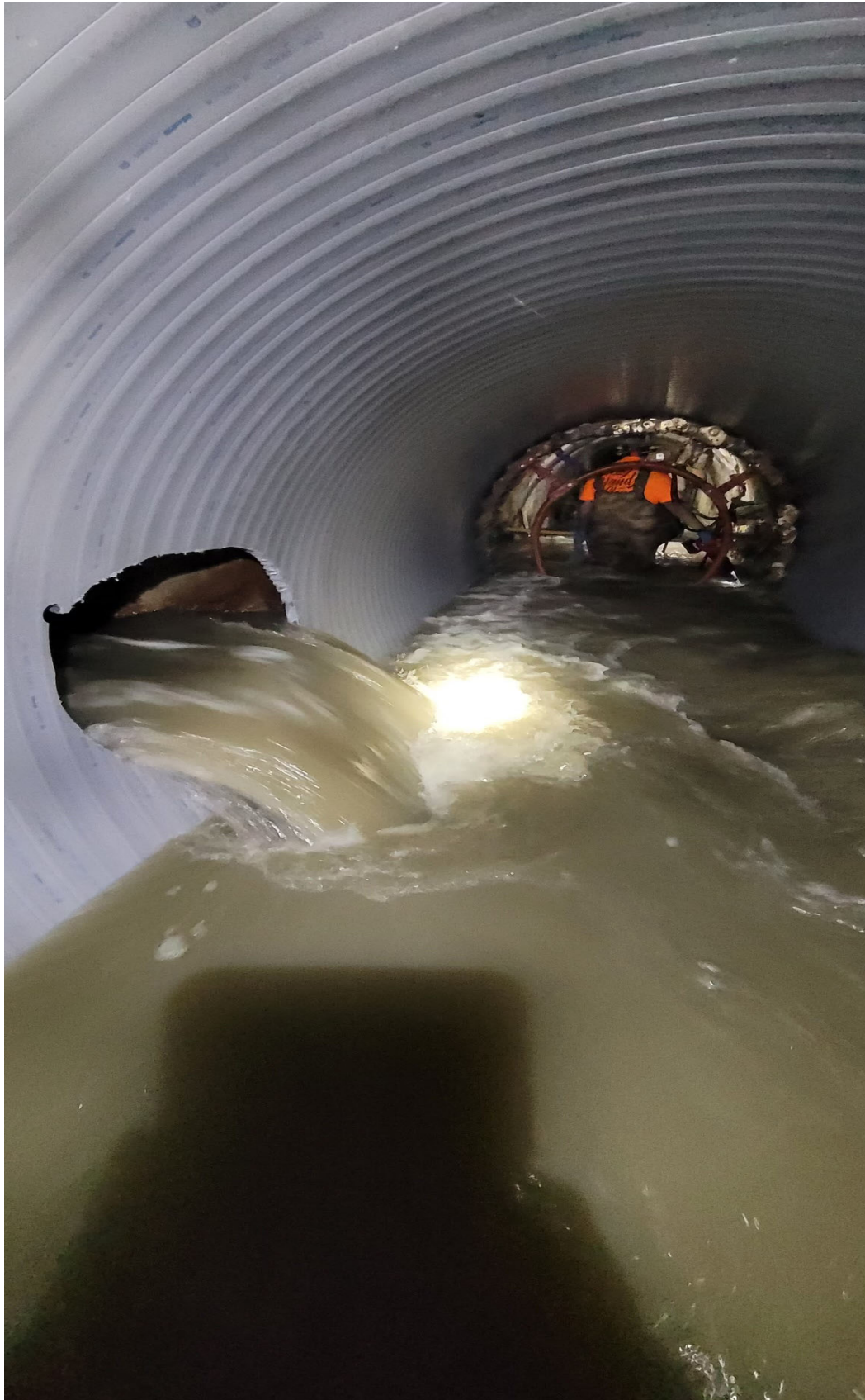
Figure 14 – Lining Past Final Community Tap
