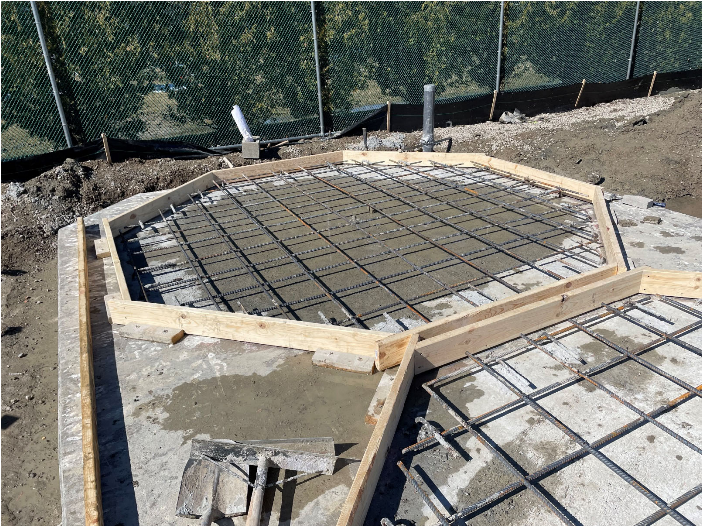
Figure 16 – Rebar for Tank Pads at NGI
