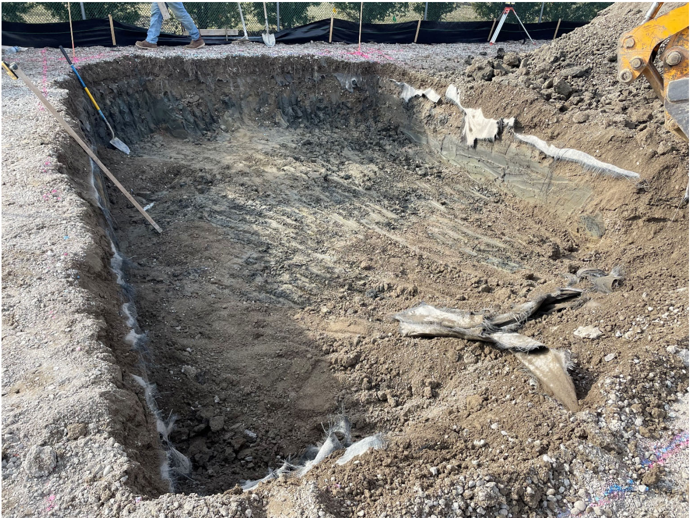
Figure 14 – Excavation for Tank Pad Foundation at NGI
