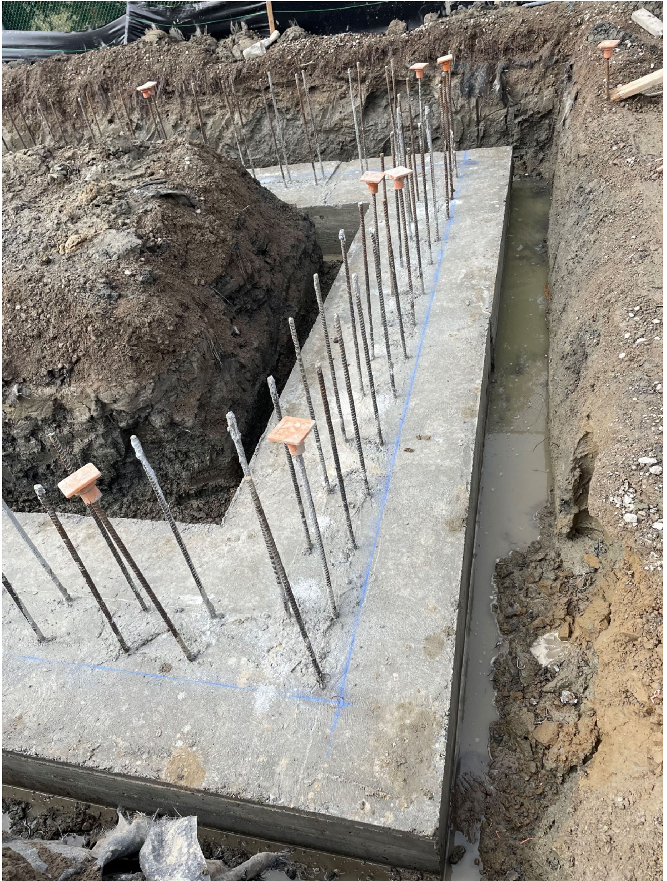
Figure 18 – NGI Building Foundation
