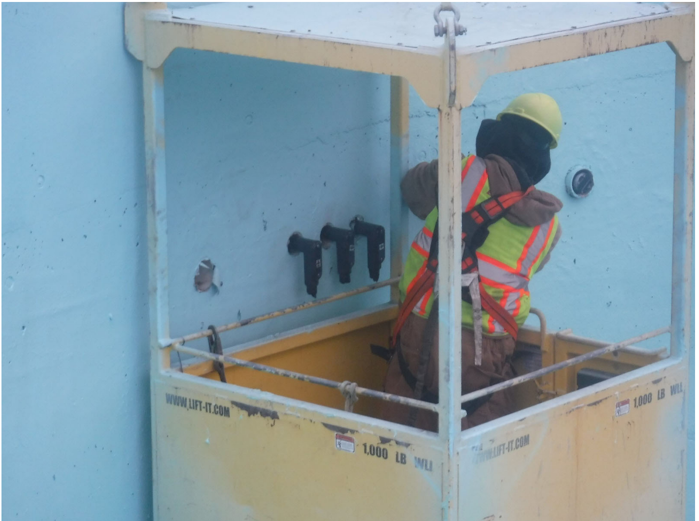
Figure 5 - CS-12 Electrical Conduit Installation
