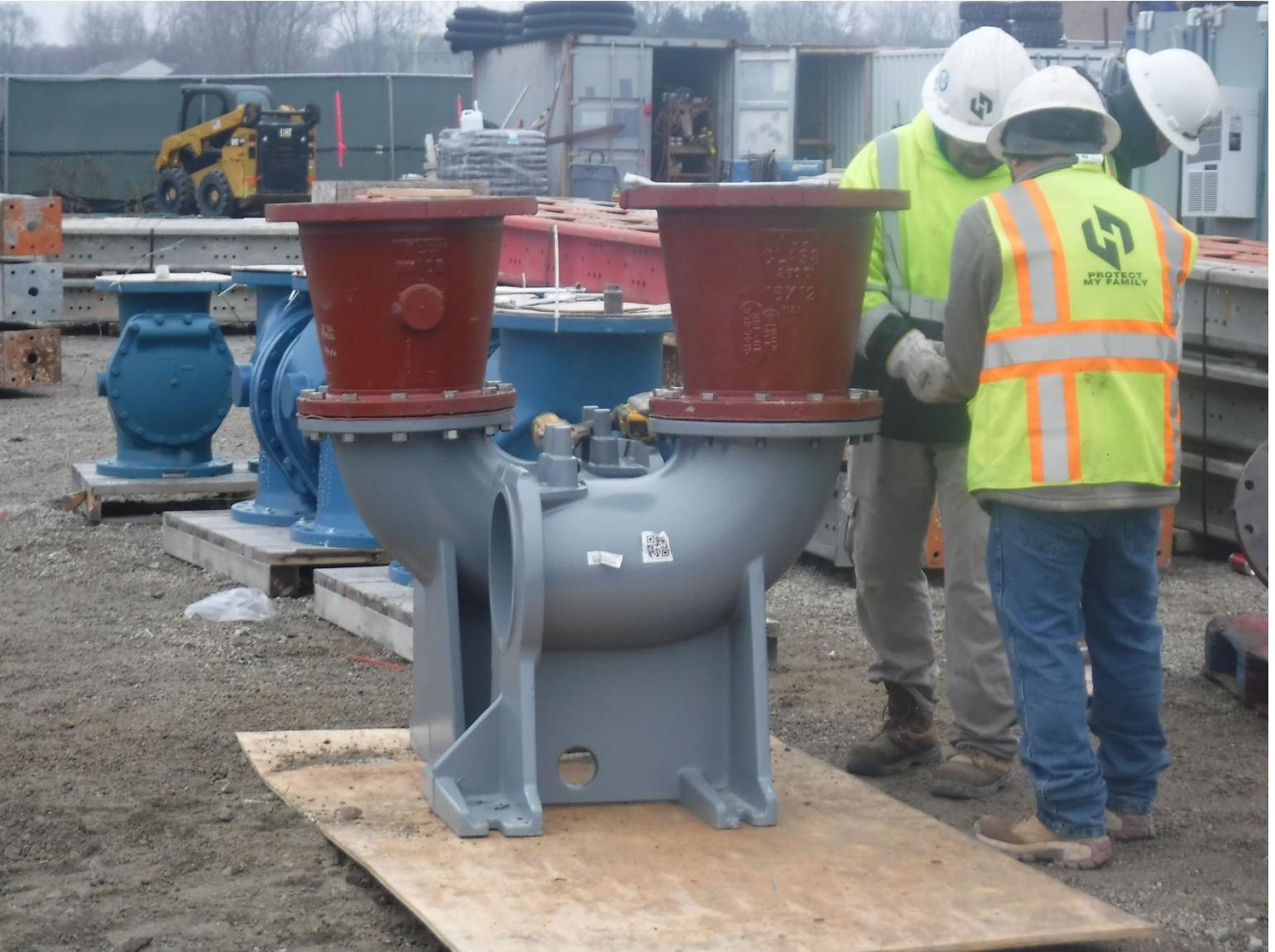
Figure 3 – Fitting Pipe at Grade
