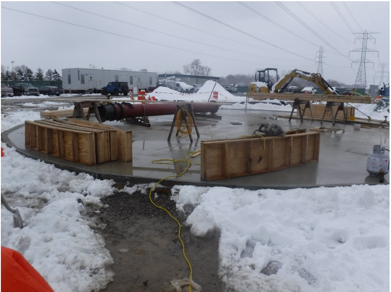
Figure 2 – Temporary Concrete Pad at CS-12
