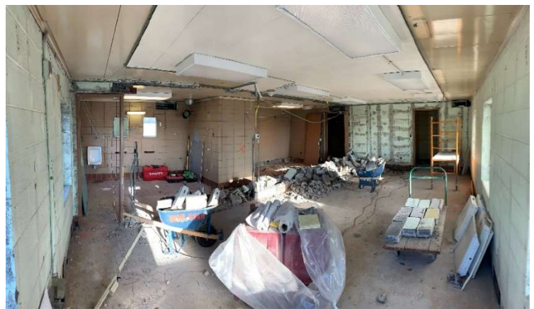
Figure 9 – Full demolition of Mezzanine level
