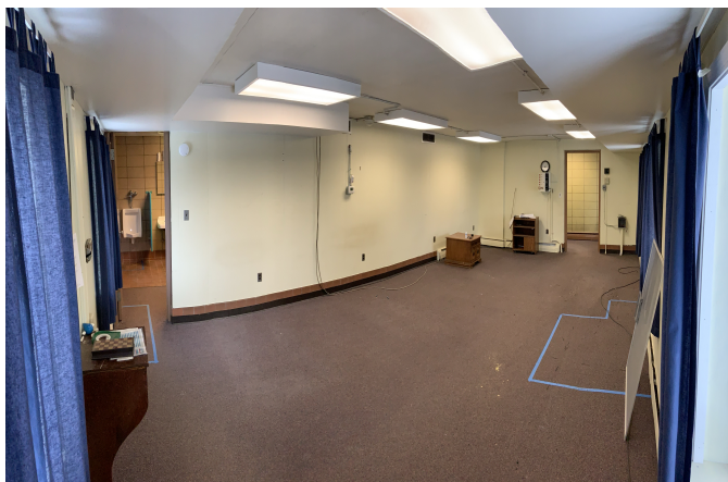
Figure 8 – Before demolition of Mezzanine level
