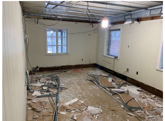
Figure 7 – Demolition of ex. office area on Mezzanine level
