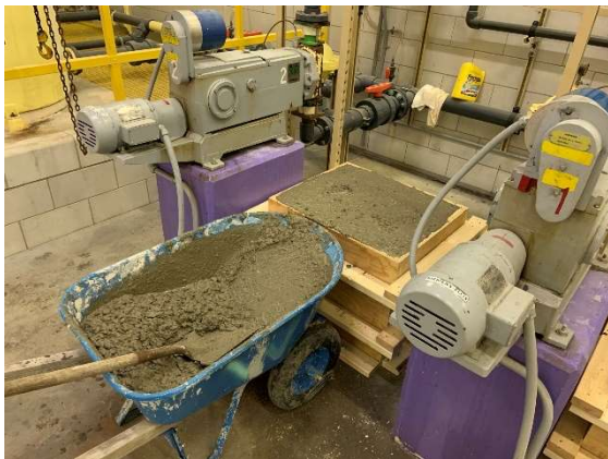
Figure 3 – New Pump Pads being poured at Martin
