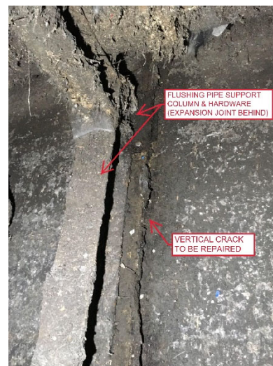
Figure 2 – Joint Repair Close-up
