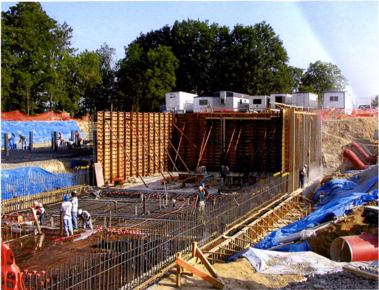
7/2/2002 8:39:12 AM - HPBS - Wall Construction - DC
