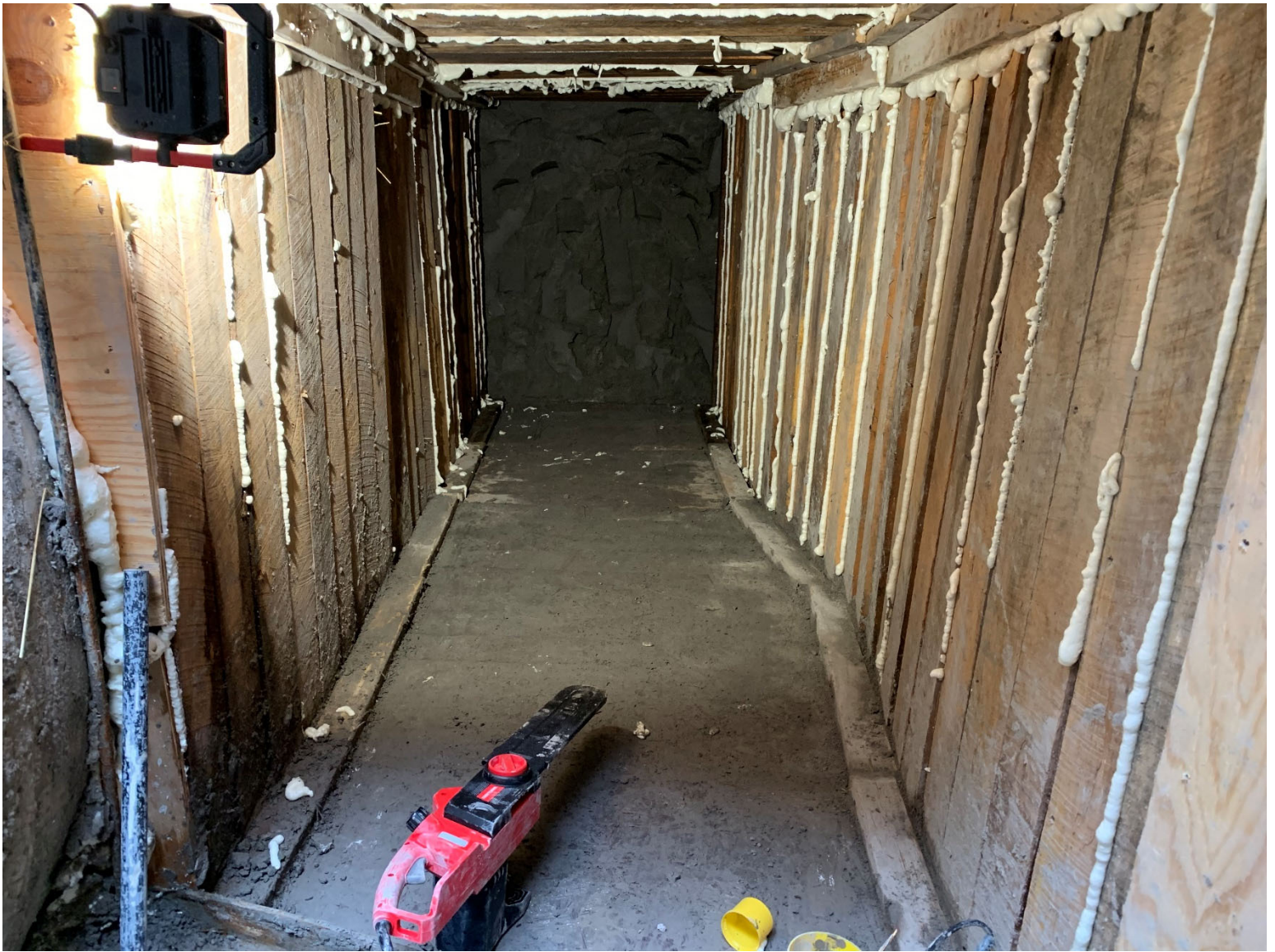
Figure 11 – Lining Completion Shaft Tail-Tunnel
