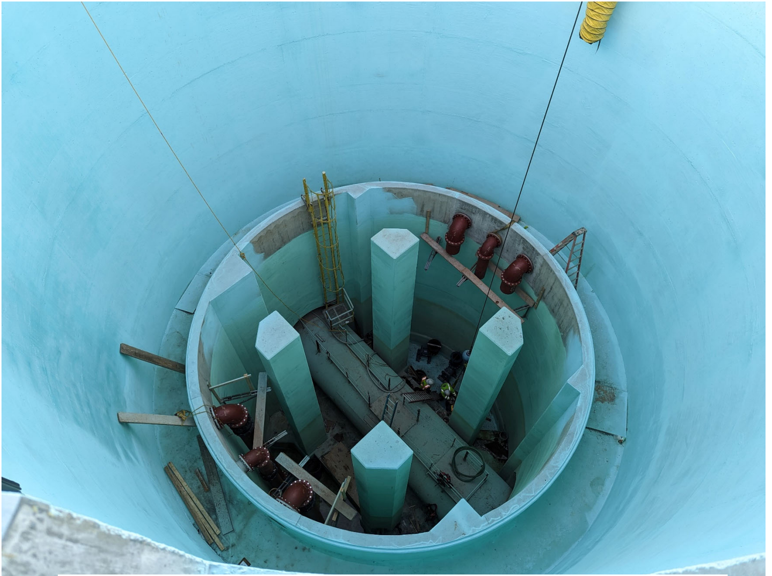
Figure 3 – CS-12 Pump & Pipe Installation
