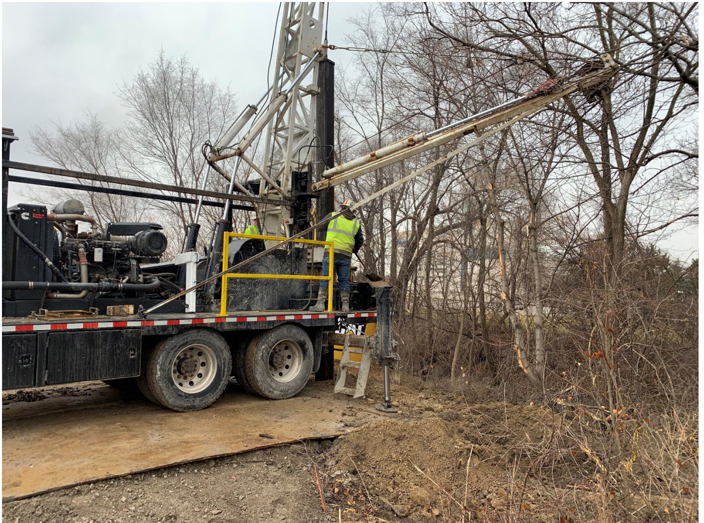
Figure 8 – Lining Completion – Drilling Dewatering Well
