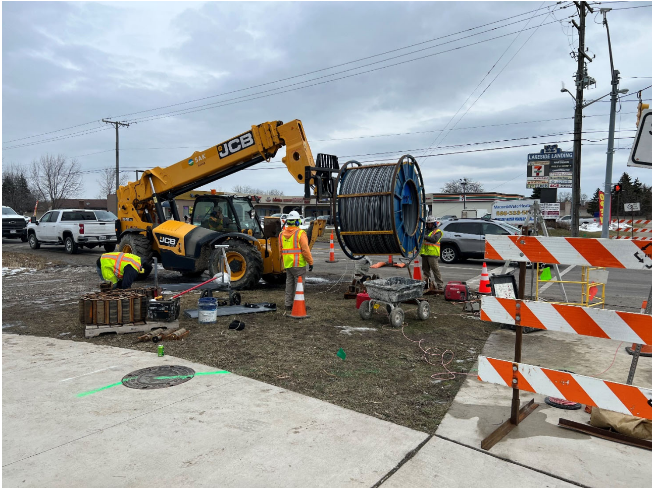
Figure 12 – Spiral Wound Lining Being Set in Place
