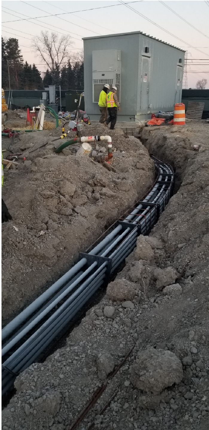
Figure 6 – CS-12 Electrical Conduit Duct-bank for Pumps
