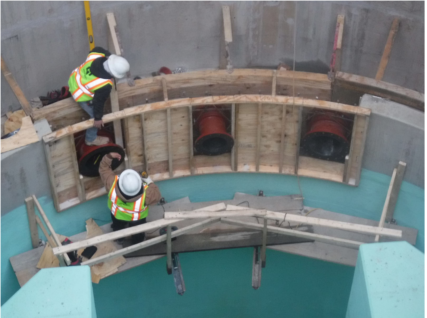
Figure 5 - CS-12 Flume Pipe Installation
