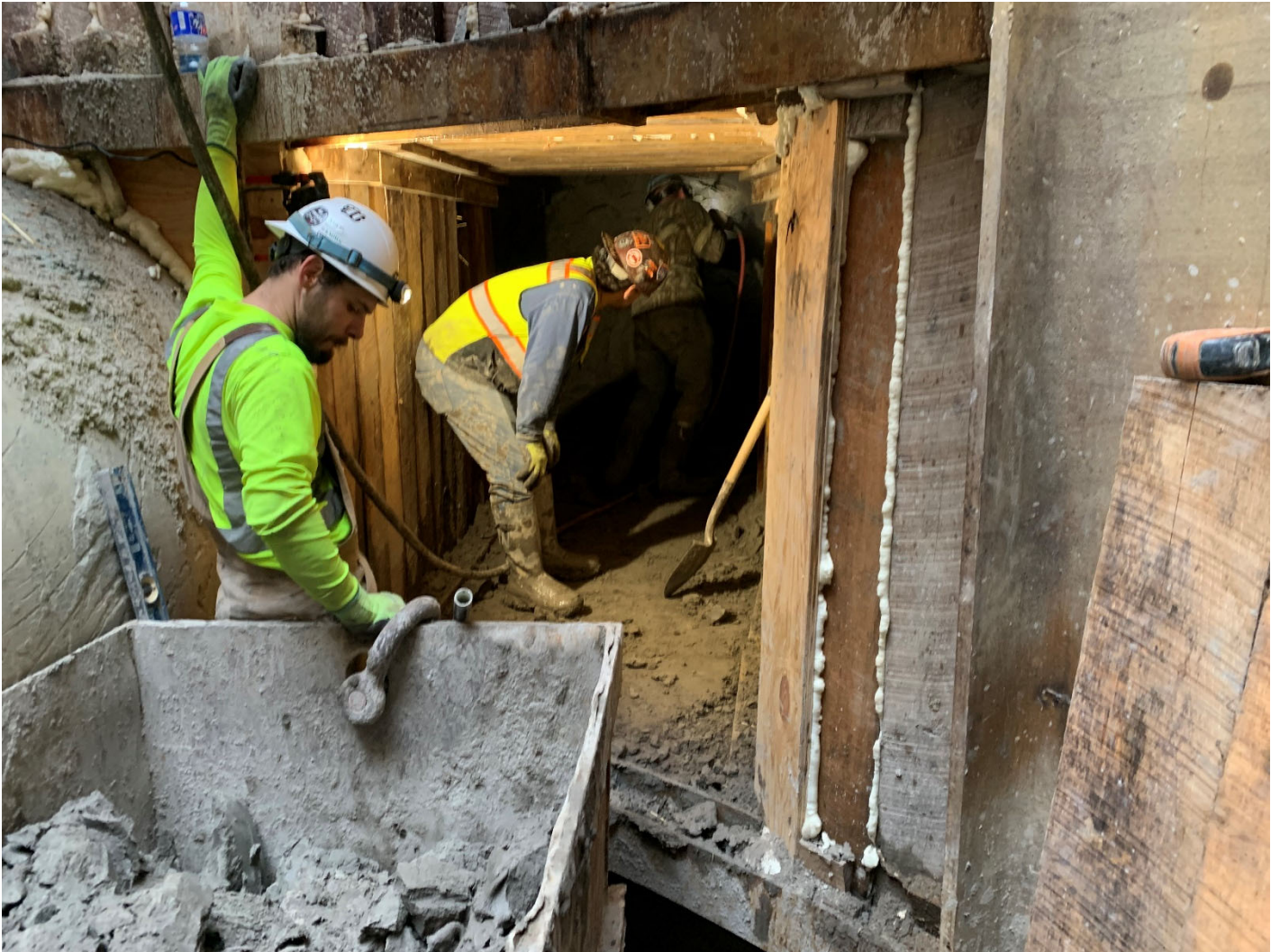
Figure 9 – Lining Completion Shaft – Tail-Tunnel Excavation
