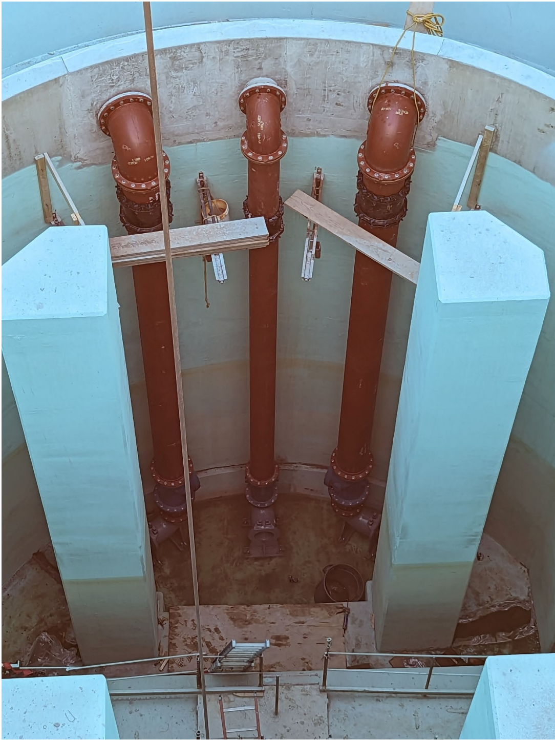
Figure 4 - CS-12 Pump & Piping Installation
