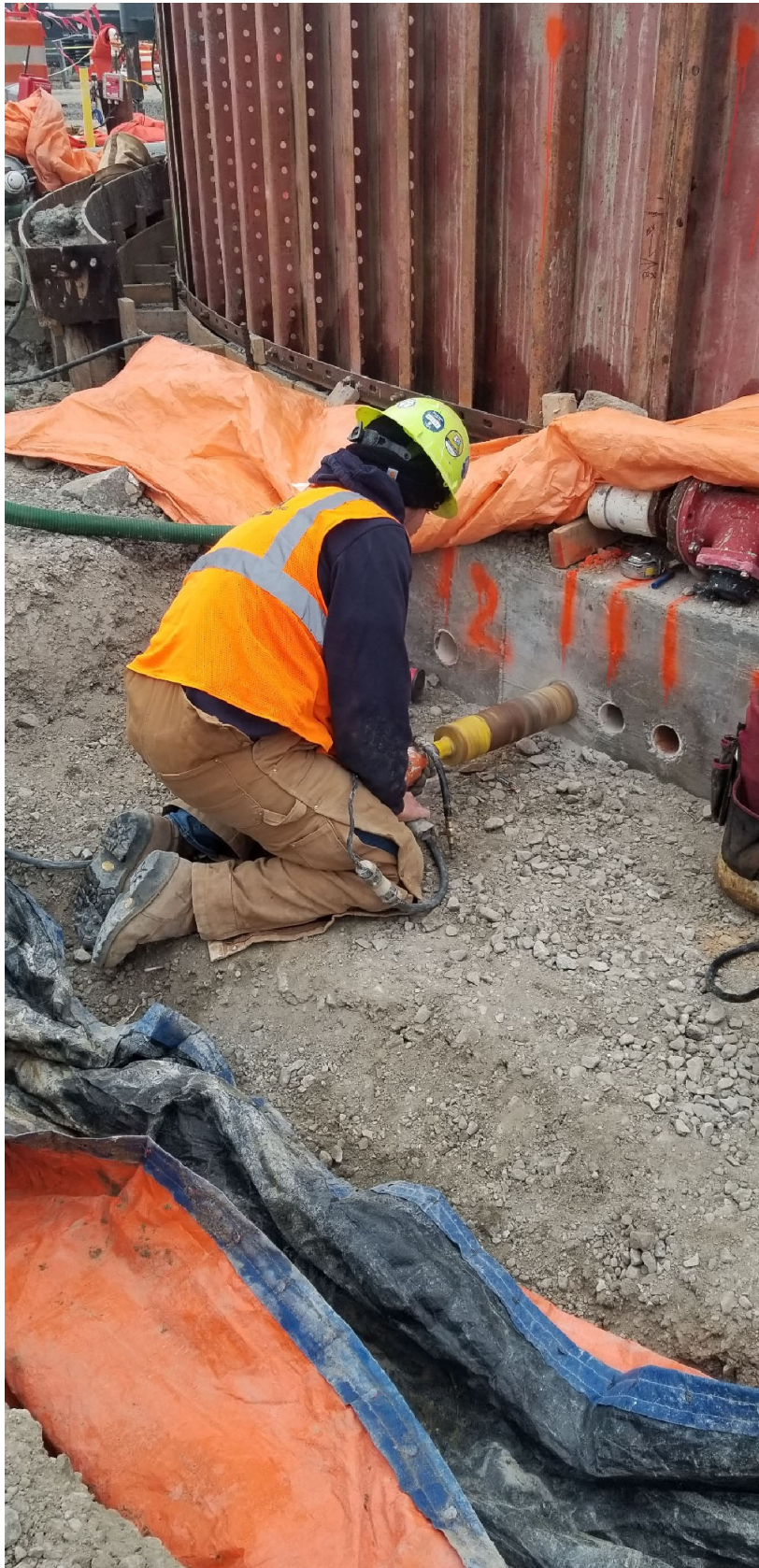
Figure 7 – CS-12 Coring Holes for Electrical Conduit
