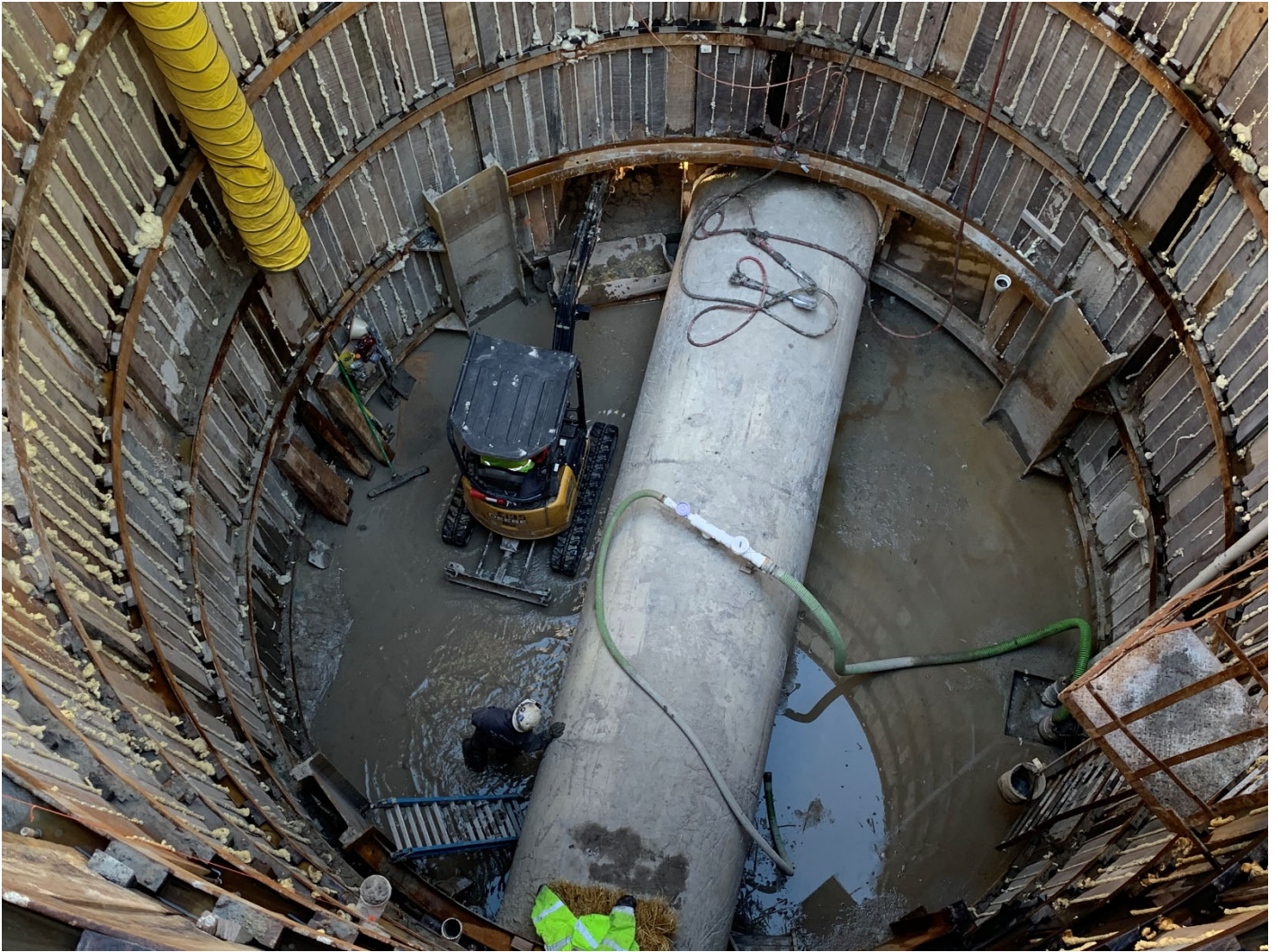
Figure 10 – Lining Completion Shaft – Tail-Tunnel Excavation
