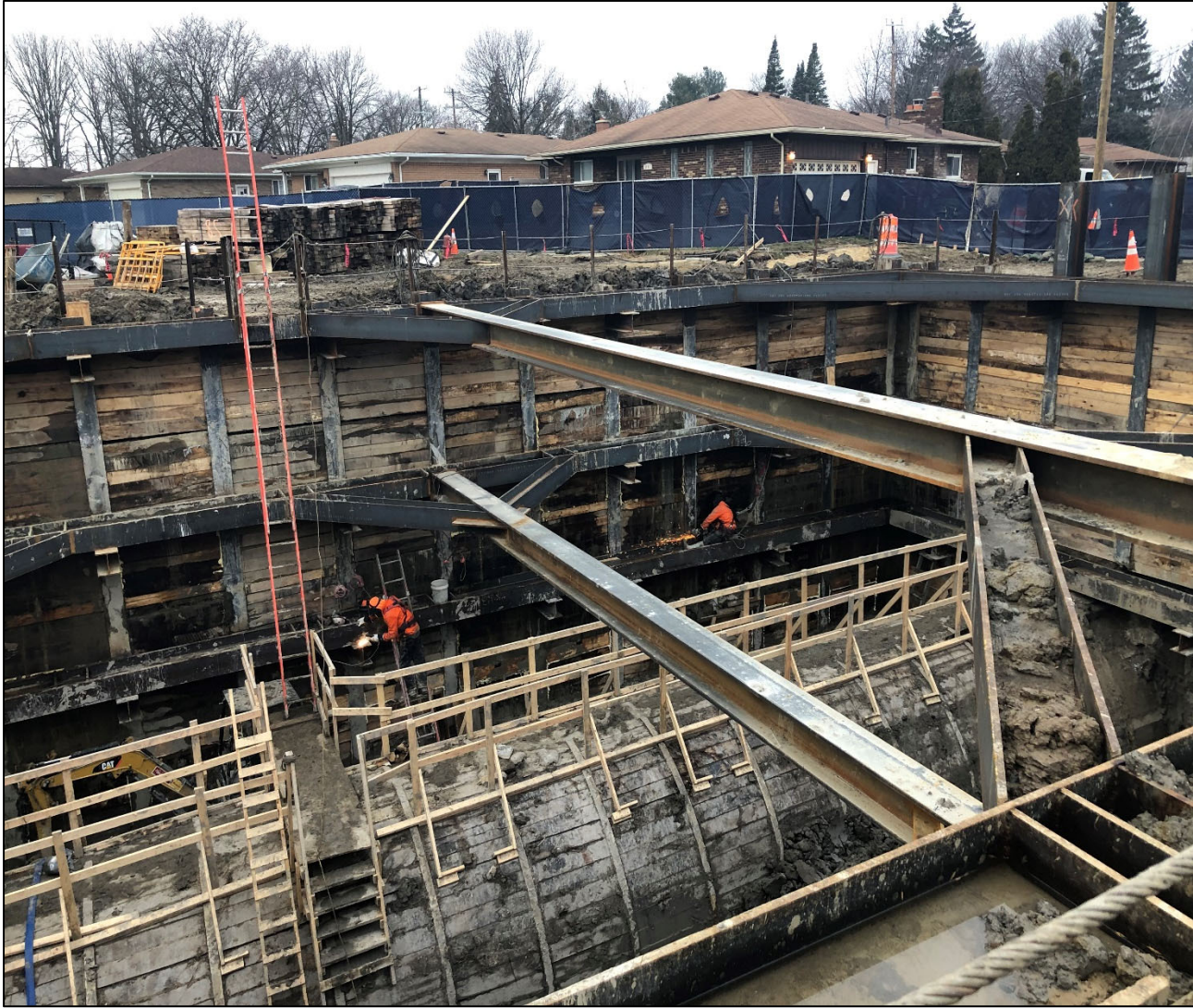
Figure 3 – Welding Lower Tier Shaft Bracing
