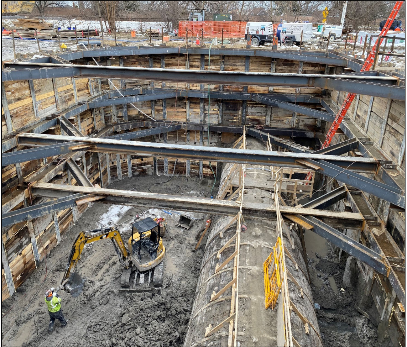
Figure 5 – Excavated Approx. 30FT Facing East
