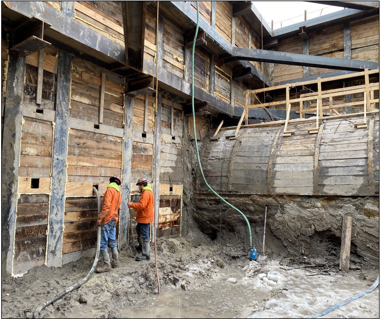
Figure 2 – Pumping Grout to fill Voids
