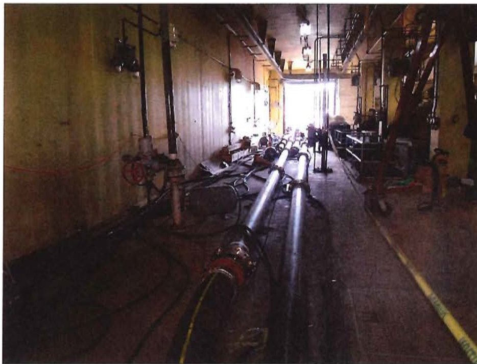
Distance from bar rack to building exit.
