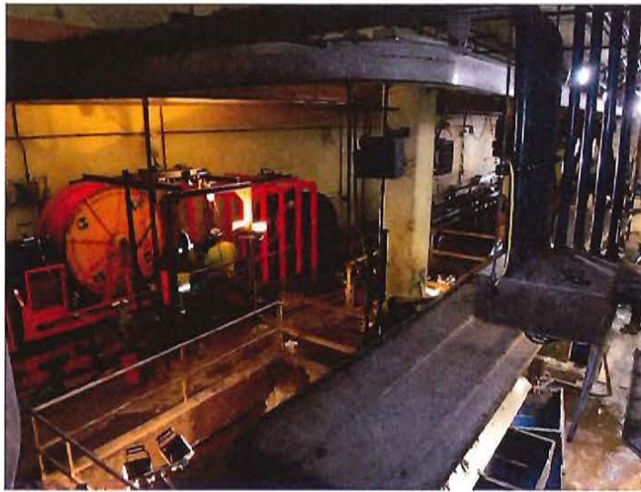
Remote reels at the bar screen
