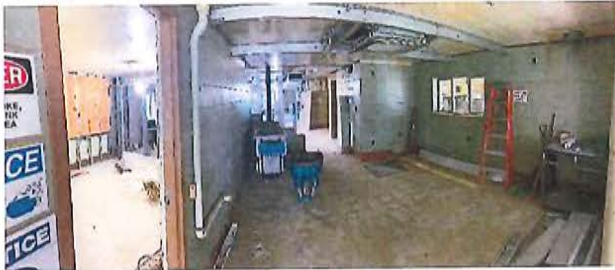
Figure 4a – Demolished old lab – SCADA Room
