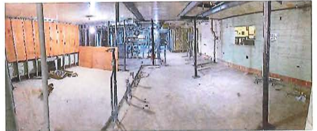
Figure 4b – Demolished remainder of interior walls – SCADA Room
