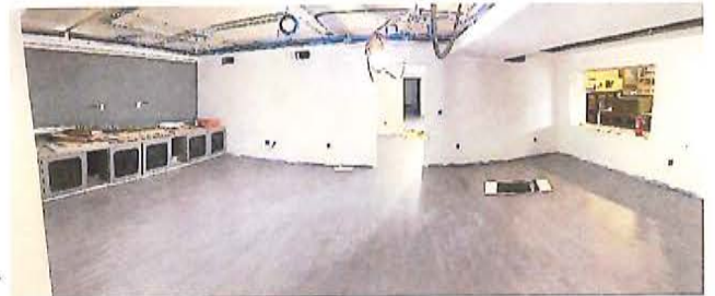
Figure 4d – Installed new drywall and flooring – SCADA Room
