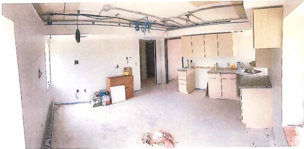
Figure 5 – New cabinetry – Kitchen Area
