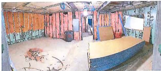
Figure 4c – Installed new studs, insulation – SCADA Room
