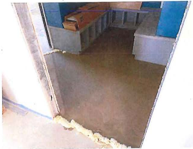
Figure 6 – Installed self-levelling compound on floors - Locker Room
